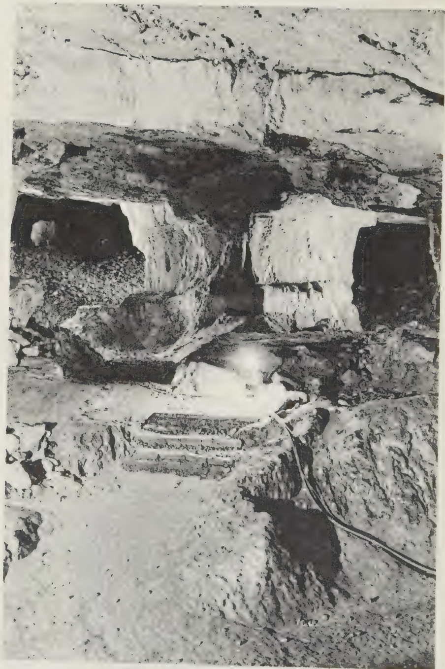
INTERIOR OF ZEDEKIAH'S GROTTA SHOWING ROOF SUPPORTING COLUMNS
