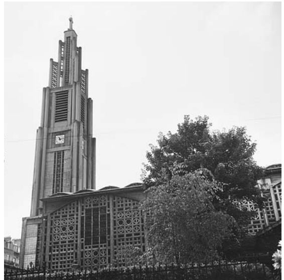
Notre-Dame du Raincy, c. 1911. This is the first architectural expression of the modern liturgical movement in France. (Le Raincy, France) (Photo by Roger-Viollet Collection/Getty Images)
