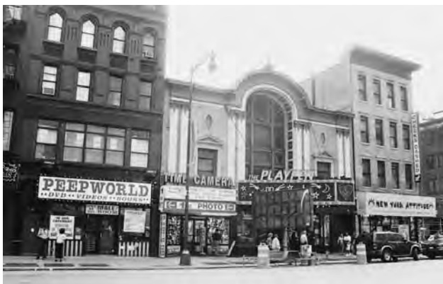
The way 8th Avenue north of 42nd Street looked in 2001 as Disney and friends were redoing the theatre district a few blocks south. Photograph by Richard Schechner.
