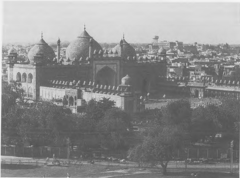
141 Agra, Jami c Masjid, 1058/1648, seen from the Hathi Pol of the fort; the eastern courtyard wing was demolished by the British during the Indian Mutiny in 1857. (Photo 1979)
