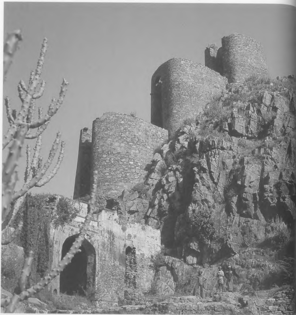
X Ajmer, Chashma-i Nur, completed 1024/1615. (Photo 1982)
