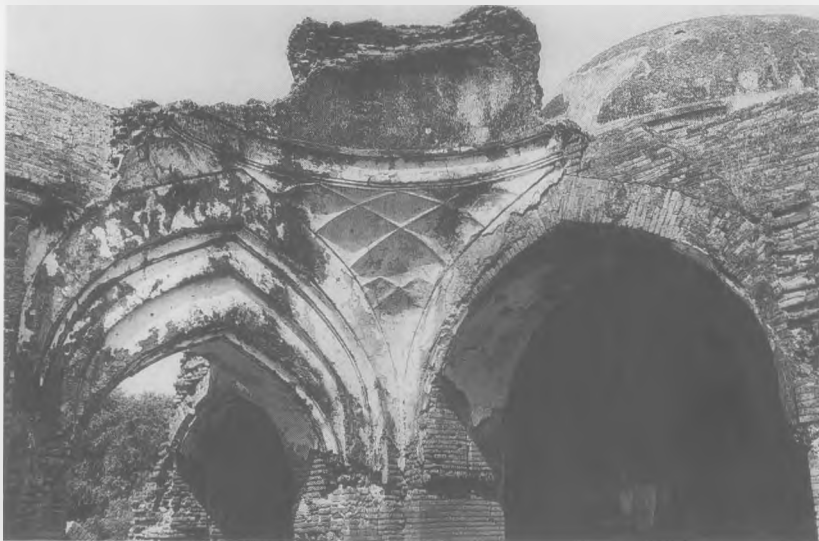
1 Panipat, Kal Bagh Masjid, some wing of the prayer-hall, ruined bay with arch-netting and pendentives in pseudostructural plaster relief-work (Photo 1982)
