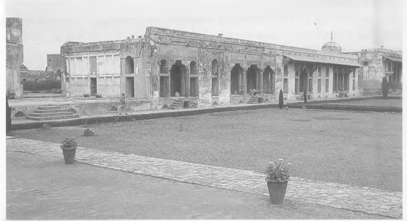
44 Lahore fort, Jahangir's Quadrangle, completed 1620, west wing. (Photo 1979)
