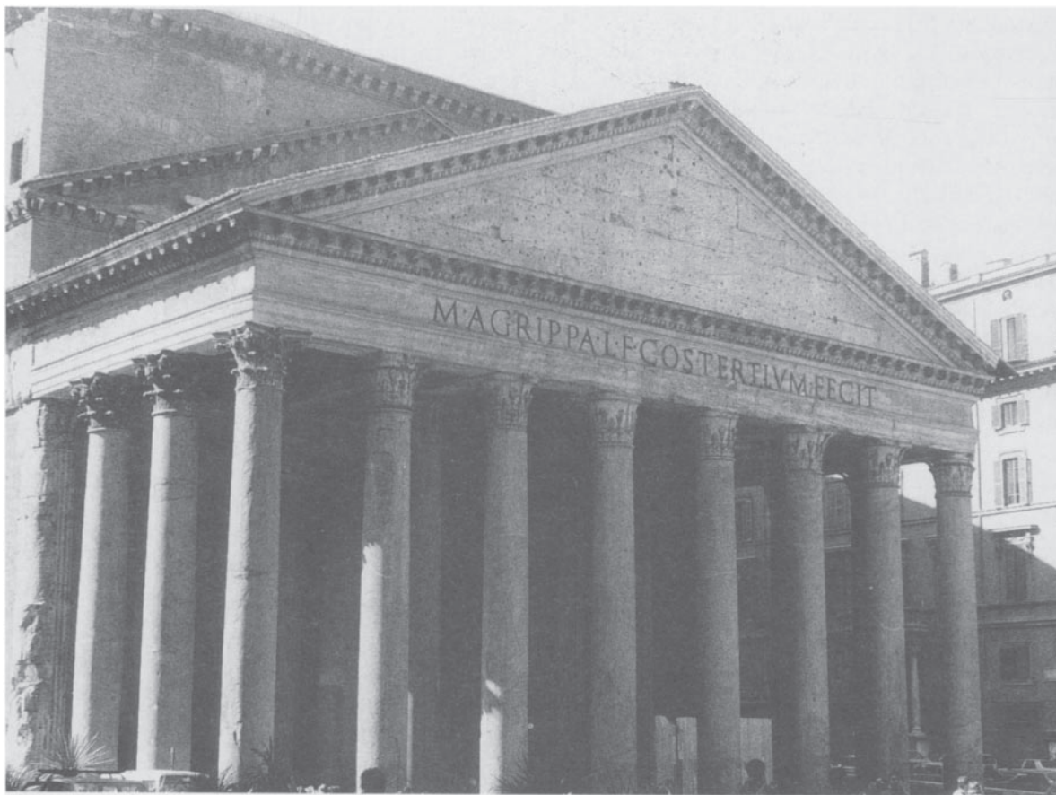
6 Pantheon, Campus Martius , Rome. 27–25 BC, but completely rebuilt under Hadrian.
