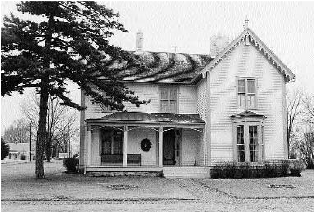
Figure 5. The T-shaped house became popular in the late nineteenth century; it retained the interior spaces of traditional houses but presented to the public a facade decorated with the “carpenter Gothic” ornament of the day (birthplace of World War I Allied forces Gen. John J. Pershing, Laclede, Linn County, Missouri).
