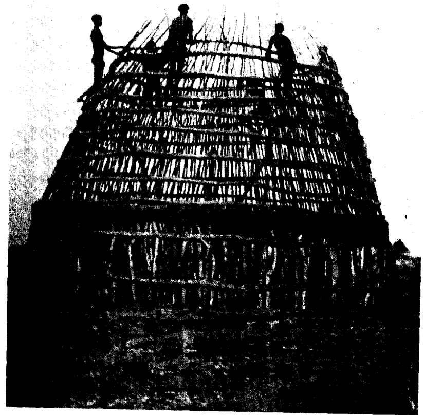
Building a cattle byre (Eastern Jikany)
