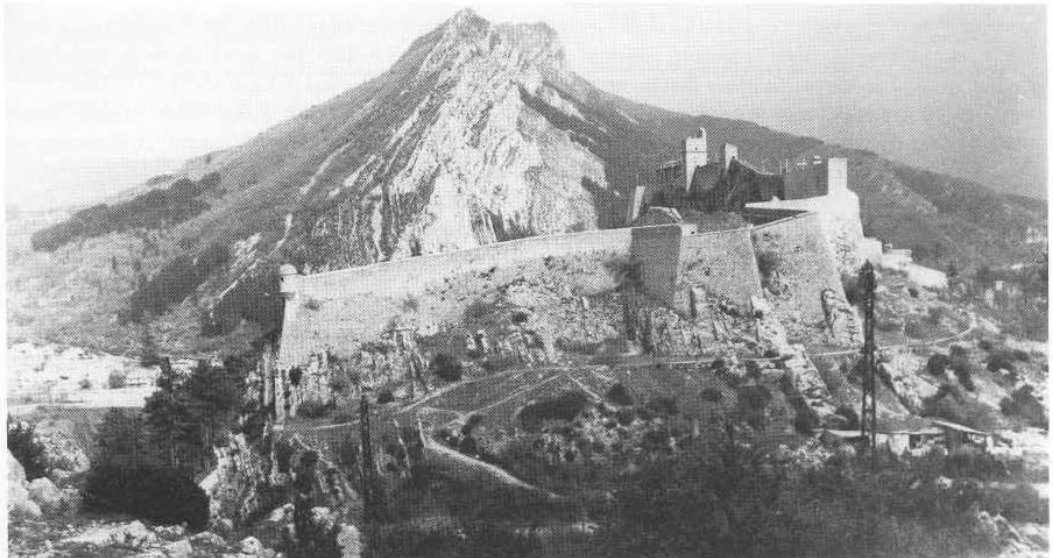
49 Sisteron. The plug-like limestone rock of Sisteron is sited at a point where the valley of the Durance narrows between tall hills. It therefore commanded an important avenue between Provence and Dauphiné. The rock was originally fortified in 1597 by Jean Errard de Bar-le-Duc, and drastic measures were taken to protect the interior from fire from the outlying heights – most notable is the tall arcaded screen wall to the right of the photograph. Vauban re-made some of the works after the Piedmontese incursion down the Durance in 1692
