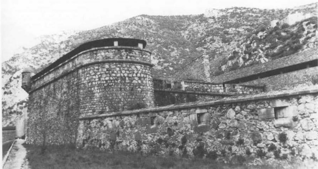
53 Bastion at Villefranche-de-Conflent. Here the rampart is protected by a heavy timber gallery
