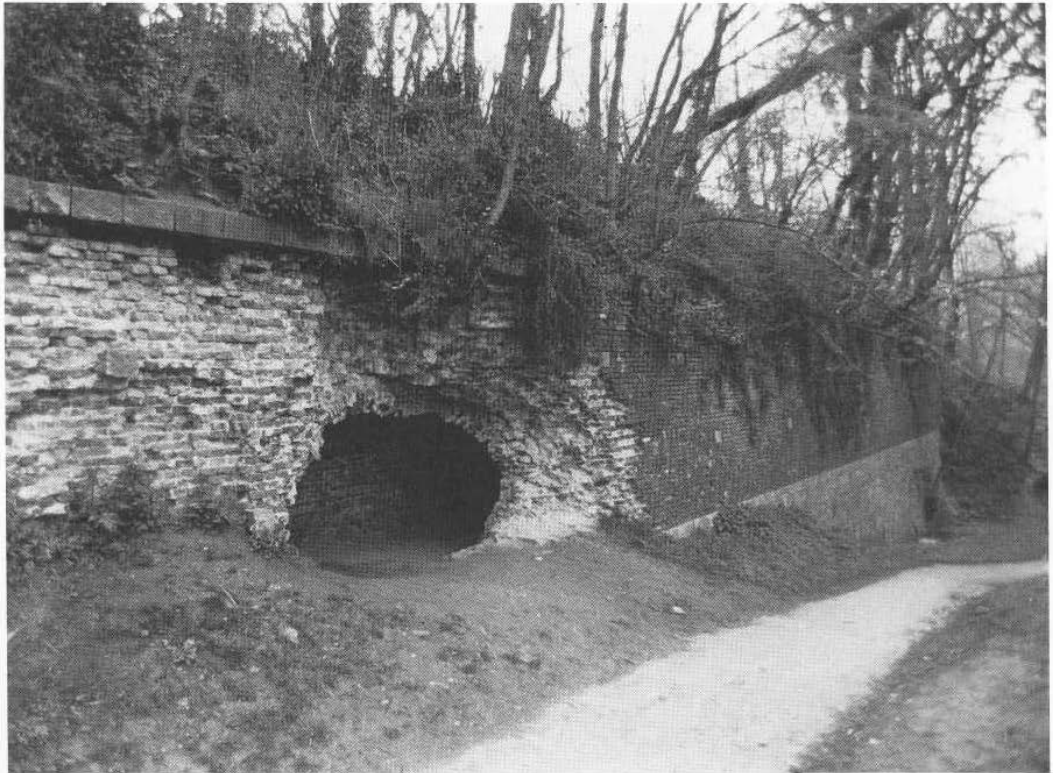
45 Countermining gallery, ravelin at Le Quesnoy. Revealed by tree-damage at this sadly neglected fortress
