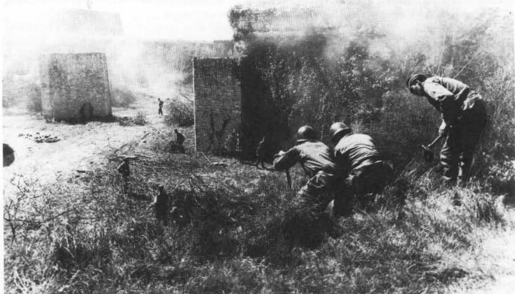
154 Modern French engineer troops clearing vegetation at Blaye. An expression of the current world-wide interest in the restoring of artillery fortifications
