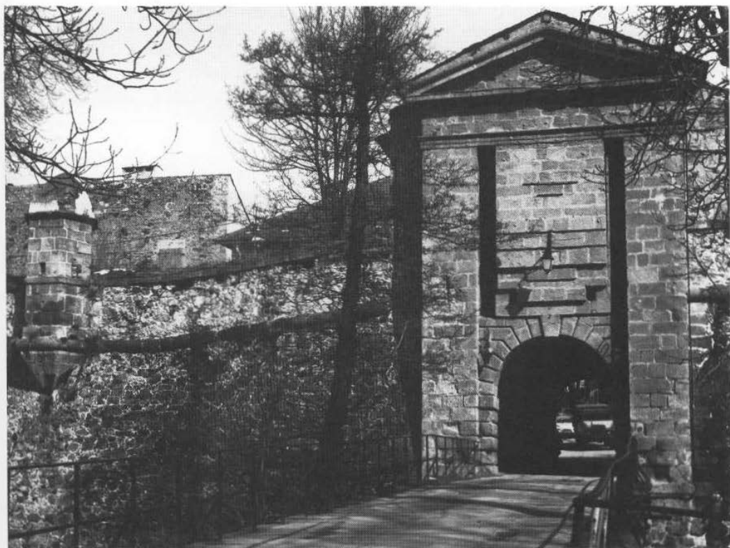
67 Hornwork gate, Mont-Louis
