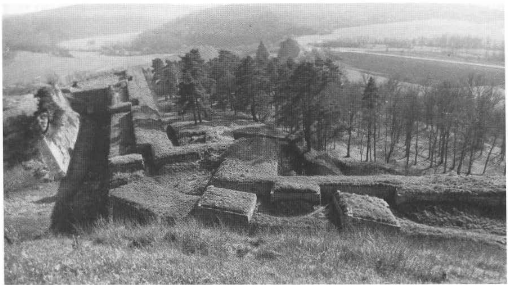
7 Covered way with multiple traverses (Montmédy Citadel). A small re-entrant place of arms is at the left centre
