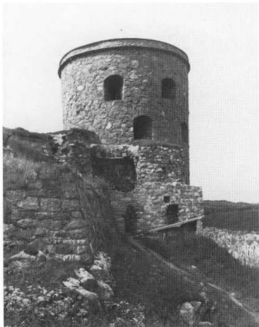
117 The Fars Hatt Tower, Bohus Castle. A four storeyed-work, built by Dahlberg to replace a small medieval tower badly damaged in the siege of 1678
