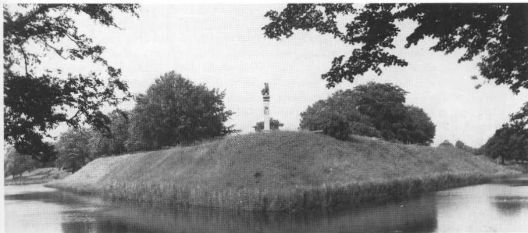
120 The Landskrona Bastion, Landskrona Citadel. Part of the earthen perimeter built by the Swedes in the 1660s and 1670s
