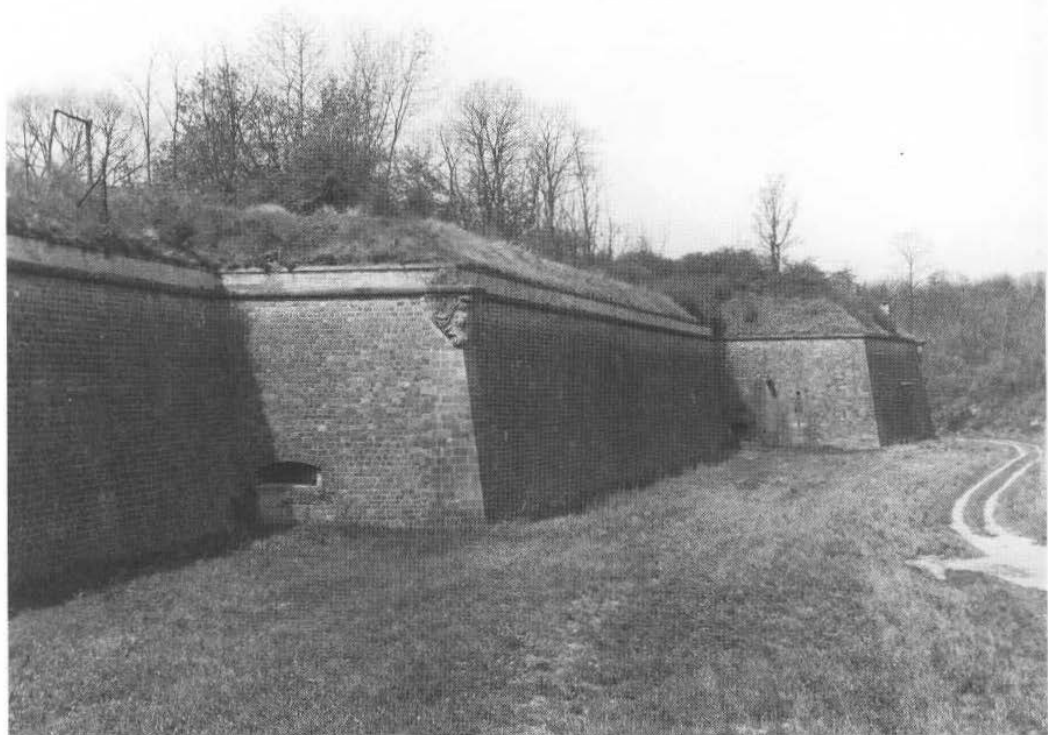
57 Rampart at Neuf-Brisach, showing (left to right) the recessed curtain, bastion flank and face, and the bastion tower (with blocked-up embrasures)
