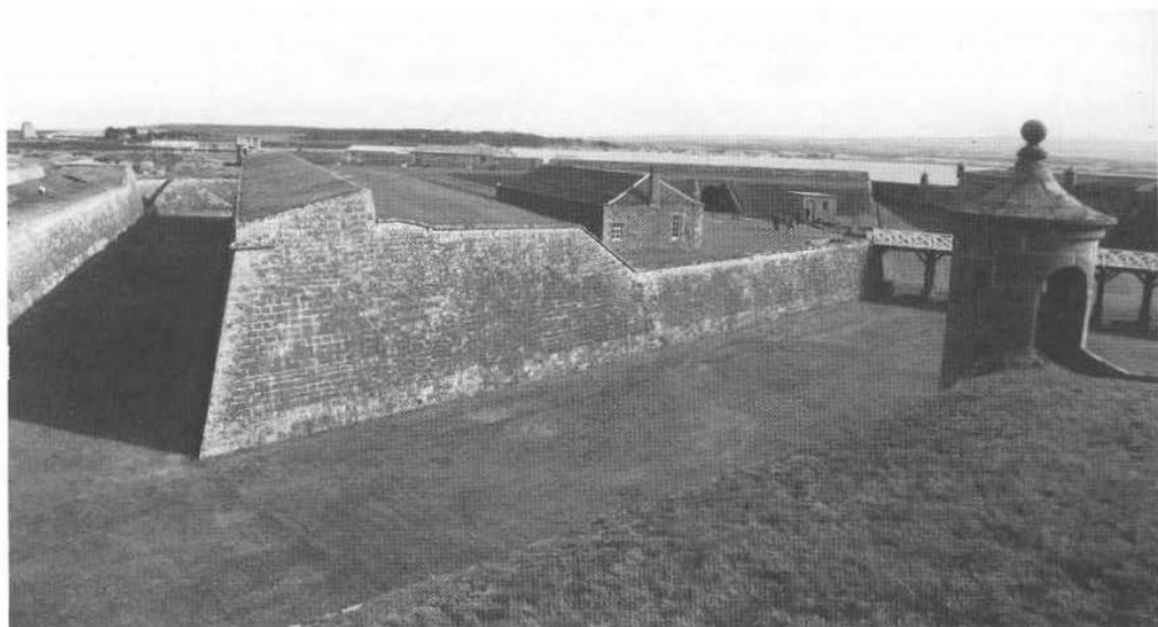
105 Fort George, Inverness. Designed by William Skinner in 1747 to secure the inner reaches of the Moray Firth after the '45. One of the very rare examples of eighteenth-century bastioned fortification on the British mainland
