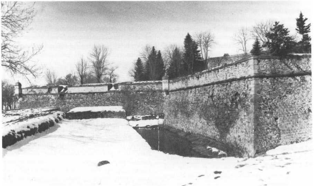
6 View down a covered way to a snow-topped traverse (Mont-Louis). The covered way is commanded by a ravelin (right), and by the embrasures of the bastion face beyond
