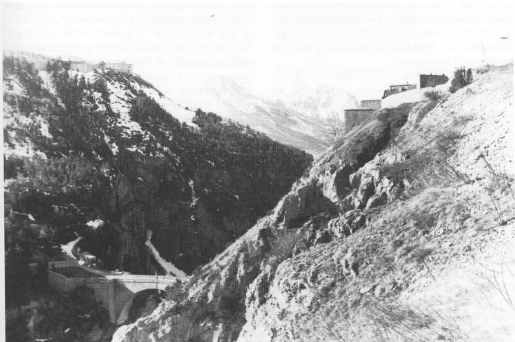
93 The Durance gorge at Briançon, with the Pont d'Asfeld. Briançon town to the right, Fort de Randouillet to the left
