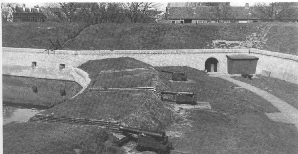
38 Double retired bastion flank at Naarden, showing guns emplaced in lower storey
