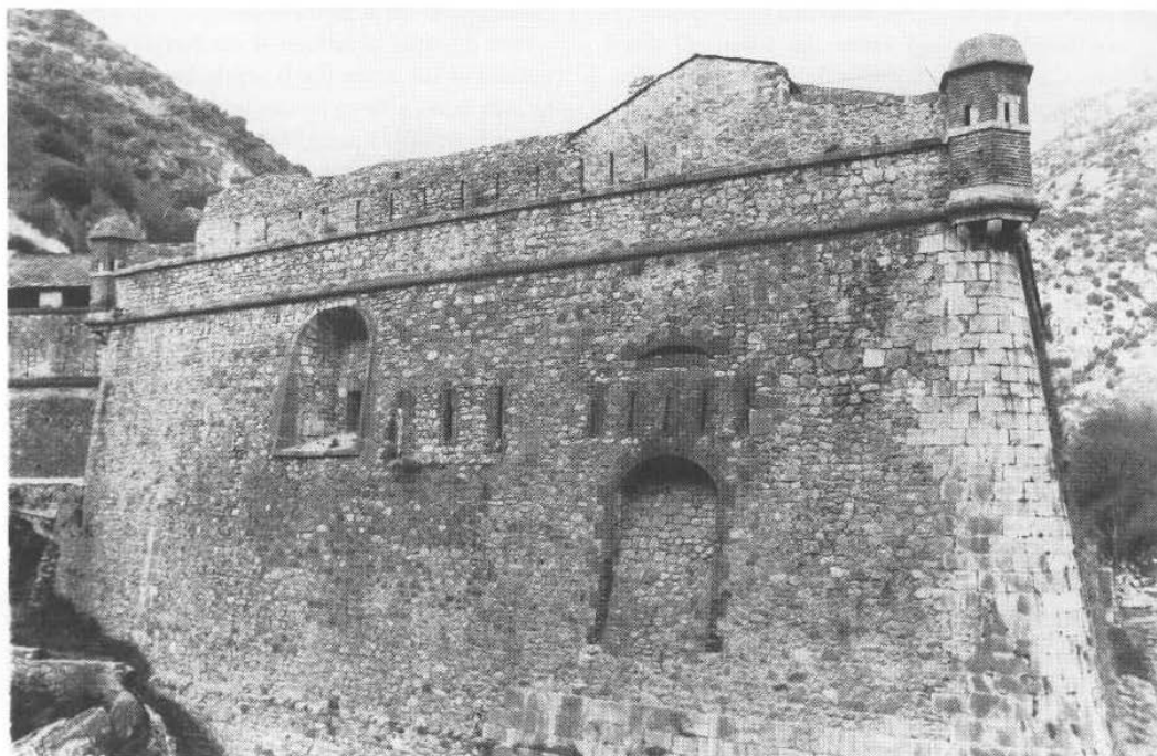
52 Villefranche-de-Conflent, Bastion du Dauphin. This little fortress in the eastern Pyrenees shows how Vauban solved the problems presented by a narrow site overlooked by mountains. Here we see a loopholed and casemated bastion which offered good protection against Spanish miquelet snipers
