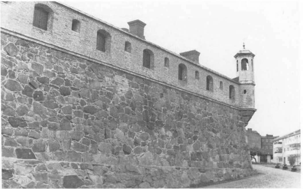
114 The Aurora Bastion, Karlskrona. Part of the redoubt which closes up the eastern end of the dockyard wall
