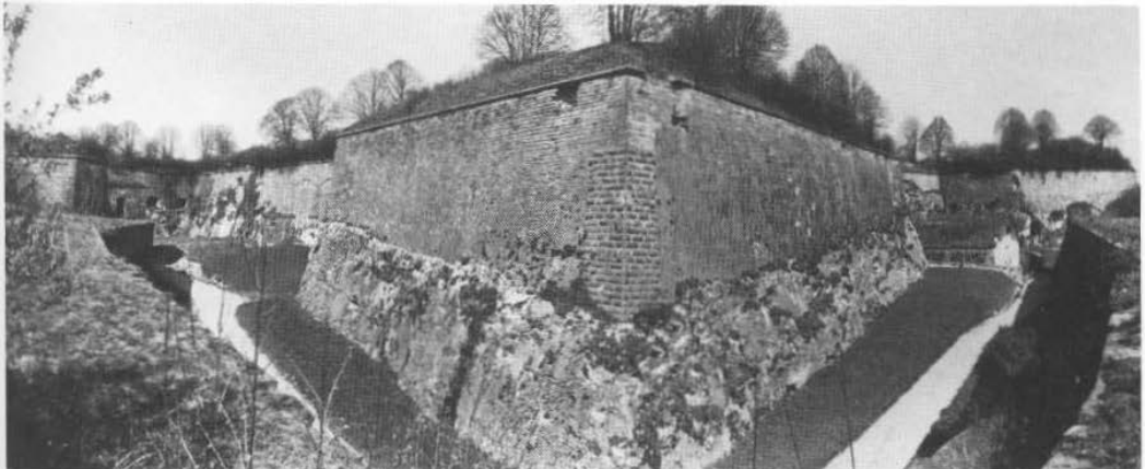
63 Belfort Citadel, with shell damage from the famous Prussian siege of 1871
