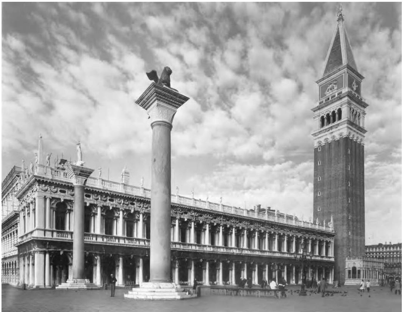
Jacopo Sansovino The library of San Marco (Bibliotheca Marciana) is housed in the Libreria Sansoviniana on the Piazzetta, Venice. Begun by Sansovino in 1536, it was eventually completed by Vincenzo Scamozzi in the 1580s. Anthony Kersting, London
