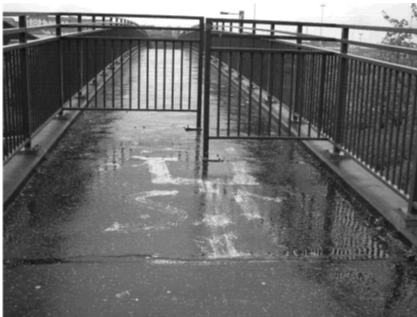
Figure 3 'SYM' on the tarmac on the lead-in to Sighthill estate, Glasgow.
