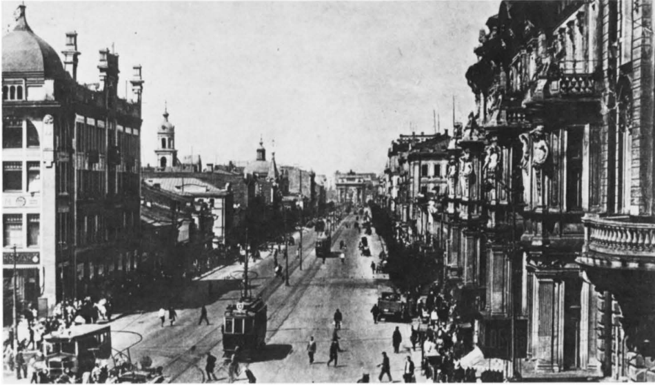
Tverskaia Street with triumphal arch in background.
