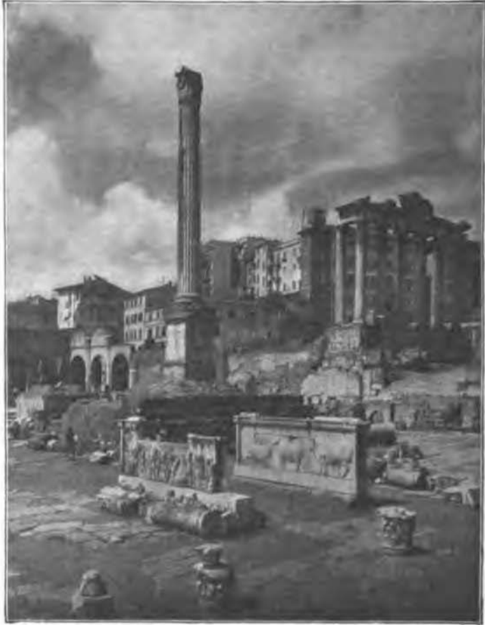
THE COLUMN OF PHOCAS IN THE FORUM (608 A. D.). REMAINS OF THE TEMPLE OF SATURN IN THE BACKGROUND TO THE RIGHT. 1
