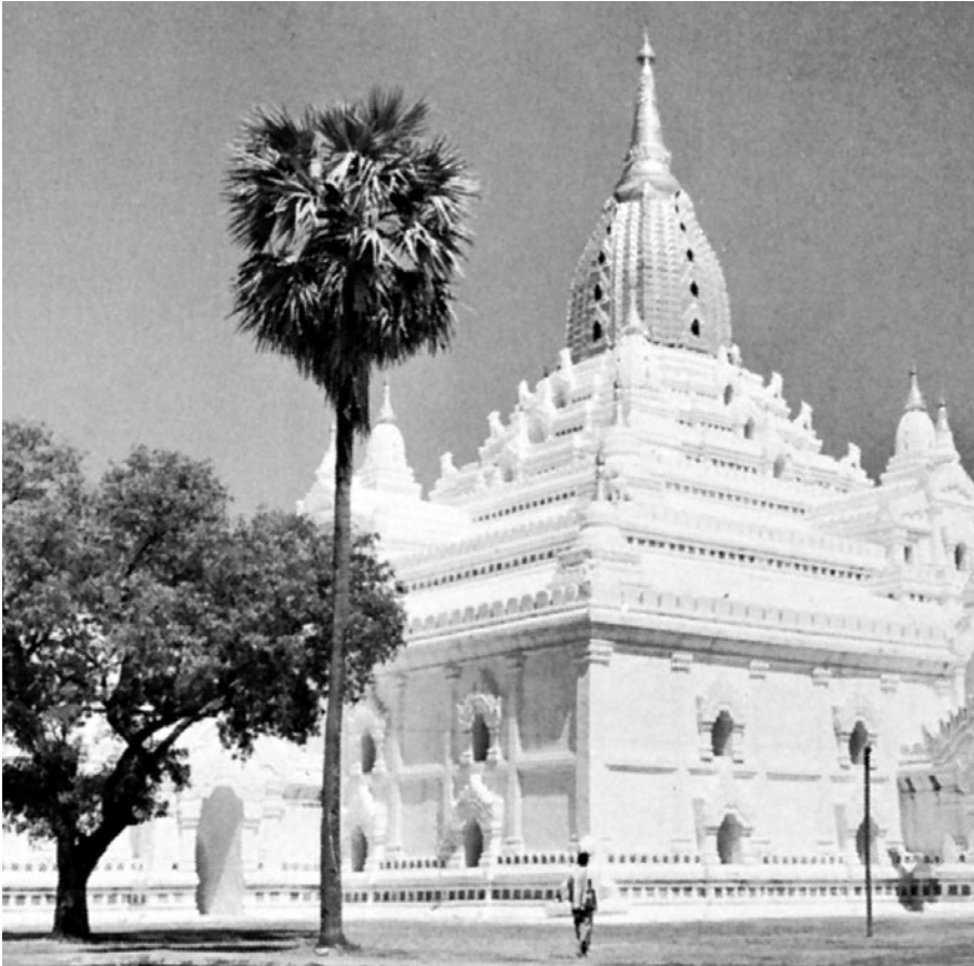
The Ananda Temple at Pagan, restored after the 1975 earthquake
