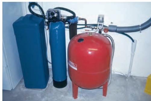
**Water filter (blue cylinder) for purification of fresh water and a hydrophore (red in colour).**
