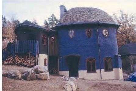
Nibble school in Solvik outside Järna, near Stockholm, Sweden. The buildings are made using several different earth construction techniques. This building is made of wet loaves of loam stacked in a masonry pattern without mortar, and covered with clay plaster.
