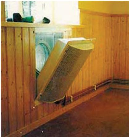
There are various methods for preheating intake air. Intake air can be introduced via a box behind a radiator or through a special air intake radiator. The photo shows such a radiator made by Clean Air System, which is designed to withstand damage from freezing.
