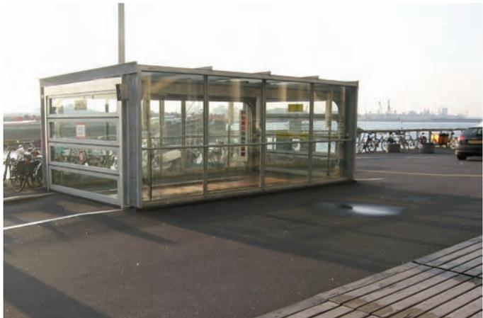
**This is all what you see of an underground garage at the block of flats Si-lodam (Architects MVRDV) in Amsterdam. In this parking garage, the driver places the car at the entrance and an automatic mechanism parks the car.**
