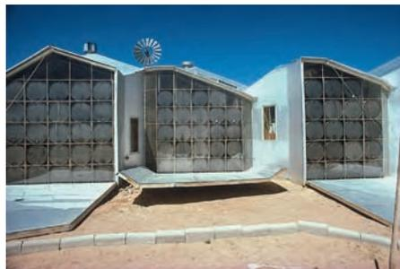
Steve Baer's famous passive solar house in Arizona, US, where insulated shutters are opened and closed on the south-facing glassed-in façade. Water-filled gas barrels behind the windows store solar heat.
