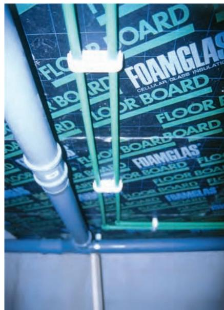
Photo of a suspended foundation, insulated with foam glass, showing sewage and clean water pipes made of polythene, a more eco-friendly choice than PVC or copper.
