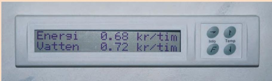
Individual metering is being introduced in new buildings. The photo shows the individual meter display, giving energy and water cost per hour, used by the housing company Svenska Bostäder in a building in Hammarby Sjöstad, Stockholm. The display is located so that personal consumption is easily visible.
