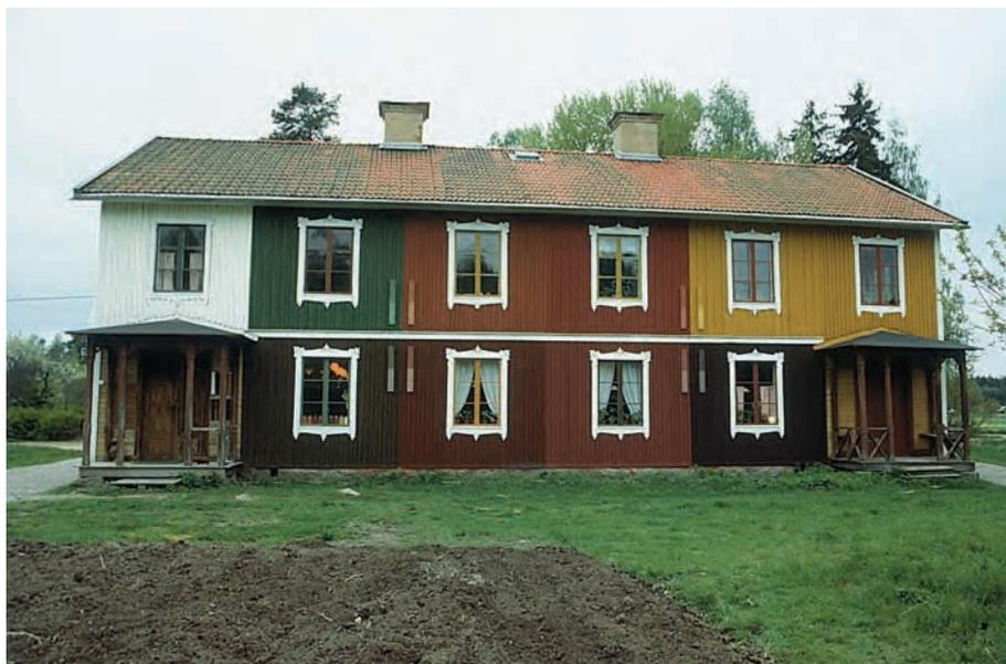
A variety of distemper paint tests on timber cladding at The Gysinge Centre for the Preservation of Historic Buildings (between Gävle and Uppsala, Sweden).
