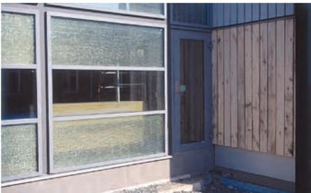
As it is not possible to see through transparent insulation material (TIM), it is alternated with glass.
