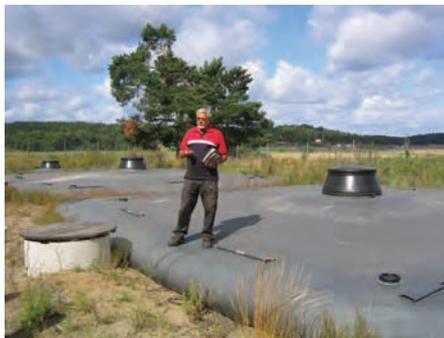
Storage tanks for human urine at the Björnsjön research facility, Sweden, which has been managed by Stockholm Water since 1996. The tanks are filled by gravity from a tanker. Each of the three tanks holds 150m<sup>3</sup>. The tanks are placed near fields where the urine is spread using feeder hoses on spring grain used as fodder.
