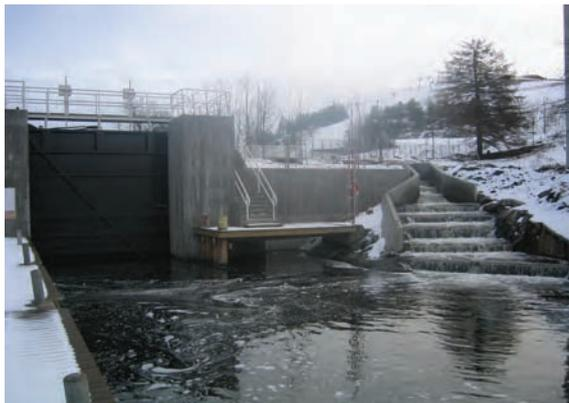
**Fish ladders make it possible for fish to bypass small-scale hydropower stations and locks, here at Sickla lock in Hammarby Sjöstad, Stockholm.**
