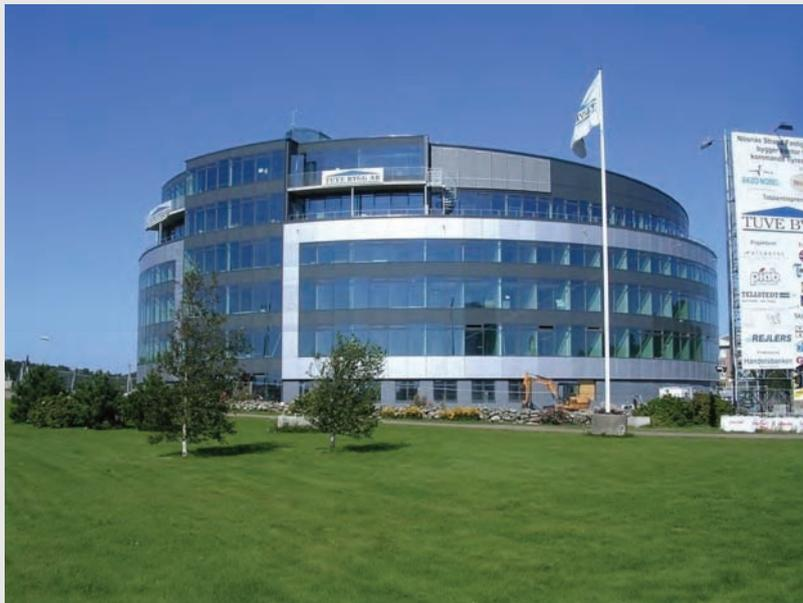
**Office building for Akzo Nobel in Stenungsund. This office building is built using heavy materials. The heavy mass is used to balance heating and cooling needs. The building is ventilated through small windows. These windows, made by Window Master, are closed and opened as necessary by self-regulating sensors, which regulate both temperature and relative humidity. This concept significantly lowers energy needs.**
