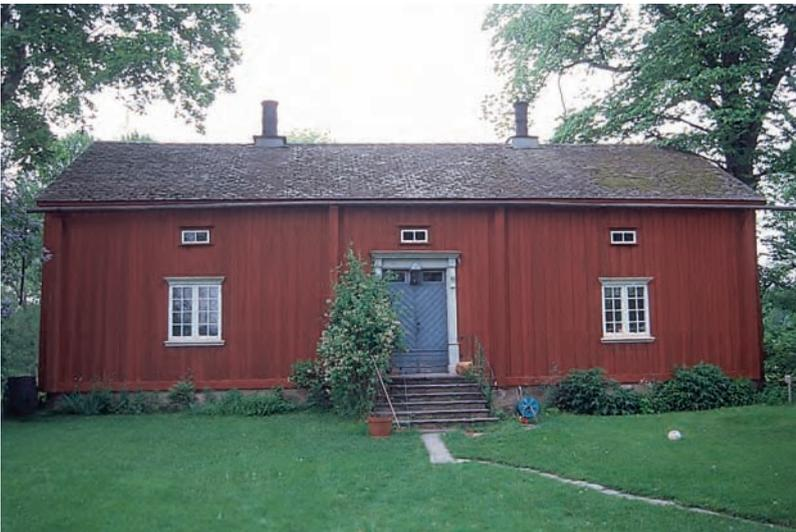
A wing of the Von der Eckerska farmhouse in Värmland, painted with the typical Swedish distemper paint (Falun Red paint), and with two iron chimneys.
