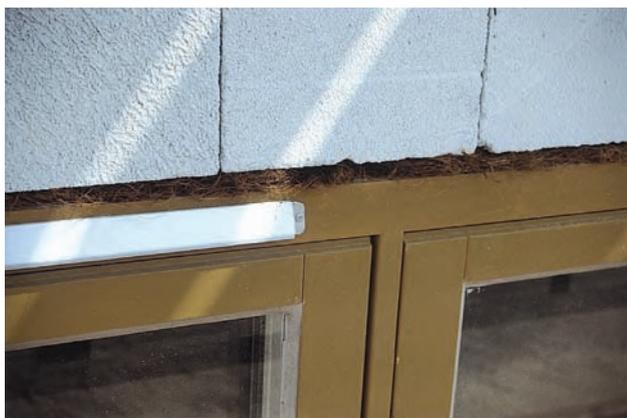
Coconut fibre packing in a lightweight concrete wall.
