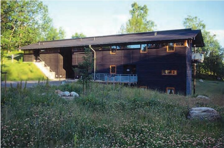
**Residential area in Hestra, Borås, Sweden, with both cladding and roofs of black corrugated cement-based boards (fibre cement boards).**
