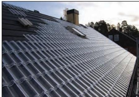
**Roofing tiles made of glass by SolTech Energy. They act as a roof, a watertight layer and as solar air collectors to heat water in the accumulator tank, via a heat exchanger (air to water).**
