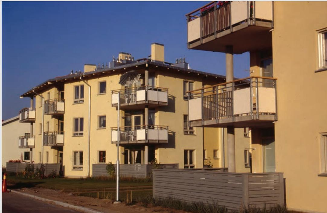
**Multi-family houses, 'Birgittas Trädgårdar' in Vadstena. Fresh air is introduced through an earth-pipe to an air chamber in the foundation. Individual ducts take air to every room. Every kitchen and bathroom has its own ventilation chimney with a rotating cap.**
