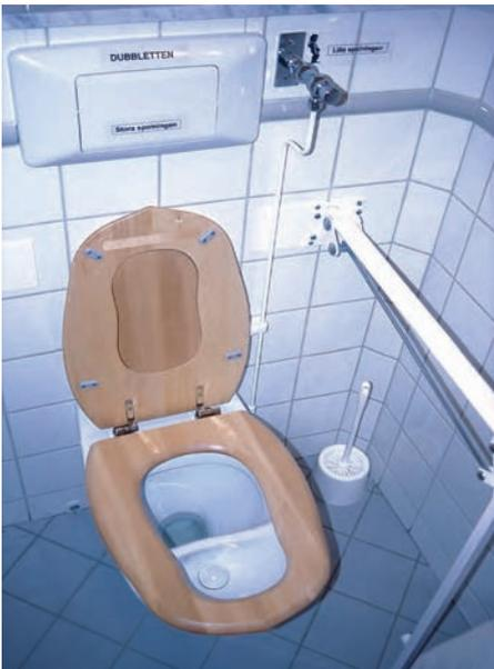
The urine-separating flush toilet *Dubbletten*. It has two bowls and two flush buttons, one for 'the large' and one for 'the small'. It also has an extra cover that can be lowered so that it can be used by children.
