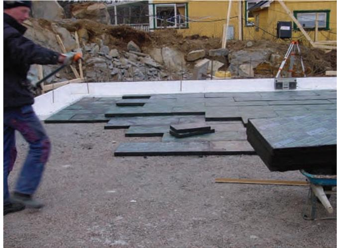
**Cellular glass blocks** ( $\lambda = 0.15\text{W/mK}$ ) are made from loose cellular glass (85 per cent) and cement (15 per cent). They are used as load-bearing and insulating building blocks. It holds its shape, withstands frost, mould and fire, and contains no hazardous additives.
