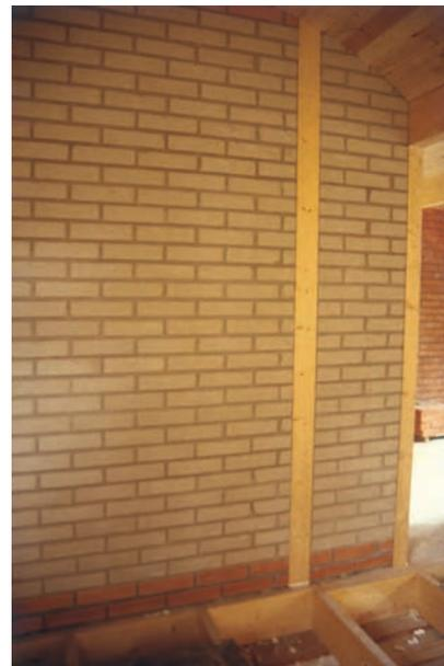
Clay-stone wall built with a load-bearing wood construction.
