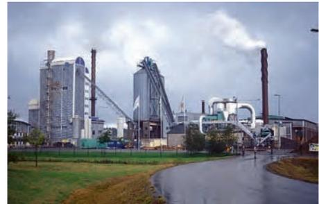
**Biomass gasification combined heat and power plant in Värnamo. Energy is extracted in three stages: first as electricity in a gas turbine and then in a steam turbine, followed by district heating to heat the town.**
