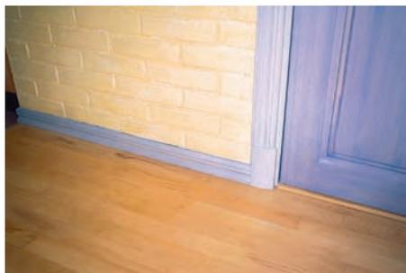
**A wall of unburnt clay bricks, coated with casein paint.**
