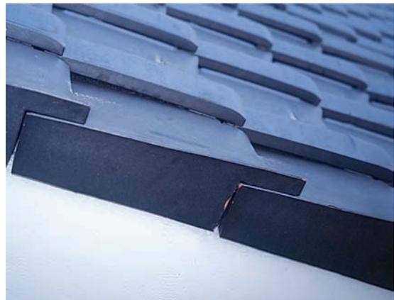
**Clay tile roof in China. In China there are three kinds of roof tiles: ridge tile, roof tile and verge tile. Verge tile is made in order to provide a harmonious finish to the roof. Wooden bargeboards at the outer edge of a tile roof are not used in all countries.**
