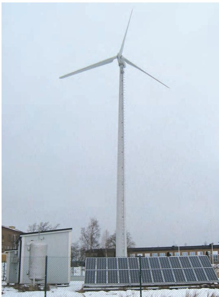
The Swedish company Morphic produces an energy system where wind energy is transformed into hydrogen gas that can be saved and transformed again to electricity via fuel cells when there is no wind.
