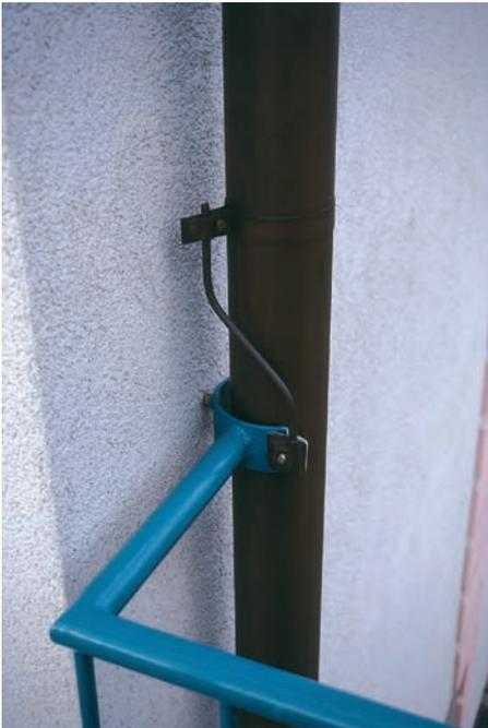
**To reduce the effects of electromagnetic fields produced by metal in building components (caused by capacitance), these may be earthed.**
