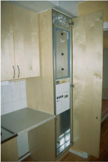
This is how a heat exchanger in a single-family house can be fitted in a kitchen cupboard. This house in Lindås, Gothenburg, Sweden has no heating system.
