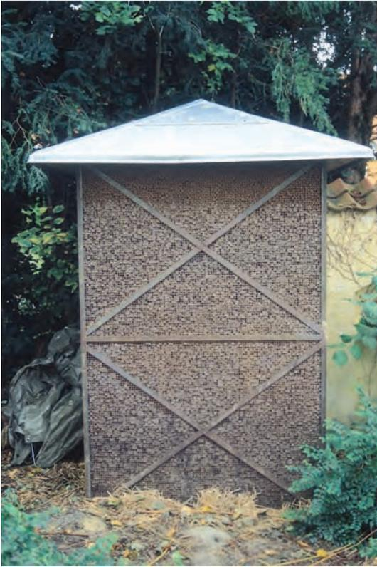
Intake air can be cooled using evaporative cooling. The photo shows the air intake to an underground duct filled with expanded clay pellets which are sprinkled with water in the summer. The intake air is thus cooled first by evaporation and then by the cool underground temperature.
