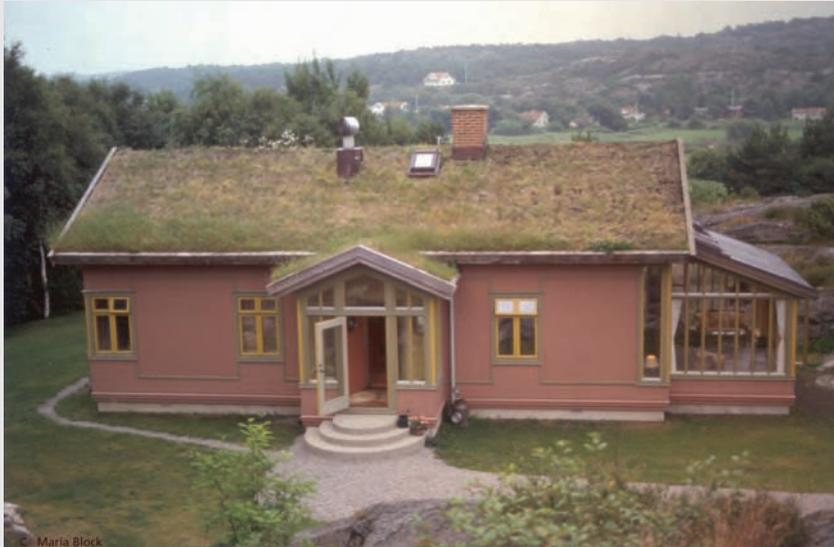
**The Hus Torkel building in Kovikshamn, Bohuslän, is ventilated with fresh air through three earth-pipes, and the exhaust air is removed through a ventilation chimney with a rotating cap. One of the earth-pipes cools the larder.**
