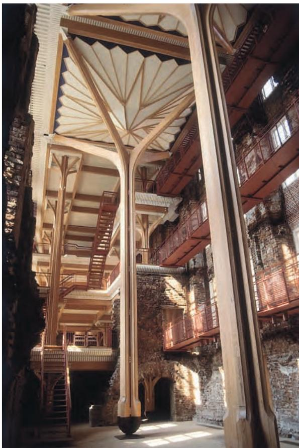
**Renovation of an old castle ruin in Koldinghus, Denmark. The new load-bearing construction is built of glulam.**
