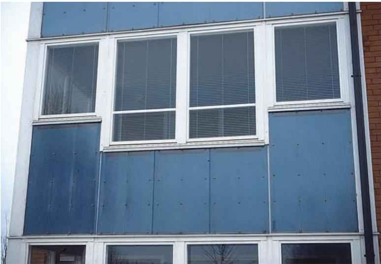
Bengt Hidemark is an architect who has applied the preheated intake air method. The spaces between the bottom of the windows and the floors in this home for the elderly in Märsta, Sweden are designed as solar walls.
