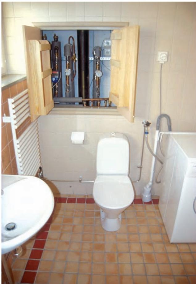
**In the Birgitta’s Garden flats in Vadstena, all services are confined to a few vertical shafts. Access to the service shaft is via a small door in the bathroom, where the meters for cold and hot tap water, heating and electricity are situated.**
