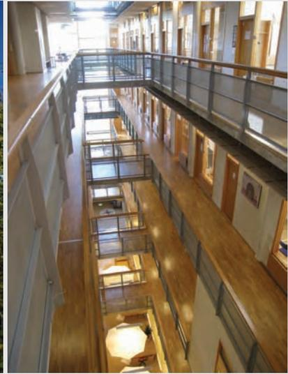
**An educational building of the Royal Institute of Technology in Haninge, Stockholm. The air is introduced through an earth-pipe into a common space. This open space goes through all the floors and is ventilated through windows at the top. The individual rooms are ventilated through this open space. There are also ducts from the classrooms to fan-equipped ventilation chimneys on the roof. The system is computer-controlled.**
