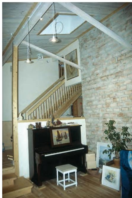
A living room with an interior brick wall. The purpose is to obtain a relatively thin but heavy wall section that can store heat throughout the day.
