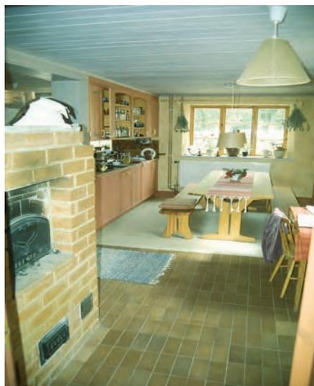
A Finnish bake oven built according to the tiled stove principle in a kitchen, Alma farm, near Arboga, Sweden.
