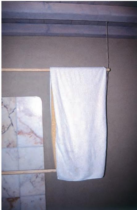
**Bathroom with marble splash areas and clay walls as moisture-buffering material. Marble has a high pH value and is antiseptic.**
