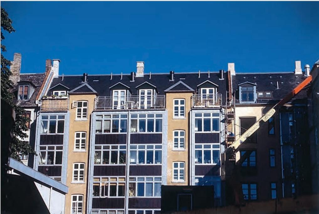
The flats were made a little larger by adding bay windows to the sides facing the yard. This made it possible to add bathrooms with a shower in the apartments. Solar cells were placed on the south-facing bay windows. Insulation was added to lofts, and windows were sealed and a third pane added.
