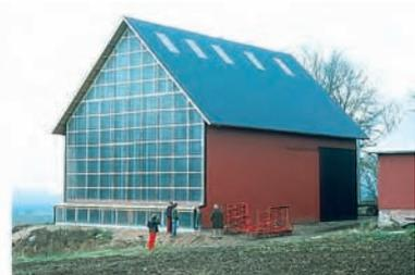
In Umeå, northern Sweden, there is a car dealership located in an environmentally designed facility called Green Zone. Intake air to the car dealership rooms is brought in through an air solar collector which preheats the air. In northern Sweden it can be warm in the sun despite below-zero temperatures.
