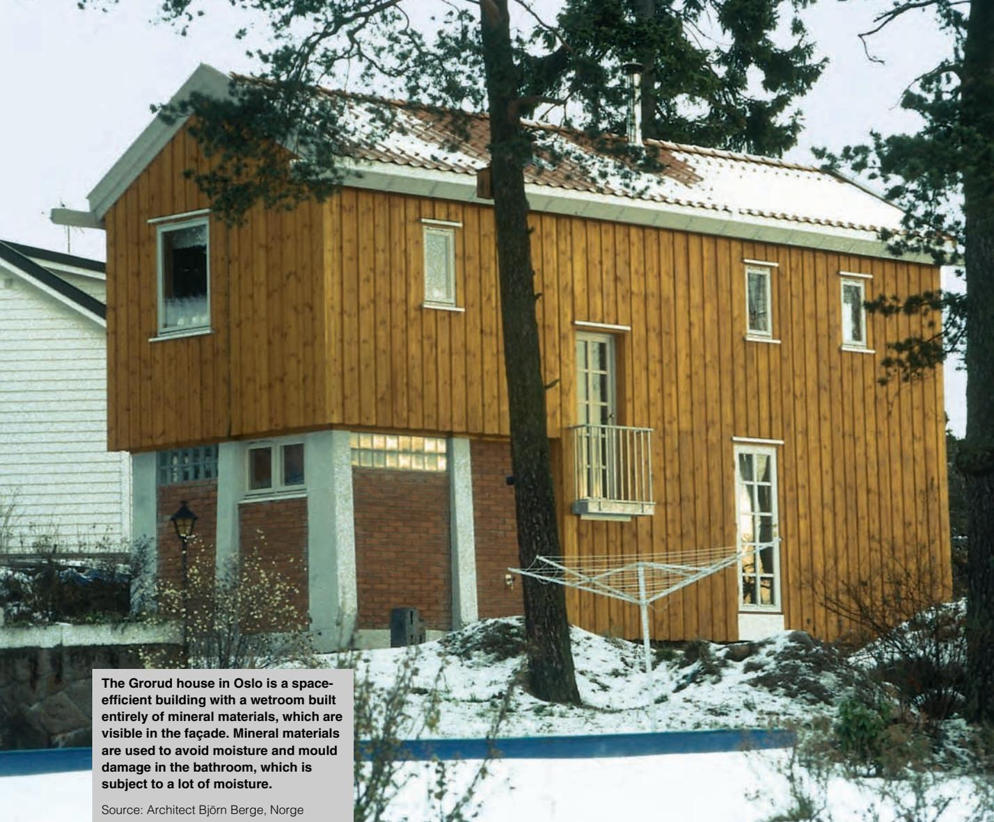
The Gorud house in Oslo is a space-efficient building with a wetroom built entirely of mineral materials, which are visible in the façade. Mineral materials are used to avoid moisture and mould damage in the bathroom, which is subject to a lot of moisture.
