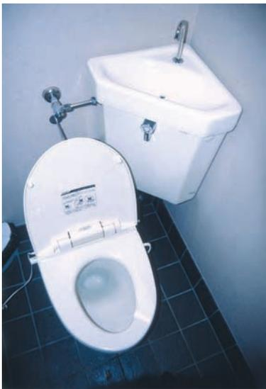
In Japan there are toilets that, when flushed, refill the cistern with water from a small sink where hands can be washed. So the water is used twice.
