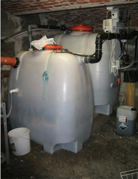
**Biovac's mini purification plant, with batch treatment, placed accessibly in a cellar.**
