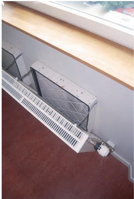
Modern ventilation slots are often combined with a metal box behind the radiator where air is preheated. If necessary, a filter can be placed in the box. The photo shows this type of radiator, which can be opened to facilitate changing filters and cleaning the air intake duct.
