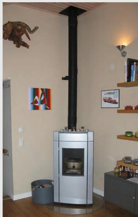
**The pellet stove with water jacket in the living room of the Karlson Hus. It's a 12KW Palazzetti where more than 80 per cent of the heat is stored in an accumulating tank.**
