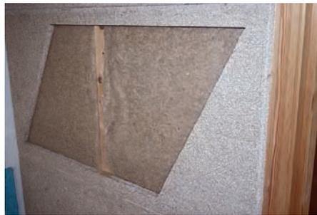
Flax insulation in the form of boards mounted in a demonstration wall.
