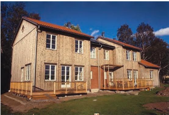
**Wood cladding treated with inexpensive green vitriol at the Understenshöjden eco-village, Stockholm. Some parts of the cladding are brick, behind which are bathrooms built entirely of mineral materials.**
