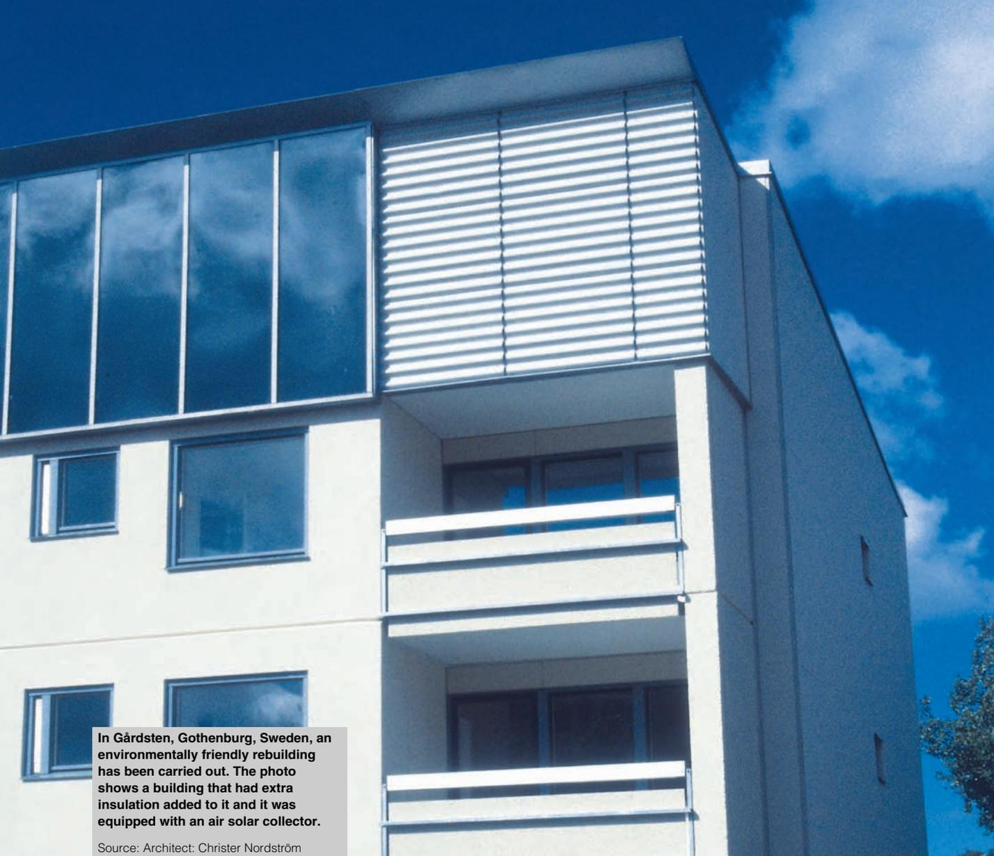
In Gårdsten, Gothenburg, Sweden, an environmentally friendly rebuilding has been carried out. The photo shows a building that had extra insulation added to it and it was equipped with an air solar collector.
