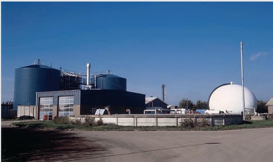
One of Europe's largest biogas facility is located in Helsingør, Denmark. It treats 20,000 tonnes of waste per year from 70,000 households. The 3 million m<sup>3</sup> per year of gas produced can heat 700–800 single-family homes.
