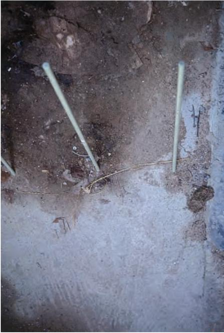
**An example of how a concrete building foundation can be reinforced with fibreglass instead of metal.**
