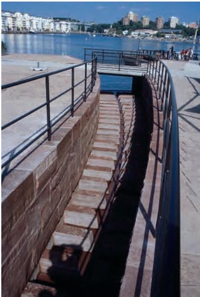
When artificial water surfaces are included in developments, the water must be able to flow and be oxygenated so that it doesn't start to smell. The photo shows a stairway for water to flow over in Hammarby Sjöstad, Stockholm, in order to oxygenate surface water.
