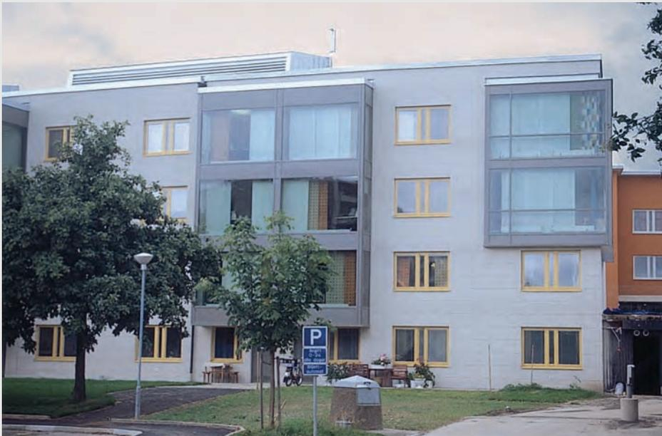
Parts of the ring were demolished to open up the view and the tall buildings were reduced to three storeys to obtain a more human scale. Energy conservation measures were carried out – insulation was added, and windows were sealed and replaced. The buildings were renovated and freshened up with pleasant colours, and some of the buildings were made into workplaces.
