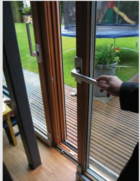
Openable windowdoors with a U-value of  $0.7 \text{ W/m}^2\text{K}$ .
