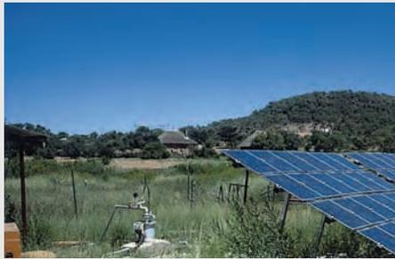
Solar cells can be used to run water pumps. An advantage of this technology is that batteries are not needed. The water is pumped when the sun shines and is stored in a reservoir.
