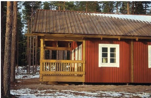
Wood roof with notched boards, that is boards with grooves so water can run off easily, on a test building in the eco-village of Engeshöjden near Gävle, Sweden.
