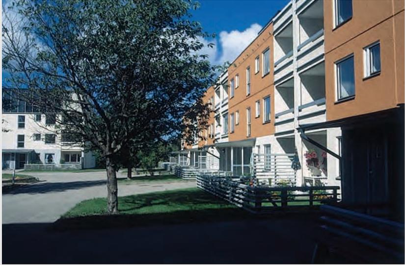
Before renovation. The long side of the high deck-access blocks faces south, which was a good precondition for renovation. The rebuilding changed the area fundamentally with the addition of solar collectors on roofs, glazed-in balconies and glazing-in the ground floor, which transformed windy areas to conservatories.
