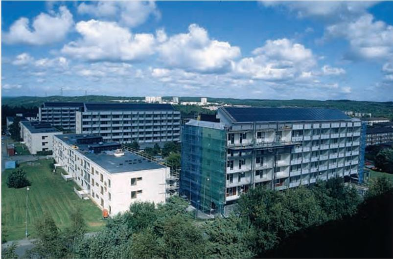
Gårdsten was designed in the 1960s. Badly maintained deck-access blocks made of concrete gave a grey and dull impression. The buildings stand partly on pillars and the open walkways under the buildings were very unpleasant windy spots due to the west wind.
