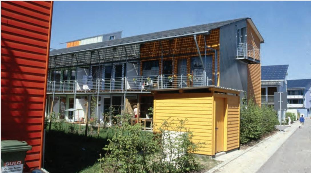
**Plus-energy houses in Schlierberg, Freiburg, Germany. These passive house have photovoltaic roofs that produce more energy than they use on a yearly basis.**
