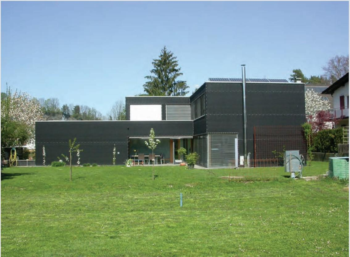
A solid wood passive house with culvert ventilation, active solar water heating, clay plaster internal wall finishes, natural paints, etc – plus an innovative and economical textile façade.
