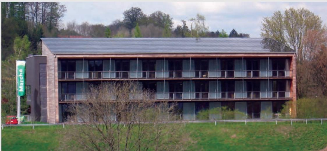
**Award-winning office headquarters for the Marché company, Switzerland's first zero-energy commercial building, constructed at normal cost. It includes an integrated photovoltaic roof, salt-hydrate heat storage in translucent façade panels, solid wood, and standard passive construction.**
