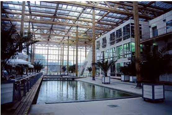
**The town centre and continuing education academy in Mont-Cenis Sodingen, Herne, in the Ruhr region of Germany. The centre is made up of various buildings built inside a large glass building. The glass building is supported on a wooden construction. It has solar cells on the roof and is ventilated with natural ventilation via underground pipes. So a microclimate has been created in the enclosed centre.**
