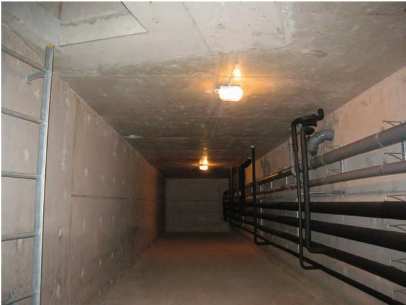
**A well-designed culvert permits quick assembly and simple future additions, as well as easy service and replacement. What is more, overall costs may be lower. The culvert can also be used as an air intake (an earthpipe) that preheats air in winter and cools air in summer.**
