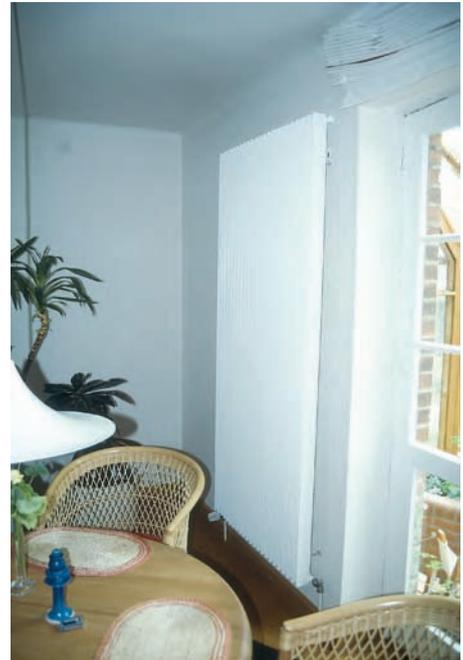
**The heat radiating surface of large, waterfilled wall radiators is large, which improves comfort.**
