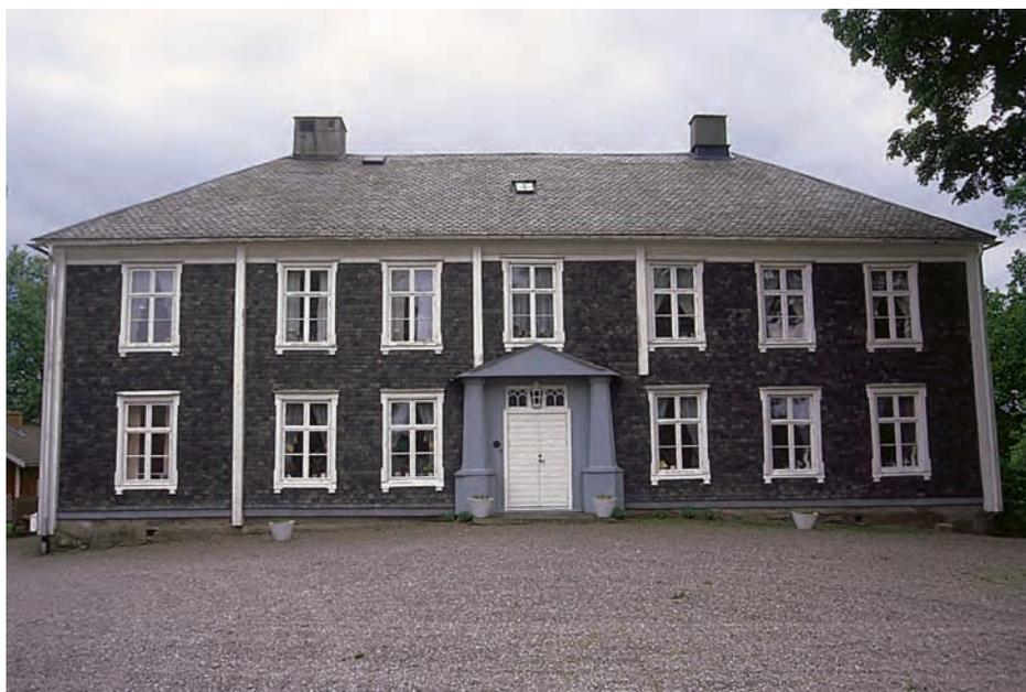
Both the roof and cladding of Gunnarsnäs manor in Dalsland, Sweden are made of slate.
