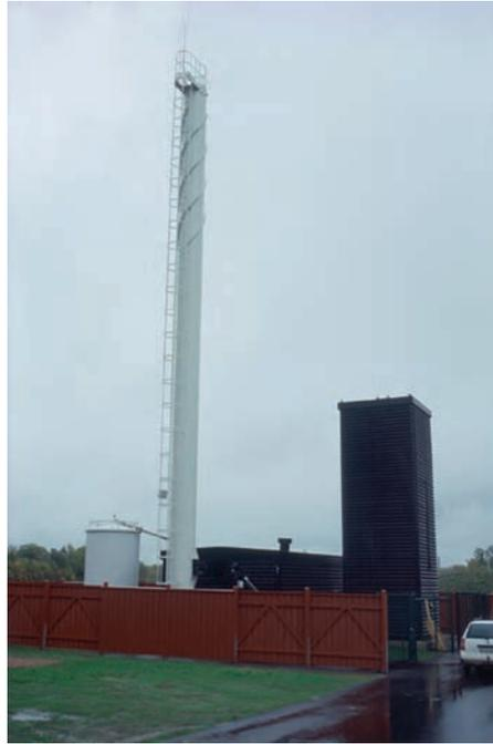
Pellet boiler with silo and chimney at Tegelvicks school in Kvikksund, near Eskilstuna.
