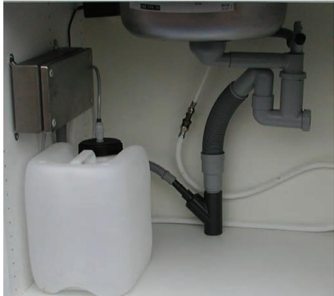
**One problem with local sewage purification has been phosphorus leakage. To reduce this, small sewage treatment facilities can be supplemented with chemical precipitation. The method improves older infiltration facilities, new filter beds and mini purification plants.**
