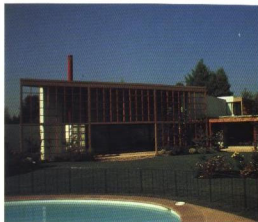
Above: View of the living room from the swimming pool.
