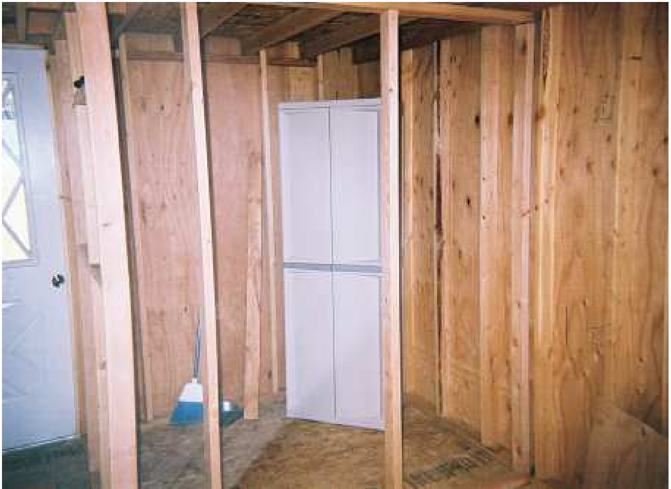
Bathroom walls being built
