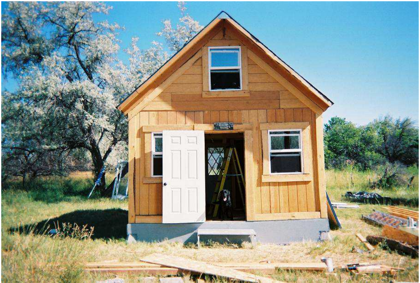
Front of cabin under construction
