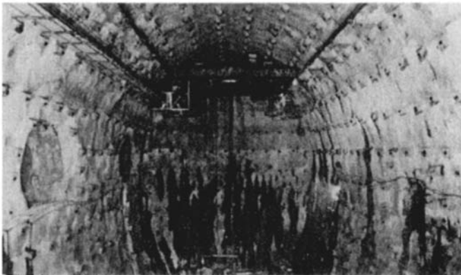
Fig. 1-10 Cavern for powerhouse at Waldeck II pumped-storage scheme. (VSL-Losinger.)
