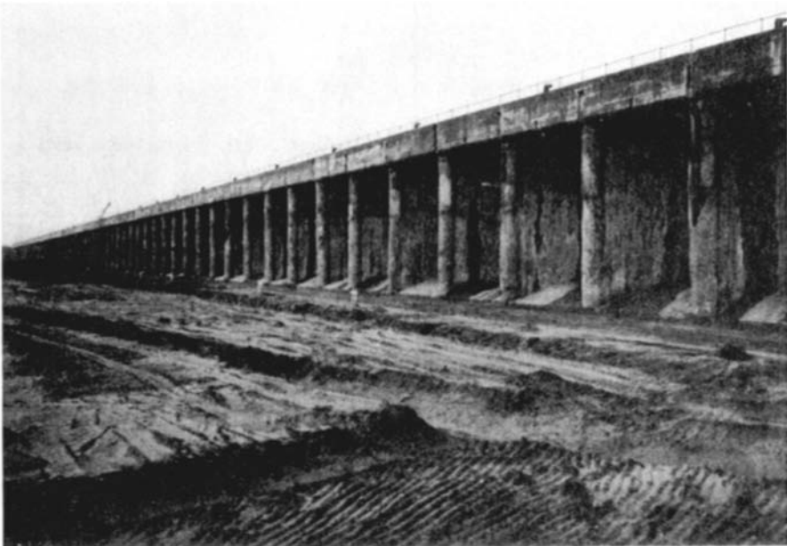
Fig. 1-21 View of Seaforth dock arch wall, Liverpool.
