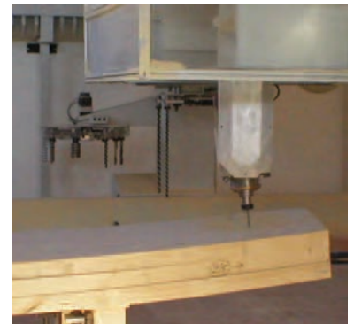
5-axis CNC cutter forming the timber roof members of the Education Resource Centre for the Eden Project, Cornwall.
