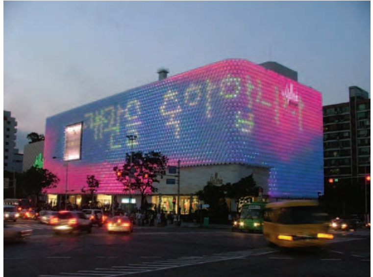
Photo credit: Rogier van der Heide / Arup
