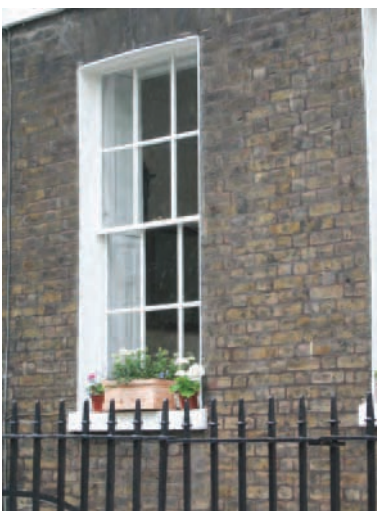
Timber window recessed from face of brickwork of Georgian terraced houses at Highbury Fields, London built in 1789.
