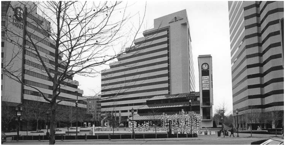
Figure 2.8 MetroCenter, Bethesda, Maryland in 1993.
