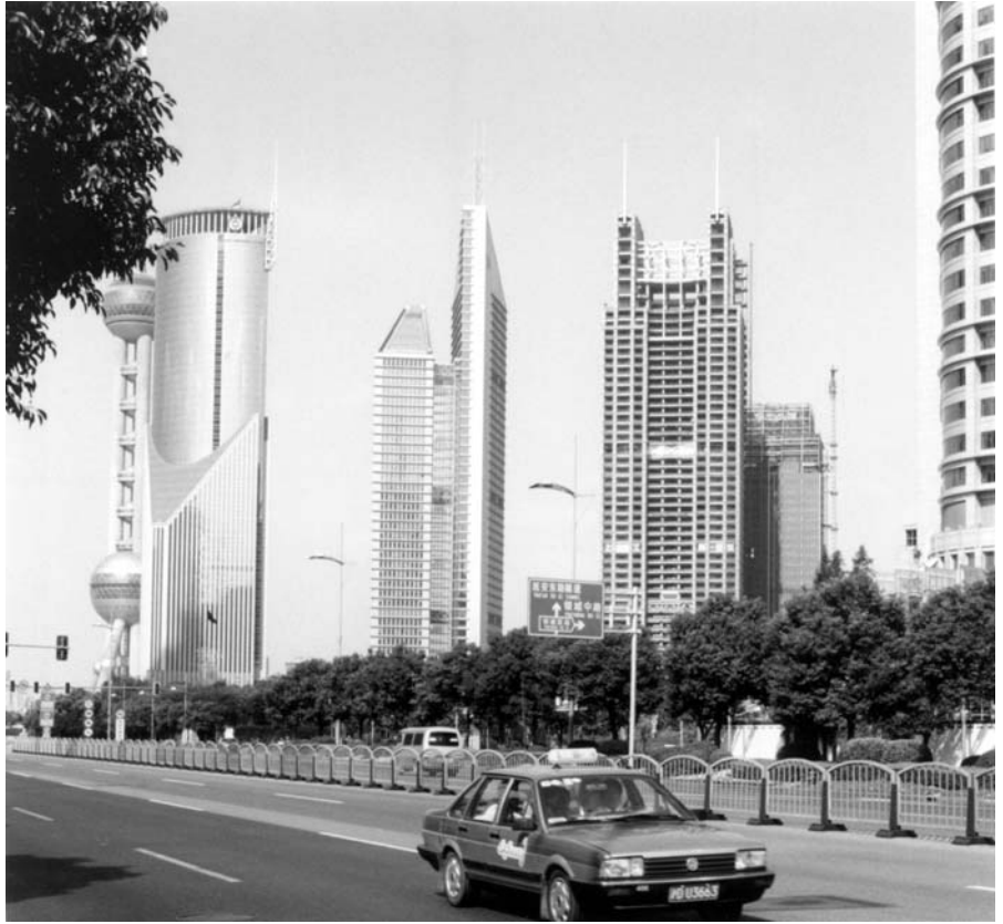
Figure 11.7 The architecture of Lujiazui, Shanghai in 2004.
