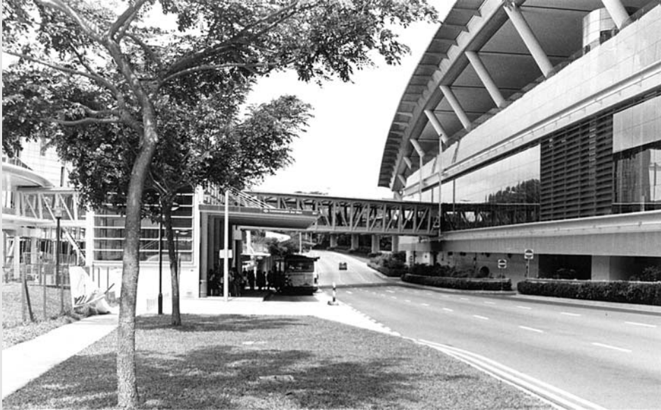
Figure 10.14 Dover station with links to the bus station and technical college (extreme left).
