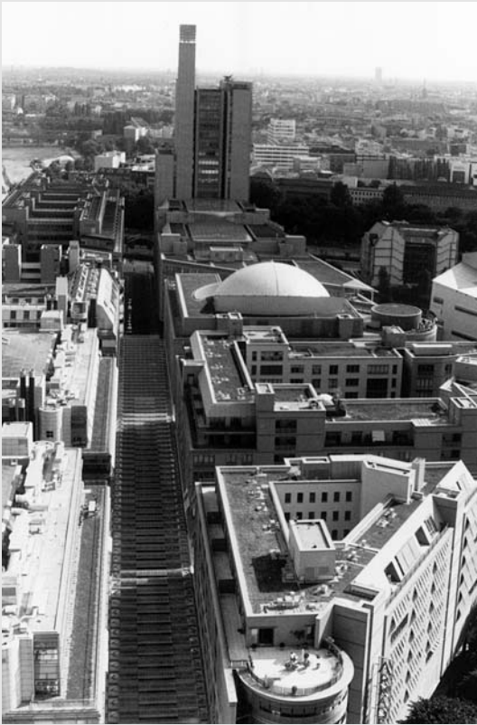
Figure 8.49 A view south towards Marlene-Dietrich-Platz with the Arkaden in the foreground.
