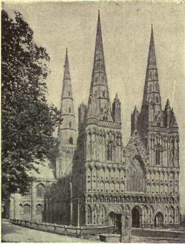
FIG. 139.—WEST FRONT, LICHFIELD CATHEDRAL.
