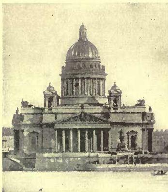
FIG. 212.—ST. ISAAC'S CATHEDRAL, ST. PETERSBURG.
