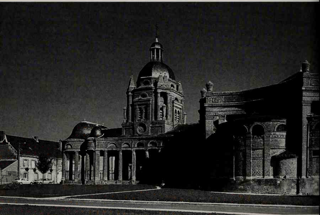
241. The church of St Didier at Asfeld in France (1680) is a mystery. The strange rotunda on the right is the choir with the much narrower domed nave on the left. Unlike other churches in the region, it is built of brick.
