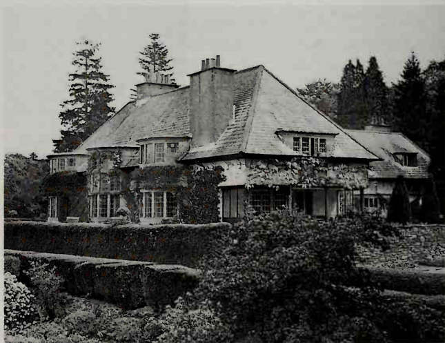
349. Broadleys, overlooking Lake Windermere (1898), is C. F. A. Voysey's most elaborate and self-conscious house, with three bay windows corresponding to dining room, hall and drawing room, carried up into the next storey for bedrooms.
