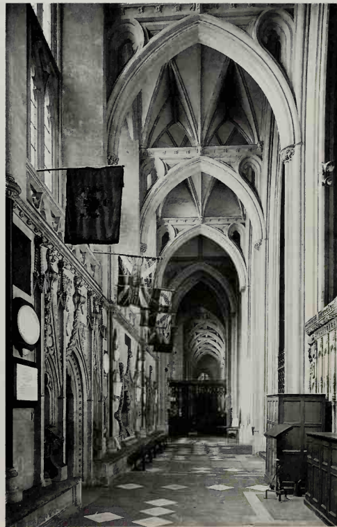
94, 95. The Ely octagon and the aisles of Bristol are two of the leaps of spatial imagination that make the English Decorated style unique. At Ely (below left) the crossing area, damaged by the fall of the tower, was thrown into a single space covered by a wooden octagonal lantern and lit by diagonally placed windows. At Bristol (below) the thrust of the main vault is carried across the choir aisles by miniature bridges with complete vaults of their own.
