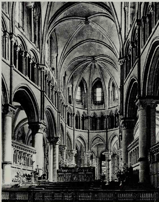
87. The choir of Canterbury Cathedral (1174), whose building history can be followed in unique detail in a contemporary account, marked the decisive beginning of Gothic architecture in England. Its first architect was French, William of Sens. The classically inspired columns and sexpartite rib vaulting (over the foreground bays, not visible) come from France; but much of the ornament and the use of Purbeck marble are English. The curious 'pinched' look is caused by the need to retain Romanesque towers on each side of the original apse, beyond which the Trinity Chapel – by William the Englishman – opens out to house the shrine of St Thomas Becket.
