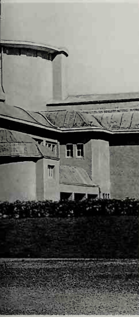
394. Henry van de Velde's Werkbund Theatre at Cologne (1914) was designed as a model theatre for an exhibition demonstrating new ideas in the field. Architecturally, the emphasis was on unity, the concrete construction welding together the foyer, auditorium and fly tower.
