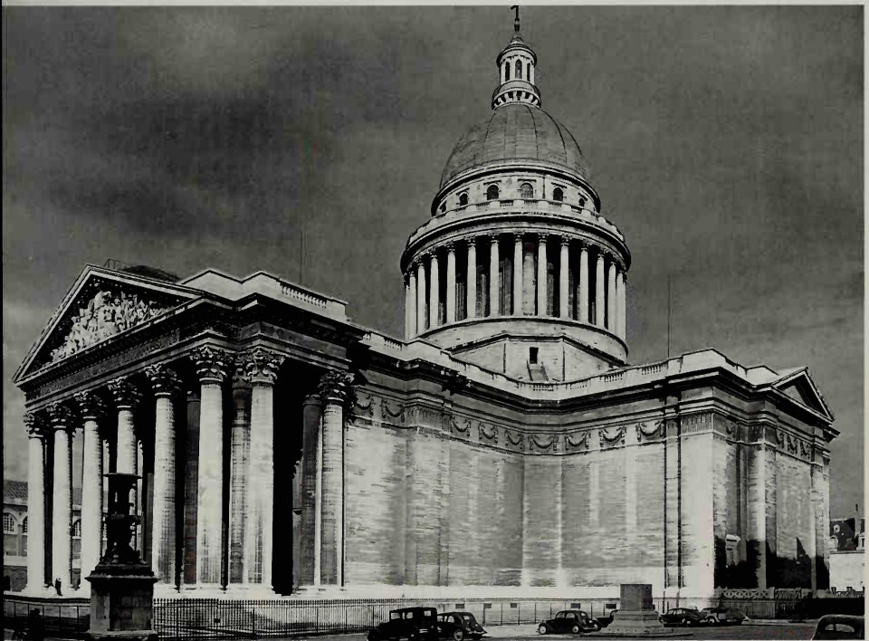
297. Ste Geneviève, the Panthéon, Paris (1754 and later), by Soufflot. The places where the windows have been walled up can clearly be seen.
