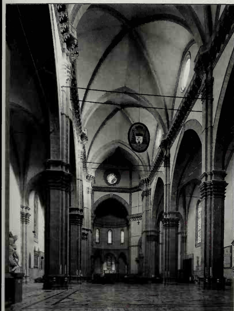
113, 114. Two Italian churches whose Gothic qualities are compromised not only by the width of the bays but also by the use of tie-rods or beams: Florence Cathedral (above, 1334 onwards), and SS. Giovanni e Paolo in Venice (above right, 1260 onwards).
