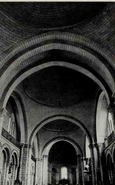
47, 48. Aquitaine and Anjou are distinguished by unusual vaulting techniques. Angoulême Cathedral (above) has Byzantine domes resting on pendentives. Angers Cathedral (above right) employs quadripartite vaults that rise in the centre giving a domical effect.
