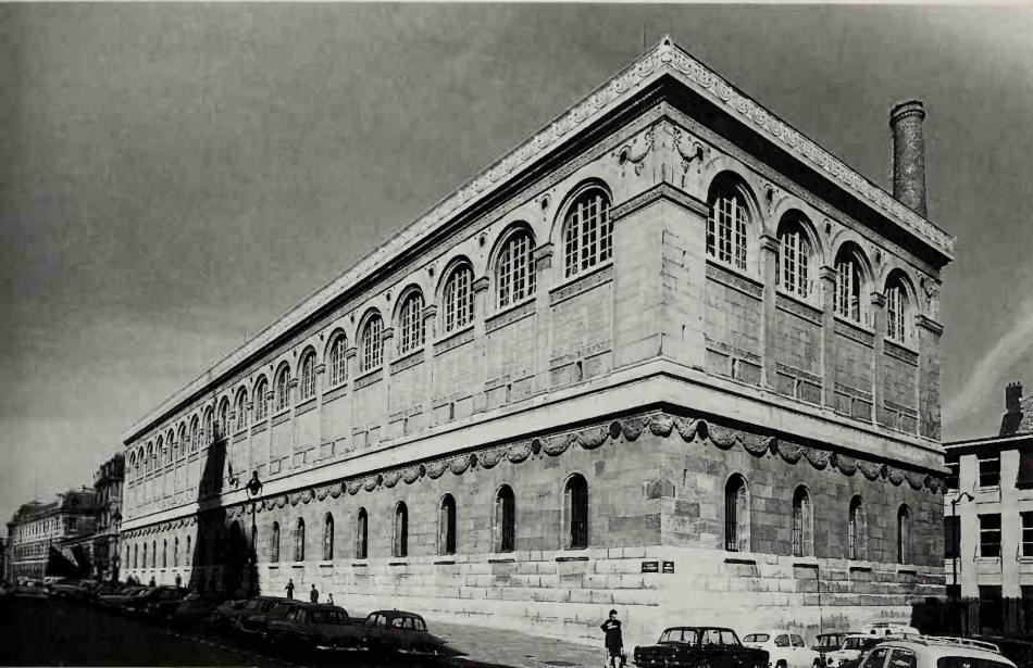
333. In the Bibliothèque Ste Geneviève, Paris (1845), Henri Labrouste produced an experimental building of unusual subtlety. On the exterior the bookcases are expressed by the high walls of the upper storey. The unsuspected interior is all iron.
