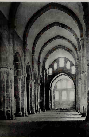
41, 42. Pontigny (above) and Fontenay (below), both in Burgundy, are among the earliest Cistercian foundations – 1114 and 1140 – and show the order's formal austerity. Fontenay keeps its early pointed tunnel vault and square east end; Pontigny was rib-vaulted about 1170 and given an apsed choir with flying buttresses around 1185–1210.
