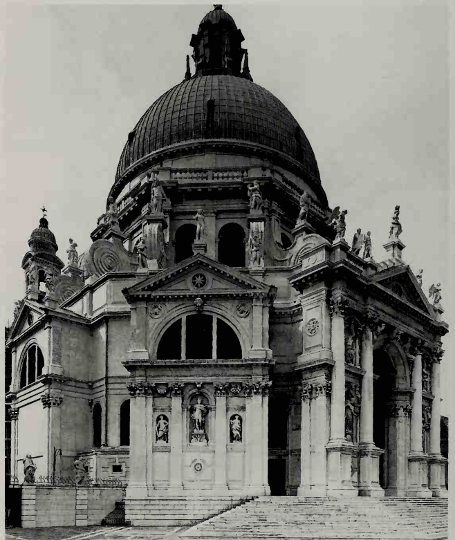
202. Longhena's S. Maria della Salute, Venice (1631) is the dominant accent at the entrance to the Grand Canal. Here is Baroque drama at its most rhetorical – eight sides, sixteen scroll-buttresses and a single dome, visible from every angle.
