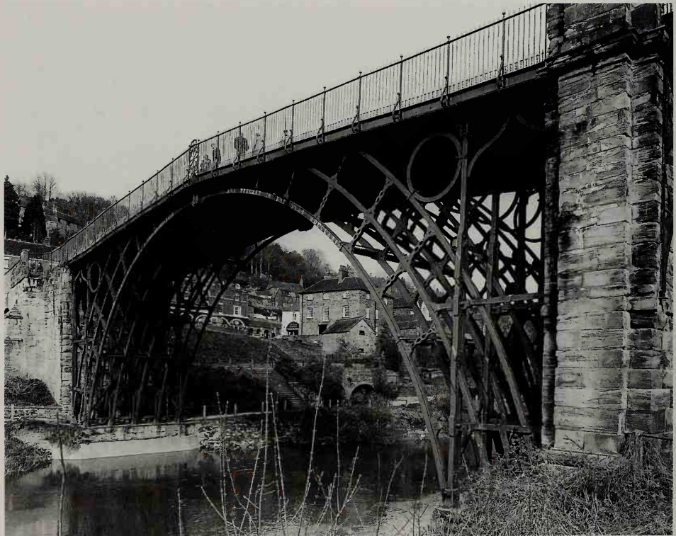
354. The bridge at Coalbrookdale, Shropshire (1778), was the first iron bridge in the world, the result of collaboration between the architect T. F. Pritchard and the ironmaster Abraham Darby. It was the beginning of the specialized division of labour between architect and engineer.
