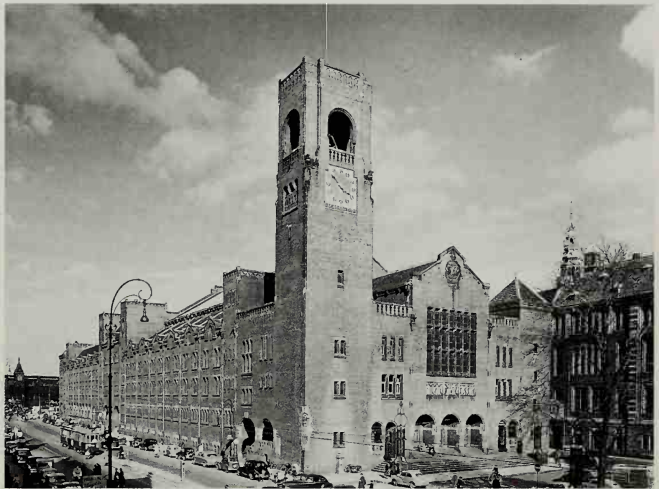
374. Hendrik Berlage's Amsterdam Stock Exchange (1898) stands firmly within a historical tradition (not an entirely Dutch one), but makes full use of modern structural technology.
