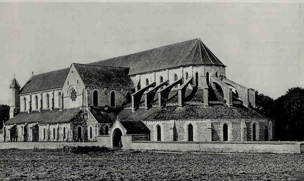
41, 42. Pontigny (above) and Fontenay (below), both in Burgundy, are among the earliest Cistercian foundations – 1114 and 1140 – and show the order's formal austerity. Fontenay keeps its early pointed tunnel vault and square east end; Pontigny was rib-vaulted about 1170 and given an apsed choir with flying buttresses around 1185–1210.
