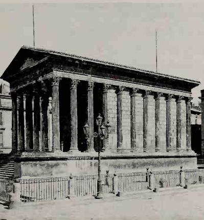
9, 10. The Romans modified the concept of the temple in several ways. One was a new emphasis on direction, with a deep portico marking the entrance, and the rest of the peristyle 'recessed' into the wall (below: Maison Carrée, Nîmes, 16 BC); another was to enhance the status given to the interior (right: Temple of Bacchus, Baalbek, 3rd century AD).
