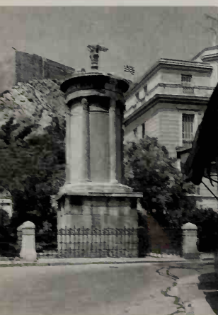
8. The Choragic Monument of Lysicrates in Athens (334 BC) reflects the form of a Greek tholos , a circular structure that goes back to Mycenaean tombs. The order here is Corinthian.
