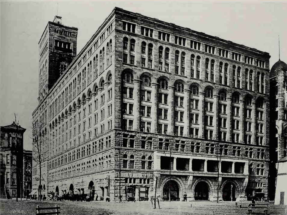
347. The Auditorium Building in Chicago (1886) is the fruit of cooperation between two great men, the engineer Dankmar Adler and the architect Louis Sullivan. Sullivan had not yet evolved his full style, in which Art Nouveau ornament is combined with sheer surfaces (ill. 353). The Auditorium Building's rock-like exterior comes closest to Richardson's Neo-Romanesque (ill. 329) and is still articulated in a way that disguises rather than expresses the structure.
