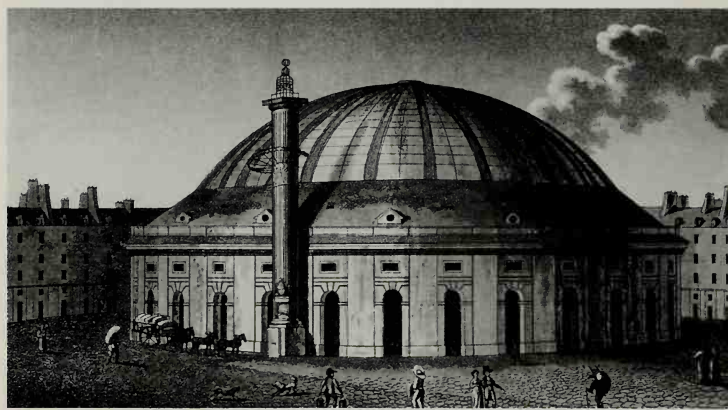
258. The Halle au Blé, or Granary, in Paris, was originally (1762) a circular building with an open courtyard. Twenty years later this was covered by a dome of wood and glass, prefiguring the technical advances of the next century.
