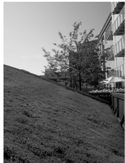
Figure 4.30 An example of a green roof which would reduce runoff
