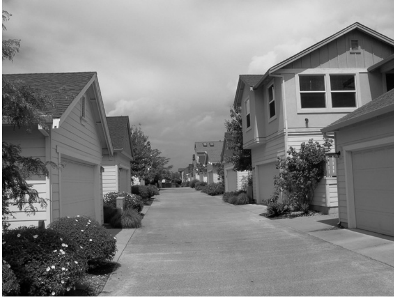
Figure 5.12 New urbanist schemes in the USA often have rear parking alleys as part of a grid
