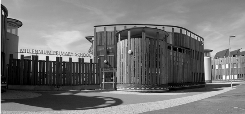
Figure 6.24 The new school in the Greenwich Millennium Village in London showing how defensive a school can be within its context
