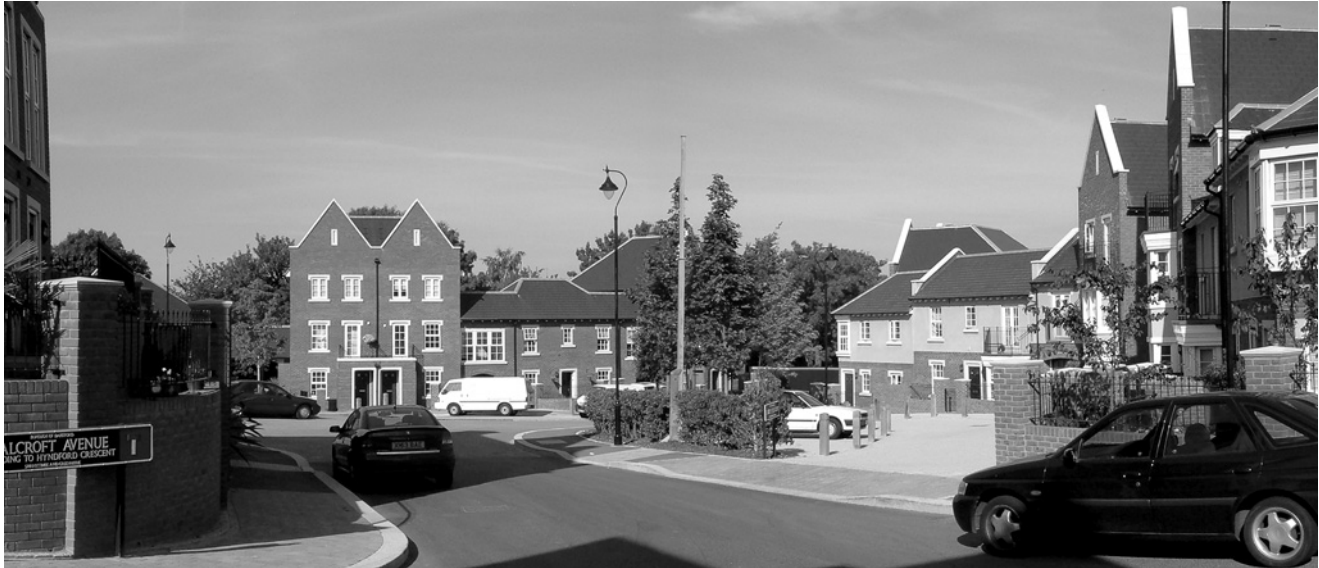
Figure 7.2 A distinctive node at a road junction where the buildings and space create a special emphasis
