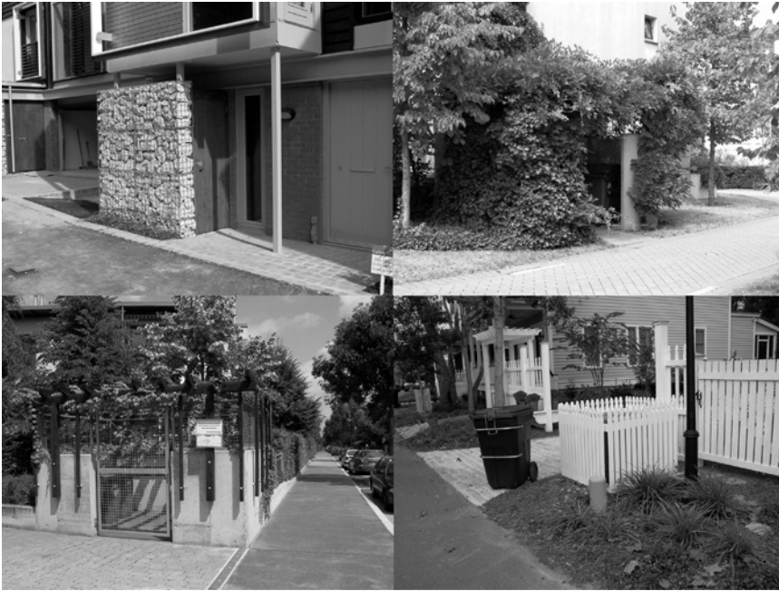
Figure 8.49 Bin stores should be designed as an integrated element of façades or shielded by planting or fencing
