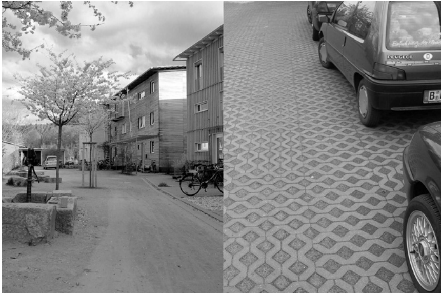
Figure 4.31 Minimise impermeable surfaces
