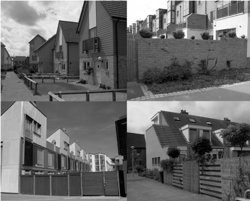
Figure 8.45 Boundaries can cheapen the appearance of an otherwise good scheme or add a sense of quality so their form and materials should be selected carefully
