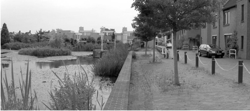
Figure 4.34 A retention pond
