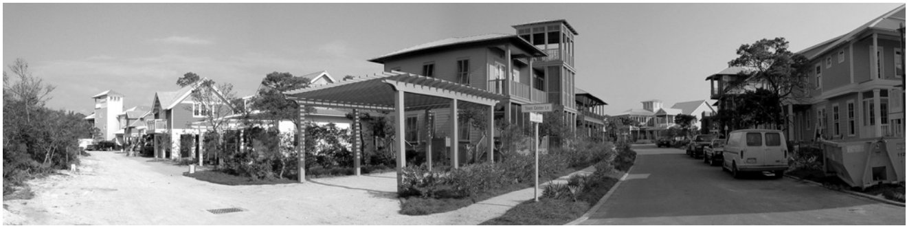
Figure 2.38 Watercolor in Florida is located to exploit the commercial success of the Seaside community next door
