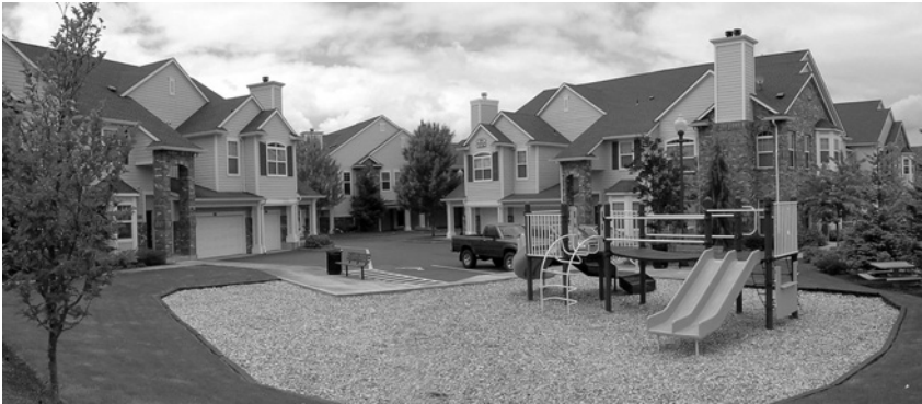
Figure 4.14 New urbanist schemes in the USA try and attain net densities of between 15 and 50 units per hectare, although densities will vary across a scheme
