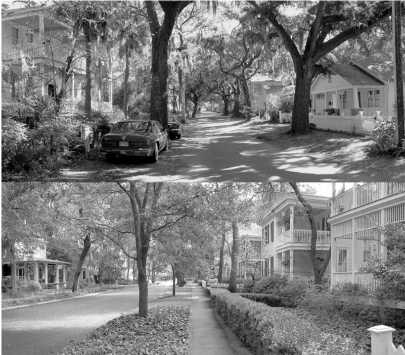
Figure 8.51 The code writers of New Point (bottom) have required house builders to recreate the townscape of Beaufort (top) in South Carolina
