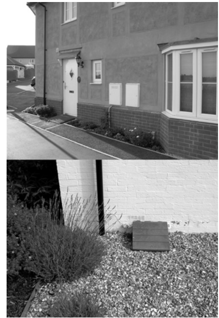
Figure 7.45 Meters should be located in the public realm to reduce the incidence of bogus callers but rather than dominating façades (above) they can be located and integrated more sensitively
