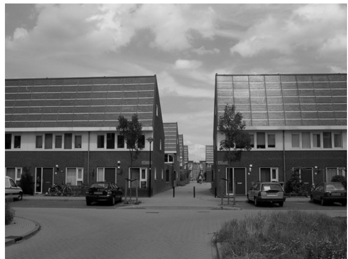
Figure 4.36 The sun can passively and efficiently create electricity using photovoltaic cells or heat water using passive solar water heating systems which should be located on south facing surfaces
