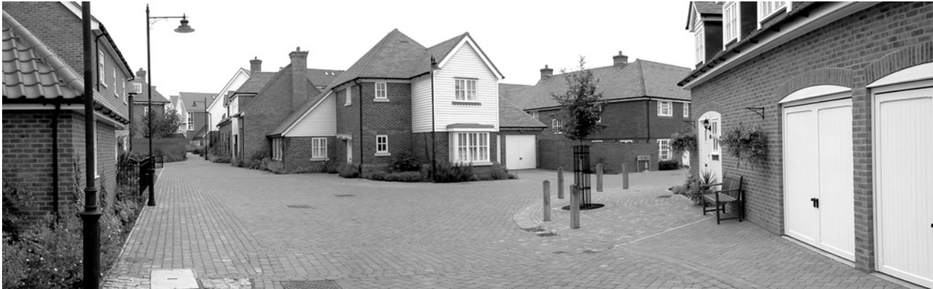
Figure 8.43 Paving materials should be selected to complement those used in the buildings, whilst colours, textures and patterns should be used sparingly so that the hard landscape remains relatively unfussy
