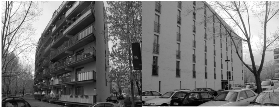
Figure 9.14 An apartment building making the most of solar gain but with a less interesting façade within the public realm undermining the qualities of the street
