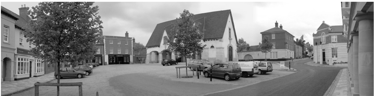
Figure 6.30 The car parking shown here in Poundbury, Dorchester is conceived of as a function of the main square
