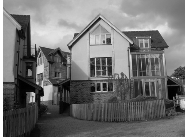
Figure 4.39 Sun spaces on southerly facing façades help to warm a home, particularly when combined with thermal mass within the building structure
