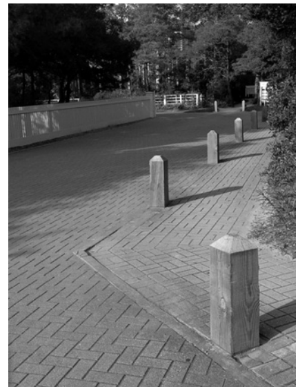
Figure 5.53 Surface materials can help give an impression of a suitable driving speed and help to define areas designated for types of activity
