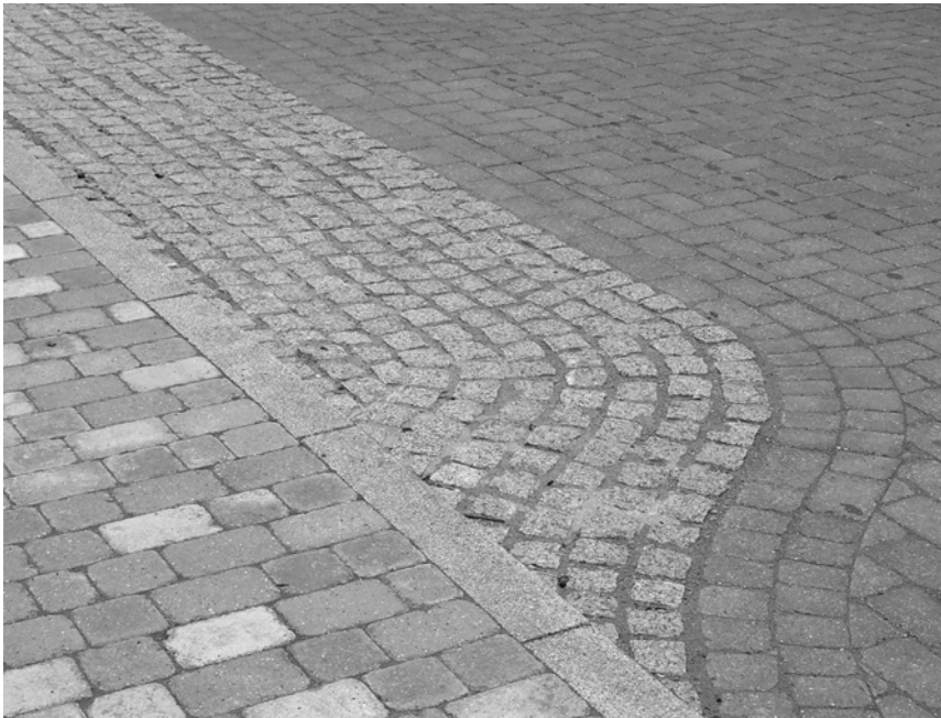
Figure 5.52 Occasional strips provide surfaces suitable for larger vehicles on narrower routes
