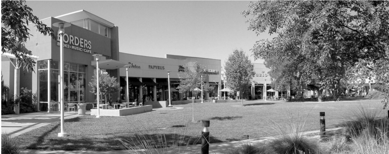
Figure 6.29 The anchor book store in the new development next to the town centre of Davis, California, where secondary uses take neighbouring units
