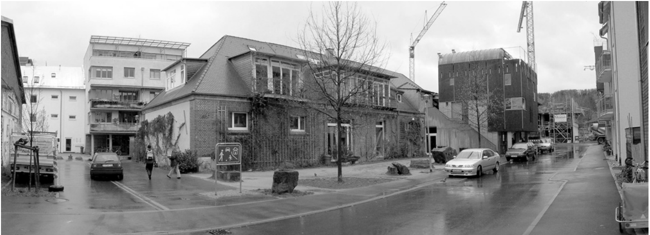
Figure 4.28 Within any scheme it is always desirable to consider the scope and viability of reusing existing buildings so that resources are recycled
