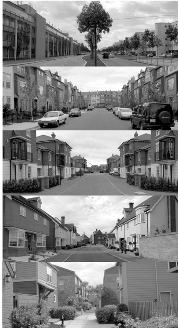
Figure 3.34 Vary the scale of streets to reflect the role of the street within the layout
