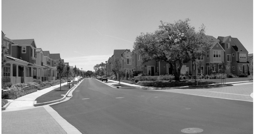
Figure 7.24 Retaining existing landscaping can make new schemes seem mature whilst also making them memorable
