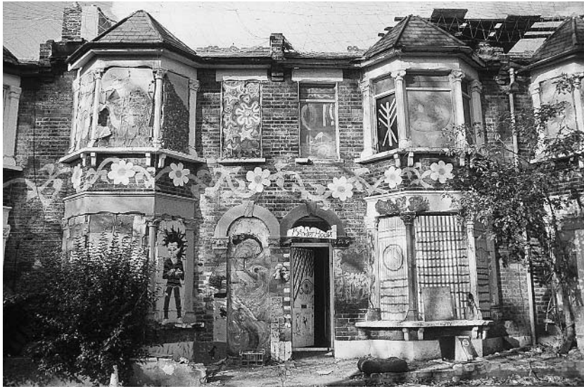
13.1 | Houses, Claremont Road, 1994.
