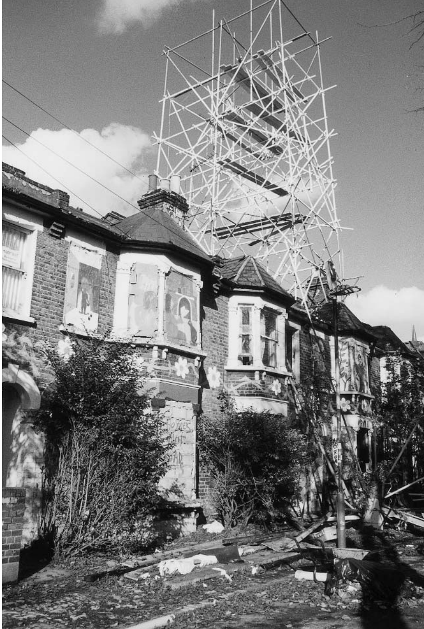
13.3 | Tower structure, Claremont Road, 1994.
