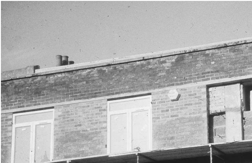
23.11 | Transforming the ex-Tesco's.
