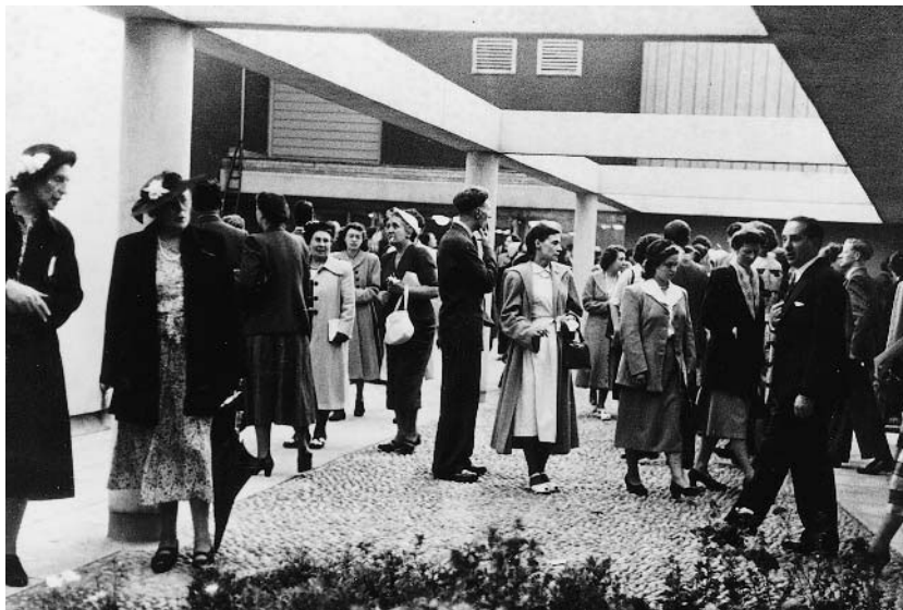
11.6 | Royal Festival Hall, roof terrace. Contemporary photograph.
