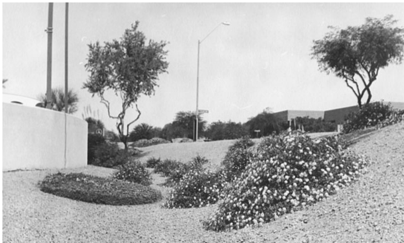
Figure 10.3 Small commercial lot detention facility.
