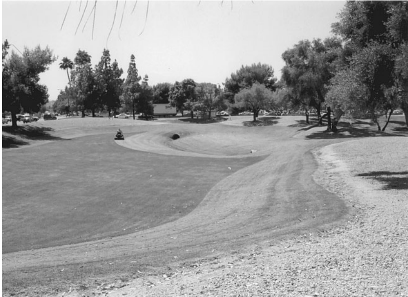
Figure 10.6 Shopping center detention pond.
