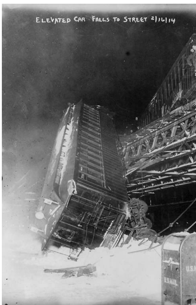
"Elevated car falls to street"—New York City, February 16, 1914
