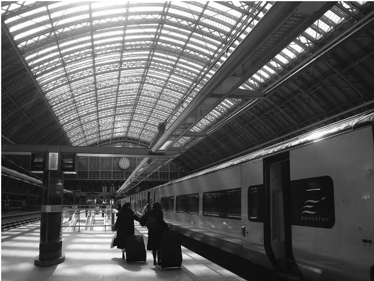
The St. Pancras International station in London includes access to both commuter trains (the Tube) and long-distance trains, such as the Eurostar line that crosses into France and Belgium.
