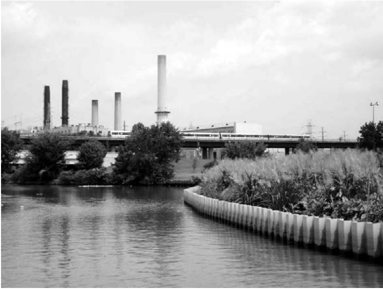
Fig. 29.4. River fringe marshes along the Anacostia River, visible on the right of the photograph. Note plastic sheet piling protecting marshes from erosion. Not visible are fences to prevent Canada geese from grazing planted wetland vegetation.
