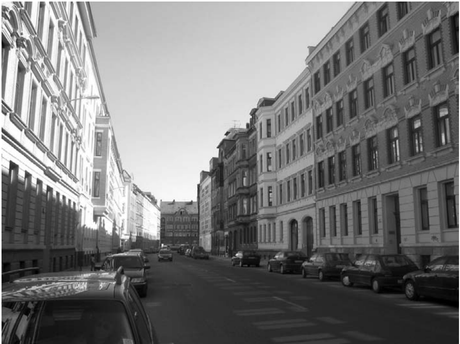
Fig. 21.6. Example of detached kerb-close apartment buildings with open courtyards (1870 to World War I) (photograph J. H. Breuste).
