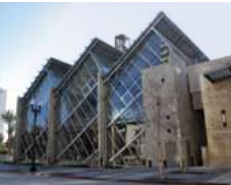
New Children's Museum by Rob Wellington Quigley, San Diego, 2008. The bays of the museum echo the size of earlier plats and thus buildings in the district, establishing a scale that both fits with existing patterns and creates more comfortable rooms and facades than would a building based on a whole-block scale.
