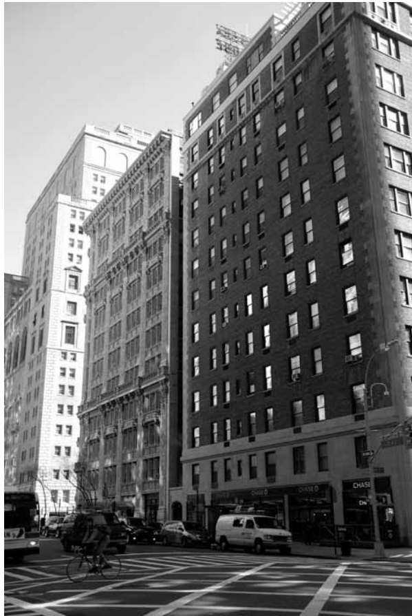
These adjacent buildings in New York share massing, punched openings in a mass wall, and other fundamental characteristics, but differ in the tastes expressed in their facades.
