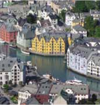
Ålesund, Norway. The built fabric of multistory Jugendstil buildings, waterfront and inland streets, and forested greens establishes a venue of precedents and relationships by which new projects will be judged.
