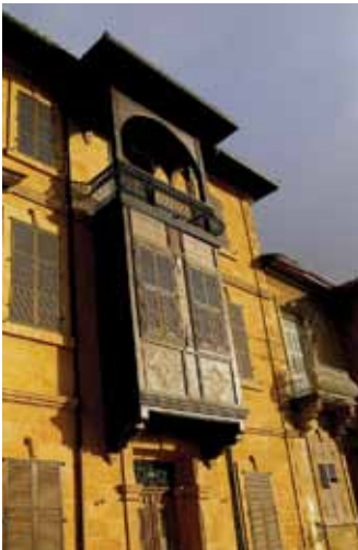
Balcony in Nicosia, Cyprus, extending into the finis. The ancient Levant convention of the finis is a zone along the street wall of a building in which balconies, downspouts, entry steps, and other features may protrude as long as they do not impede horse- or camelback riders or other users of the street. Typically, permanent protrusions must allow a given clearance. In many places, the building owner has rights to this space, including the ability to rent it to street vendors.
