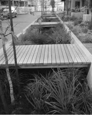
Detail of a street in Portland, Oregon, providing water detention and filtering.
