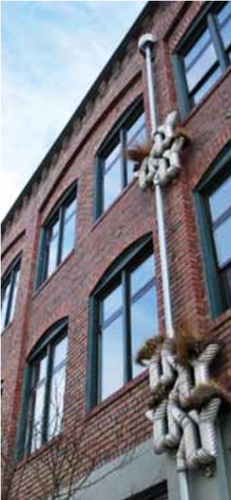
Downspout Garden by Buster Simpson, Seattle, 1999. Designers can rethink established patterns of built form, particularly “unglamorous” forms such as parking lots or power substations, to create delight or other public benefits.
