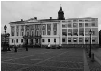
Göteborg Law Courts addition by Erik Asplund, Sweden, 1937.
