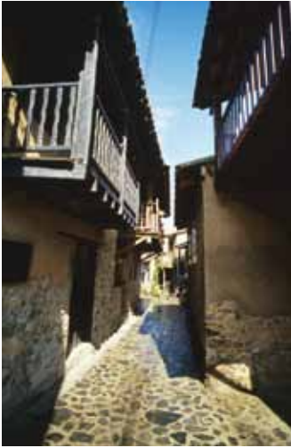
Kakopetria, Cyprus. Town morphologies (e.g., building to the street edge and overhanging balconies) and building typologies and tectonics (e.g., stone bases, plastered adobe walls, and wood) work together to create a pleasantly coherent street and village.
