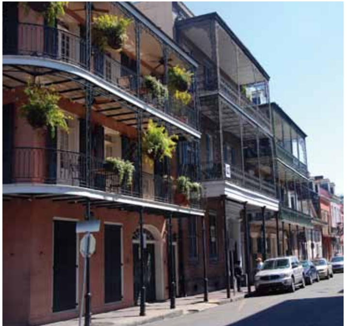
The balconies on these buildings in New Orleans are a separate design level from the main structural system. They can be repaired, replaced, or removed with minimal effect on the mass walls.
