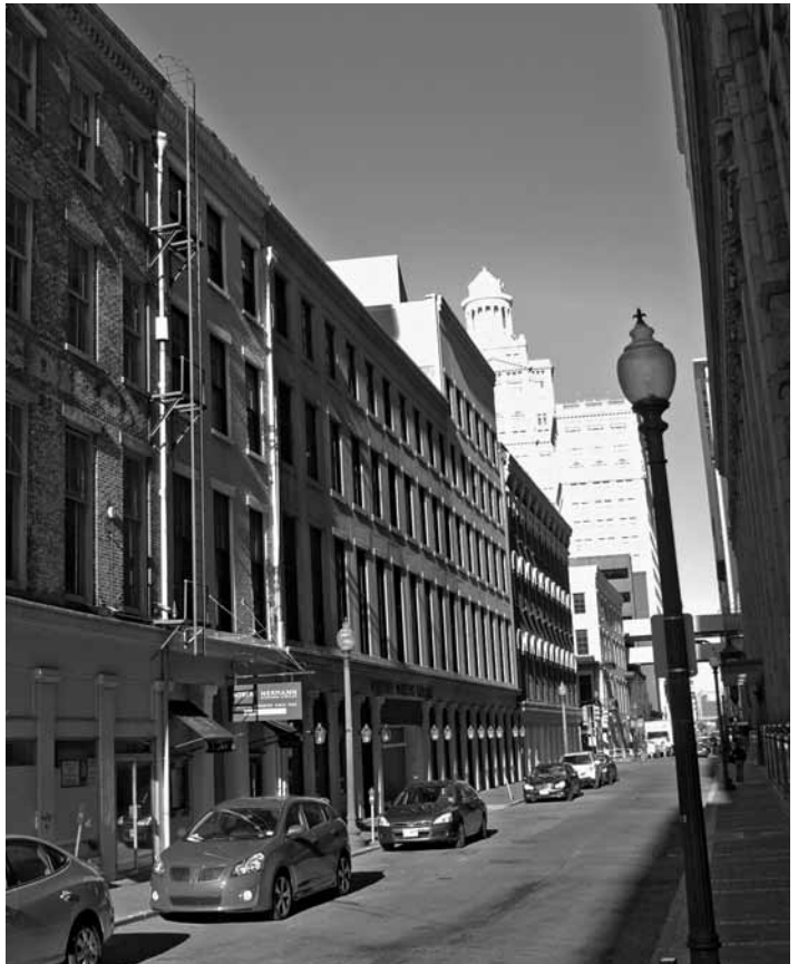
The parking garage on this New Orleans street was carefully designed to blend with the existing context.
