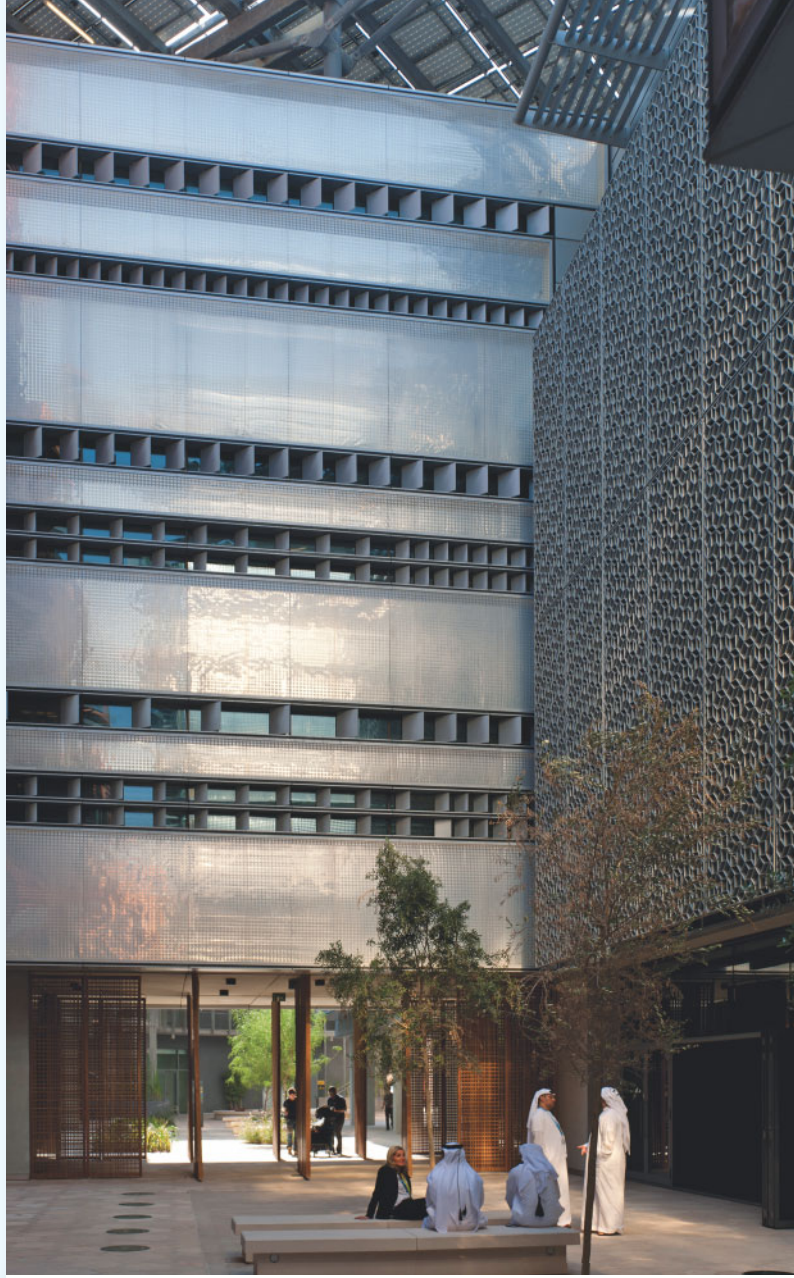
Interior courtyard of the Masdar Institute with wall openings of various sizes.
