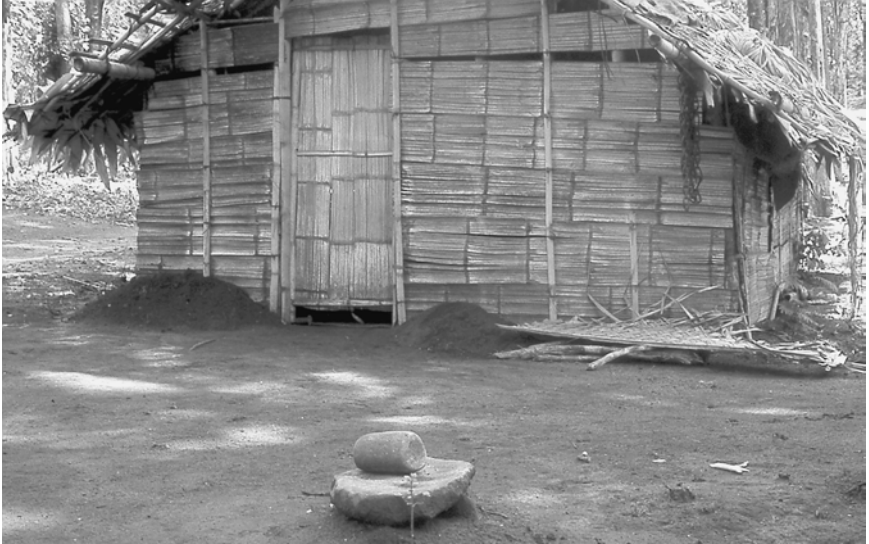
6-1. Bamboo structural members, thatch roof, and palm-leaf panels make up this tropical house from Tamilnadu, India. Unless the roof is soon repaired, the house will not be inhabitable for much longer (photo by the author, 1976).
