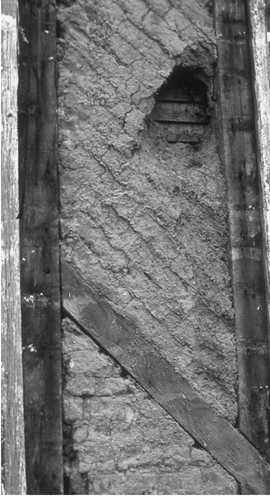
6-10. Layers of mud nogging placed at an angle determined by the cross-brace of the timber frame. The mud was added in rows with each row allowed to dry before the next row was applied. Ruins of a house near Columbia, Missouri (photo by the author, 1980).
