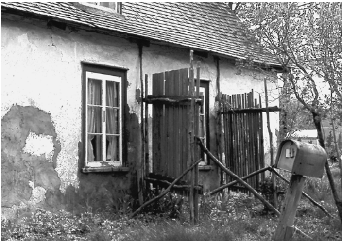
10-7. Simple wooden shields deflect the strong winter winds away from the windows of this old French-built cottage on the Ile d'Orleans, Québec (photo by the author, 1976).
