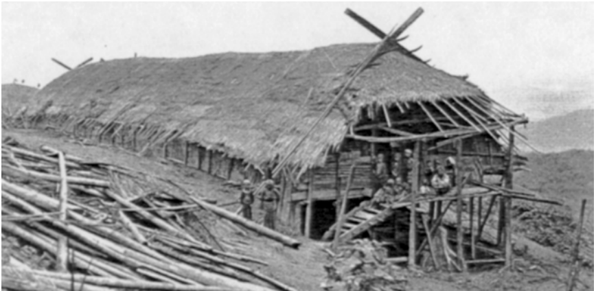
13-4. Stilt-supported longhouse from northern Myanmar (Burma). This particular structure, built on a slope, uses poles of unequal length to support horizontal floors (from Scherman 1915, tafel 8).
