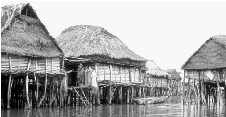
7-13. These thatch-roofed stilt houses are well above normal high tide in the coastal lagoon at Ganvie, Benin (photo by the author, 1975).
