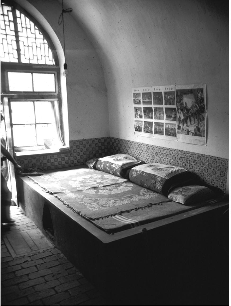
7-9. The interior of a loess cave. The adobe or stone bed (kang) occupies much of the space. The ceiling is vaulted and plastered. This cave even has electricity, as witnessed by light bulbs and radio (photo by the author, 1977).
