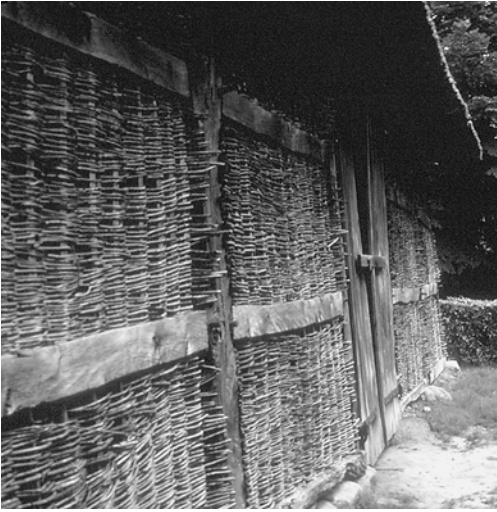
6-3. Wattle construction is one of the simplest and cheapest forms of building. The mud daub may be plastered on one or both sides of the wattle. These wattle panels are on a building in the Cloppenburg Open-Air Museum, Germany (photo by the author, 1983).
