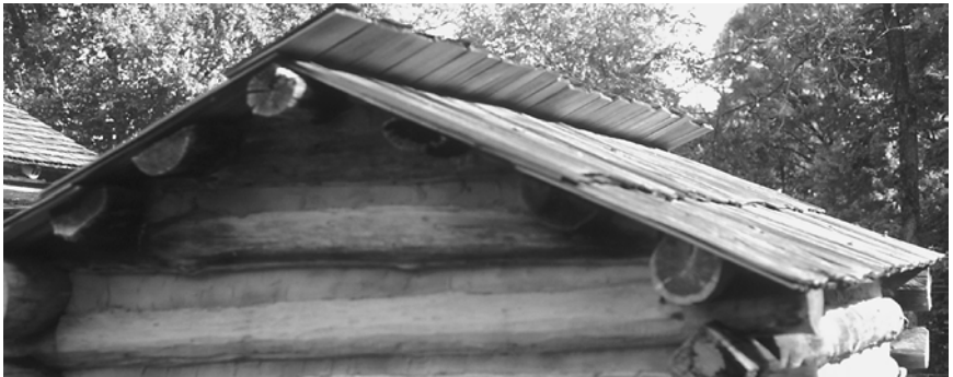
8-9. Reconstructed log building at New Salem State Park, Illinois. The ridge combing always slants upward and away from the direction of prevailing winds (photo by the author, 2002).
