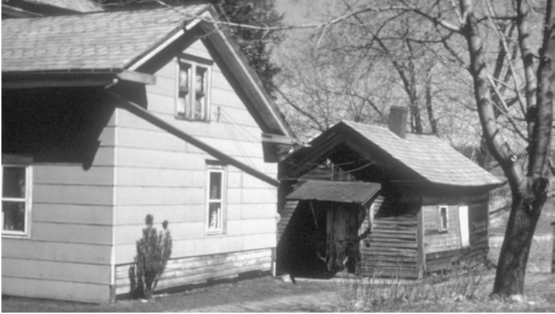
11-5. This small frame-and-log summer kitchen in northeastern Ohio is now very close to the house because the house wing is a later addition to the original structure (photo by the author, 1982).
