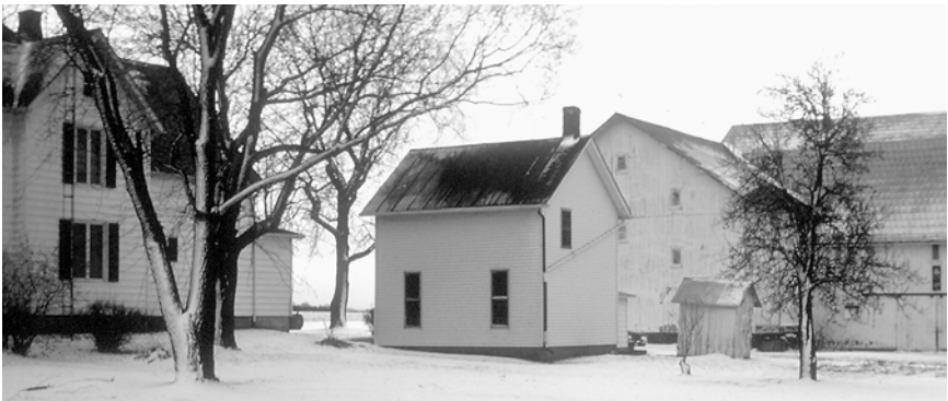
11-4. The gable window of the summer kitchen indicates a loft used for storage and perhaps earlier for sleeping during harvest, when additional hands were needed. The off-center location of the window probably indicates an interior-positioned gable chimney. The farm is located near Findlay, OH (photo by the author, 1982).
