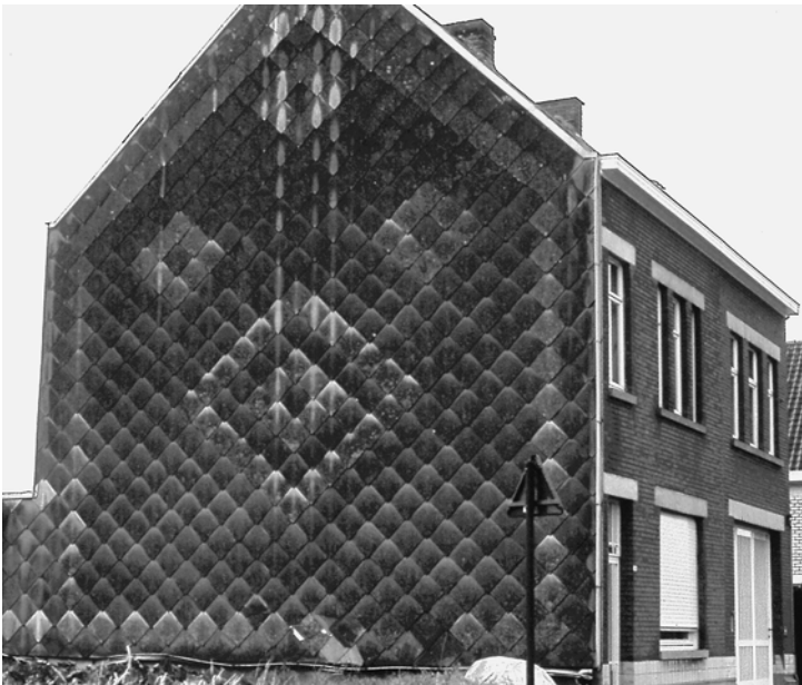
5-10. Slate-sided houses are found in several districts of Europe. This example is located near Brussels, Belgium. Only the gable wall facing the direction of prevailing wind and storm has been slated. Decorative patterns are formed by using slates of differing color (photo by the author, 1984).
