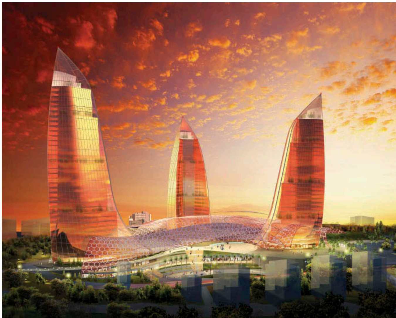
22.9 Baku Flame Towers: use of a standardised panel despite complex geometries and varying storey heights. Architect: HOK, London, UK Image: HOK, London, UK
