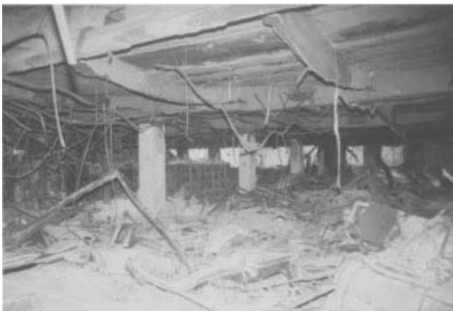
15.4 (right) Buckling of a column and beam flange in the 9-story WTC 5, and (above) sagging of a floor system in the 38-story One Meridian Plaza office building, due to fire
