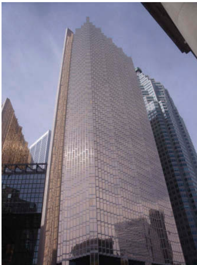
13.2 Once famous for the energy-saving gold coating to its glazing – gold worth more than $1 million at the time was used – Toronto’s Royal Bank Plaza (1979) is now cooled by the waters of Lake Ontario
