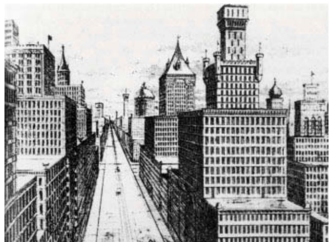
1.6 Louis Sullivan’s “High Building Question” of 1891 showed a proposal for ameliorating Chicago’s overbuilt condition—a setback skyscraper city that predicted New York’s Zoning Resolution of 1916 Image: Illustration from The Graphic , 1891
