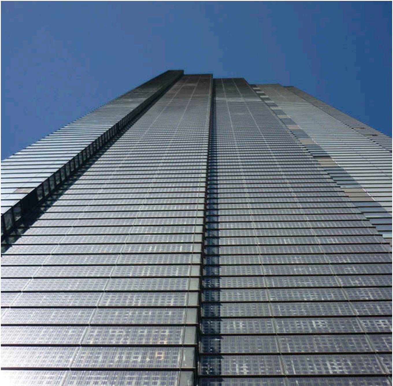
13.5 London's Heron Tower features a facade-mounted solar PV array Image: Kohn Pedersen Fox
