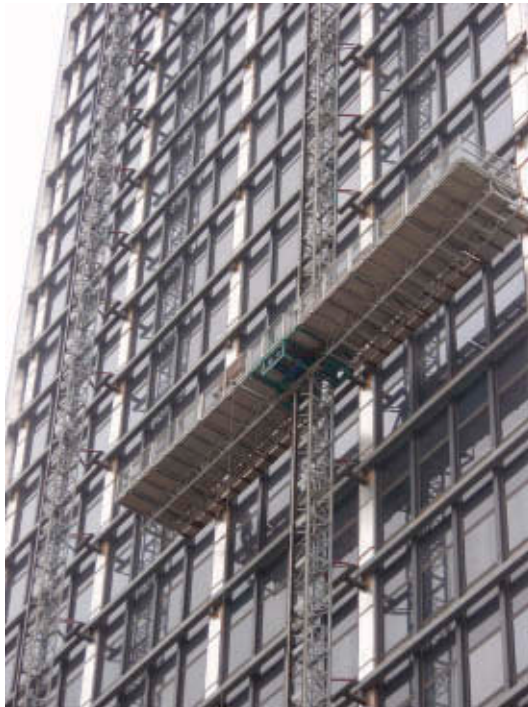
5.5 Construction photograph of the 36-storey 1 Indiana Square Image: Thornton Tomasetti Engineers
