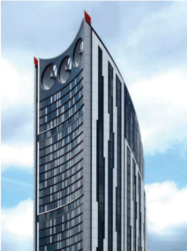
13.6 Integrated wind turbines are expected to generate 8 per cent of the energy needs of London's Strata SE1 Image: Yui Law/BFLS
