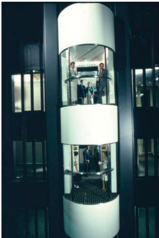
25.3 Double-deck lifts can be a very effective means of minimizing the size of the core in very tall buildings, but can struggle to cope with the noon peaks in modern offices Image: Otis
