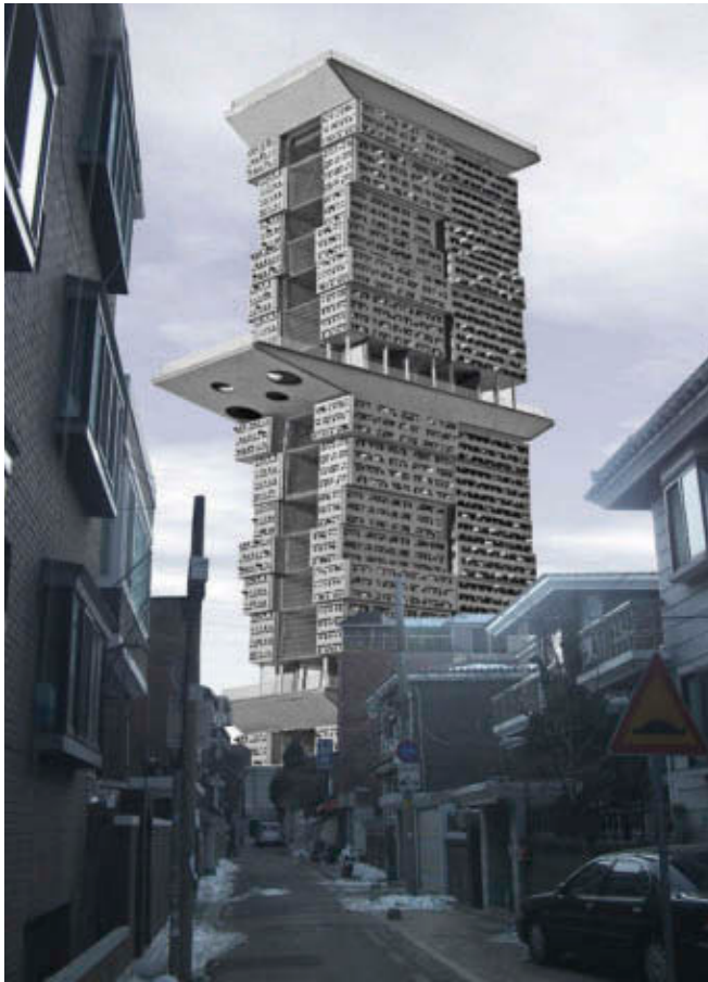
27.5 Gyoook Tower (education tower), Seoul. An example of a tall building designed with more envelope opacity, not as an all-glass transparent box. Gyoook Tower is aimed at developing a high-rise habitat to foster the education of Seoul's children
