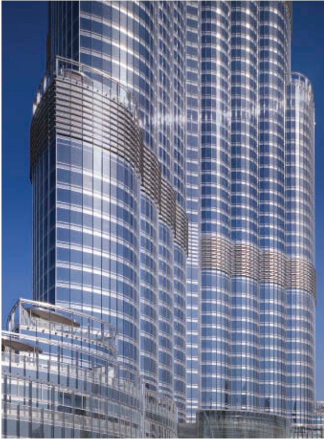
2.1 Cladding on the Burj Khalifa, Dubai Image: SOM/Nick Merrick
