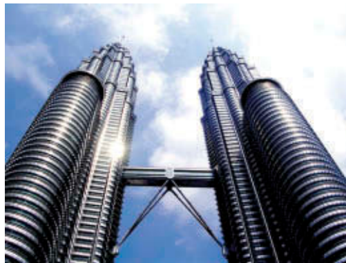
2.3 The skybridge on the forty-first and forty-second floors of the Petronas Towers, Kuala Lumpur
