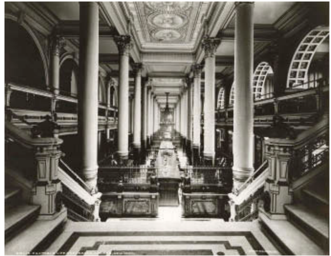
1.2 Gilman & Kendall, Architects and George B. Post, Equitable Building, business hall, New York, 1889
