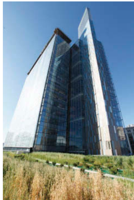
3.3 Manitoba Hydro Place
