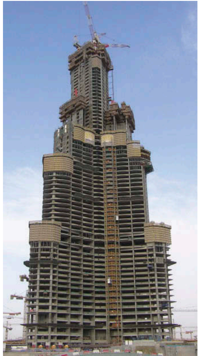
17.7 Self-climbing formwork and tower cranes
