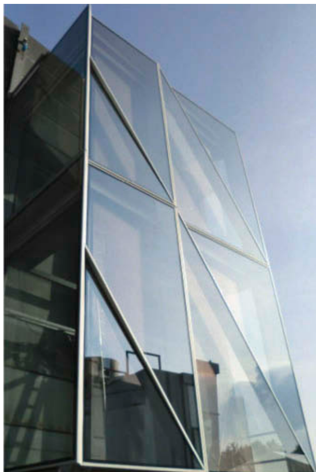
21.9 Sealed cavity system testing mock-up
