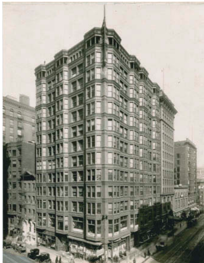
1.4 Holabird & Roche, Tacoma Building, Chicago 1886–89
