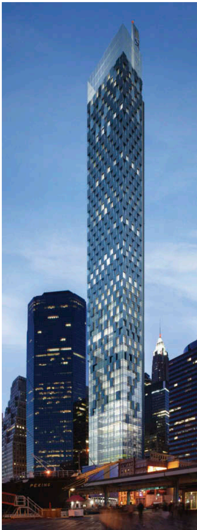
12.4 The mixed-use Water Street Tower, planned for Lower Manhattan, utilized BIPV (building integrated photovoltaics) to achieve almost net zero energy Image: COOKFOX Architects
