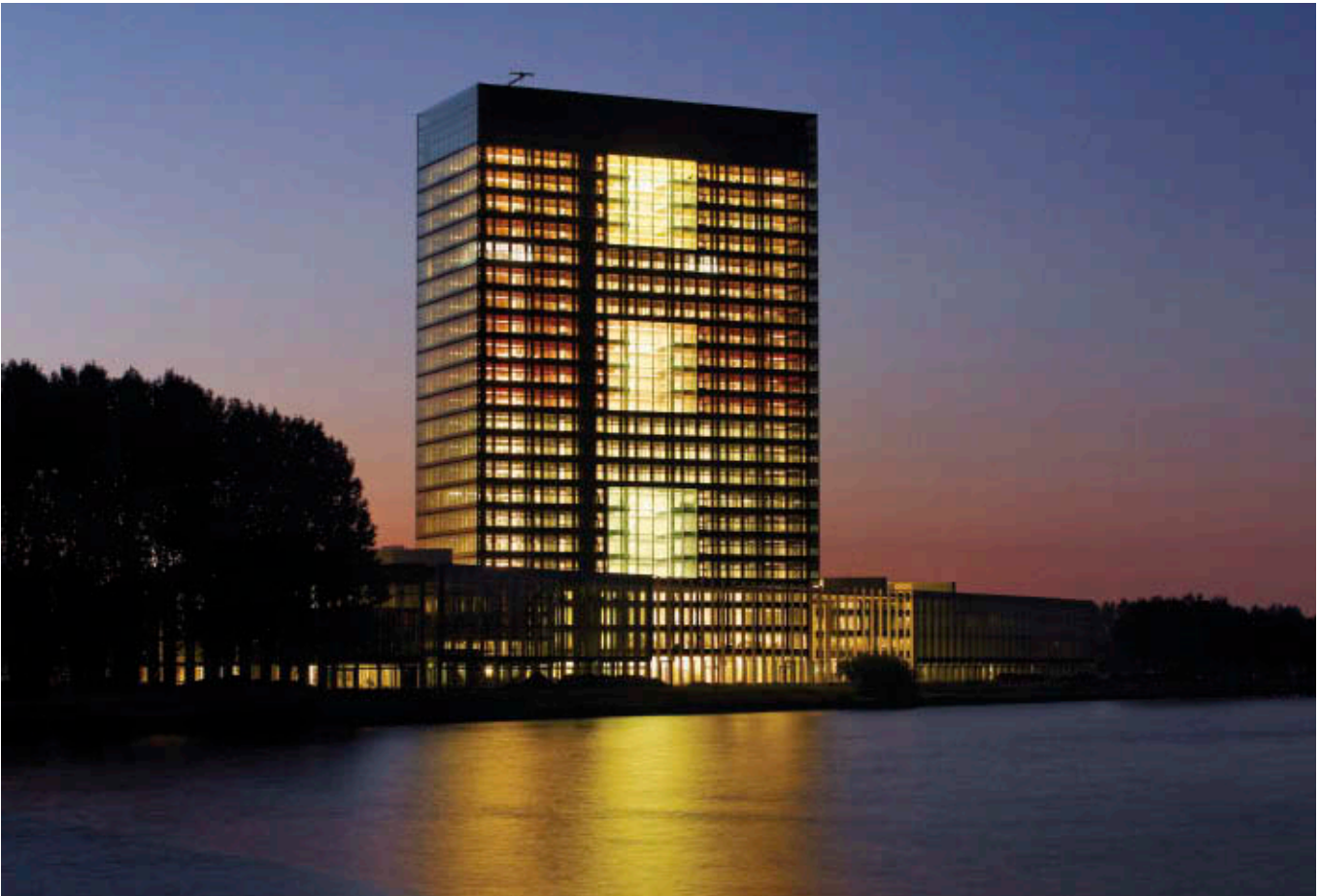
5.10 Westraven Tower in Utrecht. Tall buildings can pose special challenges in terms of logistical and regulatory concerns
