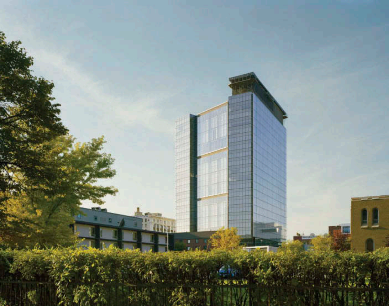
3.4 Manitoba Hydro Place
