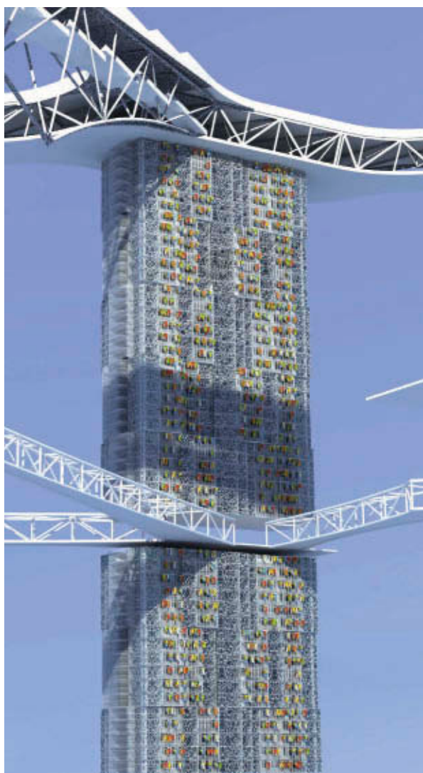
27.2 Swadeshi Tower (textile tower), Mumbai. An example of how there should be a variance in skin and texture throughout a building, depending on the responsibilities of each different horizon within the form. In the Swadeshi Tower, inspired by the Dobi Ghat washing areas in Mumbai, textiles are integrated into the building aesthetics and materiality through the application of a weave-like cladding to the facades, providing residential spaces with shading from solar gain and privacy Image: © CTBUH/IIT, Nishant Modi and Hiren Patel
