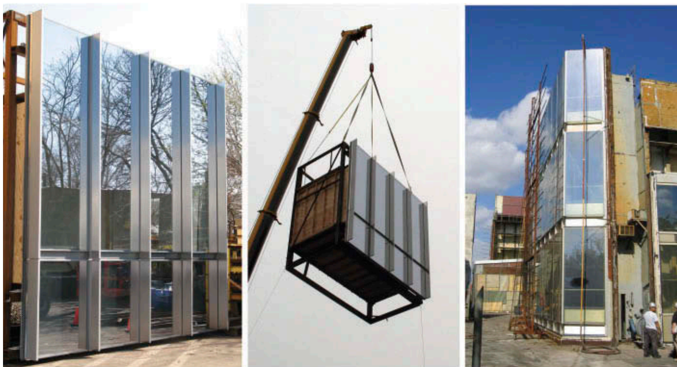
21.8 Visual curtain wall mock-ups test the visual aspects of the wall and are often hoisted onto a crane to simulate final viewing angles; performance mock-ups test the system's weather tightness and structural integrity
