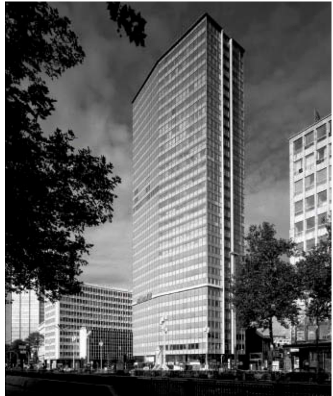
5.6 Madou Plaza, constructed in 1965 Image: Marc Detiffe
