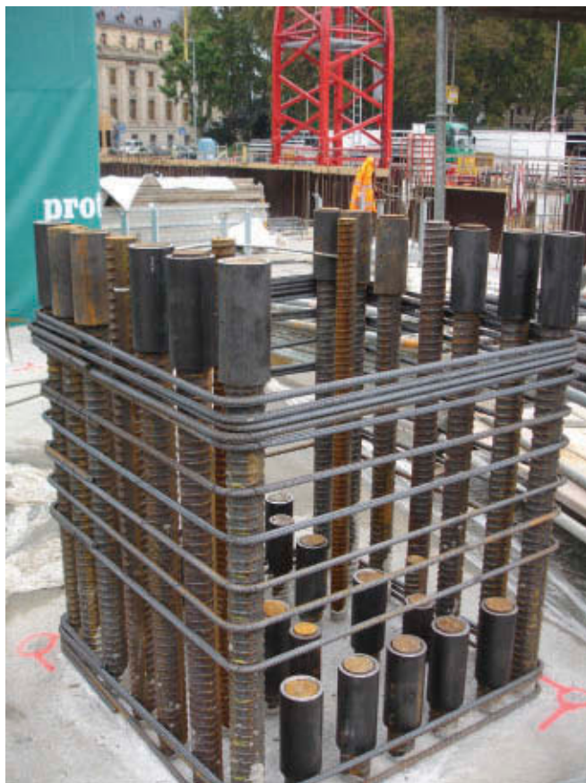
14.7 (left) High-strength, large diameter bars to reduce reinforcement congestion in compression-controlled sections. (top) Standard reinforcement, 6% (bottom) High-strength, large diameter reinforcement, 6% Images: Courtesy Buro Happold
