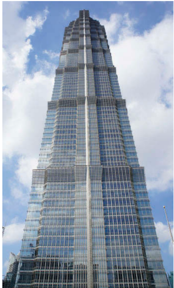
5.3 Jin Mao Tower, completed in 1998, was able to make a 20 percent energy saving by recommissioning its mechanical systems
