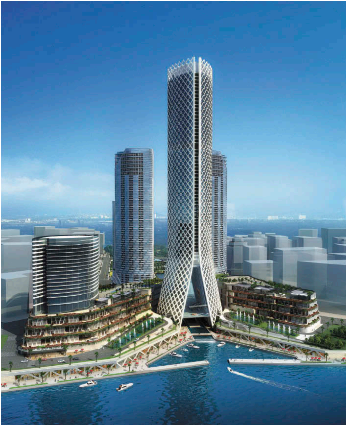
16.10 The original Tameer Tower design featured a diagrid exterior with sloping members acting as both columns and braces. Rendering Image: Gensler
