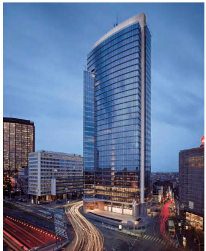
5.7 Madou Plaza after refurbishment Image: ASSAR Architects
