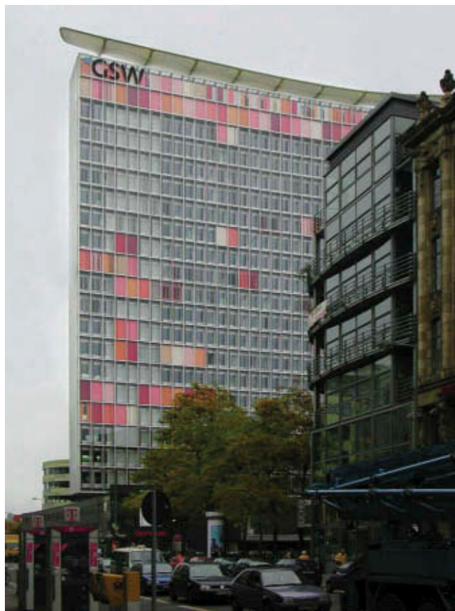
12.3 Retrofitting older tall buildings will be one of the most important sustainability strategies in many cities. The GSW Building in Berlin is a highly successful example of adding a new high performance envelope to an existing tall structure. The south façade features occupant adjustable sliding panels that are part of a system to modulate light and airflow
