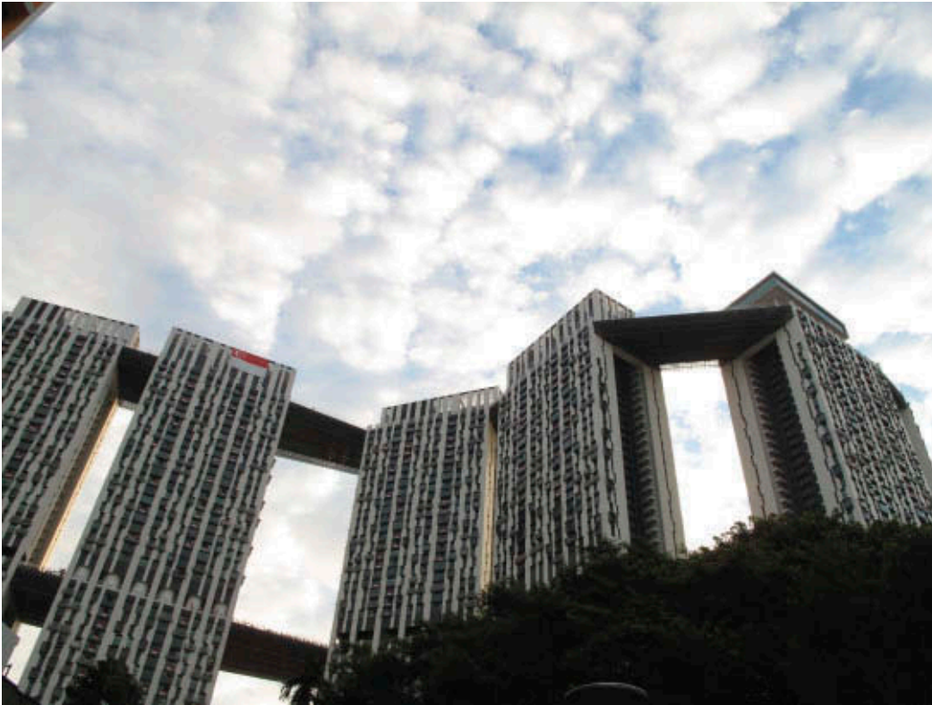
10.6 Sky gardens in the Pinnacle project, Singapore, provide a series of elevated social spaces that create pedestrian permeability Image: Arham Daoudi
