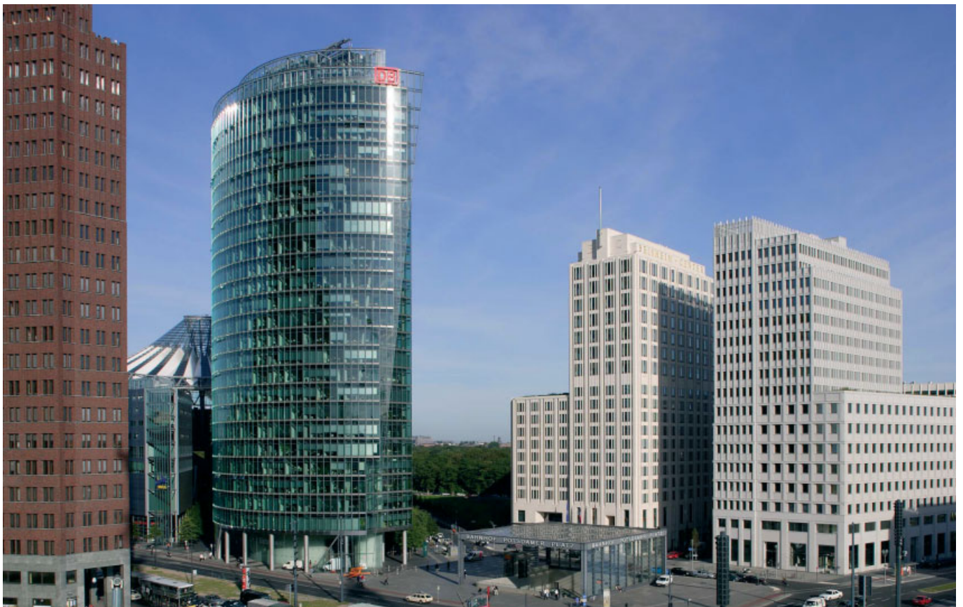
The Beisheim Center, Helmut Jahn's Sony Center and Hans Kolhoff's Potsdamer Platz No 1 all point towards the centre of the Platz.
