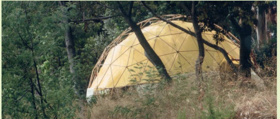
John Zerning's transportable holiday home, designed to fit in a suitcase: timber (birch) dowel and nylon parachute (total weight 41 kilograms/90 pounds) first constructed 1972. See Δ Vol XL III 2/1973.
