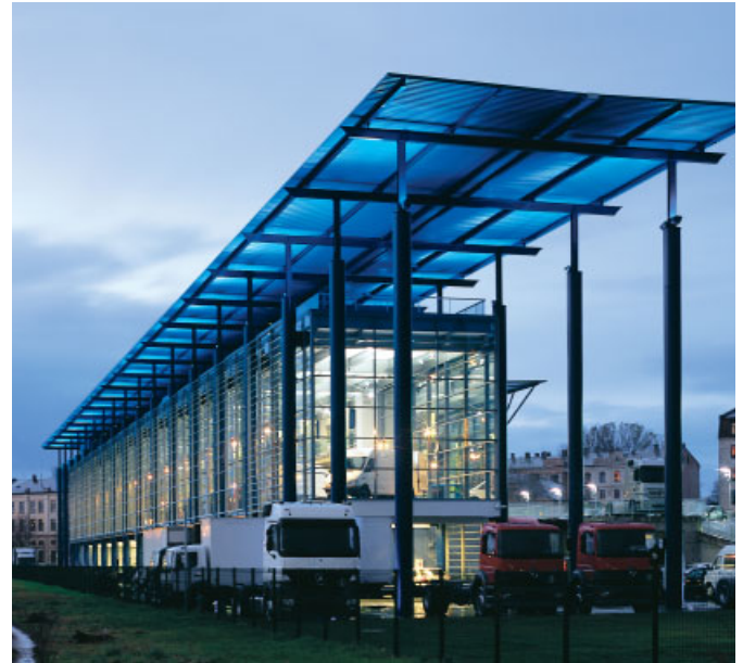
Silis, Zabers & Klava, Mercedes-Benz trade centre, Krasta Street, Riga, 2004 Conflating the company's powerful image with the genius loci of this showcase of Riga, by architects Andris Silis and Peteris Klava, the Mercedes-Benz building has become the true landmark of this traffic junction.
