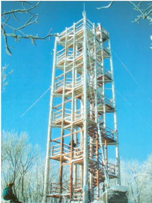
Vlastimil Dohnal, Observation Tower, Vel'ká Homol'a Hill, Slovakia, 2001 The latest Slovak version of a landscape dominant. The open wooden structure of this observation tower was designed by older-generation architect Vlastimil Dohnal and was a finalist for the ARCH 2002 prize awarded by the Slovak ARCH magazine.
