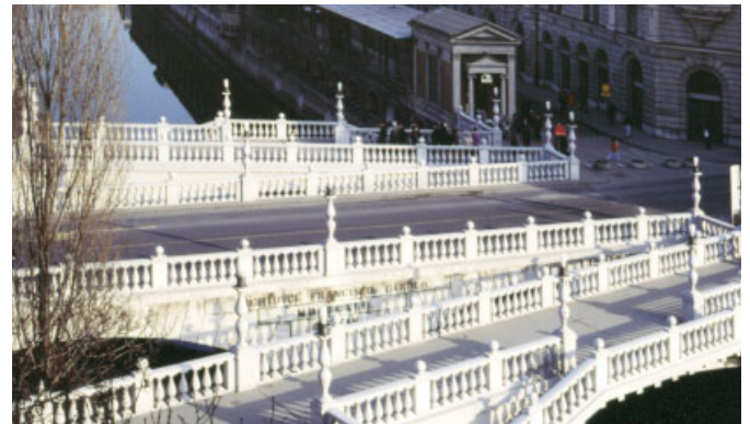
Jože Plečnik, The Three Bridges, Ljubljana, 1932 Instead of replacing the old bridge over the Ljubljanica River with a larger one, Plečnik preserved the existing one and added two smaller pedestrian bridges on either side of it. This solution was not only cheaper, but also enabled him to take the large Preeren's Square over the water towards the town hall. He said: 'We should not destroy what our fathers have done well.'
