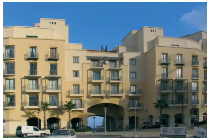
One of the entrances to the Portomaso apartments.
