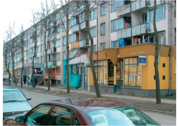
Typical Soviet block, Siauliai city centre, 1975 During the Soviet period, housing lost its indigenous identity and came to resemble a giant ghetto with depressing spaces, architecture and lifestyles.
