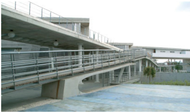
Chrysanthos Chrysanthou and Eraclis Papachristou, Student housing, University of Cyprus, Aglantzia, Nicosia, 2004 An arrangement of 'blocks' connected through a series of ramps creates a variety of in-between spaces.
