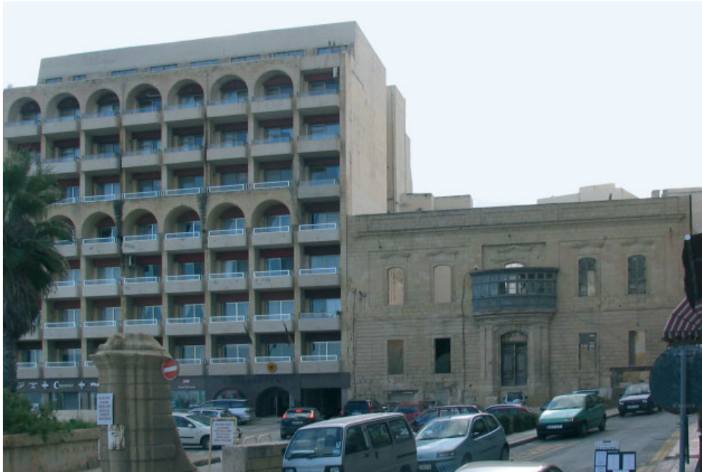
Multistorey buildings facing Ghar id-Dud Bay.
