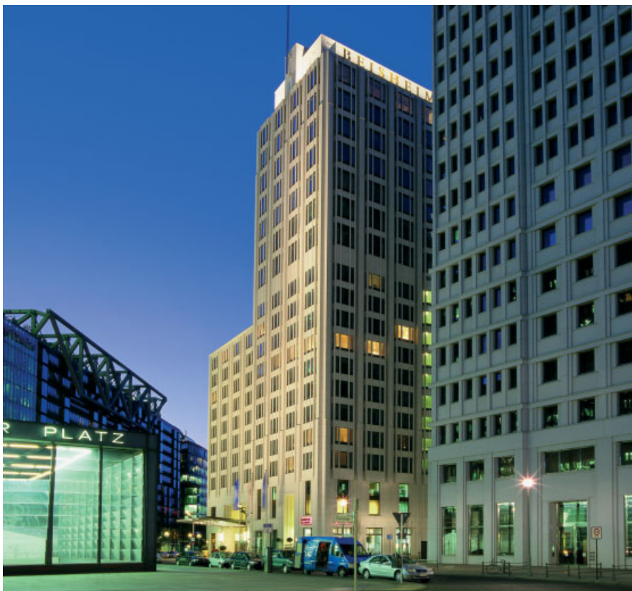
Hilmer & Sattler und Albrecht, Beisheim Center, Potsdamer Platz, Berlin, 2005 Above and opposite top: The towers of the Chicago School-inspired Beisheim Center, which completes the Potsdamer Platz development.
