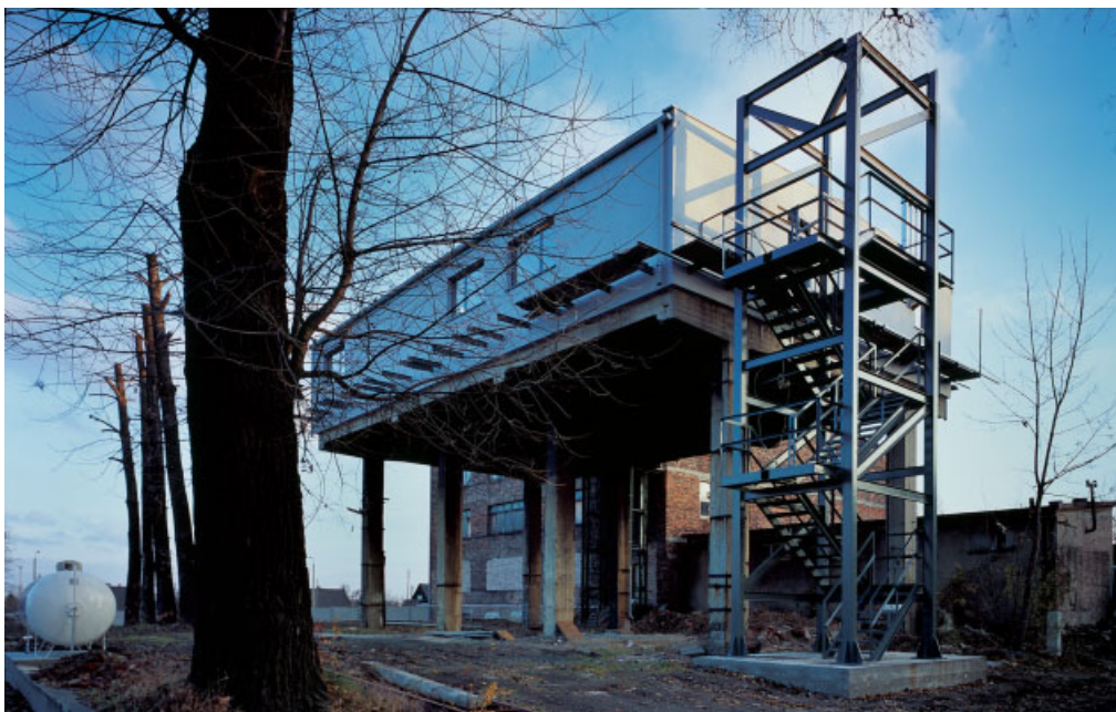
medusa group, Bolko Loft, Kruszcowa Street, Bytom, 2003 medusa group partner Przemek Łukasik converted this derelict mine-lamp depot into his own house – as witty as it is unexpected. View of the stairs and the former coal-mine tower.
