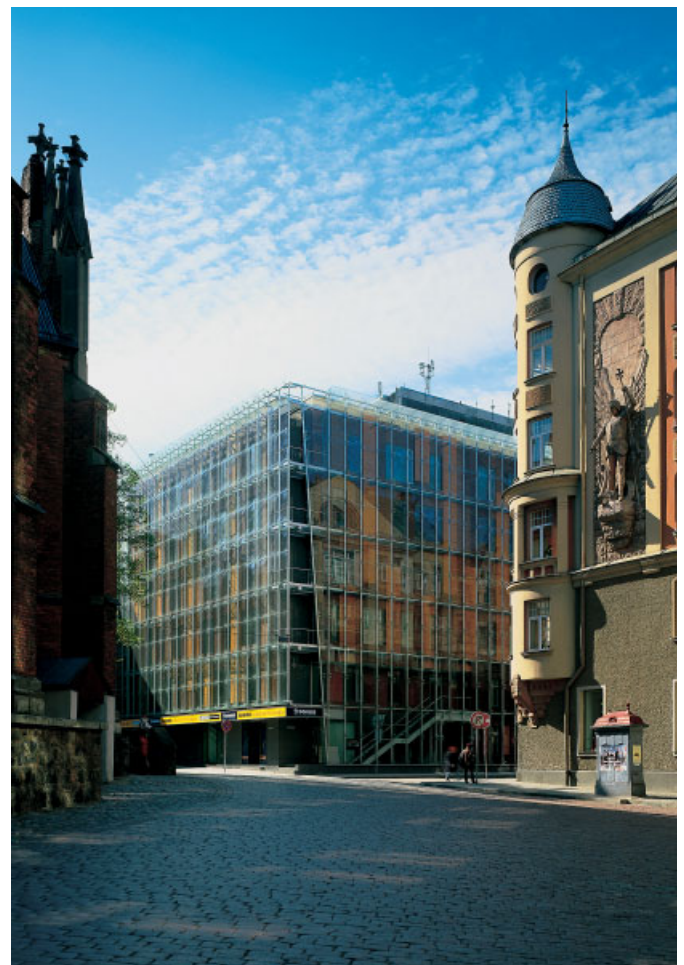
Arhis architects, Gertrudes Centrs office building, Baznicas Street, Riga, 2003 The inclusion of fragments from the original wooden building on this site posed a risk to the architects (Andris Kronbergs, Brigita Bula, Eduards Beernaerts and Vilnis Schlars), who had to bow to pressure from conservationists. The sophisticated double-skin facade includes old and new wood.
