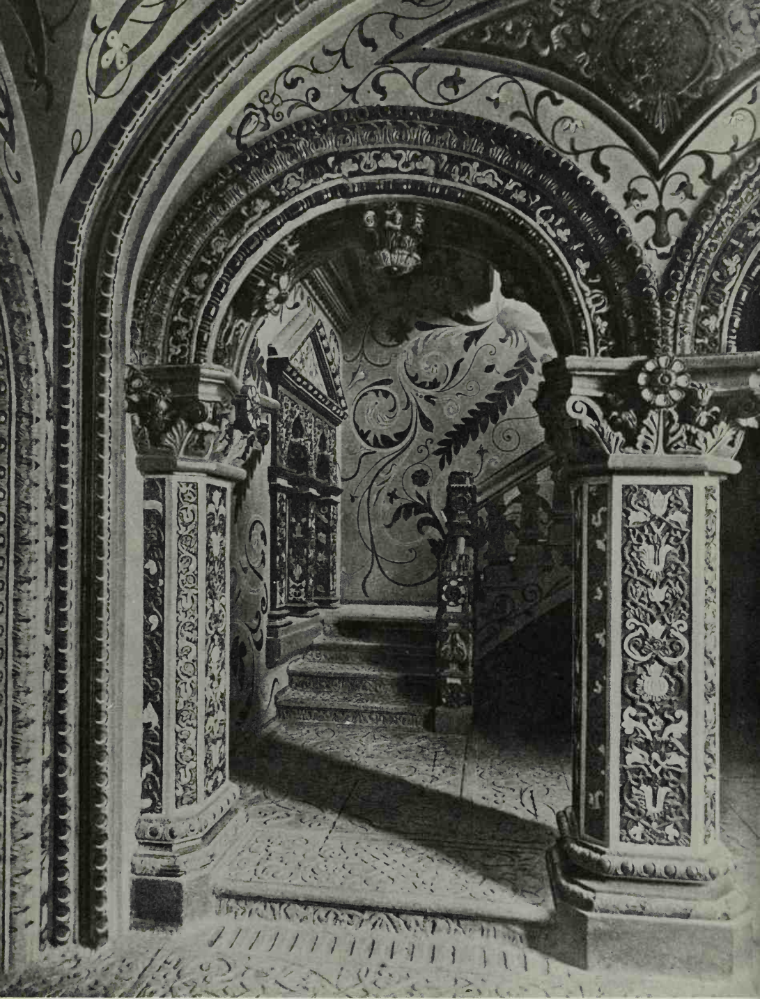
PLATE 112: Stairway, Terem Palace, Kremlin, Moscow, 1635.
