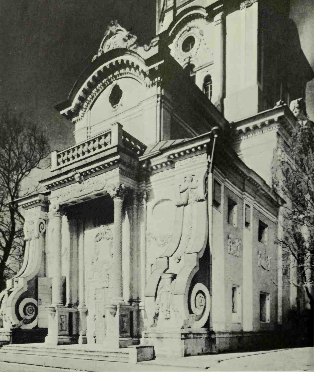
PLATE 99: Church of the Archangel Gabriel (Menshikov Tower), Moscow, main entrance, 1705-1707.
