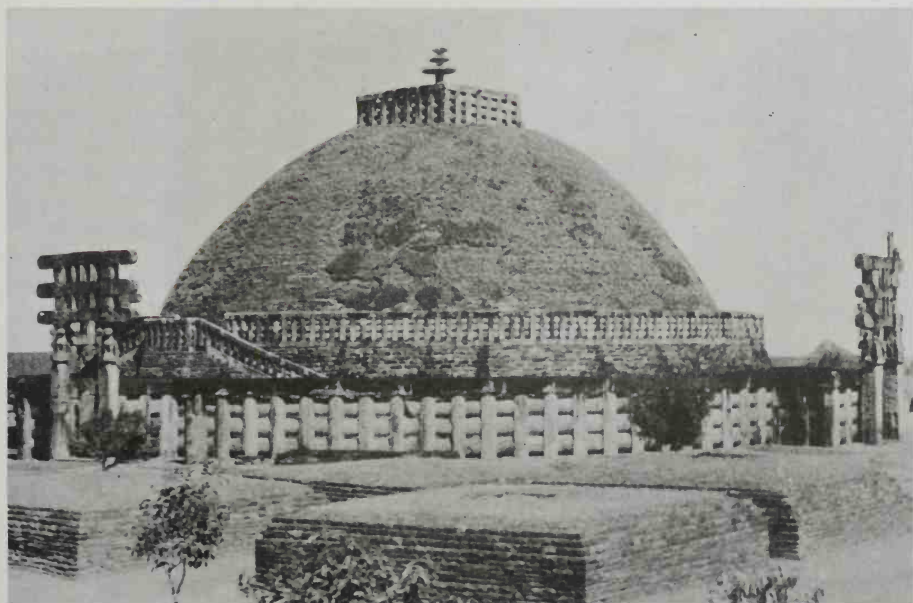
41. Sāñchī, Great Stupa, from the north-east
