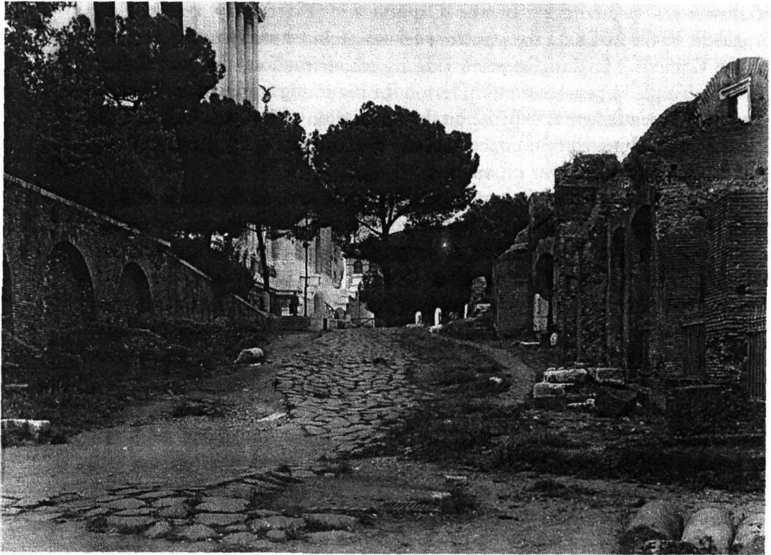
Figure 114. View from the Forum Romanum looking northwest up the Clivus Argentarius. Photo: Fototeca Unione AAR 5900.
