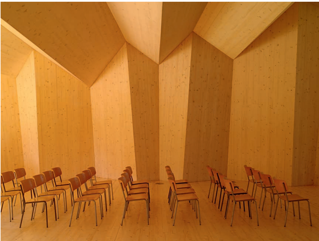
Illustration 13.25 Temporary St-Loup Chapel. The chapel profile rises from the entrance to the chancel, and the highly irregular folding patterns are used to address acoustic and lighting design objectives; the panels are all of different shape and were fabricated and milled in a factory, then precisely connected together by folded steel plates along the creases and simply cap screwed, producing quite an economical and quick method of construction that was nonetheless visually distinctive.
