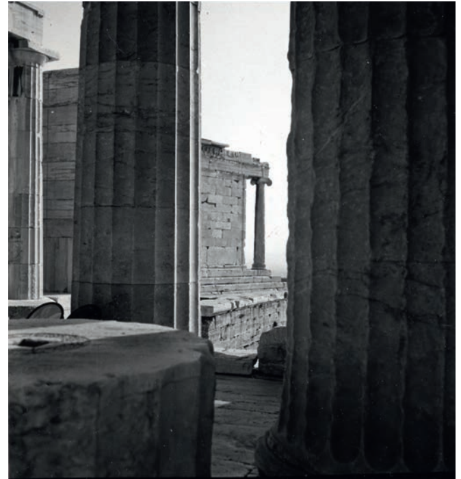
Illustration 8.4 Temple of Nike at Acropolis, Athens, Greece (453 bc). View between the Propylaeum's columns. Architect: Kallikrates.
