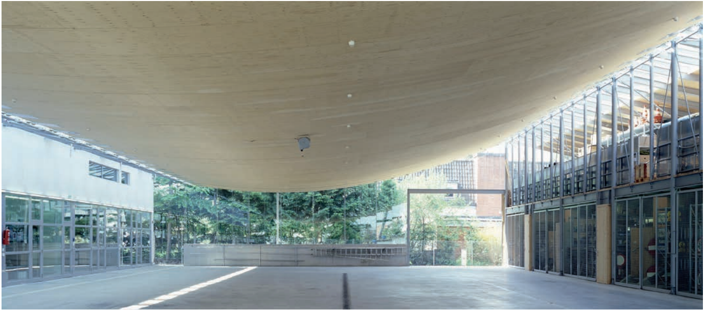
Illustration 11.24 Municipal garage, Hohenems, Austria (2000). Distinctive suspended wood panel roof above exterior municipal garage's work space. Architect: Reinhard Drexel. Structural engineer: Merz, Kaufmann und Partner.
