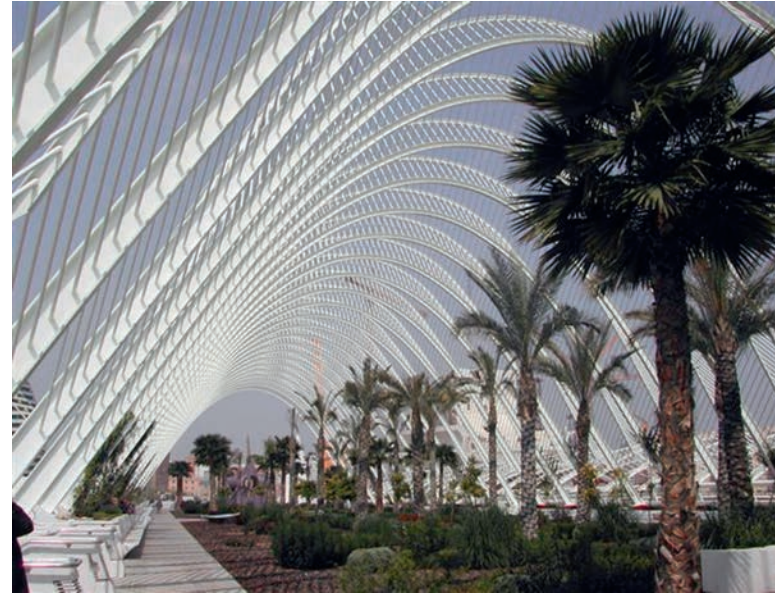
Illustration 12.16 L'Umbracle, City of the Arts and Sciences, Valencia, Spain (2002). Catenary (nearly parabolic) profile of light steel arch ribs corresponds to uniform-along-the-arch loading condition produced by self-weight of ribs and cross bars, resulting in “pure” compression forces along the arch. Architect and structural engineer: Santiago Calatrava.
