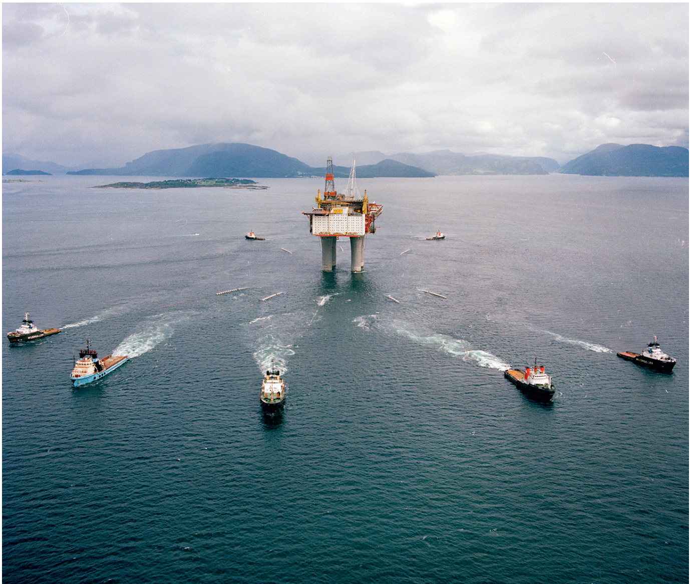
Illustration 4.14 Pulling of the Condeep oil platform in the North Sea (1987). The tugboats' lines of forces will sum up to help establish the speed and direction of the platform's movement through the water.
