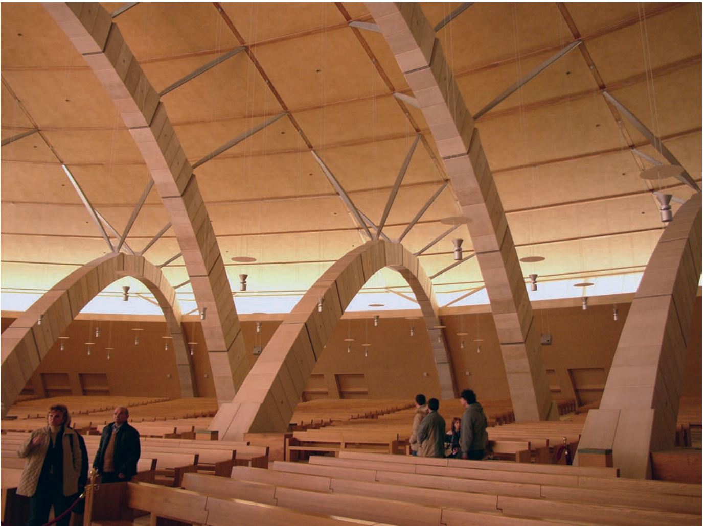
Illustration 12.4 Padre Pio Church. Arched stone ribs vary in height and span. Thin V-configured steel struts serve to raise the timber-lined roof above arches and side wall.
