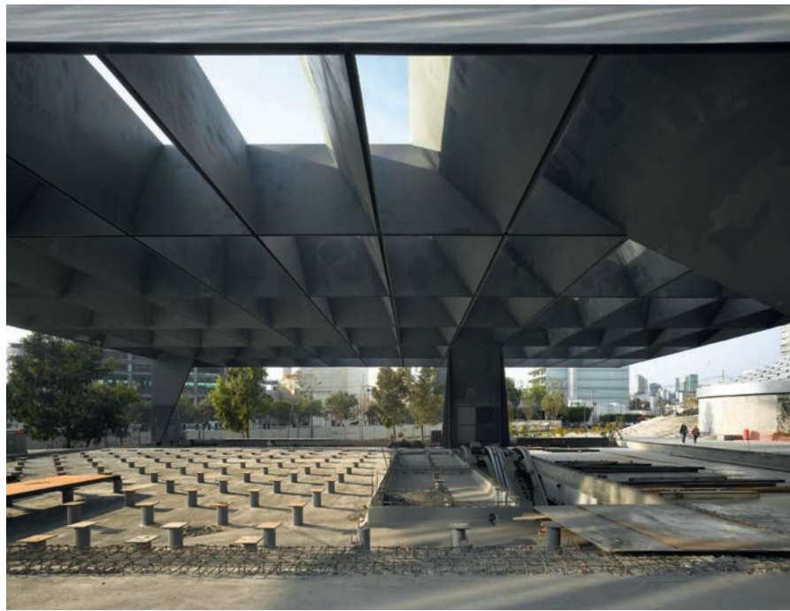
Illustration 7.41 Telcel Theater, Mexico City, Mexico (2012). Distinctive two-way grid of angled steel plate beams acts as an urban marker for the location of a completely underground theater; also acts as a sun-shading canopy for the entrance. Architect: Ensemble Studio. Structural engineer: Colinas de Buen.
