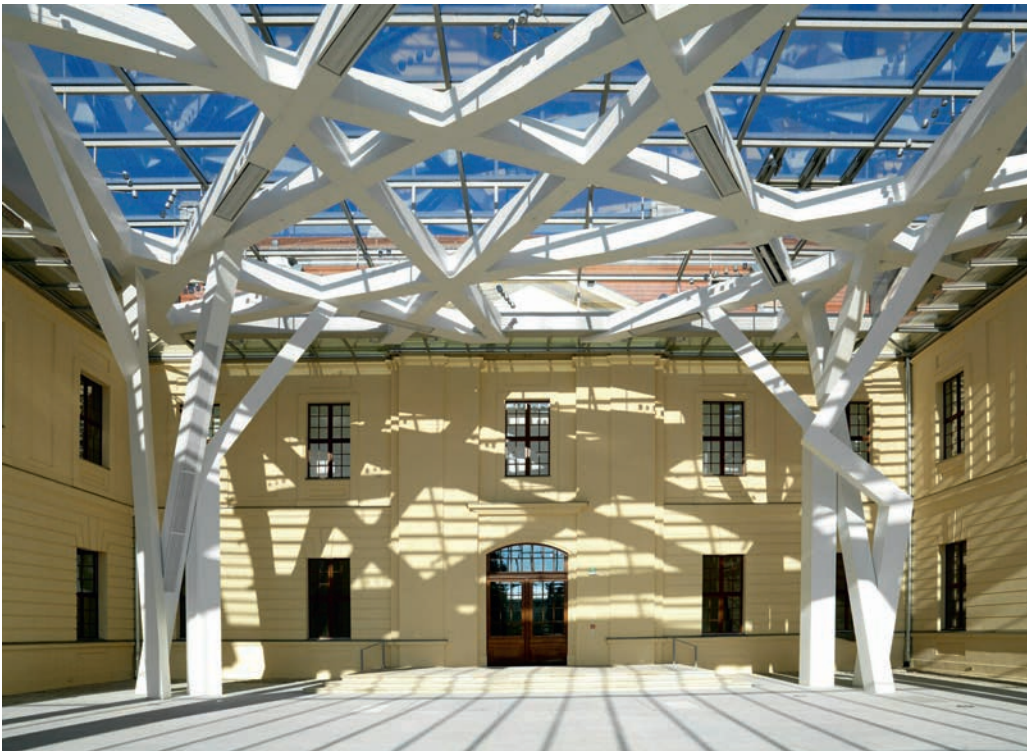
Illustration 7.5 Glass Courtyard, Jewish Museum. Irregular and skewed beam grid picks up on geometry of museum. Columns also branch out in multiple directions and unconventional forms, reducing beam grid spans and potential stress concentrations.
