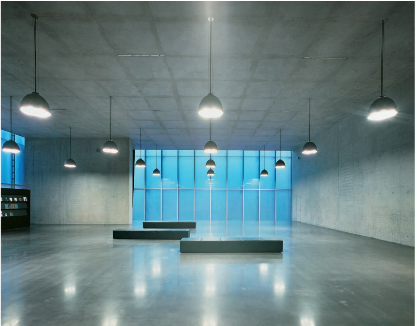
Illustration 2.5 Kunsthau Bregenz. Building's vertical structure consists of concrete load-bearing walls; these are in full view in the interior spaces.
