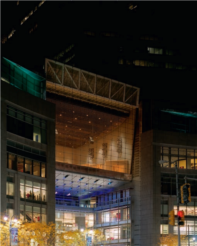
Illustration 6.3 Time Warner Center. Glass wall is suspended from truss above performance space; exterior cable net is also anchored at sides and bottom edges.
