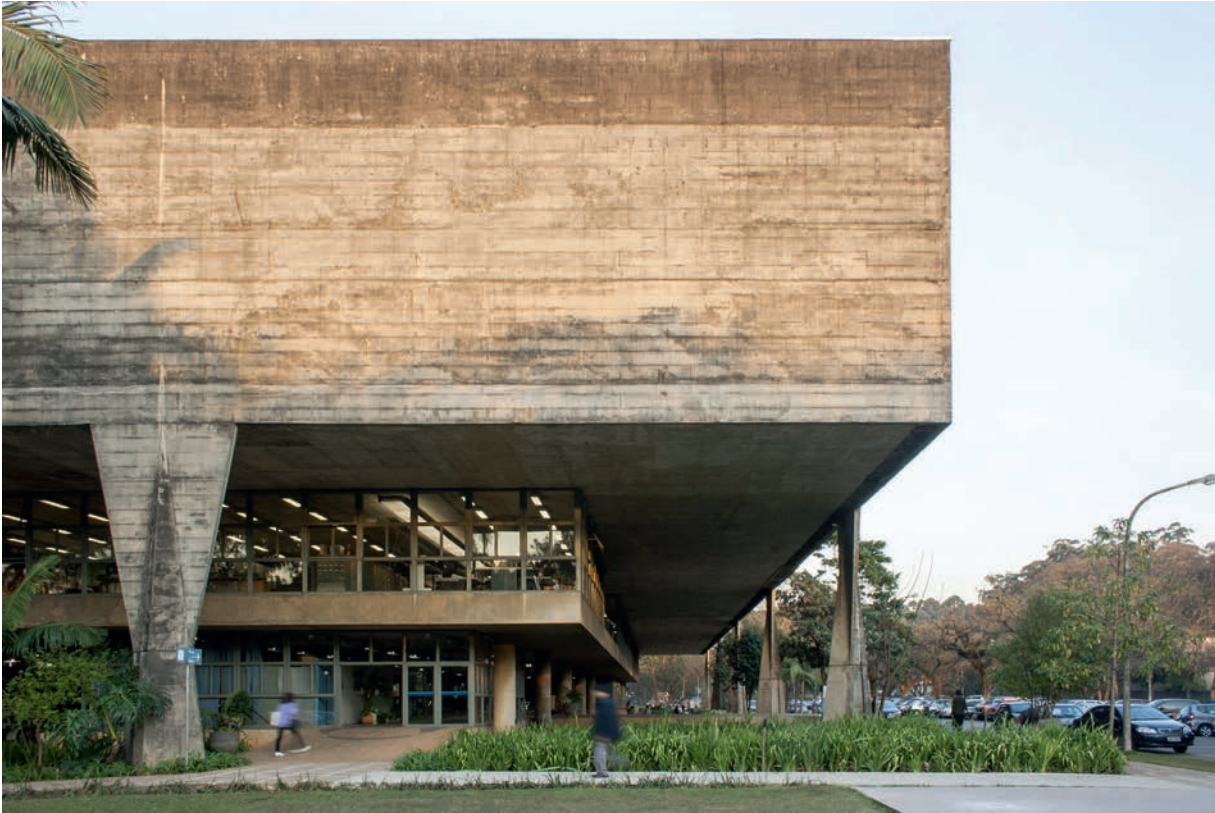
Illustration 5.20 Faculty of Architecture and Urbanism, University of São Paulo, Brazil (1968). A rough concrete finish left by formwork boards reflects a certain "honesty" of expression about the liquid-to-solid making of this material, as does – in this case – the sculpted/plastic form of the column supports for the large elevated volume. Their common surface finish also serves to unify these very different elements of the building structure. Architect: João Vilanova Artigas and Carlos Cascaldi. Structural engineer: Escritorio Figueiredo Ferraz.
