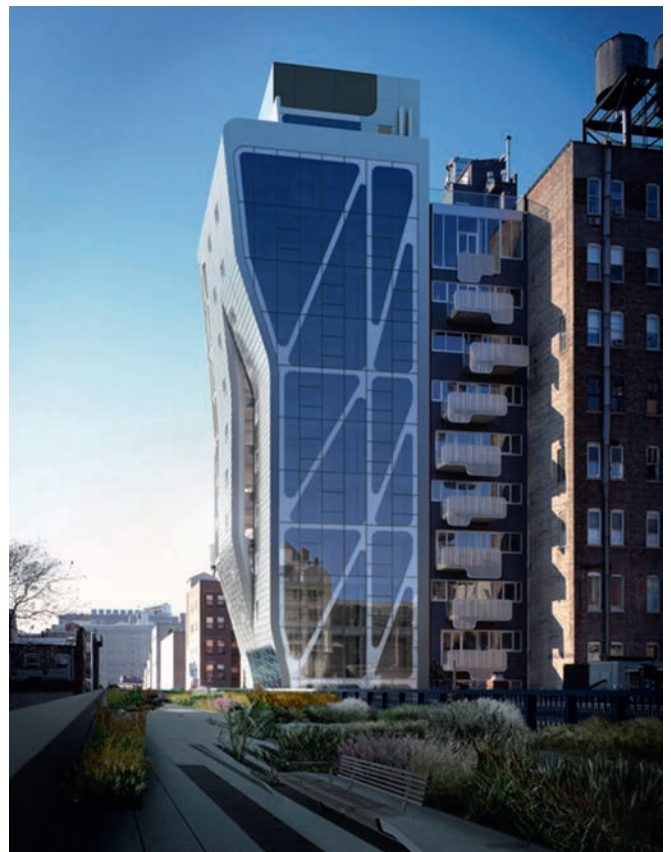
Illustration 10.22 Highline 23, New York City, NY, USA (2009). Multistory diagonals are emphasized as part of a braced frame system for resisting lateral loading on narrow building site. System provides a distinguishing feature while also allowing for views of the elevated urban parkway. Architect: Neil M. Dinari Architects. Structural engineer: Desimone Consulting Engineers.
