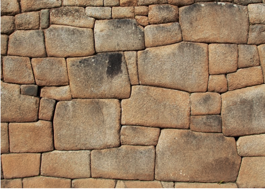
Illustration 5.23 Inca stone wall, Peru (fifteenth century). Large stones, with their inherent irregularities, were finely worked to fit and dry stacked without mortar.
