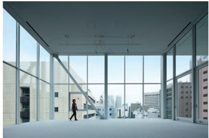
Illustration 2.12 Shibaura Office Building. Skeletal/line element system minimizes member dimensions, creating a sense of openness from the inside toward the surrounding urban context.
