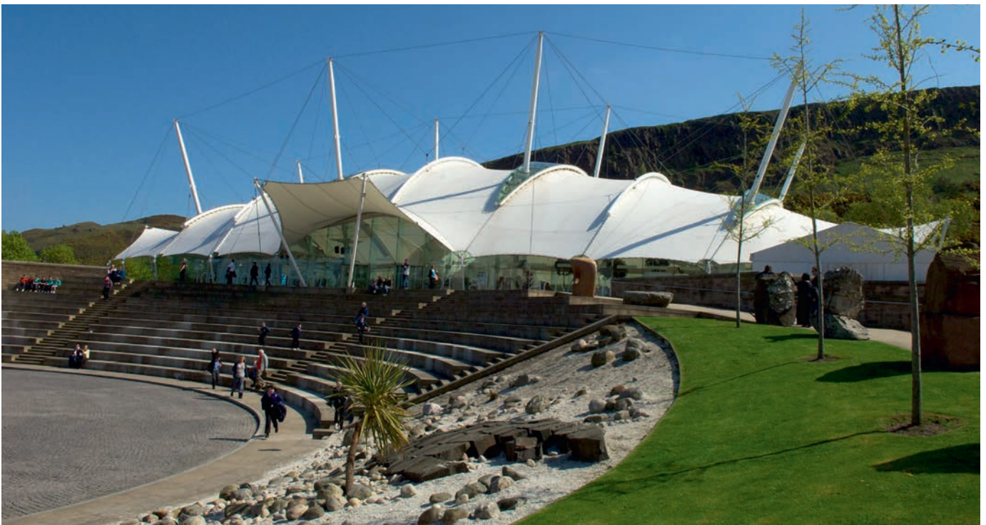
Illustration 11.43 Our Dynamic Earth, Edinburgh, Scotland, UK (1999). Steel mast-supported membrane stretched between curved ribs. Membrane can be seen to be doubly curved everywhere, but curvatures are modest, thereby increasing the magnitude of membrane forces and of the fabric strength required. Architect: Michael Hopkins and Partners. Structural engineer: Arup.
