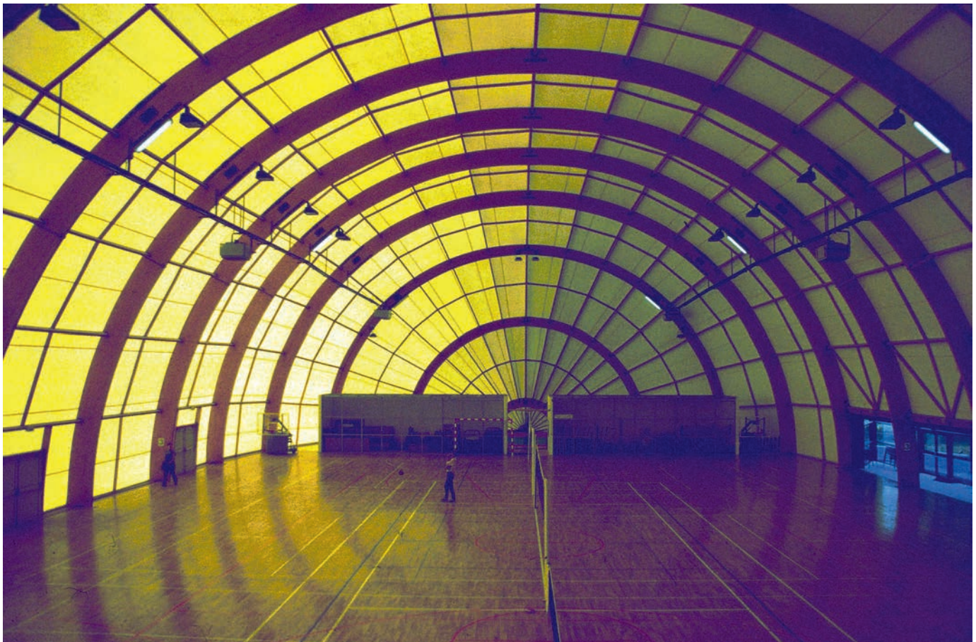
Illustration 12.29 Sports Hall, École d'Ingénieurs ESIEE, Marne-la-Vallée, France (1987). Semicircular arch profile subject to uniform load: rib thickness needs to account for bending as well as compression. Architect: Dominique Perrault Architecte (DPA). Structural engineer: B.E.F.S. S.A.
