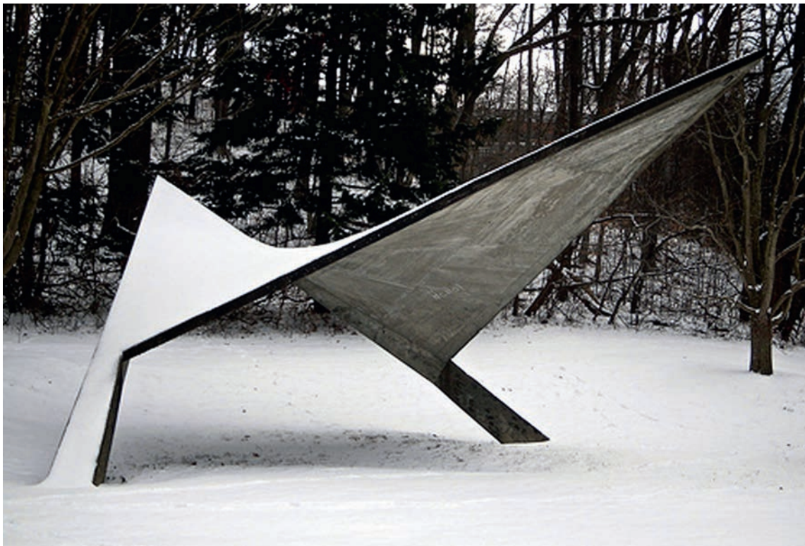
Illustration 13.36 Hypar Shell, Cornell University Arboretum, Ithaca, NY, USA (1975). “Classic” form of doubly curved hyperbolic paraboloid concrete shell. Cornell student project. Faculty advisor: Professor Donald Greenberg.
