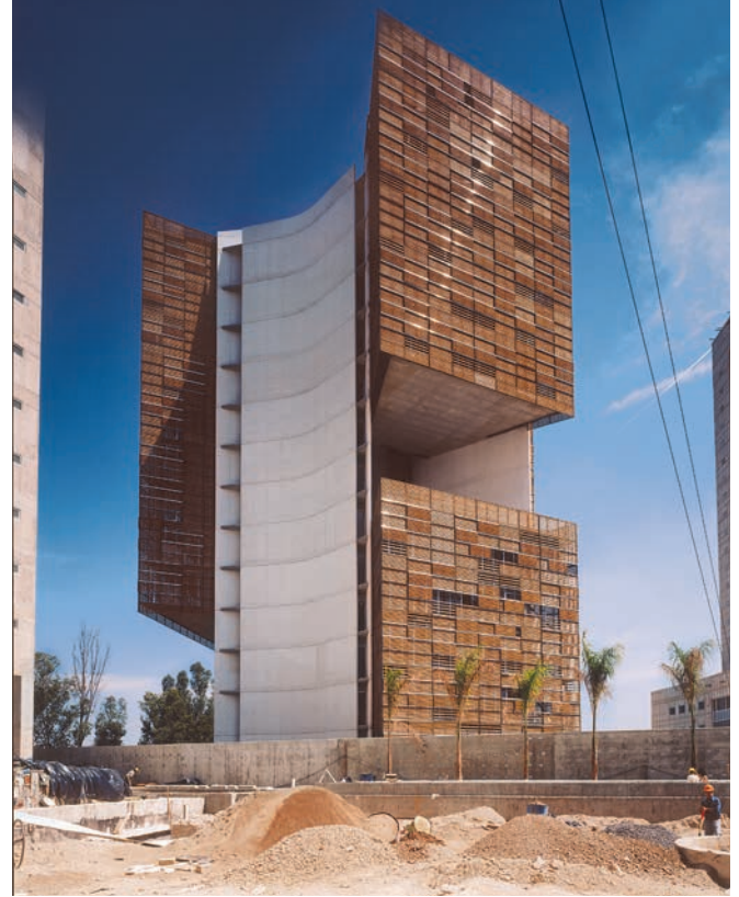
Illustration 10.5 Torre Cube, Guadalajara, Mexico (2005). Trio of tall, thin, reinforced concrete shear walls resist lateral loads, carry gravity loads from the wood-clad cantilevering volumes of residential space, and act as service/elevator cores. Architect: Estudio Carme Piños. Structural engineer: Luis Bozzo.
