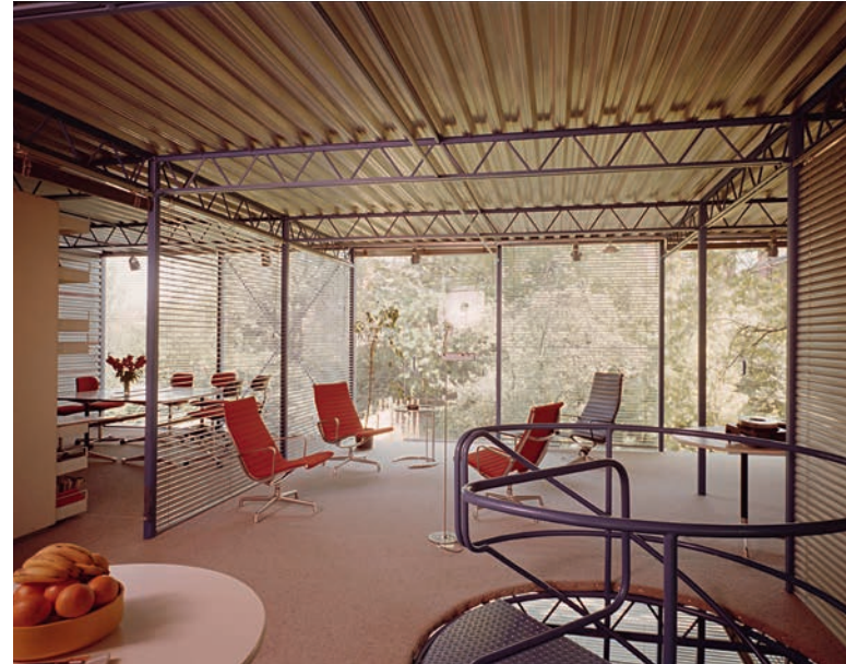
Illustration 9.17 Hopkins House, Hampstead, UK (1976). Interior view of the house, with Warren-truss-like configuration of open-web steel joists left in full sight. Diagonals' constantly changing orientation will cause them to alternately be in tension and compression. Relative openness of these trusses allows light to penetrate deep into the living space, and prevents the visual interruption that solid beam webs would cause. Architect: Michael Hopkins & Partners. Structural engineer: Anthony Hunt Associates.
