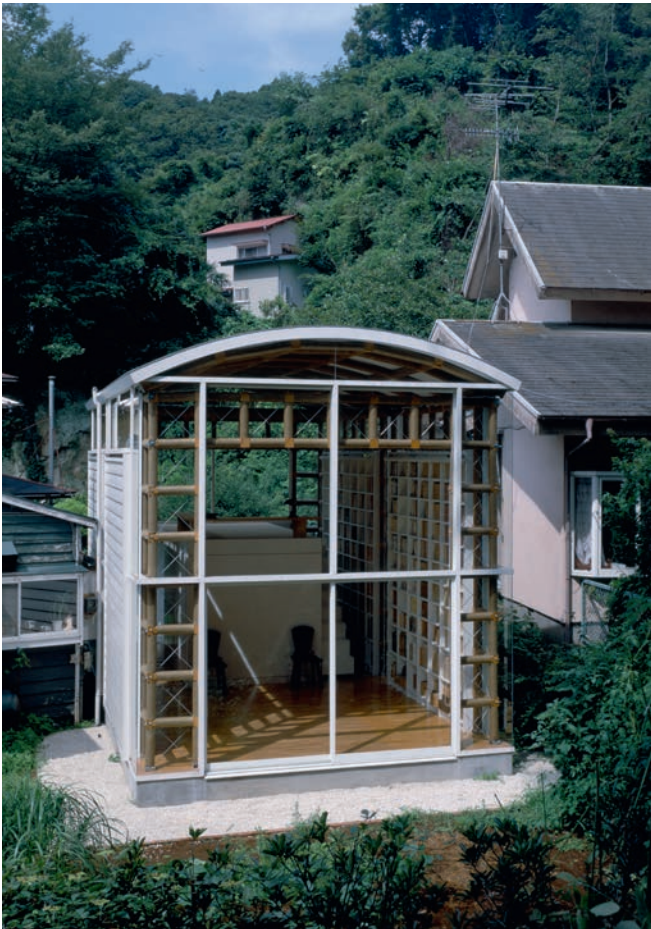
Illustration 6.25 Library of a Poet, Zushi, Kanagawa, Japan (1991). View of glass-enclosed library addition reveals overall frame structure composed of multiple short cardboard tube segments. Architect: Shigeru Ban Architects. Structural engineer: Gengo Matsui (Hoshino Architect and Engineer).
