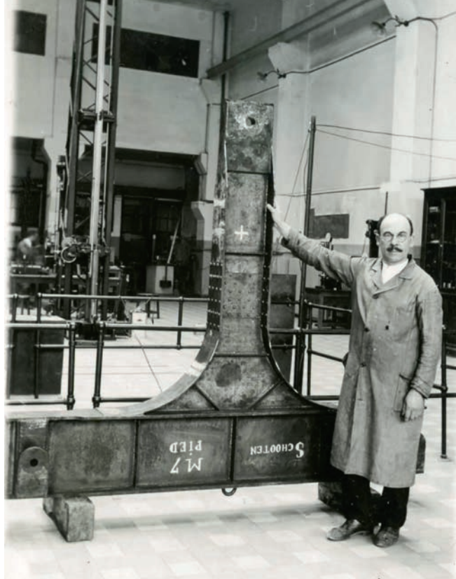
Illustration 10.65 A "classic" rigid joint connection between steel beam and column elements used for the Schooten Bridge, proudly displayed here by Belgian Professor Henri Dustin (1882–1935), Director of the Laboratory for Testing of Materials at the Université Libre de Bruxelles. (Photo taken in 1934.)
