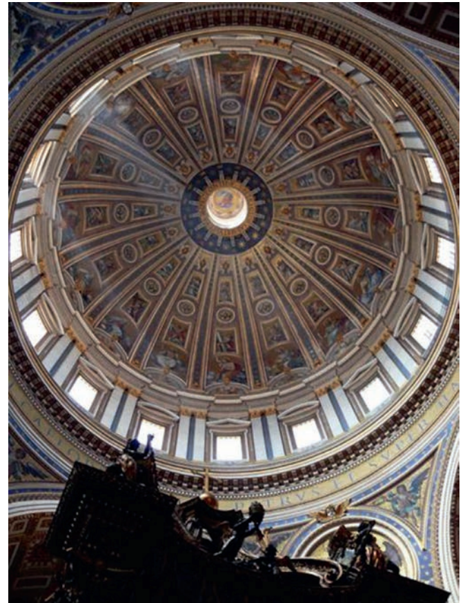
Illustration 13.14 St. Peter's Basilica, Vatican City (1590). Window openings around base of dome not only phenomenally “lift” it up into the air, but also may be a reflection of observations of radial cracking around base of such masonry structures. Architect: Michelangelo (with the involvement of others before and after).
