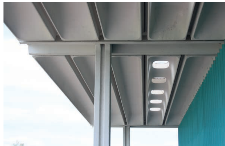
Illustration 7.20 UniFor Headquarters Building. For Mangiarotti's so-called U70 constructive system, long-spanning, precast concrete beams span side by side in one direction into precast concrete beams that are in turn carried on precast columns – all of which are configured and integrated with one another into a whole structural system of remarkable qualities.
