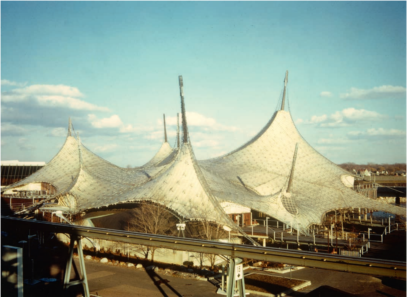
Illustration 11.29 German Pavilion, Expo '67, Montreal, Canada (1967). Multiple high points at tops of masts and low point anchorages enabled the unique double-curvature shape of the cable net surface that covered the full extent of the terraced landscape of the pavilion. Architect: Atelier Frei Otto and Rolf Gutbrod. Structural engineer: Leonhardt und Andrä.
