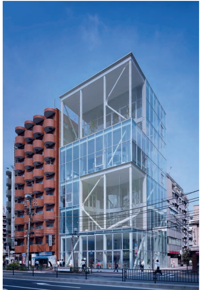
Illustration 2.11 Shibaura Office Building, Tokyo, Japan (2011). Exterior strongly expresses skeletal/line element structural system of columns, beams, and diagonal braces. Architect: Kazuyo Sejima & Associates. Structural engineer: Sasaki Structural Consultants.
