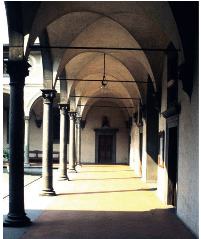
Illustration 12.37 Ospedale degli Innocenti arcade, Florence, Italy (1424). Into-the-courtyard thrust of arcade's transverse vaults countered by tension tie rods. Architect: Filippo Brunelleschi.
