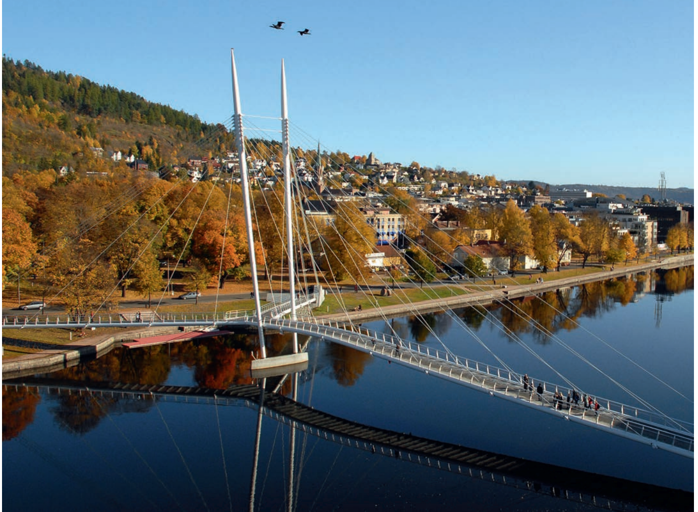
Ypsilon Footbridge, Drammen, Norway (2008). Asymmetrical cable-stayed system, including alternate pathways at north end. Architect: Arne Eggen. Structural engineer: Knut Gjerding-Smith.
