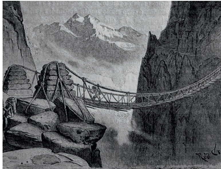
Illustration 11.7 Incan rope bridge, Andes Mountains (nineteenth century). Suspension cable profile is evident, and its "lively" nature can be sensed. Dead weight anchorage seen at left. Engraving by Rodolfo Cronau.
