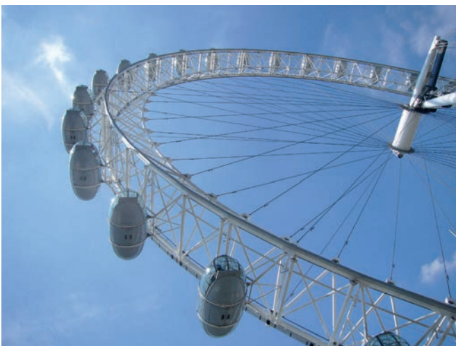
Illustration 6.6 Millennium Wheel, London, UK (2000). Tension rods provide only means of support for outer trussed ring. Architect: Marks Barfield Architects. Structural engineer: Jane Wernick, then at Arup.
