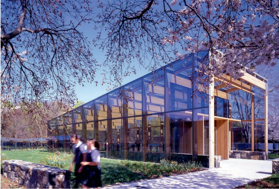
Illustration 10.3 Greenwich Academy Upper School. Glass pavilions project above the landscaped rooftop – at once creating access points from the upper level of the sloping site and drawing daylight deep into the two-story building, but also creating night-time light chambers for the work of artist James Turrell.
