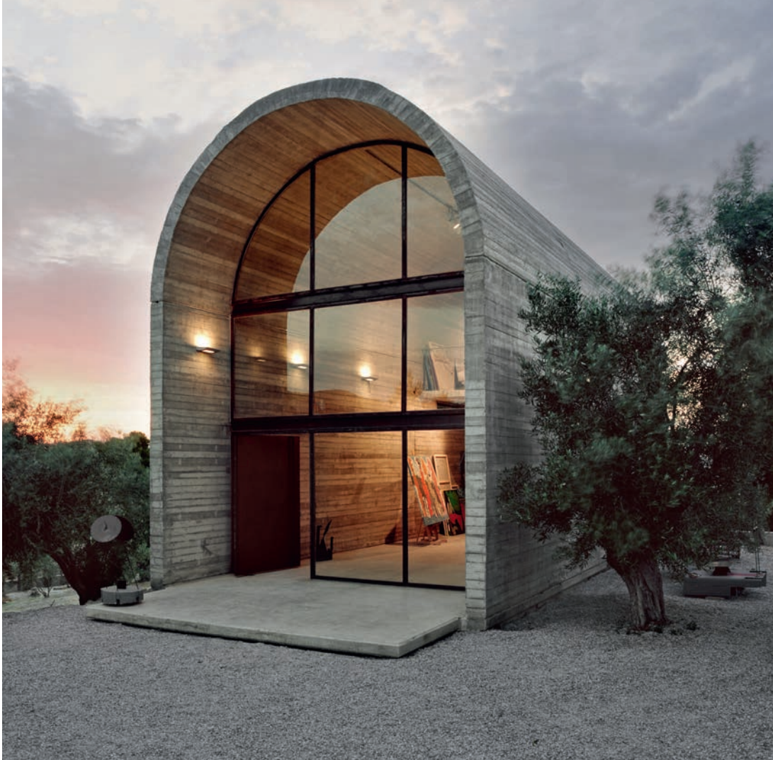
Illustration 12.41 Art Warehouse, Boeotia, Greece (2013). Smooth, continuous reinforced concrete arched form establishes most basic vaulted structure and space for this art studio/warehouse/gallery. Architect: A31 Architecture.
