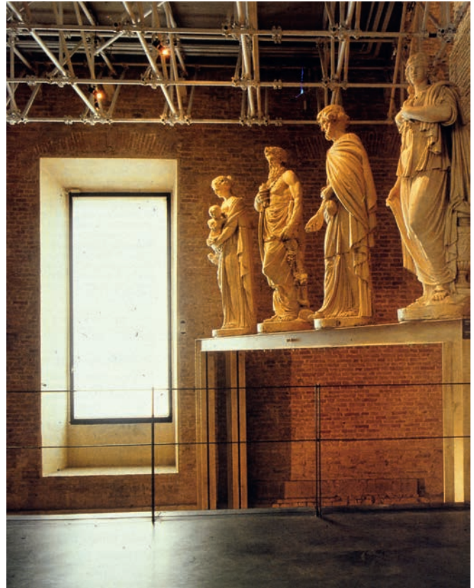
Illustration 7.9 Galleria Nazionale, Palazzo della Pilotta, Parma, Italy (1583; renovation: 1986). Steel beam supports classical sculptures as part of museum renovation. Architect (of renovation): Guido Canali.
