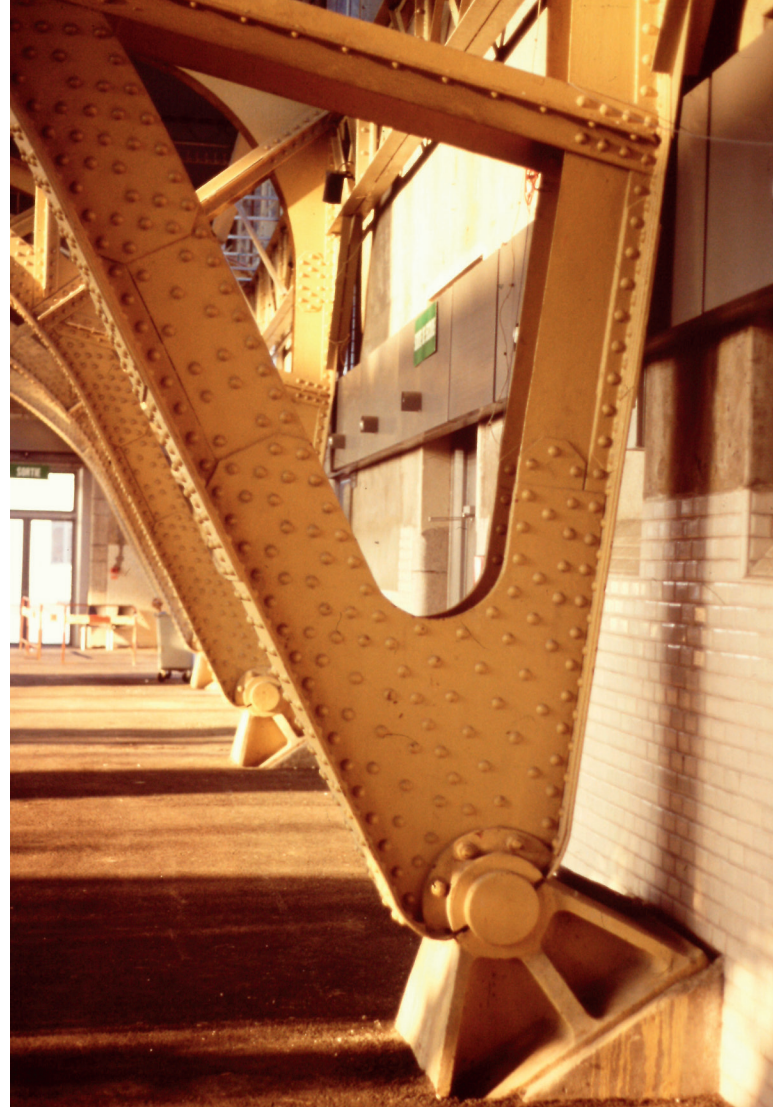
Illustration 12.23 Abattoirs de la Mouche, Lyon, France (1913). Hinge detail at base of arch that expresses ability of structure to rotate freely at that point; dimension of trussed arch rib tapers to minimum possible. Designer and structural engineer: Tony Garnier.
