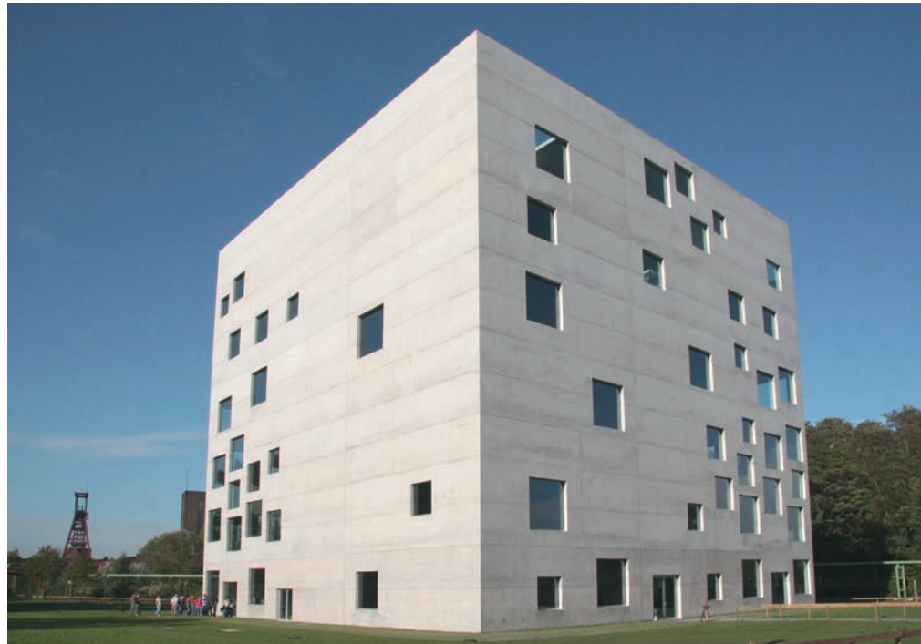
Illustration 8.31 Zollverein School of Management and Design, Essen, Germany (2006). Load-bearing concrete façade walls with openings. Architect: SANAA. Structural engineer: Bollinger + Grohmann.
