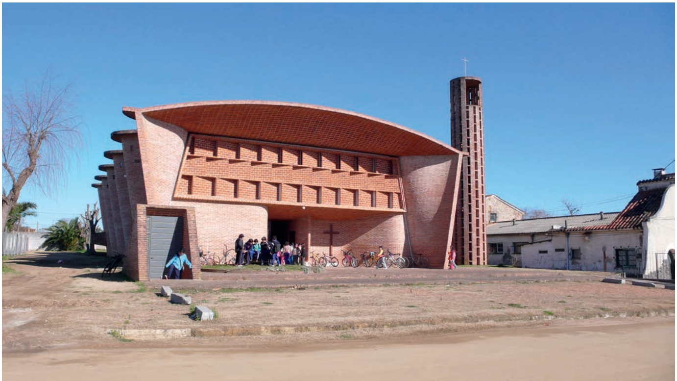
Illustration 13.41 Church of Christ the Worker, Atlántida, Uruguay (1960). The beginnings of Dieste's oeuvre of curving, long-span, thin shells made of clay bricks (post-tensioned together). Designer and structural engineer: Eladio Dieste.
