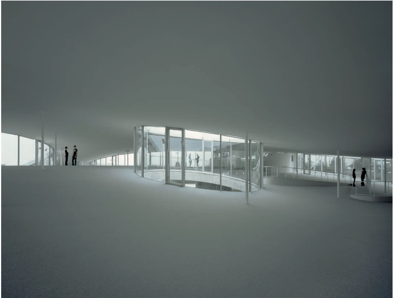
Illustration 13.51 Rolex Learning Centre. Thick concrete shell creates walkable surface "landscape."
