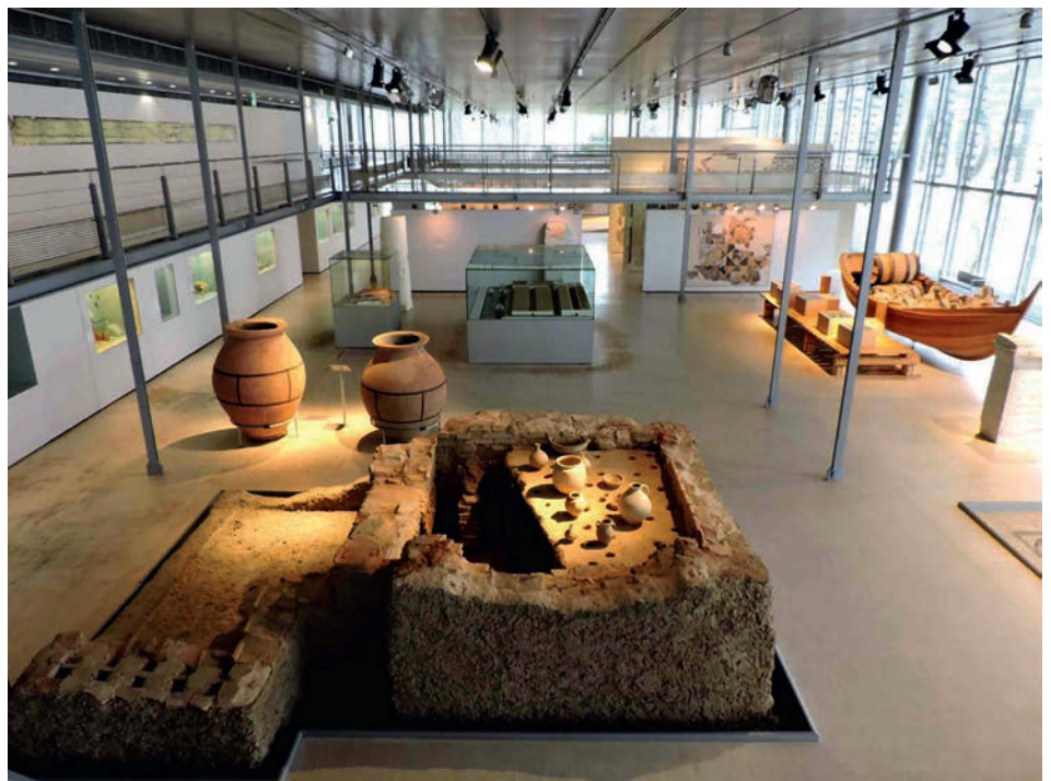
Illustration 6.14 Musée Gallo-Romain. Multiple vertical hangers are evident that support the museum floor area as well as its mezzanine walkways. Loads are carried up the underside of the transverse roof beams, hidden in this view above the hung ceiling.
