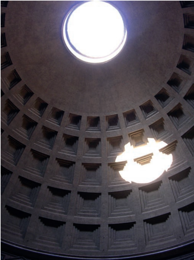
Illustration 13.19 Pantheon, Rome, Italy (AD 126). Open oculus at dome apex connects interior to the heavens/ natural elements while also serving essential structural function at the point of major stress concentration. Architect: Apollodorus of Damascus.
