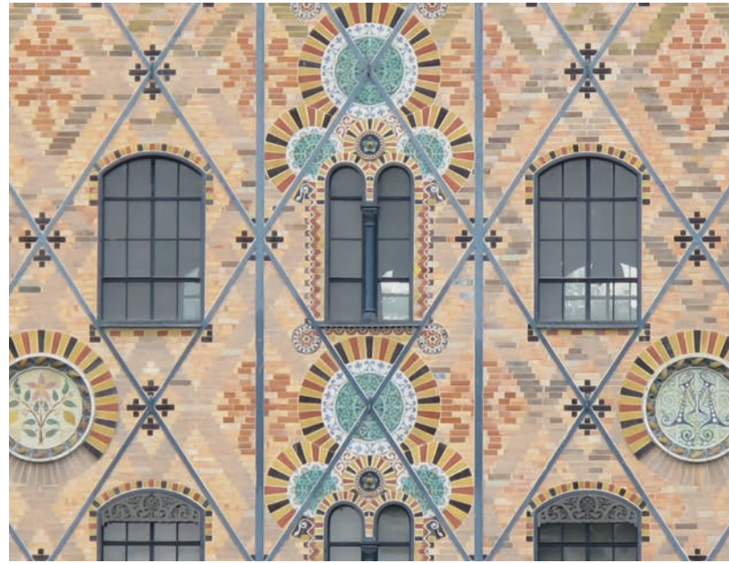
Illustration 10.28 Chocolaterie Menier. Detail of windows and medallion of tiles depicting the cocoa plant as well as highlighting the many intersection points of the diagrid bracing.
