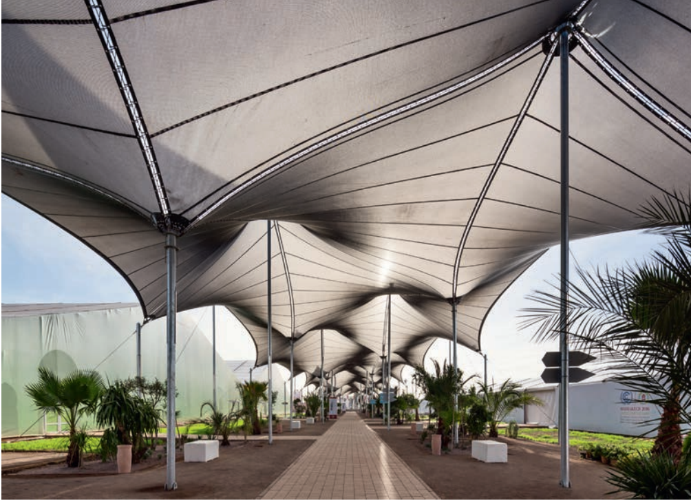
Illustration 11.42 COP 22 Village, Marrakesh, Morocco (2016). Shading fabric canopy exhibits strong membrane curvatures everywhere, giving the surface stability against excessive deformations. Architect: Oulalou + Choi Architectures.
