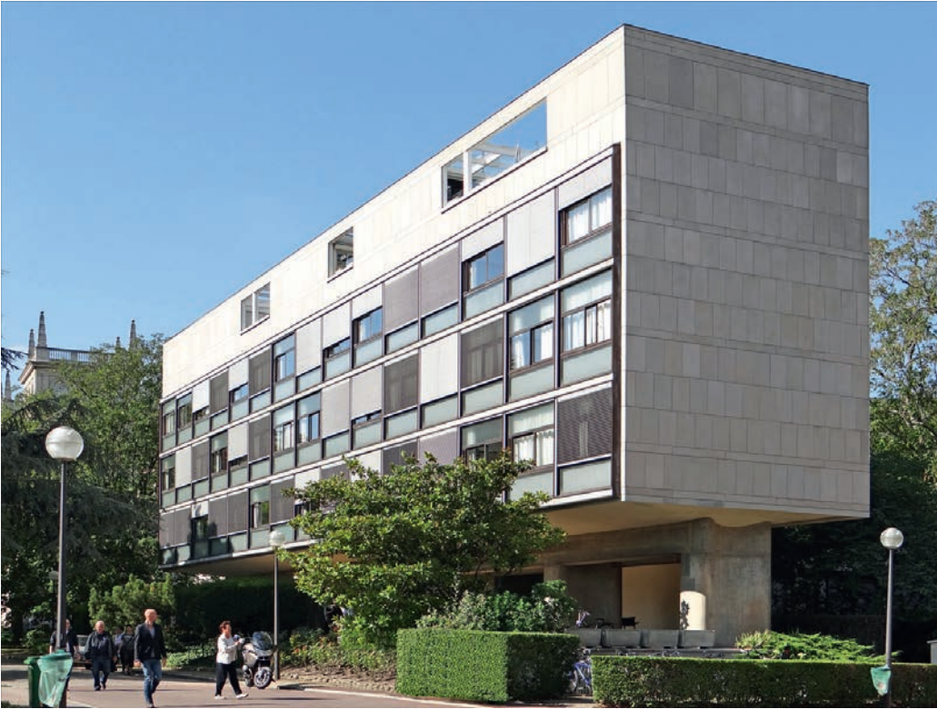
Illustration 2.2 Pavilion Suisse, Paris (1932). Exterior view of south façade of dormitory block. Architect: Le Corbusier.
