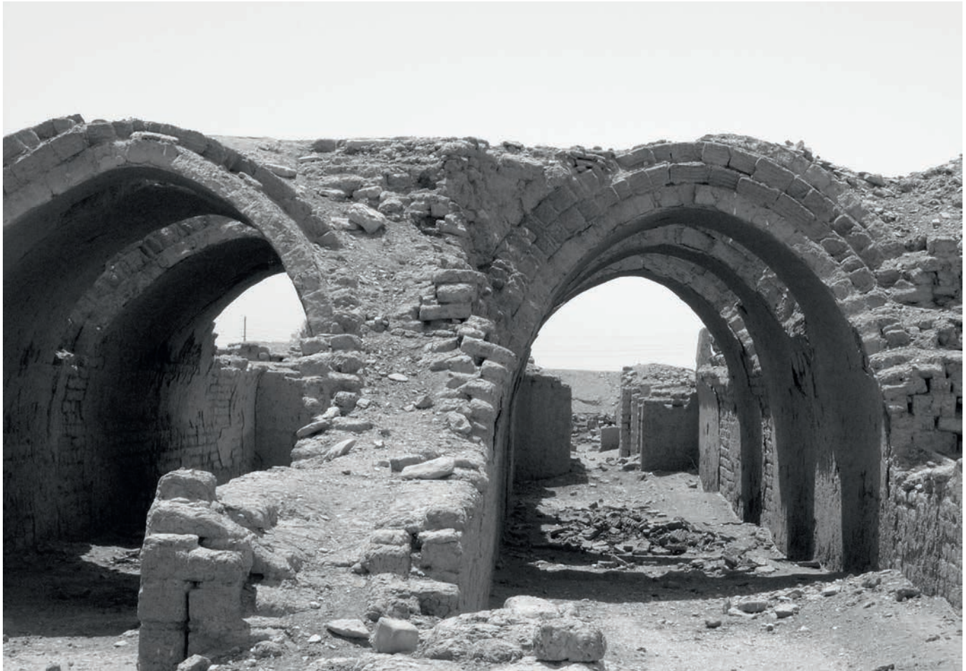
Illustration 12.5 Granaries of Ramesseum, Luxor, Egypt (approximately 1400 bc). Rubble fill above sides of clay brick vaults helps stabilize form; presages the favored Roman technique.
