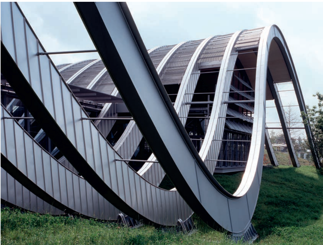
Illustration 12.22 Zentrum Paul Klee, Bern, Switzerland (2005). (top) Multiple, continuous, undulating arch ribs are subject to much bending; (bottom) each arch rib is in cross-section a deep steel plate box-girder, a form well suited to this purpose. Architect: Renzo Piano Building Workshop. Structural engineer: Arup.
