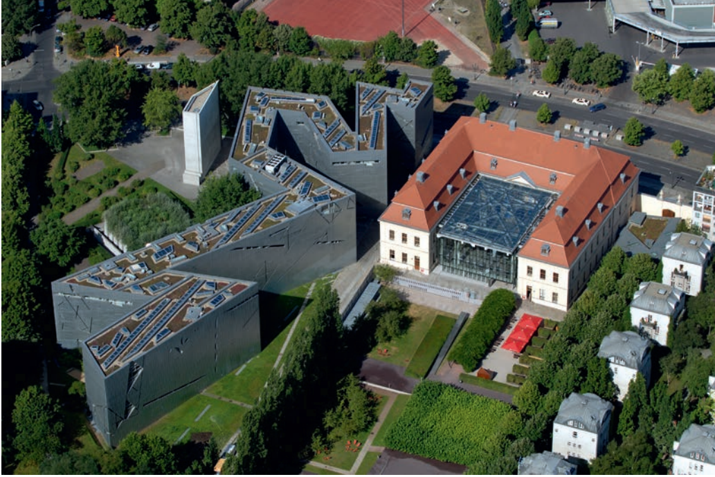
Illustration 7.4 Glass Courtyard, Jewish Museum, Berlin, Germany (2007). Aerial view shows relationship of glass courtyard to enveloping U-shaped Baroque Kammergericht, to sharply angled plan of Libeskind's museum building, and to gardens. Architect: Daniel Libeskind. Structural engineer: GSE Ingenieur-Gesellschaft mbH.
