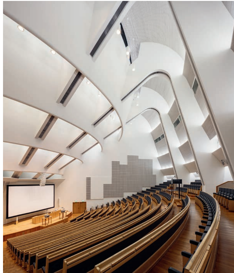
Illustration 10.60 Otaniemi Technical University, Otaniemi, Finland (1966). Series of concrete rigid frames of non-conventional form envelops the space of the auditorium. Architect: Alvar Aalto. Structural engineer: Magnus Malmberg.
