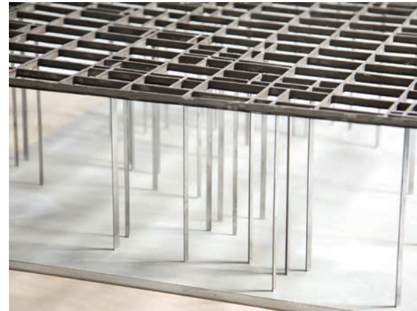
Illustration 2.10 White Forest Pavilion, KAIT, Atsugi, Japan (2007). Non-uniform interior spaces of a student workshop are created by having a large number (305) of irregularly placed, randomly oriented, small planar columns that suggest room zones and act as visual screens of variable densities aside from carrying loads. Architect: Junya Ishigami + Associates. Structural engineer: Yasutaka Konishi. Cornell model by Jordan Berta and Henry Gao.
