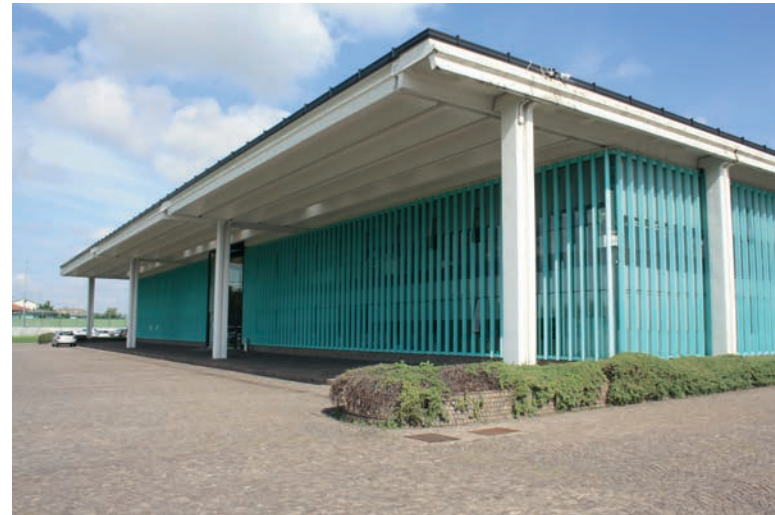
Illustration 7.19 UniFor Headquarters Building, Turate, Italy (1982). Long span roof beams are prone to significant deflection, but pre-stressing of concrete greatly reduces the problem. Compare the beam span-to-depth proportions here to those of historical stones seen in Section 7.2. Architect: Studio Mangiarotti. Structural engineer: Vintani Alberto.
