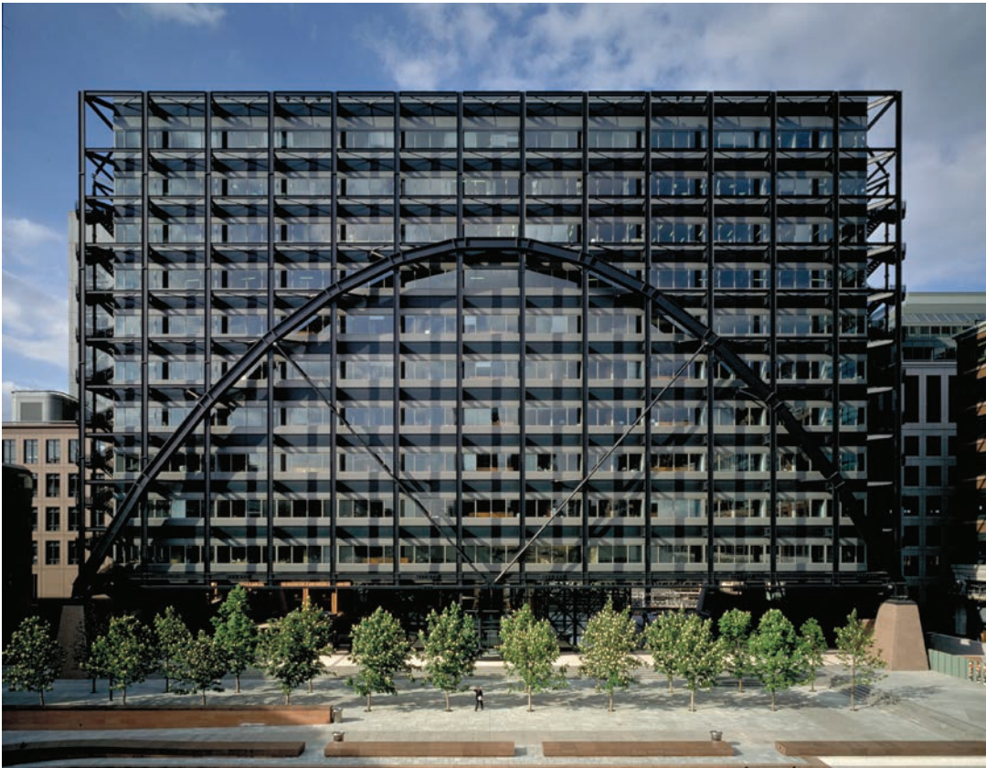
Illustration 12.32 Broadgate Exchange House, London, UK (1990). Relatively thin arches support multistory building; arch profile is stabilized by diagonal members. Outward thrusts at base supports negated through horizontal tension tie. (See Ill. 6.29.) Architect: Skidmore, Owings & Merrill (SOM). Structural engineer: SOM.
