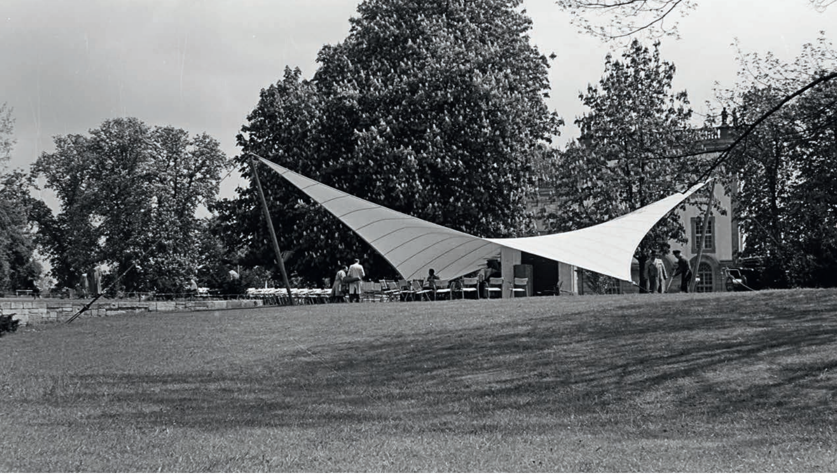
Illustration 11.45 Kassel Music Pavilion. Photo of fabric membrane pavilion.
