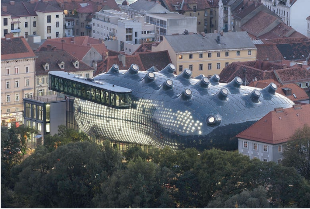
Illustration 5.48 Kunsthaus Graz, Graz, Austria (2003). Unusual form and coloration of art gallery building with acrylic glass roof contrasts with surrounding historical urban context. Architect: Spacelab Cook-Fournier; Architektur Consult. Structural engineer: Bollinger + Grohmann.
