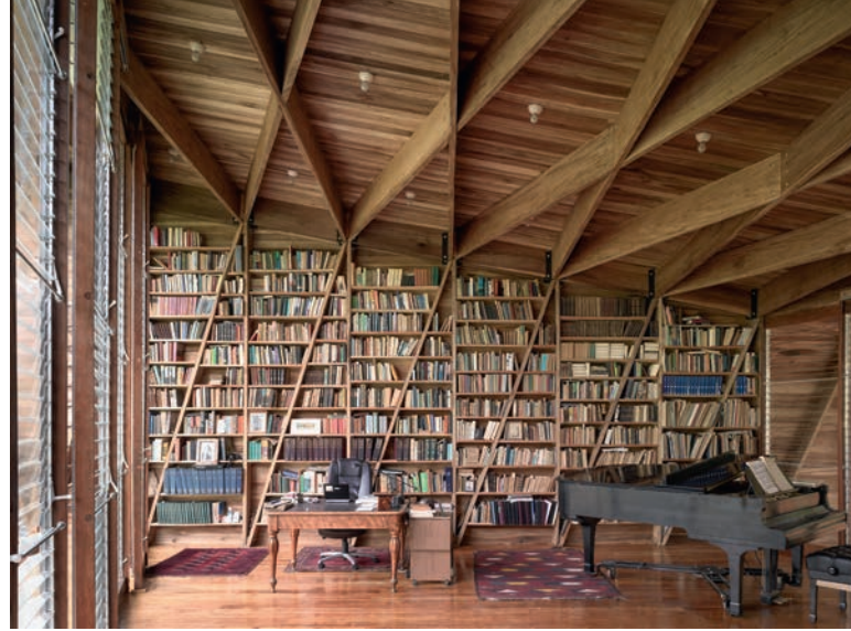
Illustration 10.21 Casa Kiké, Cahuita, Costa Rica (2007). Expressive single diagonal wood bracing members stabilize rectangular frame panels along sides of this writer’s house/pavilion. Diagonals are integrated into bookshelves, and visual pattern is extended into diagonal bracing beams for the roof. Architect: Gianni Botsford Architects. Structural engineer: Tall Engineers.
