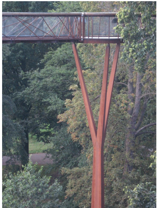
Illustration 9.21 Xstrata Treetop Walkway, Kew Gardens, London, UK (2008). This walkway runs 200m (656ft) among the trees at Kew and is raised 18m (59ft) above the ground, enabling a unique vista of the garden from the treetops. A continuous truss bridge supported on pylons, the structure features a variation of the density of the structural members: as the trusses approach the supports, the density of diagonal members increases in response to the increase of shear forces. The spacing of the diagonals is dictated by the so-called Fibonacci sequence, a mathematical relationship between numbers in a series often associated with nature's forms. 6 This principle is used both for the vertical trusses which form the balustrade, and the walkway deck structure which forms horizontal trusses resisting wind. Architect: Marks Barfield Architects. Structural engineer: Jane Wernick Associates.
