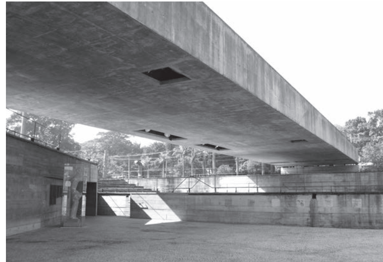
Illustration 7.25 Brazilian Museum of Sculpture, São Paulo, Brazil (1988). Deep, wide concrete beam spans across, unifies, and shelters exterior exhibition space. Multilevel “ground” actually roofs over sunken museum interior spaces. This beam is in fact of hollow cross-section – see Ill. 7.26. Architect Paulo Mendes da Rocha. Structural engineer: Escritório Técnico Júlio Kassy and Mário Franco Engenheiros.
