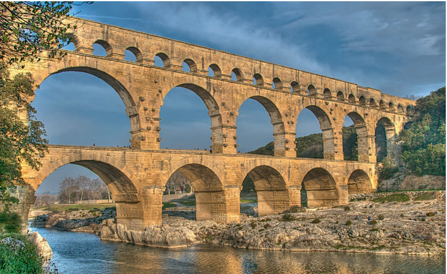
Illustration 12.8 Pont du Gard, near Nîmes, France (first century). Multi-layered series of stone arches sitting atop of one another combined to help supply Roman cities with water; lead-plate-lined channel ran along the top for this purpose.
