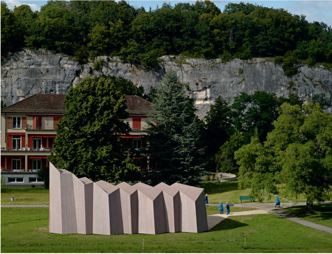
Illustration 13.24 Temporary St-Loup Chapel, Deaconess Community of St-Loup, Pompaples VD, Switzerland (2008). Built for short-term use during the renovation of this religious community's main buildings, a small trapezoidal folded plate structure was constructed from many cross-laminated timber panels, 40mm (1.5in) thick for the walls and 60mm (2.25in) for the roof. Architect: localarchitecture and Danilo Mondada Architects. Structural engineer: IBOIS – Hani Buri / Yves Weinand.
