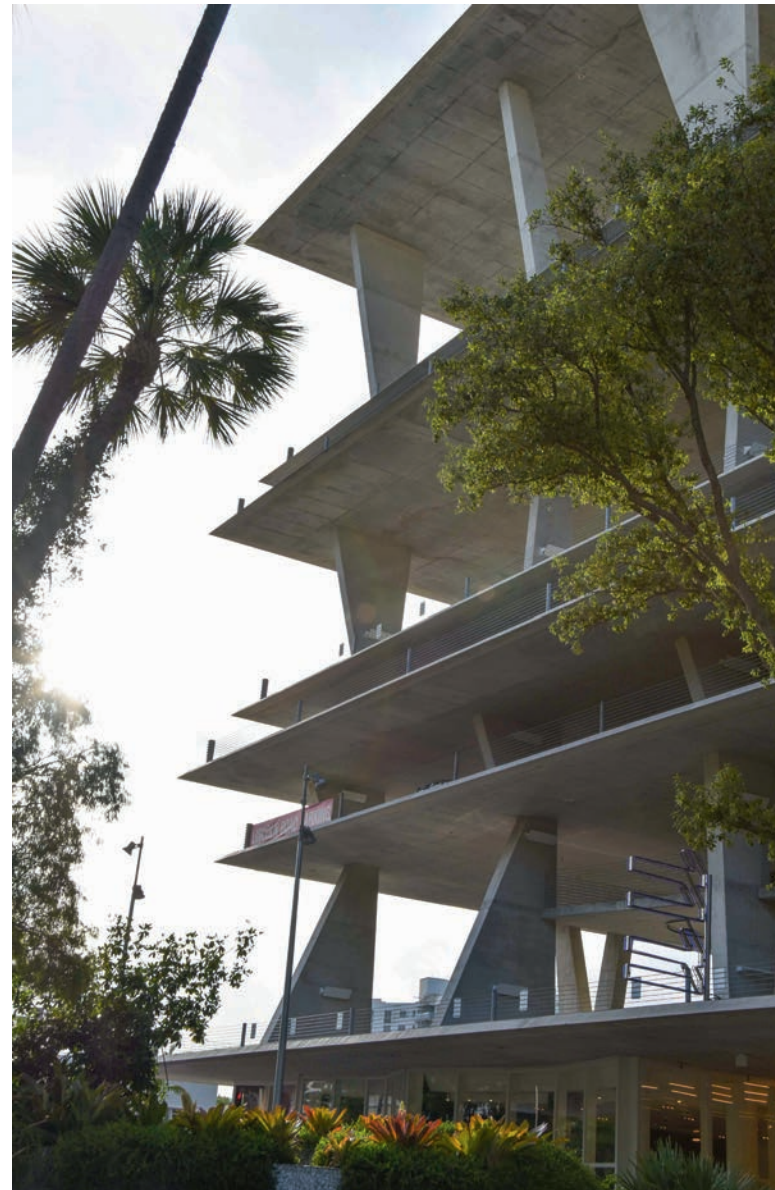
Illustration 7.55 1111 Lincoln Road, Miami Beach, FL, USA (2010). Flat plate slabs define varying floor level heights and vertically subdivide the large open structure. Architect: Herzog & de Meuron. Structural engineer: Optimus Structural Design.
