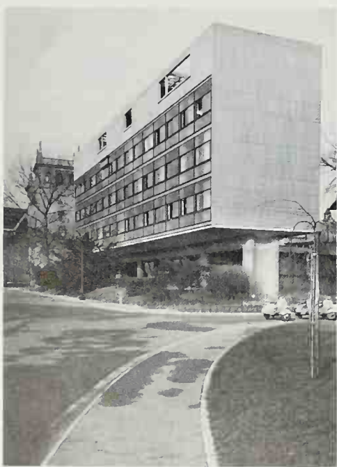
SWISS PAVILION, UNIVERSITY CITY. Le Corbusier. Paris. 1932. Elevated on sculptured concrete piers, this cantilevered residence hall for some fifty students was Le Corbusier's first major public building.
