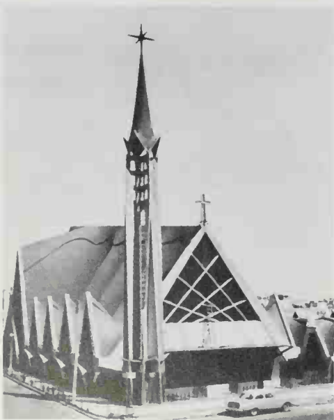
CHURCH OF THE MIRACULOUS VIRGIN. Félix Candela with Enrique de la Mora. Mexico City. 1953. The thin shell vaults of the church dramatically display Candela's superb skill with reinforced concrete.
