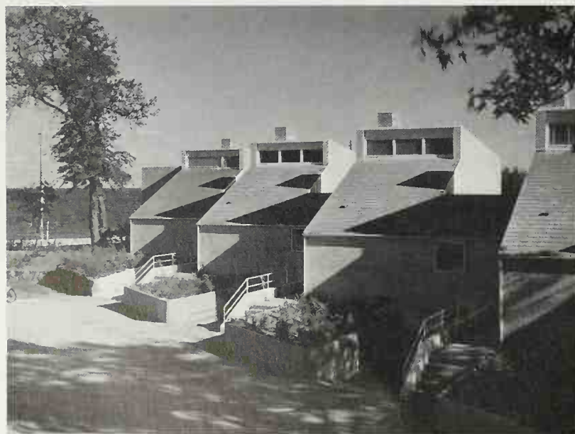
ROW HOUSES. Arne Jacobsen. Søholm, Denmark. 1950. The textured natural materials and the imaginative play of the roofs of these row houses represent a picturesque departure from Jacobsen's sleek International Style.
