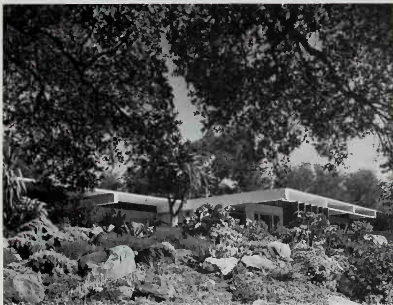
TREMAINE HOUSE. Richard Neutra. Los Angeles, California. 1929. This early modern house was a breakthrough residential use of prefabricated light steel frames, reinforced-concrete walls, and wide glass windows.
