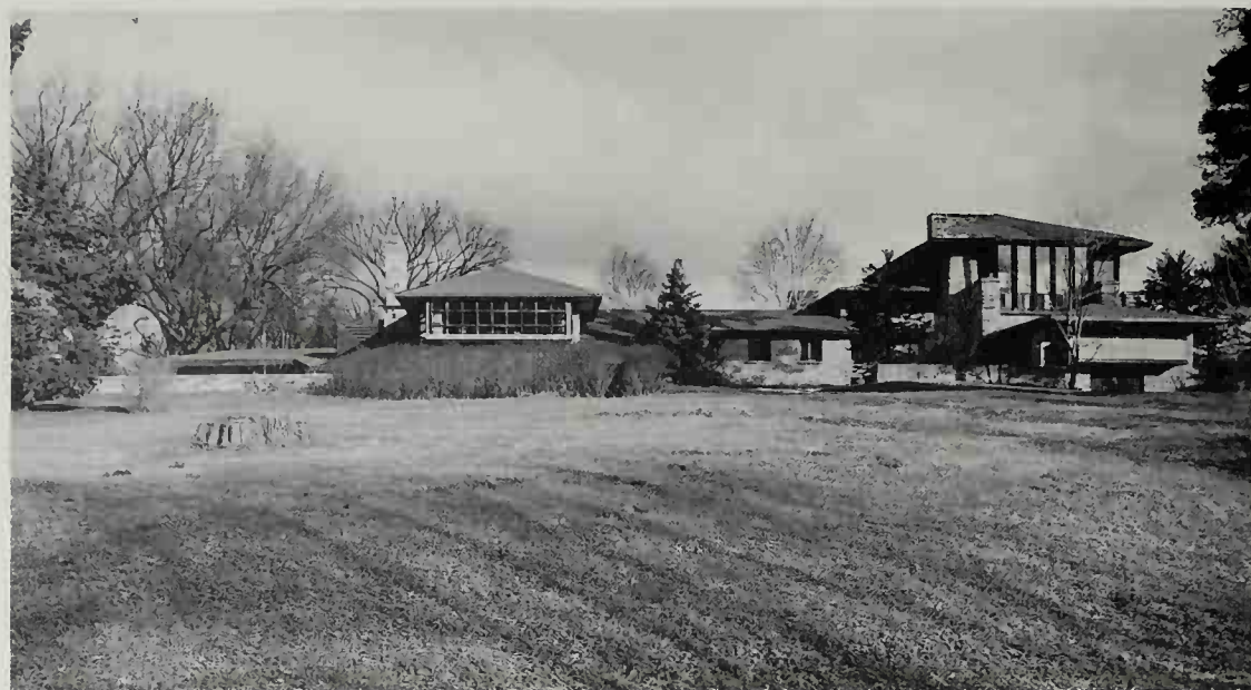
HILLSIDE HOME SCHOOL. Frank Lloyd Wright. Spring Green, Wisconsin. 1902. Wright departed from traditional educational-building styles in designing this pioneering coeducational boarding school for his aunts, Jane and Nell Lloyd Jones.
