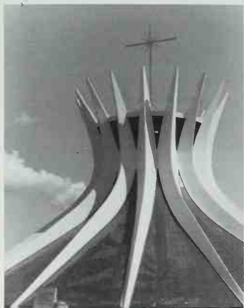
BRASÍLIA CATHEDRAL. Oscar Niemeyer. Brasília, Brazil. 1959. Arrayed in a circular plan, twenty-one converging curved buttresses open at the top in a halo-like ring to admit a strikingly spiritual cone of light.
