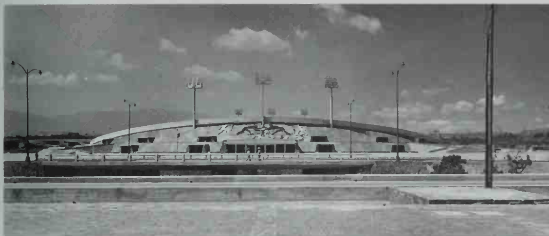
OLYMPIC STADIUM. Augusto Perez Palacios with Raúl Salinas Moro and Jorge Bravo Jimenez. Mexico City. 1951. Dug into the ground with curved concrete retaining walls and finished with lava facings, this modern sports stadium recalls the splendor of Aztec construction.
