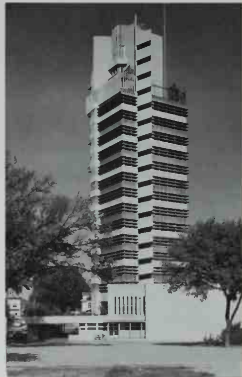
H.C. PRICE TOWER. Frank Lloyd Wright. Bartlesville, Oklahoma. 1952. The spectacular nineteen-story office and residential tower with a "tap-root" foundation is Wright's only built skyscraper.
