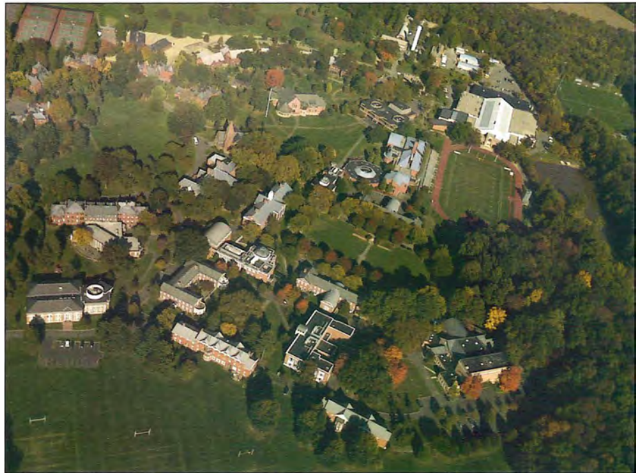
Figure 17.3 Lawrenceville School, Lawrenceville, New Jersey. View of campus showing rural, Anglicized landscape elements, original design features (the Circle) from Frederick Law Olmstead (upper left), and recent additions (upper right).
