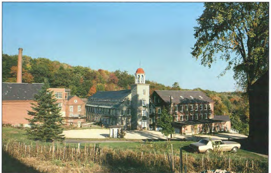
Figure 13.7 Cheshire woolen mills in Harrisville, New Hampshire, at the center of the purest surviving New England mill village from the mid-19th century. The granite Mill No. 1 (1846–1848, center) and the brick Mill No. 2 (1856, right) draw water from the millpond (behind building at left), and produced textiles until 1970.
