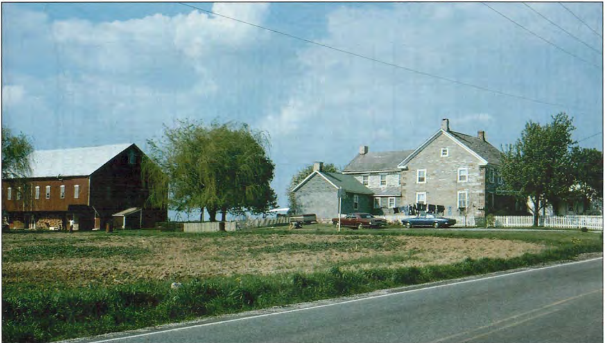
Figure 5.10 Pennsylvania barn, with its distinctive cantilevered "forebay," in central Pennsylvania, in 1979. The ground level is for stabling livestock; the second level, entered at grade via an inclined "bank" on the uphill side, contains a threshing floor; and the upper lofts are for storing hay. Barns like these are the single most diagnostic feature of Pennsylvania German rural culture.
