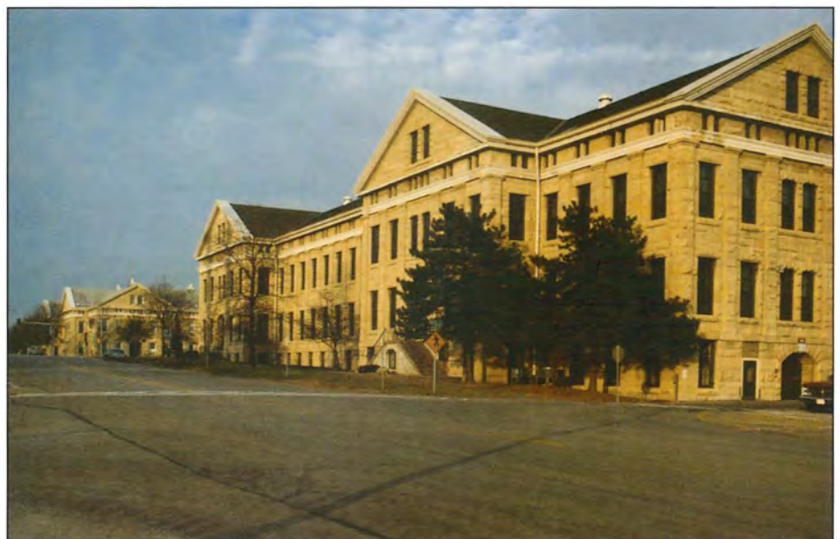
Figure 15.6 The core manufacturing buildings of the Rock Island Arsenal, Illinois. Built during the 1870s and 1880s of Joliet limestone shipped via the I&M Canal, these structures are in use to this day, although the production is restricted to replacement parts for light armaments.
