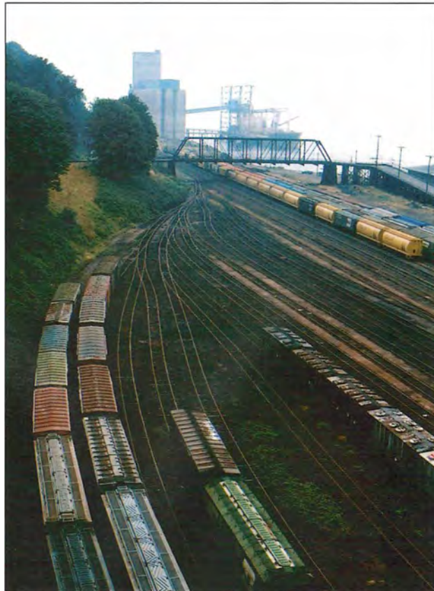
Figure 13.11 A rail yard of the Northern Pacific in Tacoma, Washington, hard against the bluffs that rim the southern edge of Puget Sound. Lumber, grain, and minerals pass through this transshipment point. In the background is an elevator with ship-loading equipment.
