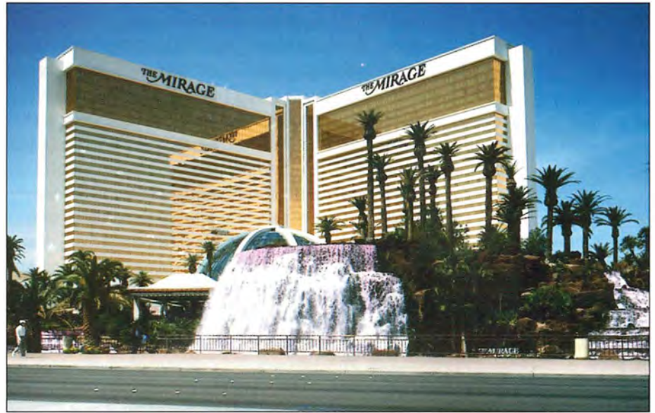
Figure 10.12 Fountains at the Mirage Hotel, Las Vegas, Nevada.
