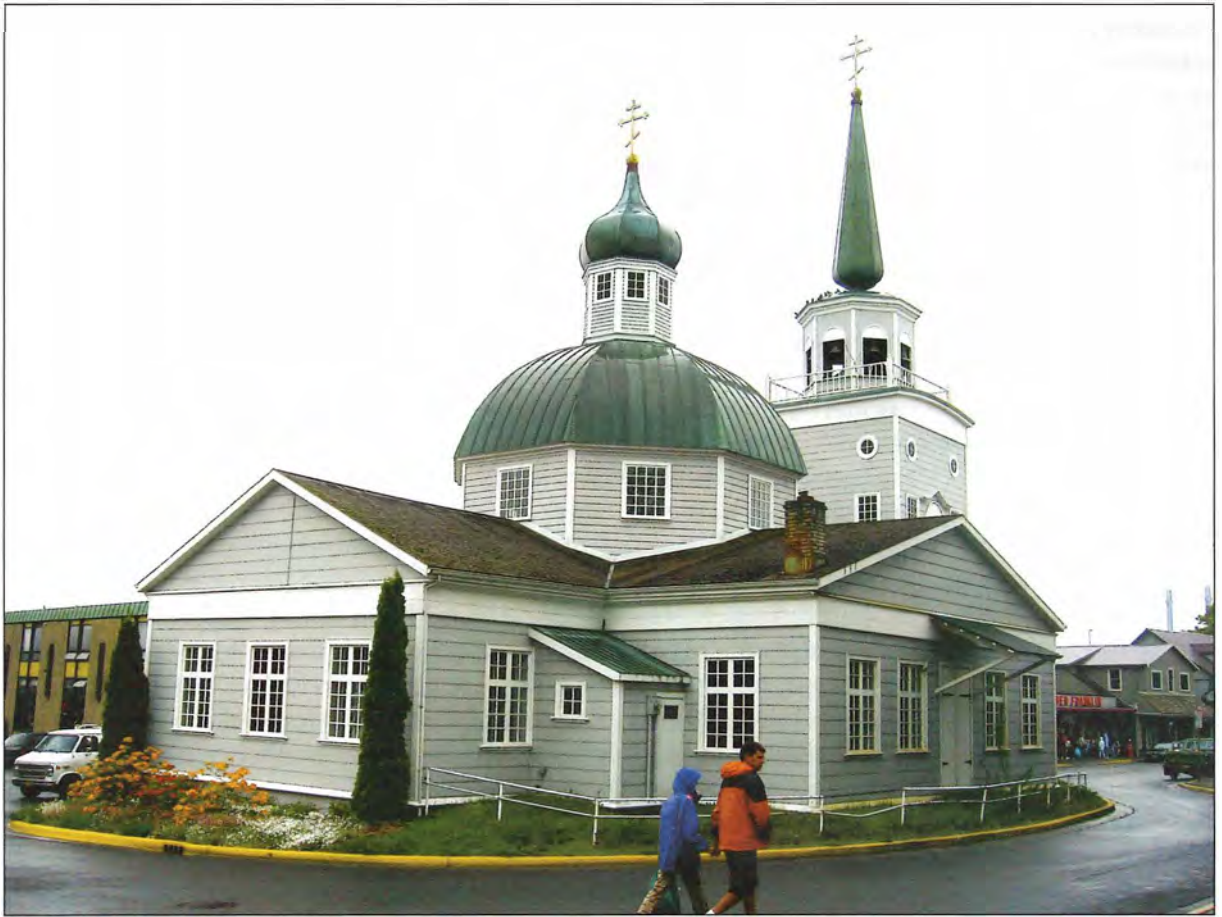
Figure 11.7 St. Michael's Russian Orthodox Cathedral at the center of Sitka, Alaska. The original log cathedral was built in 1848 and burned in 1966. The present structure, of concrete, replicates the original in every design detail.
