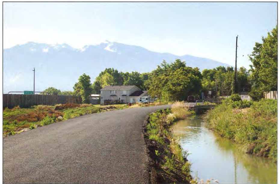
Figure 10.10 The South Jordan Canal, the second-oldest Mormon irrigation ditch in the Jordan Valley, completed in 1876, seen here in Taylorsville, Utah, in the southwestern suburbs of Salt Lake City, with the Wasatch Range in the background.
