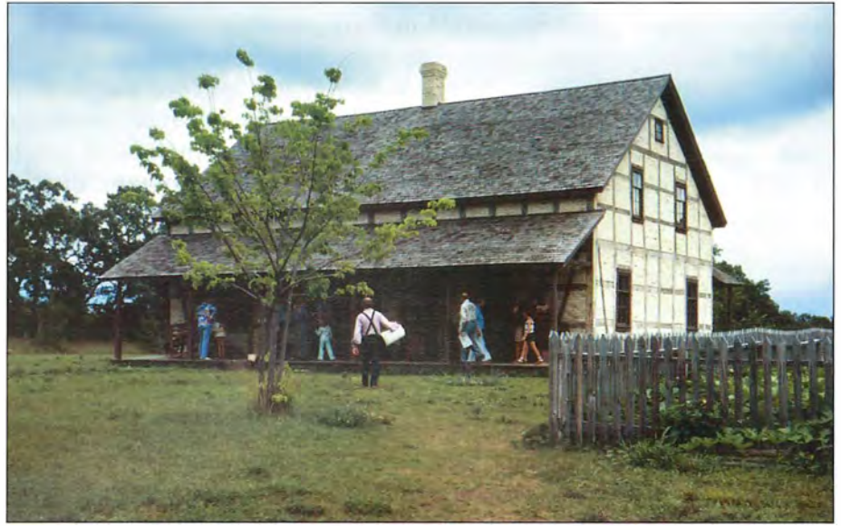
Figure 11.9 German half-timber construction in the Friedrich Koepsel Farmhouse, Lebanon, Dodge County, Wisconsin, built circa 1858. The building was moved to Old World Wisconsin and restored in 1979–1980.
