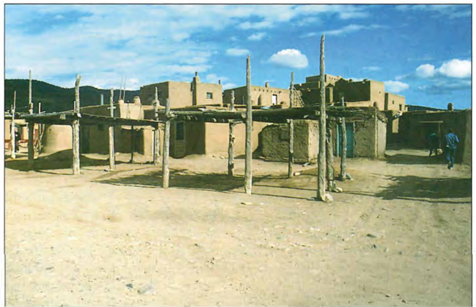
Figure 2.11 The multistoried, flat-roofed and adobe-faced masonry houses of Taos, New Mexico, are representative of surviving pueblos in the Southwest.
