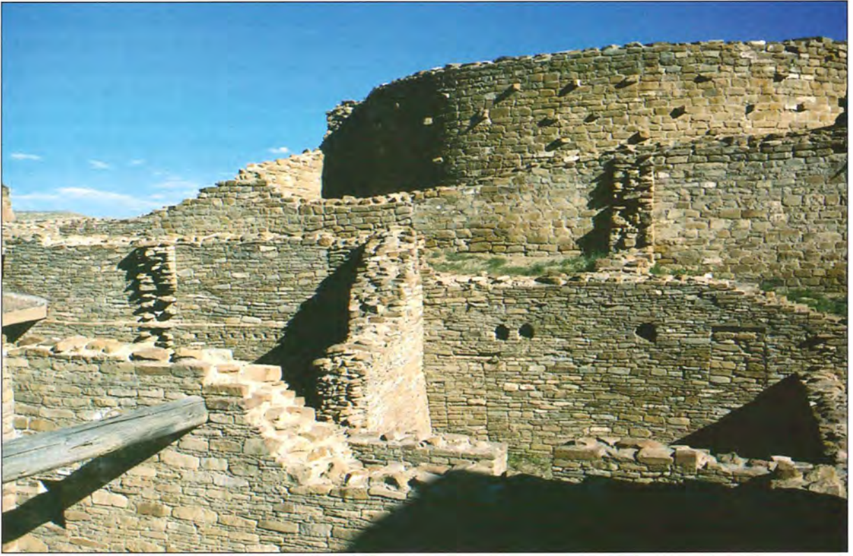
Figure 2.6 Masonry construction and pine crossbeams, Chetro Ketl, Chaco Canyon, New Mexico. Begun in AD 945, the complex gained additions as late as 1116, but was abandoned by 1120.
