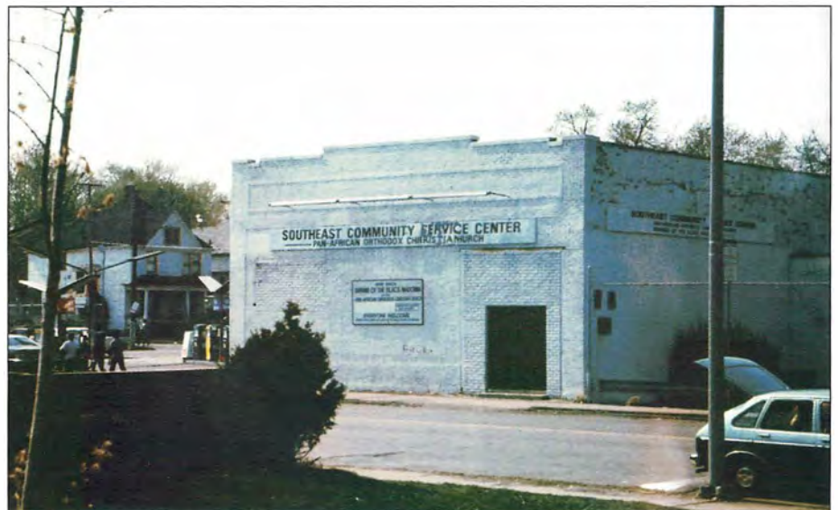
Figure 16.5 Southeast Community Service Center, Detroit, serves multiple community functions.
