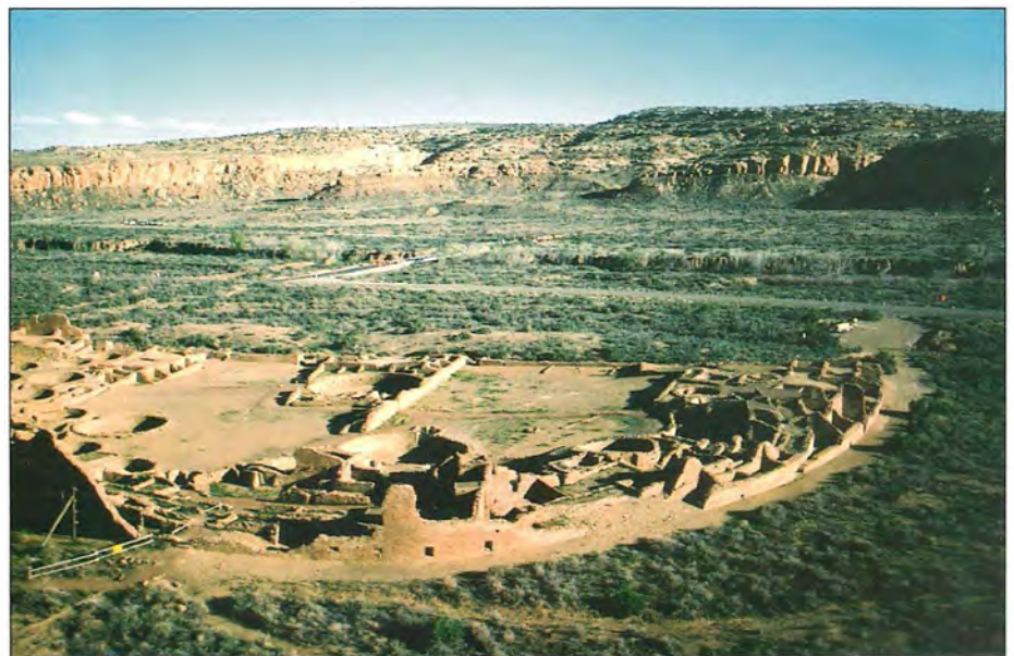
Figure 2.5 The masonry structures of the Pueblo Bonito ceremonial and population center, Chaco Canyon, New Mexico, illustrate the durability of 11th- and 12th-century settlements. The arroyo in the background was incised after AD 1100 but before abandonment, probably impeding floodplain cultivation.
