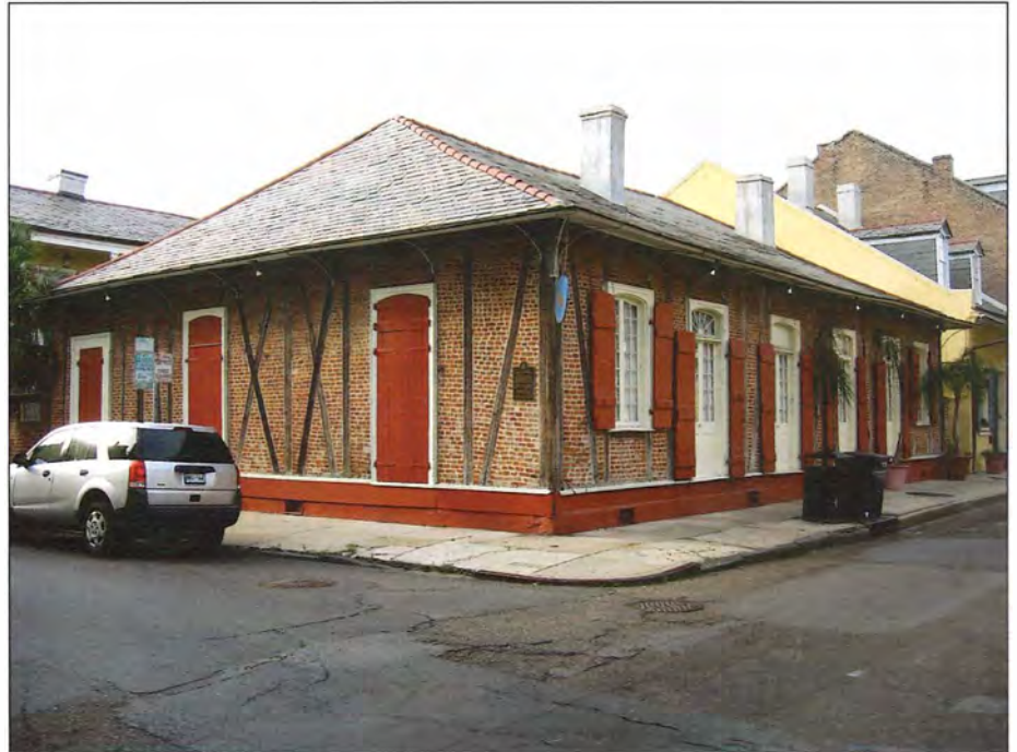
Figure 4.6 The Gabriel Peyroux House on Burgundy Street in the Vieux Carré district, New Orleans. While it was originally built on a plantation, Peyroux had it dismantled, moved, and erected here in 1780. The many French doors promoted air circulation in the languid summer heat.
