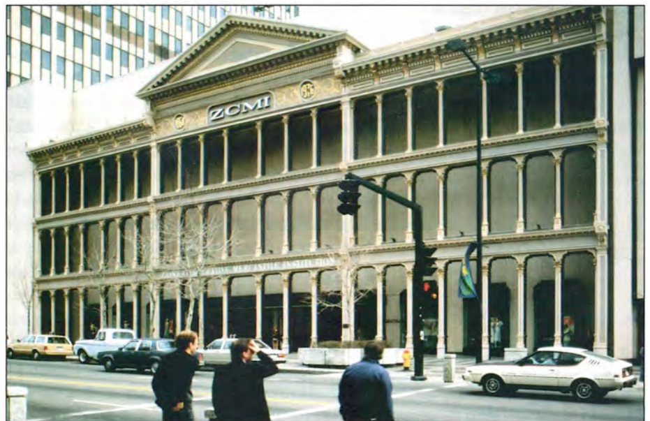
Figure 19.1 The first incorporated department store in America is memorialized here in the disemboweled reassembly of the 1876–1880 brick-and-cast-iron front of the former Zion Cooperative Mercantile Institution (ZCMI) store in Salt Lake City, stemming from its 1973 conversion to a shopping mall, seen here in 1988. Such insensitive façadism no longer passes muster with historic preservationists, and a further redevelopment of the property is planned that may substantially restore the storefront’s historic appearance.
