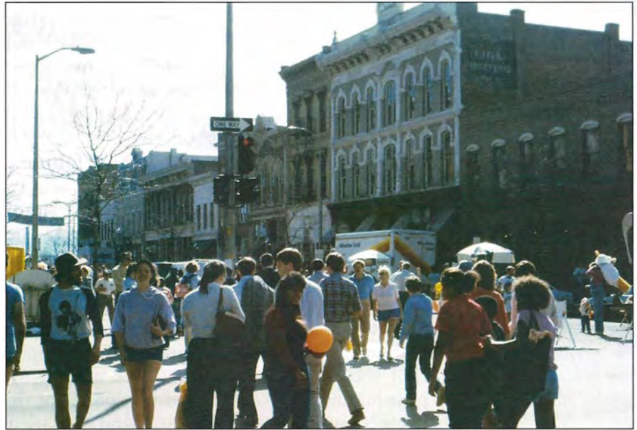
Figure 16.17 Italianate-style and other late 19th-century commercial buildings on Larimer Square in Denver contribute to the urban vibrancy that historic preservation can often support in large metropolitan centers.
