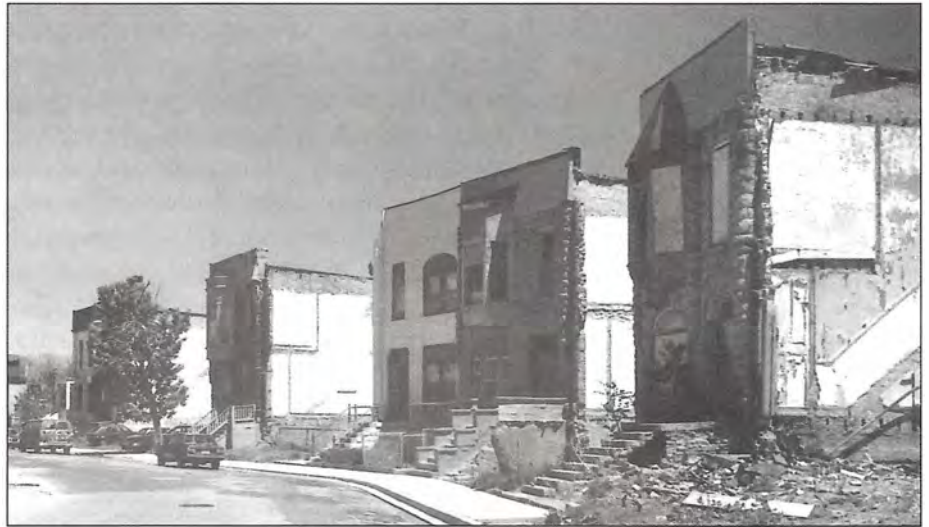
Figure 14.12 Surviving buildings on East 46th Street in Chicago, 1988. This gapped cityscape hints at the process of past neighborhood disinvestment, as torchings, and demolitions for health and safety reasons, depleted the housing stock of the worst affected districts.
