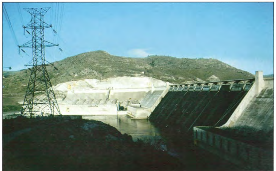
Figure 15.13 The Grand Coulee Dam on the Columbia River, Washington State, completed in 1941, is the largest concrete structure in the United States. A hydroelectric facility, its initial power generation fed the northwest wartime aluminum industry. In the longer view it has served as the centerpiece of the Columbia Basin Project, and irrigates over 500,000 acres of farmland.
