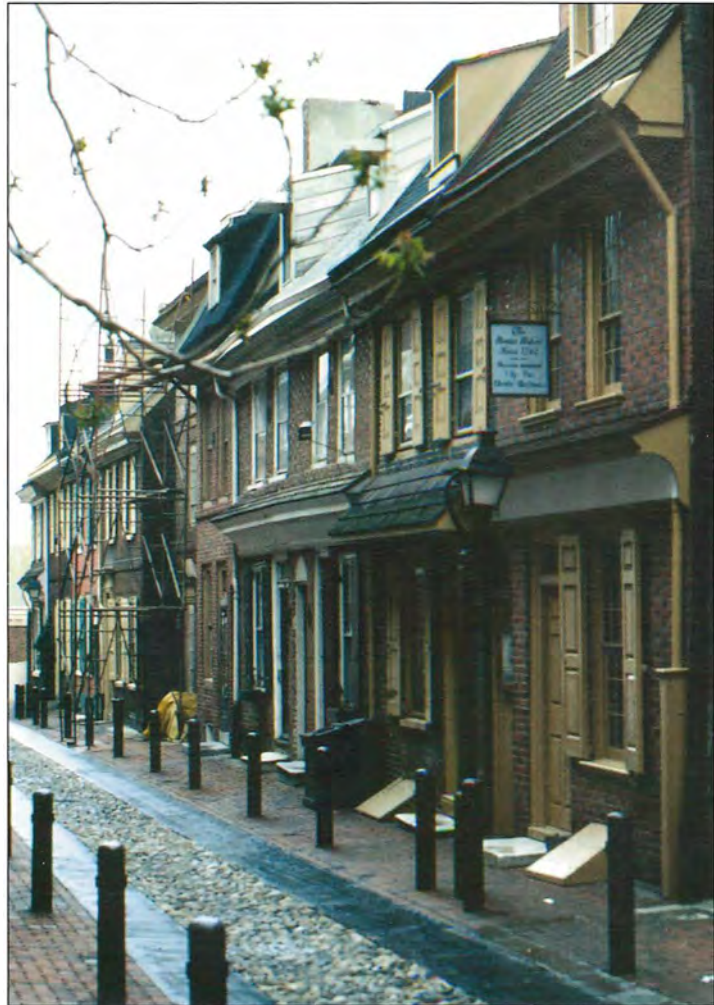
Figure 5.7 Elfreth's Alley, Philadelphia, a well-preserved remnant of 18th-century Philadelphia, is a standard bit of British urban morphology. Such brick row-houses continued to be built in Pennsylvania cities and villages until the mid-19th century, long after New Englanders had abandoned the idea.
