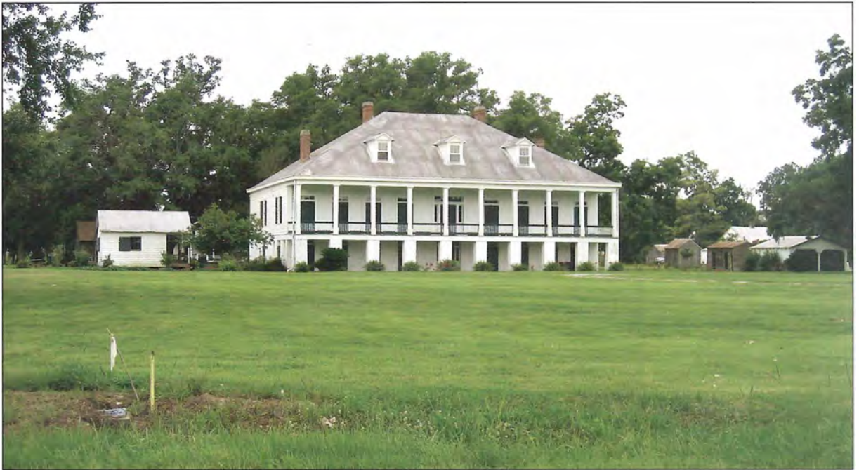
Figure 4.8 St. Joseph Plantation, built in the 1830s to raise sugar cane, is the largest of the French Creole plantation houses on the Mississippi River above New Orleans. Characteristic features include the elevated premier étage (primary living space), double gallery, and the hipped umbrella roof.
