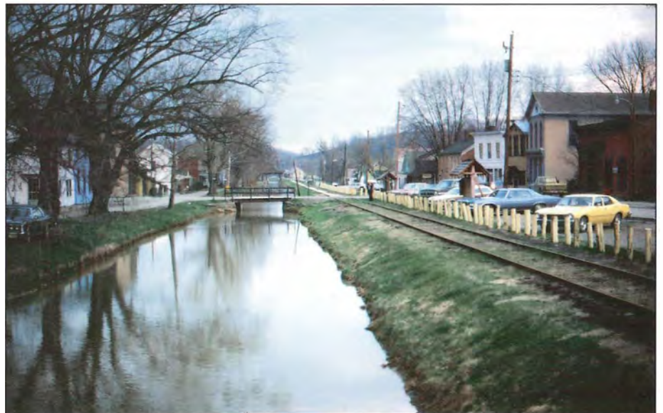
Figure 13.5 The Whitewater Canal was dug in the late 1830s to promote Cincinnati's northwestern hinterland trade and paralleled the river of the same name between Cambridge City, Indiana, and the Ohio River. Seen here passing through the small town of Metamora, it was bought by a railroad company in the 1860s, which promptly ran its tracks unceremoniously down the towpath.
