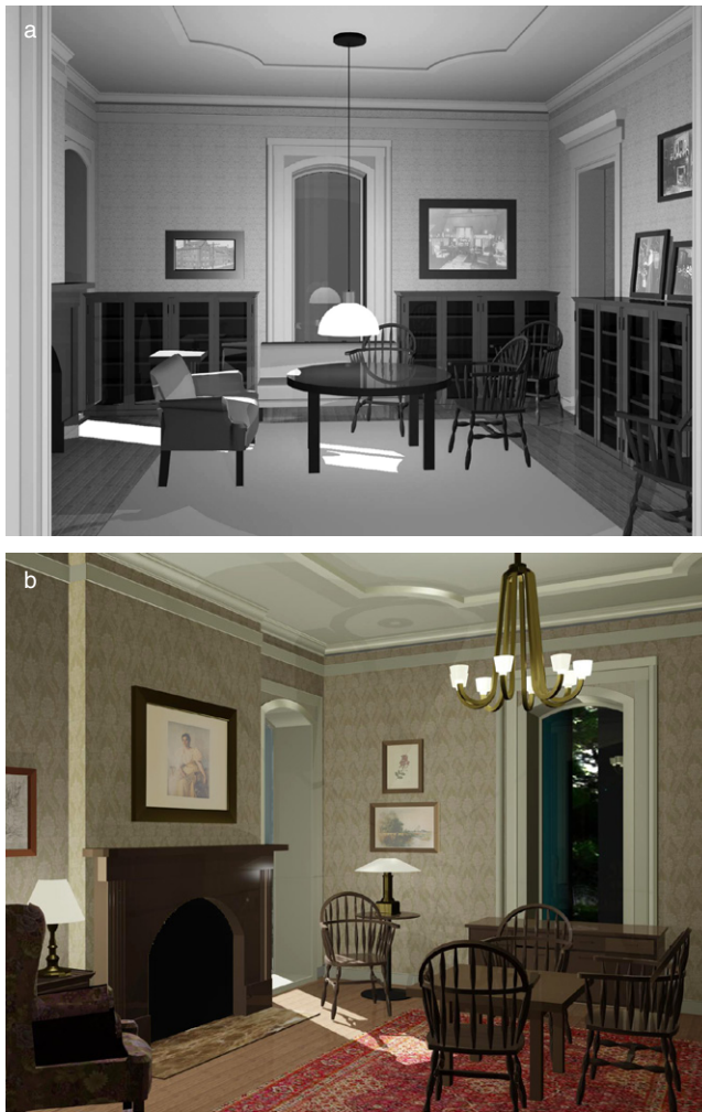
Figure 5.2 Southwest parlor before and after restoration. Images by author.
