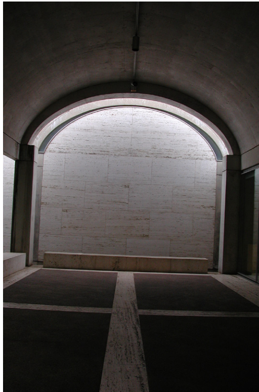
Figure 18.3 End wall daylight detail in the Kimbell Museum, Fort Worth, Texas. Designer: Louis I. Kahn. Photo: M. Kroelinger.
