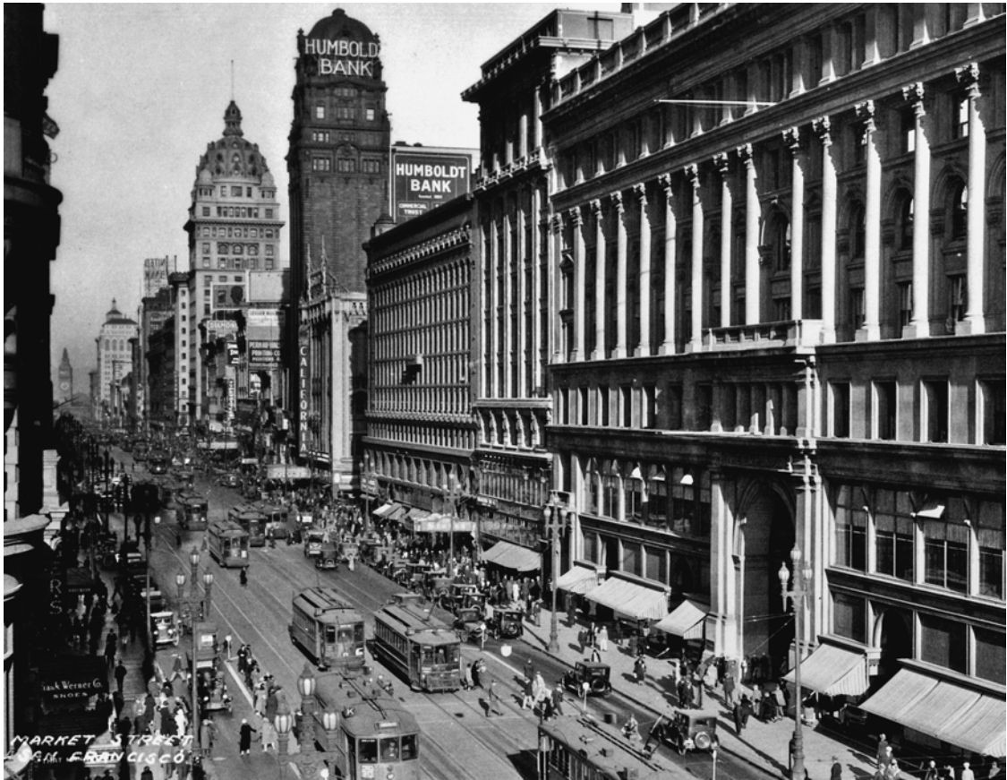
Plate 6 A modern downtown of the 1920s. One of the urban features that Friedrich Engels noted in mid-nineteenth-century Manchester, England, was the appearance of large streets where the upper classes could travel without coming into contact with the squalid living conditions of the residential slums that comprised the greater part of the city. This image of bustling Market Street in San Francisco about 1925 is typical of the new downtown of the modernist period. Note the way streetcars, buses, automobiles, and pedestrians all share the public space.
