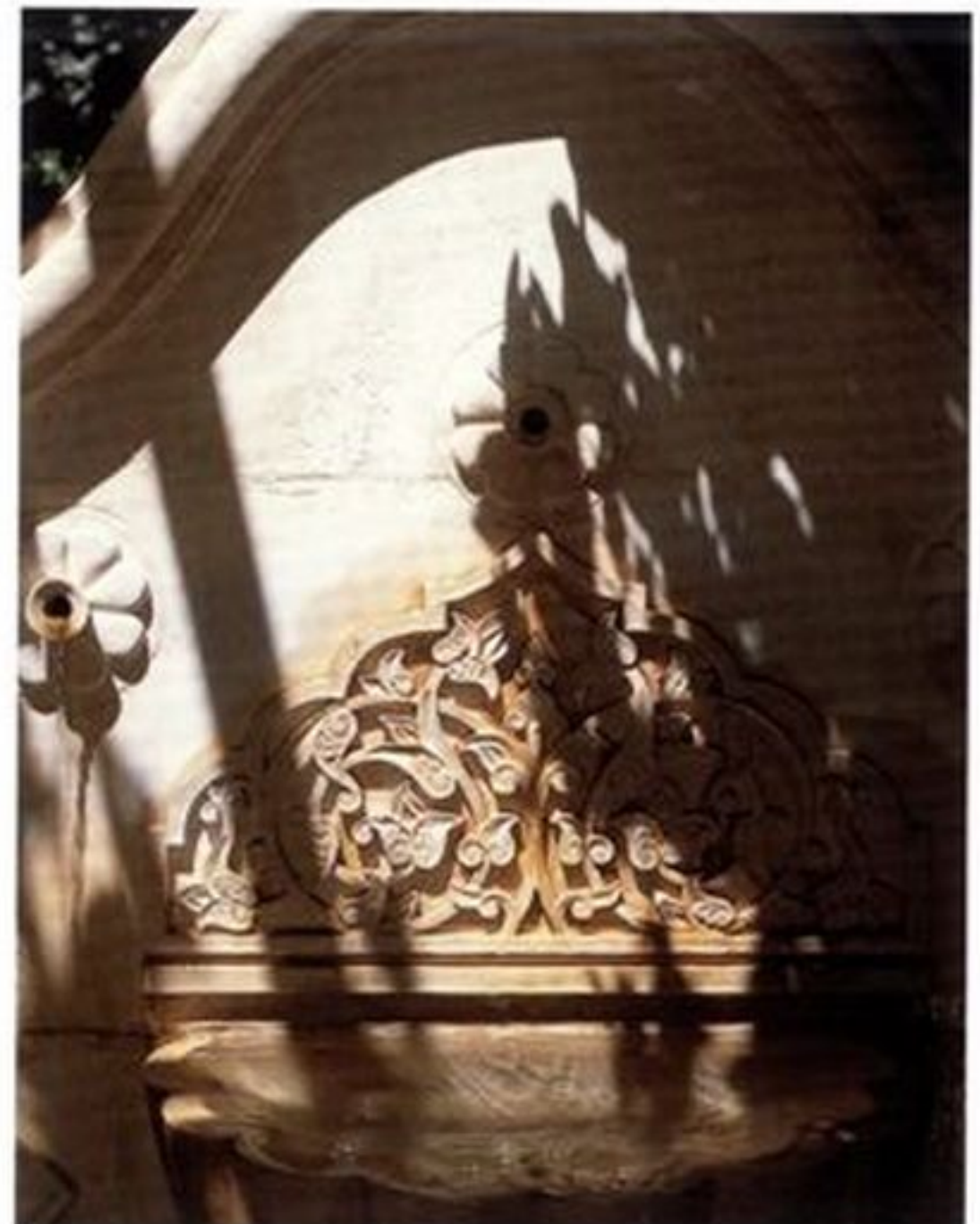
Above and right Al-Talhouni residence, Amman, Jordan. The orientation of each courtyard must be carefully adjusted to permit maximum airflow, with sectional proportions adjusted accordingly. The carved water fountains (right), designed by Rasem Badran's late father, Jamei Badran, serve an environmental purpose as well, cooling the air.
