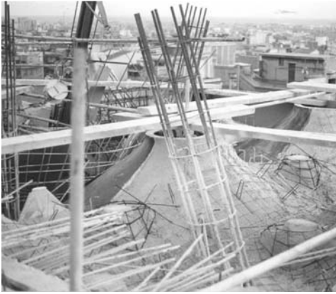
Figures 9. Polyester moulds of the lateral naves.
