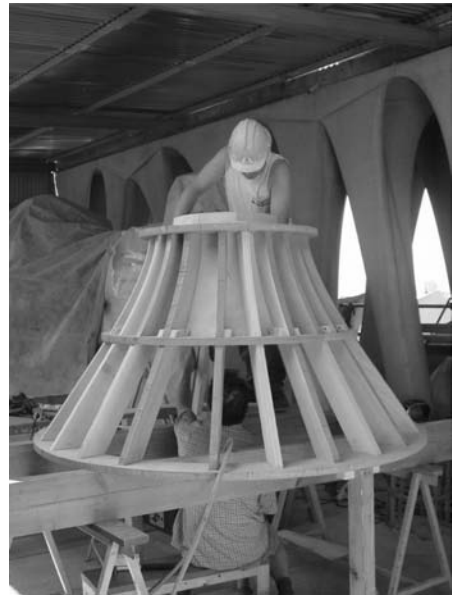
Figures 10. Hyperboloids produced with wooden ribs.
