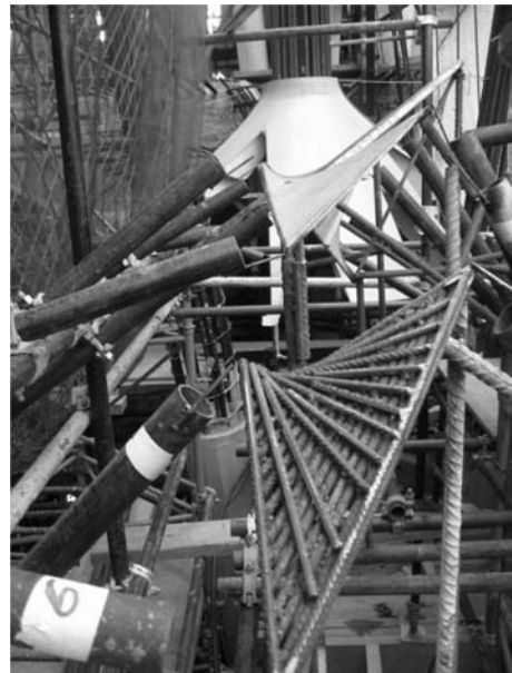
Figures 11. Hyperbolic paraboloids.
