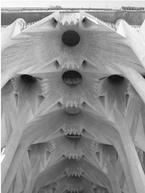
Figures 12. Flat-brick vaults (Catalan vault) hyperbolic paraboloids.
