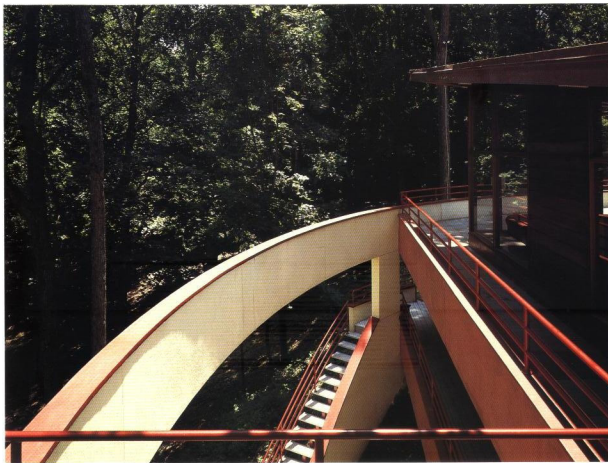
Addition to Usonian House 57 “美国风”住宅扩建
