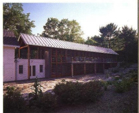
Opposite Page and Above: The roofs of the old farmhouse and the new addition are separated, gable end to gable end, establishing kinship and individual identity at the same time.
