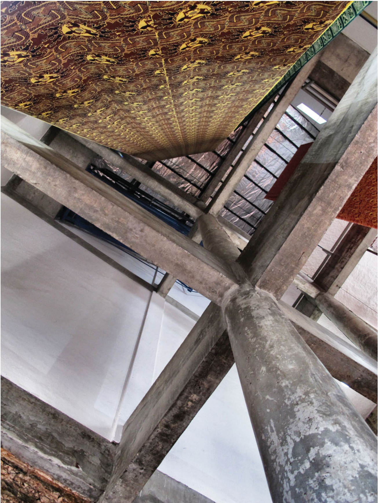
Casa do Olodum's ceiling structure, Afro-Brazilian cultural centre (Photo Calabrese)
