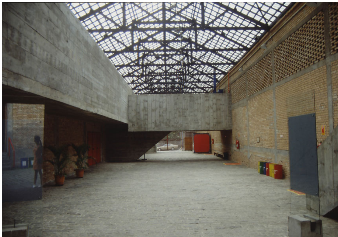
SESC Pompeia Complex Theatre entrance (Photo Calabrese)
