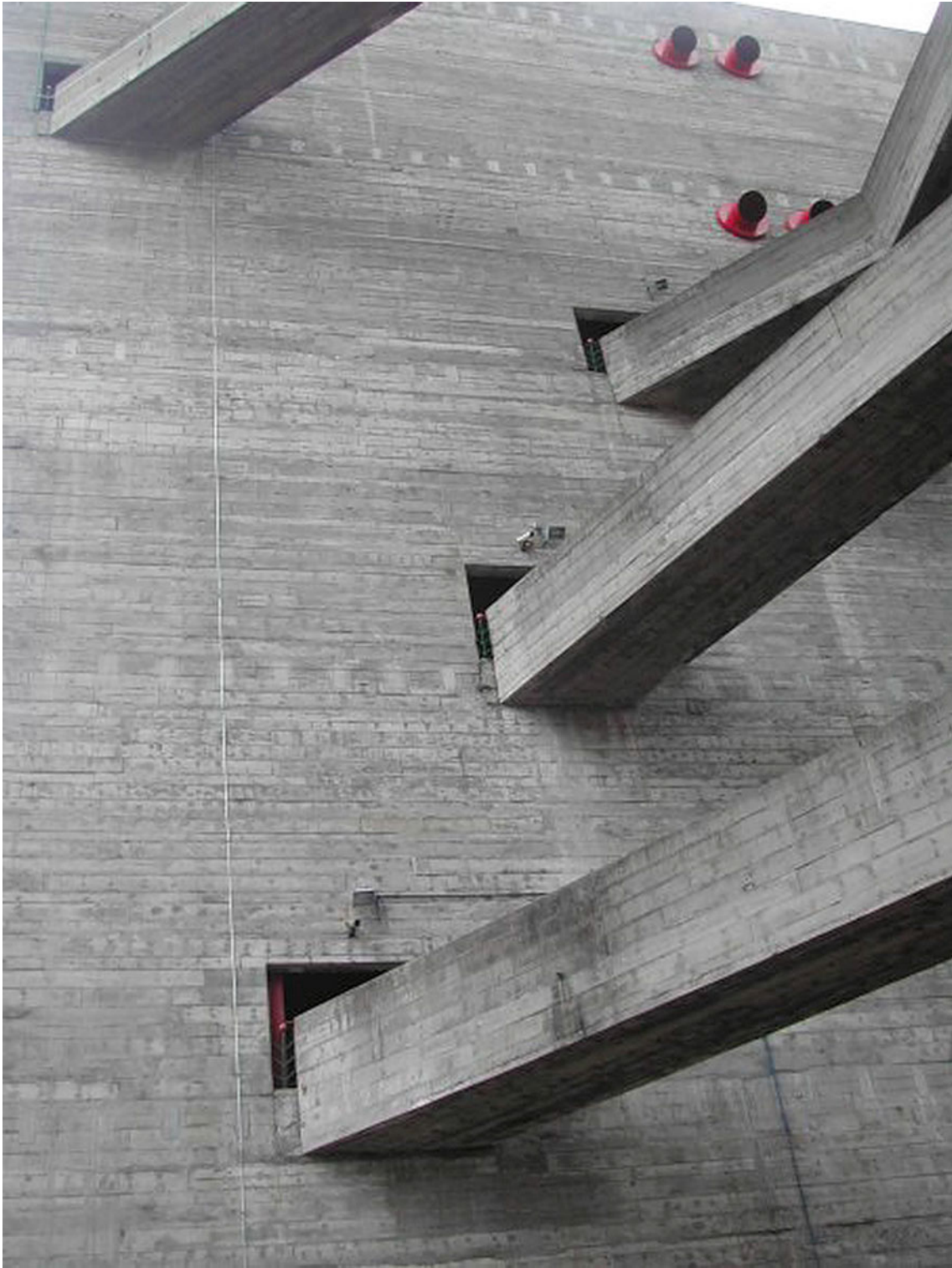
View of concrete walkways and “cactus” balustrades ( Photo Lehmann )
