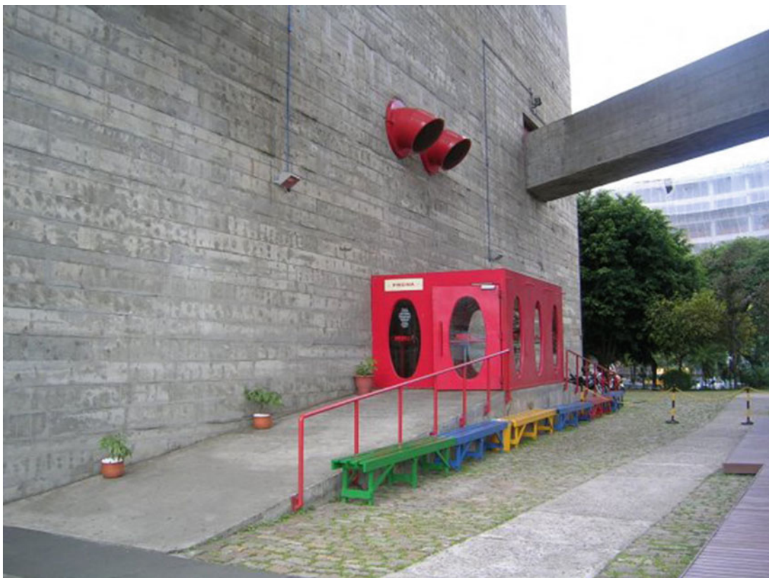
Exterior of the SESC new tower and concrete bridge ( Photo Lehmann )
