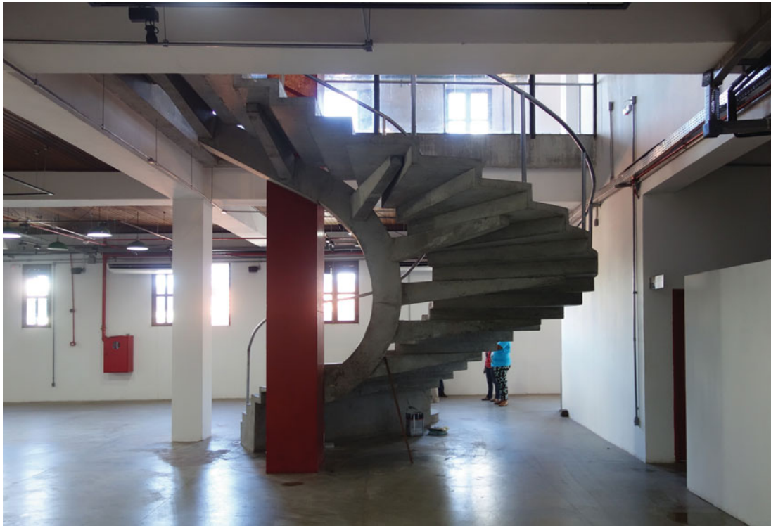
MAM interior: the large timber spiral staircase Escada de Madeira in the Solar do Unhão , Salvador (Photo Anelli)
