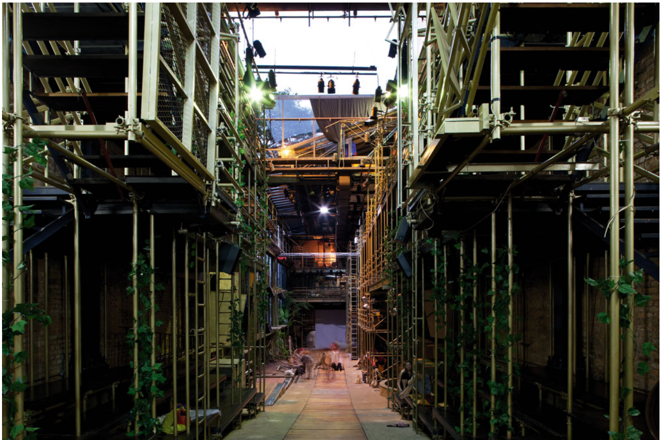
Fig. 3.13 Teatro Oficina, Lina Bo Bardi in collaboration with Edson Elito. Permanent scaffolding with climbing vines interpreted herein as a tropical fire-escape (Photo Leonardo Finotti 2009)
