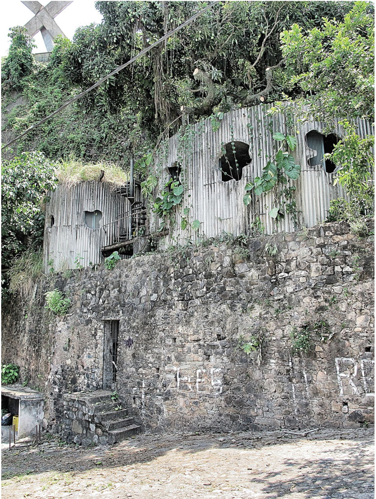
Ladeira da Misericórdia with the Restaurante do Coaty, Salvador, Bahia; in collaboration with architect-engineer João Lele Filgueiras Lima, 1987-88 (Photo Calabrese)
