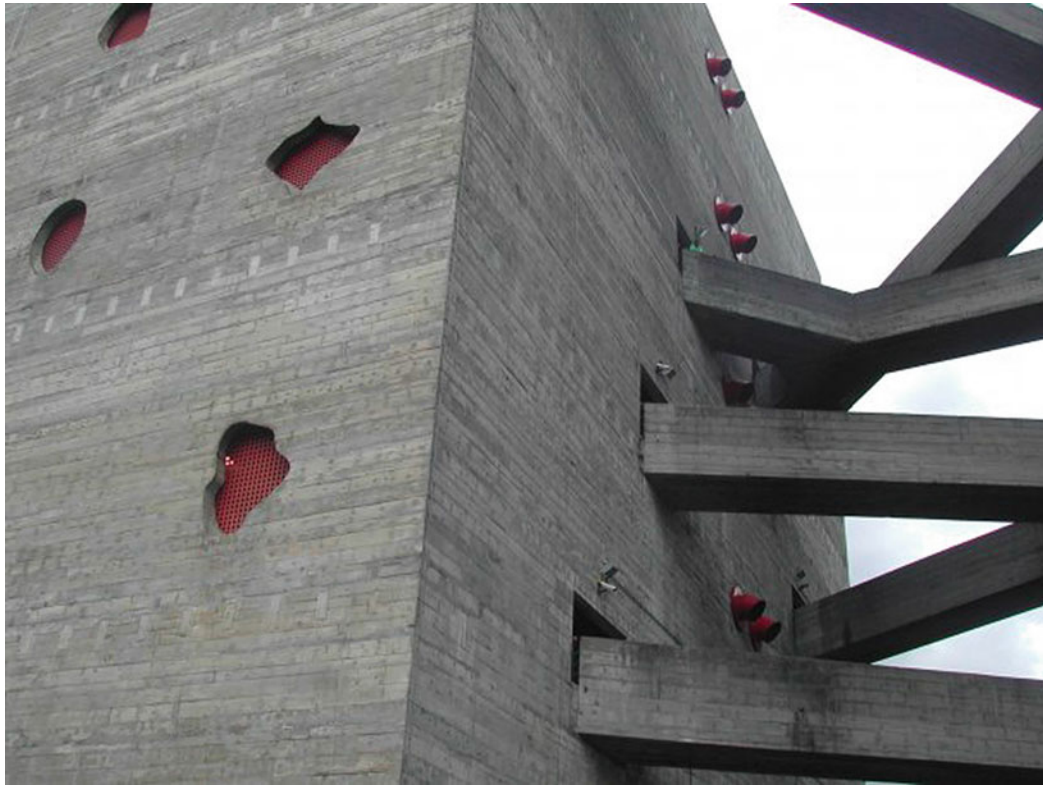
Rusticated openings in the new concrete tower and walkways ( Photo Lehmann )
