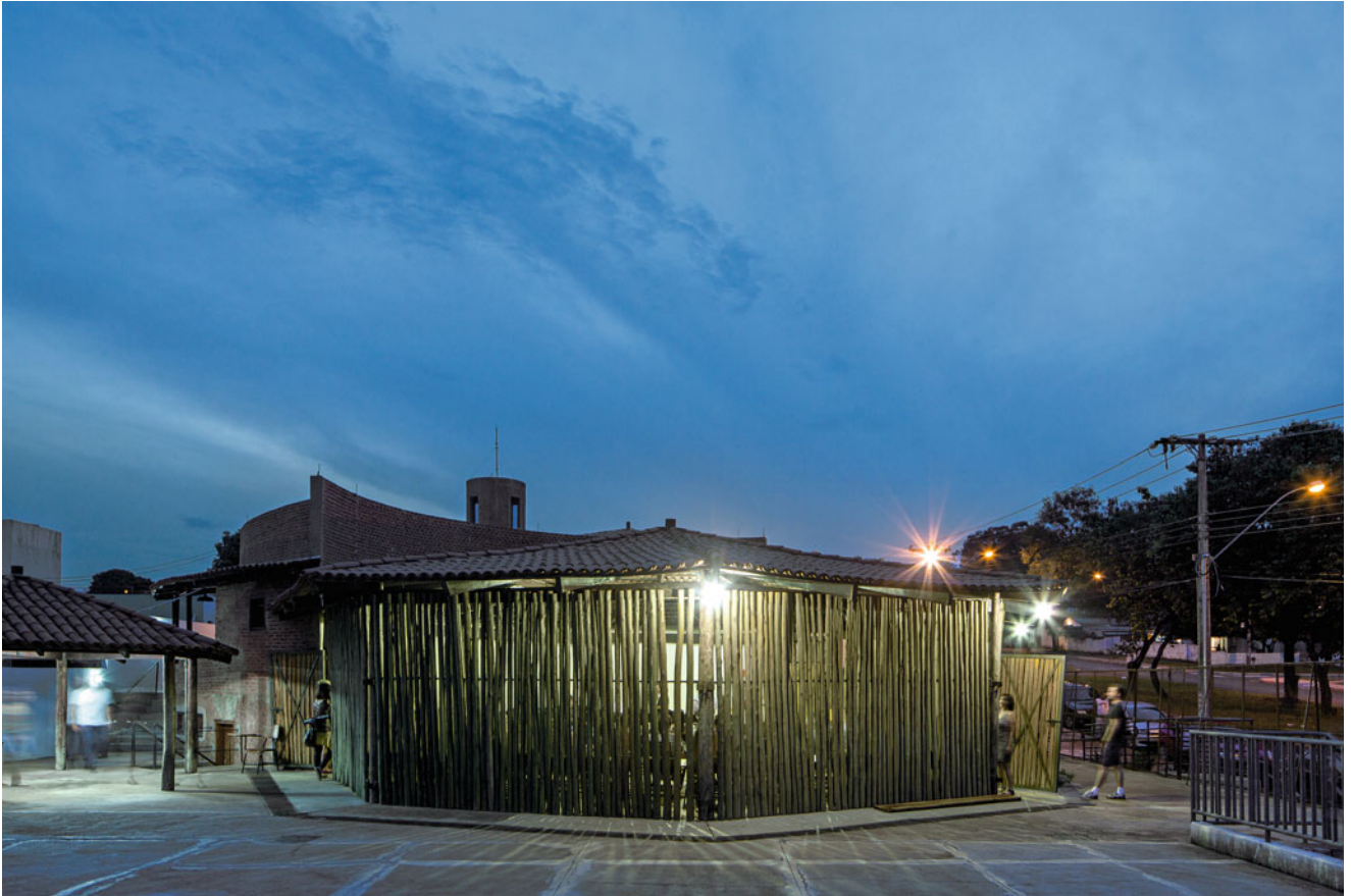
Espirito Santo Cerrado Church exterior showing slender eucalyptus trunks to encourage air to flow through the structure – a rustic brise-soleil, Uberlandia, Minas Gerais, 1976-1982 (Photo Finotti)
