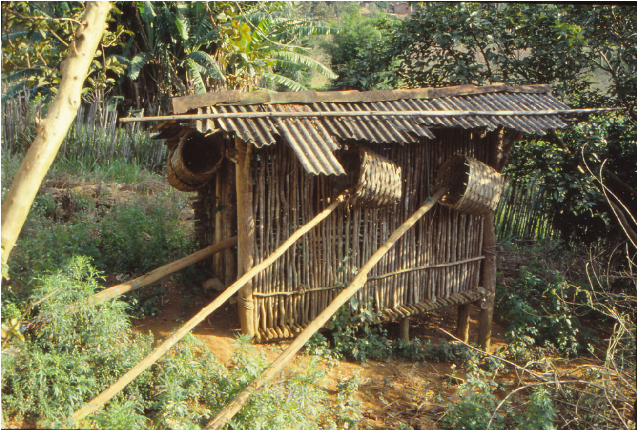
Fig. 3.15 Traditional chicken coup construction with hammock-type baskets, an early rustic brise-soleil Bo Bardi's adapted for the Cerrado Church (Photo Marcelo Ferraz)
