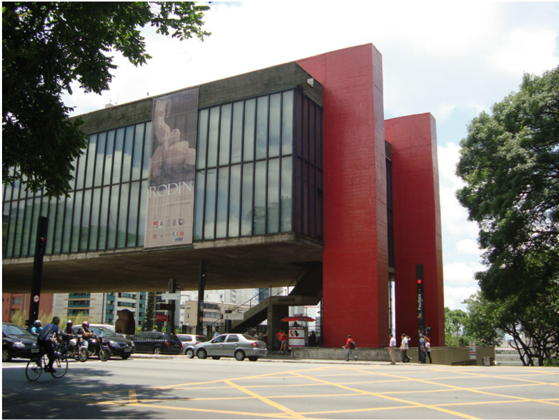
Exterior of the MASP ( Photo Lehmann )
