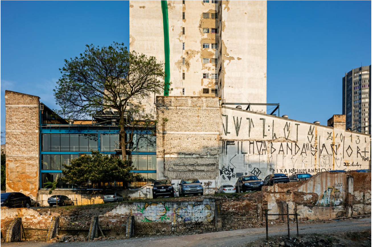
View of the Teatro Oficina from the carpark (Photo Finotti)
