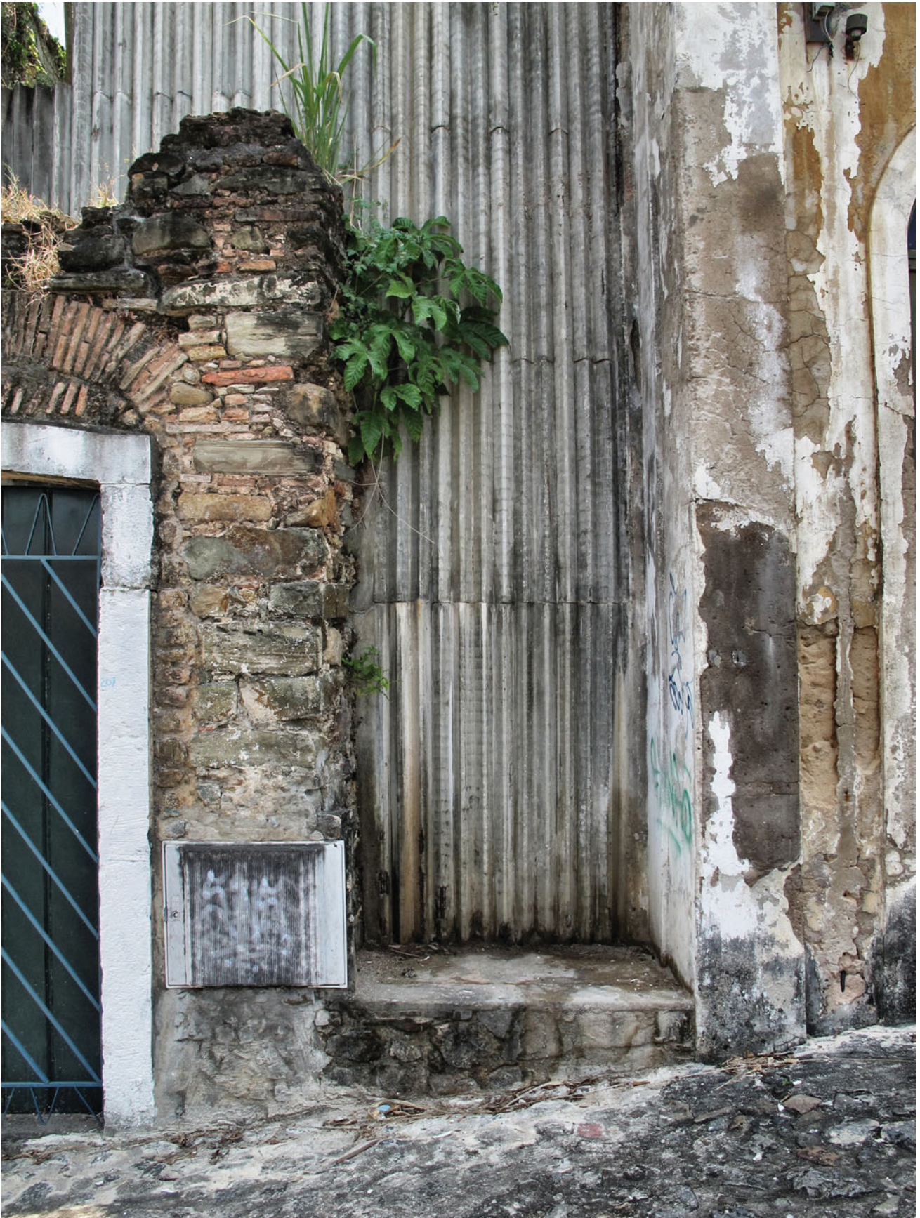
Detail of the crinkled concrete panel and the existing fragments, Ladeira da Misericórdia with the Restaurante do Coaty (Photo Calabrese)
