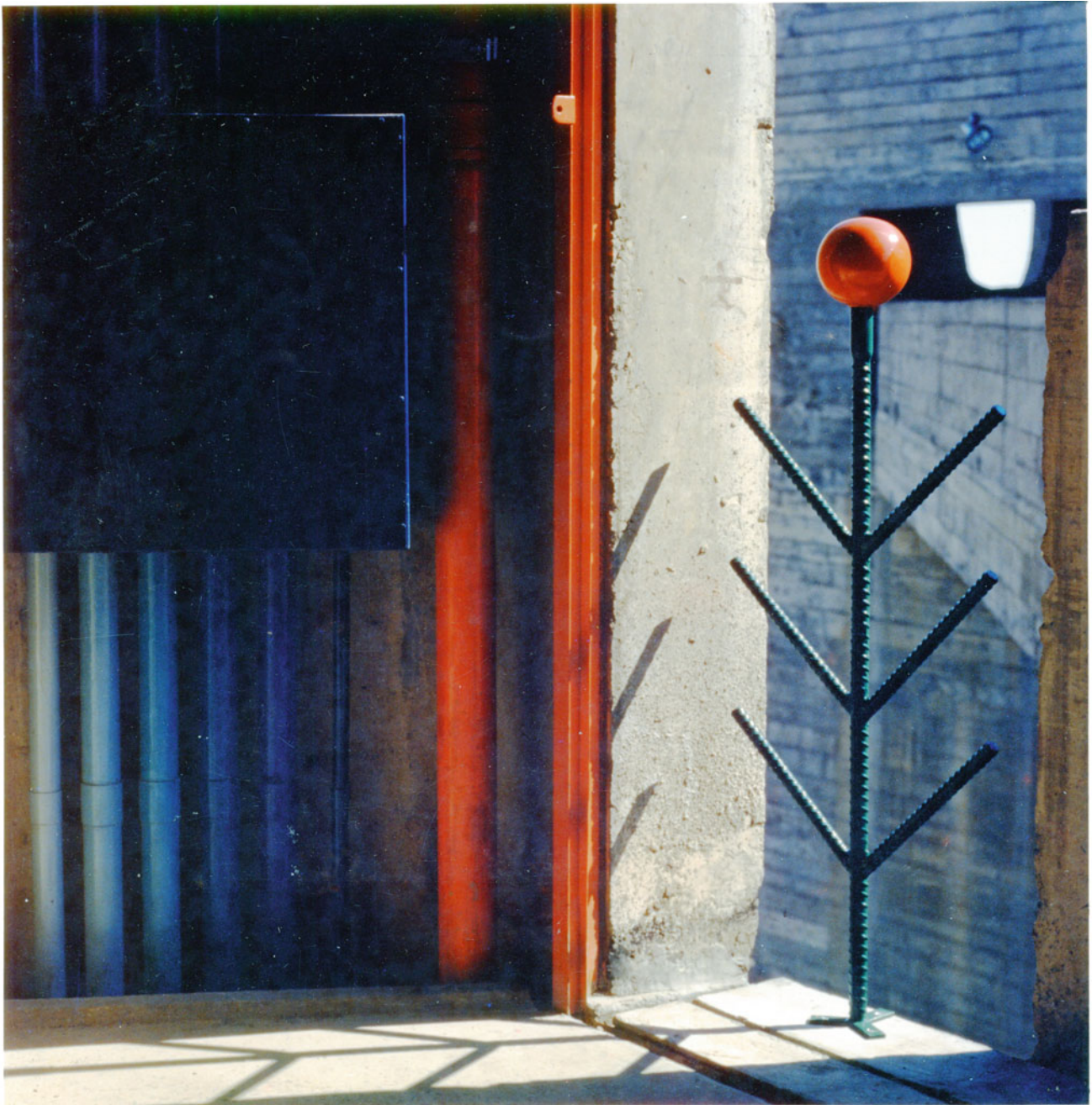
Fig. 3.11 SESC Pompeia's "vertical beach" with steel cactus flowers. Mandacaru cactus flower made out of steel reinforcement rod cut-offs welded together and used as balustrades located on each floor in pairs within the gymnasium tower (Source Instituto Lina Bo e PM Bardi)
