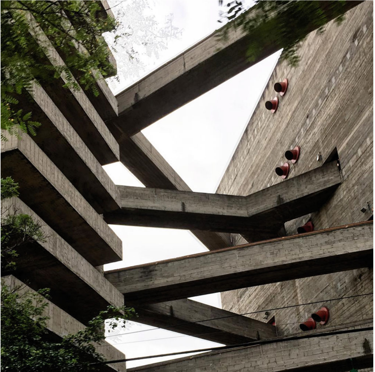
SESC Pompeia Leisure Centre in São Paulo. The concrete bridges between the new towers connecting the sports facilities with change rooms ( Photo Lehmann )
