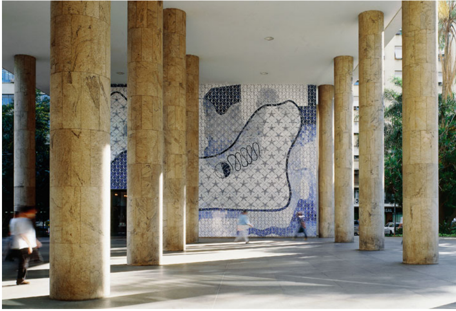
Pilotis system at the MES building ( Photo Kon )
