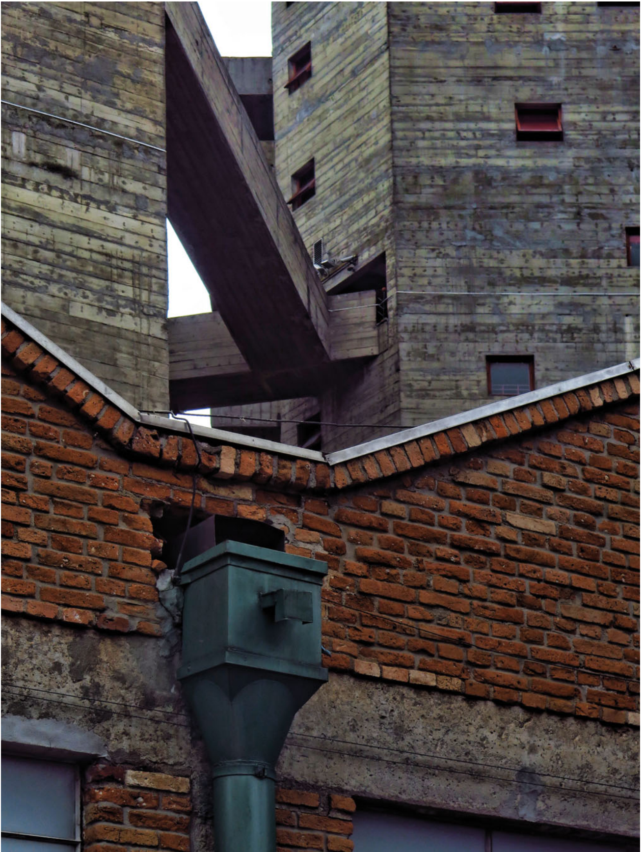
Junction between the old and new, SESC Pompeia building ( Photo Federico Calabrese )
