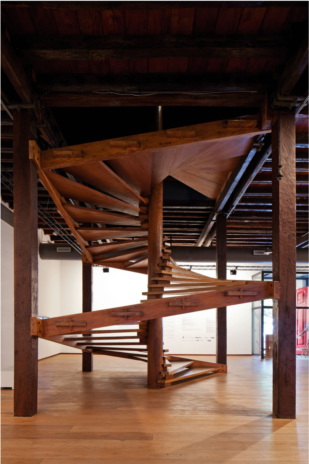
Solar do Unhão complex timber staircase, Salvador (Instituto Lina Bo e PM Bardi)
