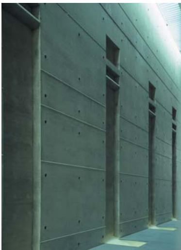
▲ 2.16 Texture and niches of the condolence hall side-walls.
