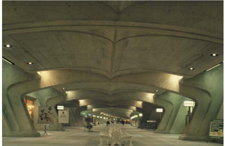
▲ 7.51 Stadelhofen Railway Station, Zürich, Switzerland, Santiago Calatrava, 1990. Cambering the beams and the 'sloping columns' visually lighten the shopping mall.
