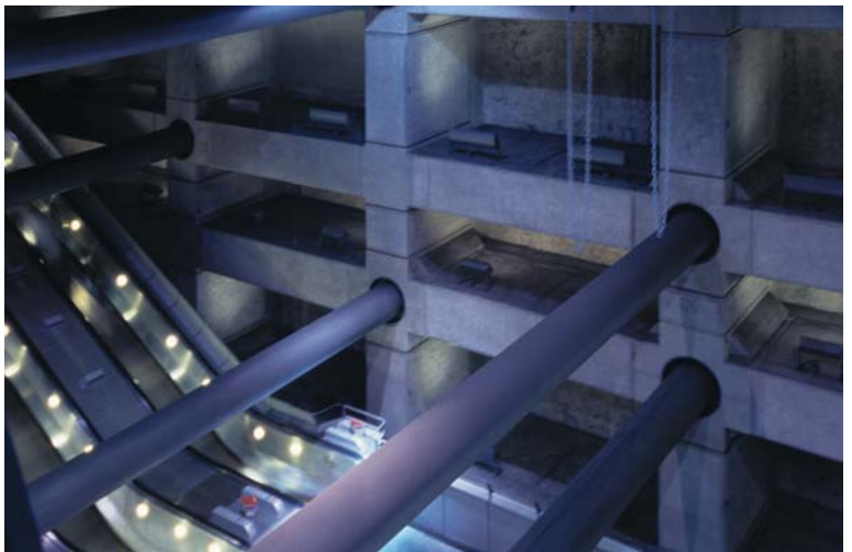
▲ 6.33 Horizontal props between side walls.
