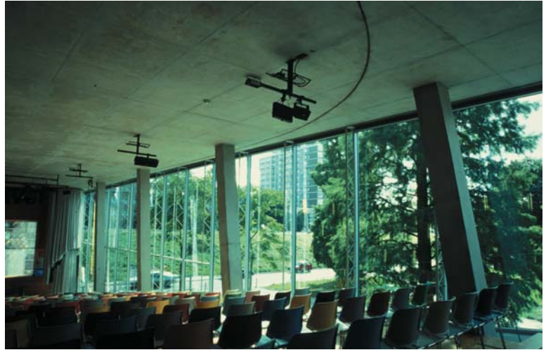
▲ 6.35 Kunsthall, Rotterdam, The Netherlands, Office for Metropolitan Architecture, 1992. Columns in the auditorium lean towards the dais.
