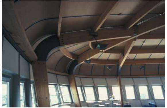
▲ 3.29 The curved roof structure.
