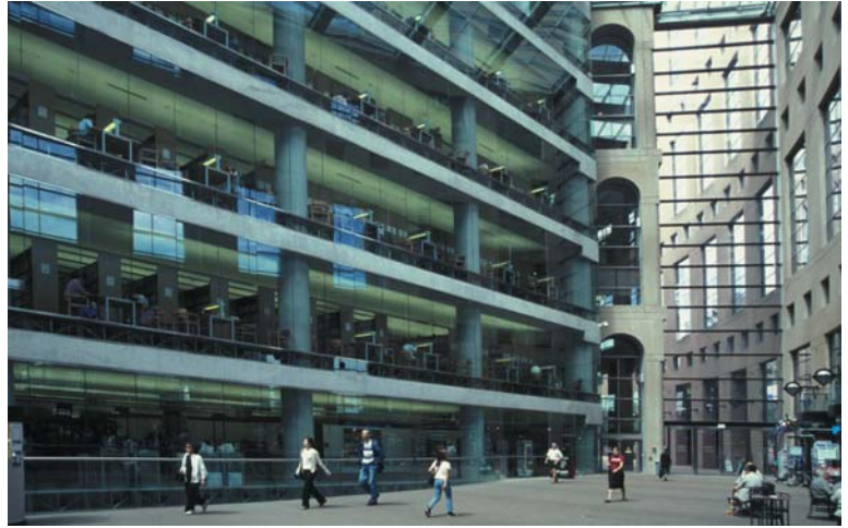
▲ 3.1 Library Square, Vancouver, Canada, Moshe Safdie and Associates Inc., 1995. A typical longitudinal frame and the end of a perimeter transverse frame.
