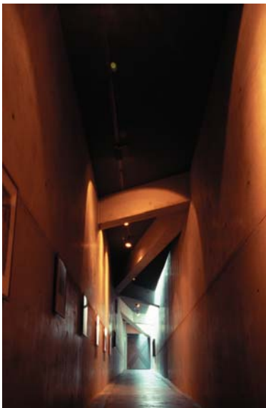
▲ 9.24 Felix Nussbaum Museum, Osnabrück, Germany, Daniel Libeskind, 1998. Dysfunctional concrete beams in the Nussbaum Corridor.
