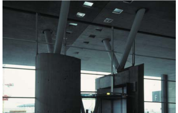
▲ 4.31 A 'split-column' viewed from inside.
