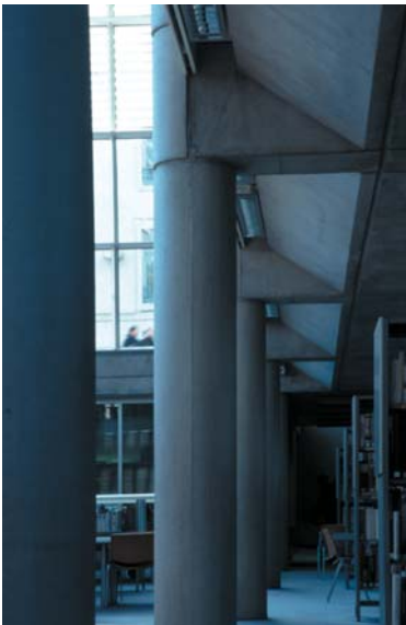
▲ 8.20 Bevelled and set-back beams.
