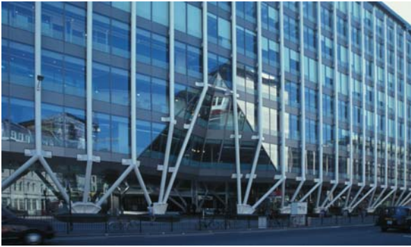
▲ 3.42 Fleet Place House, London, England, Skidmore, Owings & Merrill, 2000. Angled columns add interest to the main façade.
