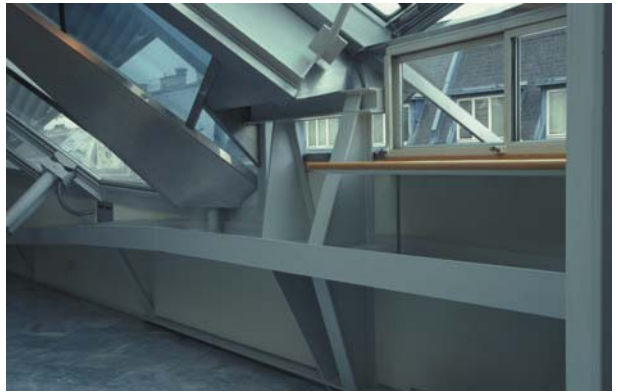
▲ 7.47 Irregularity of the form is reflected in the detailing.
