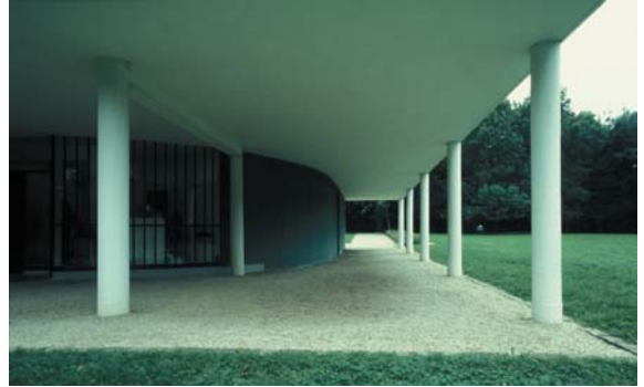
▲ 7.65 Plain exterior column and beam detailing.
