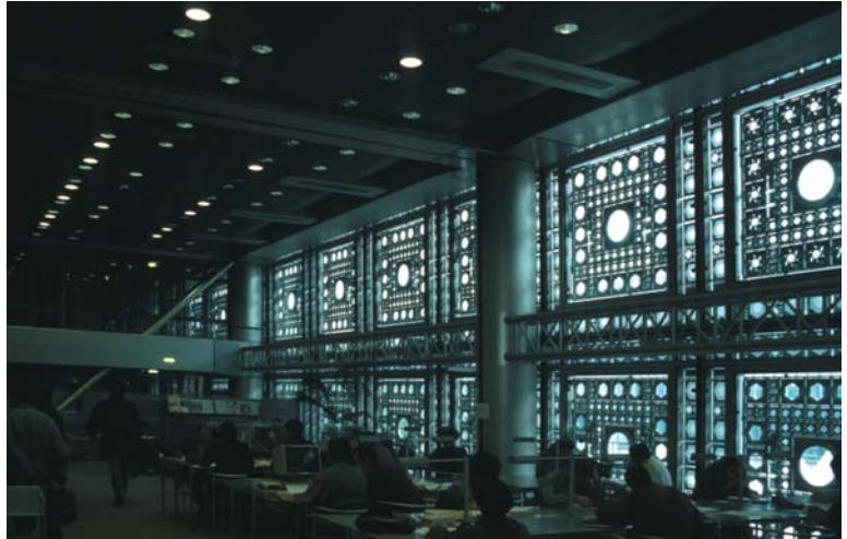
▲ 7.55 Internal horizontal trusses in the library.
