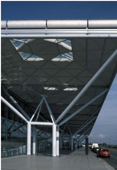
▲ 4.25 Stansted Airport terminal, Essex, England, Foster Associates, 1991. Portico 'trees' are an extension of the interior structure.
