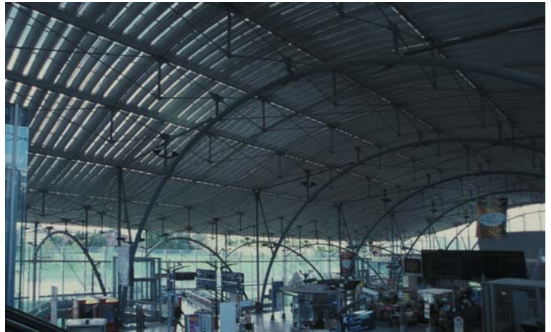
▲ 3.46 Unexpected interior arches in the TGV Station.
