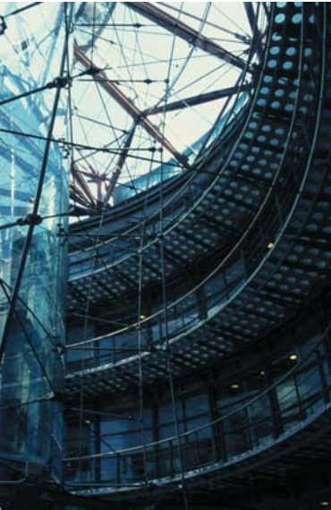
▲ 6.38 Channel 4 Headquarters, London, England, Richard Rogers Partnership, 1995. Atrium interior.
