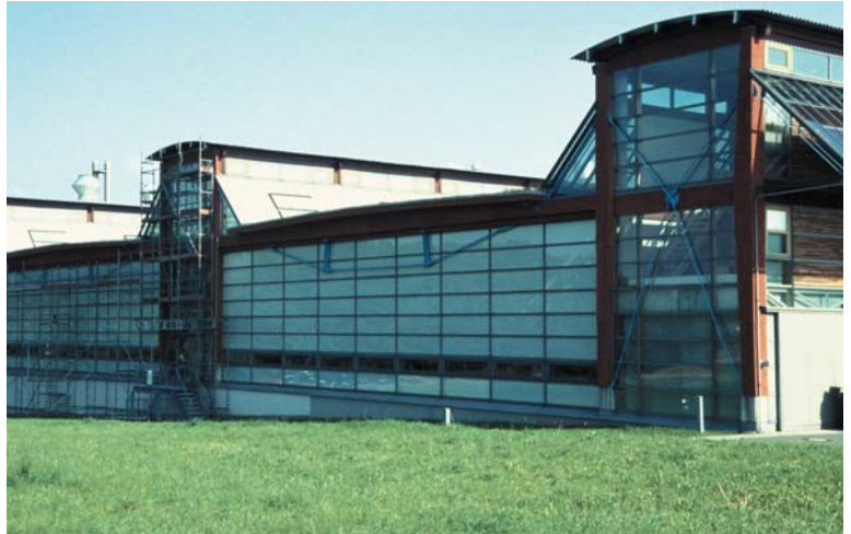
▲ 4.27 Wilkhahn Factory, Bad Münden, Germany, Herzog with Bernd Steigerwald, 1993. Longitudinal structural form is exposed.
