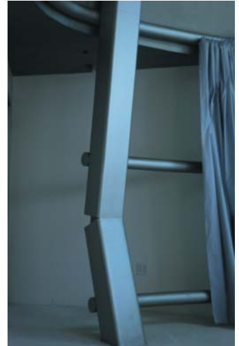
▲ 7.38 A 'broken' post at first-floor level.
