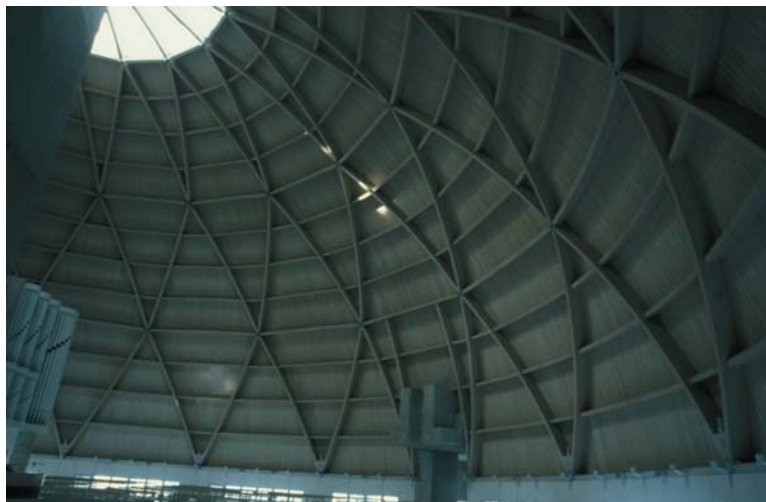
▲ 6.10 Saint Massimiliano Kolbe church, Varese, Italy, Justus Dahinden, 1994. Interior surface.
