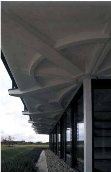
▲ 7.66 Schlumberger Extension building, Cambridge, England, Michael Hopkins and Partners, 1992. Exposed ribbed soffits around the perimeter.
