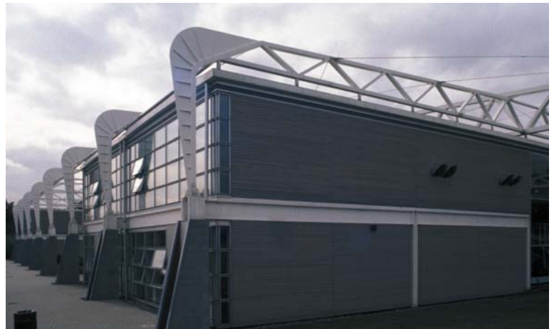
▲ 2.4 Partial portal frames span between the piers and the primary trusses or core walls.
