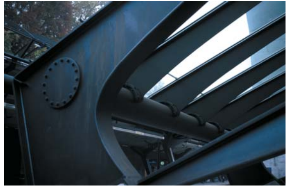
▲ 7.28 Upper cantilever-to-torsion-beam connection, with smaller canopy cantilevers in the background.
