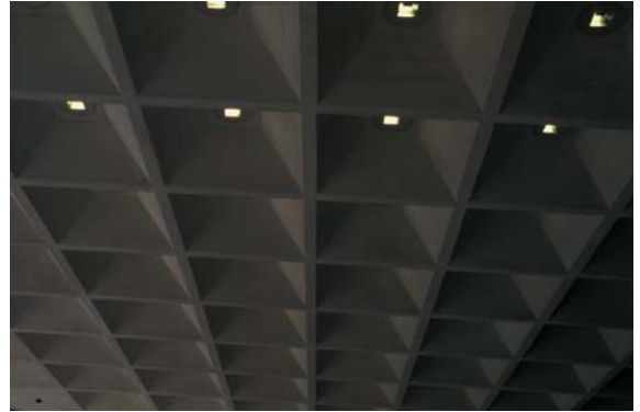
▲ 7.3 Coffered slab soffit.
