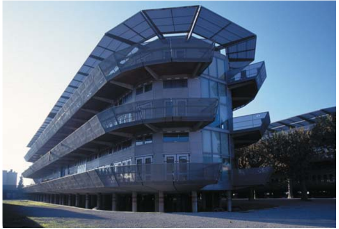
▲ 5.13 Némausus Apartments, Nîmes, France, Jean Nouvel et Associés, 1988. Columns define car parking and their spacing reflects the widths of the apartments above.
