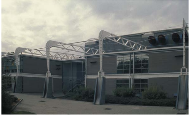
▲ 2.1 BRIT School, Croydon, London, England, Cassidy Taggart Partnership, 1991. Exoskeleton with the core behind the two-storey podium. Ventilation ducts protrude from the core wall.
