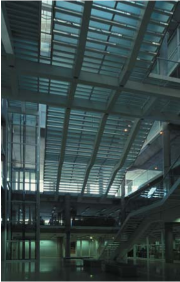
▲ 8.19 Carré d'Art, Nîmes, France, Sir Norman Foster and Partners, 1993. Glass stair-treads and the supporting structure in the atrium.
