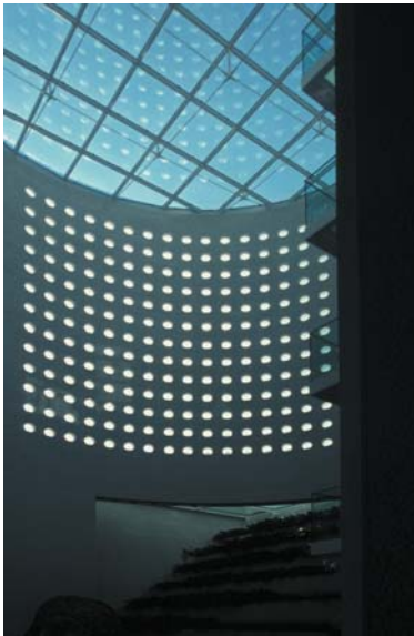
▲ 8.22 Mexican Embassy, Berlin, Germany, González de León and Serrano, 2000. A penetrated circular wall forms part of the atrium.
