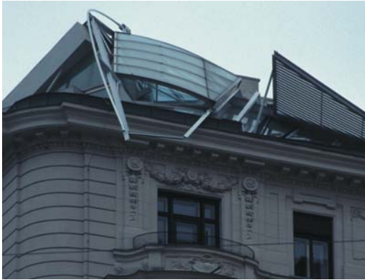
▲ 7.46 Attic conversion, Vienna, Austria, Coop Himmelb(l)au, 1988. The attic roof over-sails the existing building.
