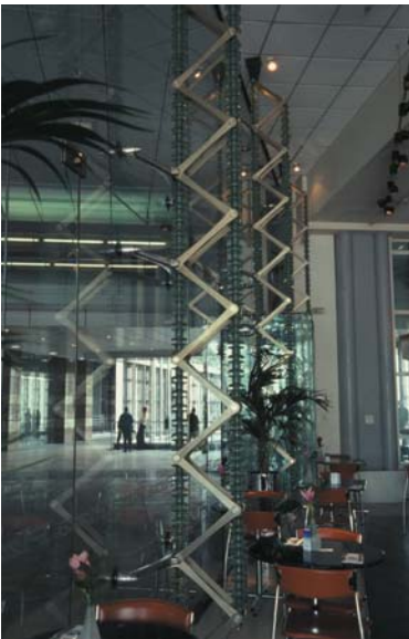
▲ 5.37 Pizza Express Restaurant façade, 125 Alban Gate, London, England, Bere Associates, 1996. Deep window mullions limit the café seating layout.
