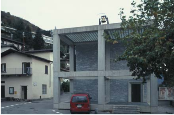
▲ 4.42 Church in Porta, Brissago, Switzerland, Raffaele Cavadini, 1997. Front elevation with a visible gap under the beam.
