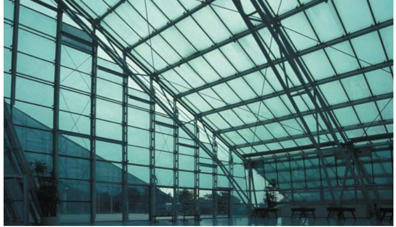
▲ 8.18 Triangular cantilever trusses support the mono-slope glazed roof.
