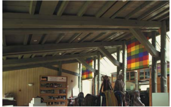
▲ 5.20 A teaching space is separated from the corridor to the right by pairs of columns.
