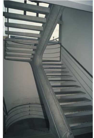
▲ 7.7 Rounded precast concrete stair stringer.
