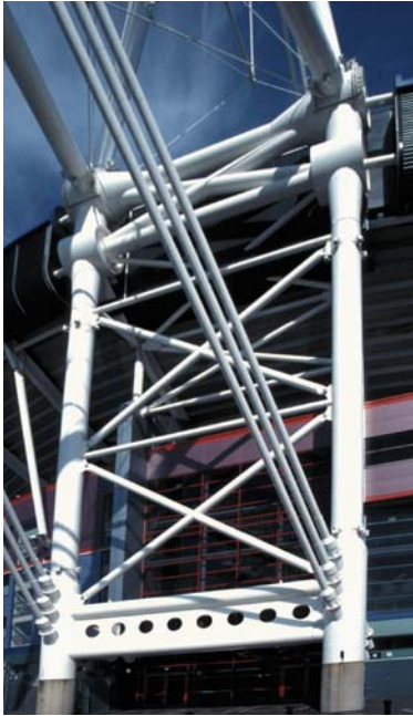
▲ 4.29 Millennium Stadium, Cardiff, Wales, The Lobb Partnership (now HOK Sports), 2000. Main entry is under the beam between the mast legs.
