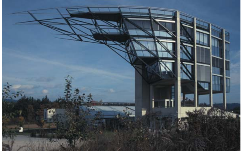
▲ 9.29 Industrial Park Office Building, Völkermarkt, Carinthia, Austria, Günther Domenig, 1996. The framed block supporting the cantilever and the lift and stair tower behind.
