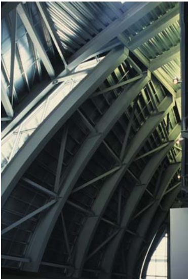
▲ 7.22 Exposed construction of an exterior wall that curves towards the theatre roof.
