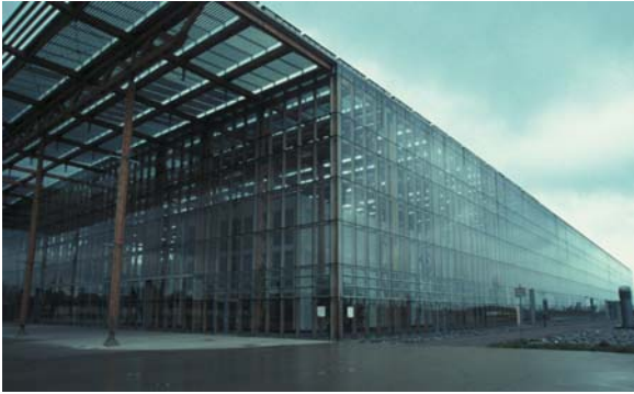
▲ 3.26 Mont-Cenis Academy, Herne, Germany, Jourda & Perraudin, 1999. A glazed box with an entry canopy.
