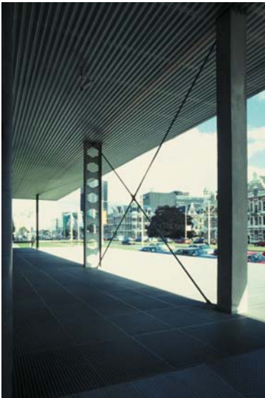
▲ 7.11 Two of the three differently detailed columns.
