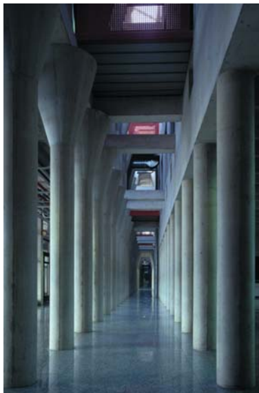
▲ 5.16 Public University of Navarra, Pamplona, Spain, Sáenz de Oiza Arquitectos, 1993. Columns to the left run along the corridor length and those to the right define the corridor width in the absence of side walls.
