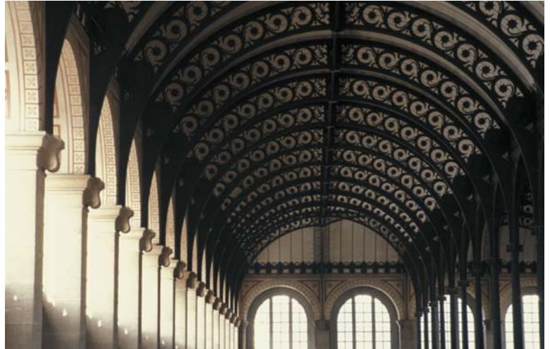
▲ 7.67 Bibliothèque Sainte-Geneviève, Paris, France, Henri Labrouste, 1850. Curved iron beams over the reading room.
