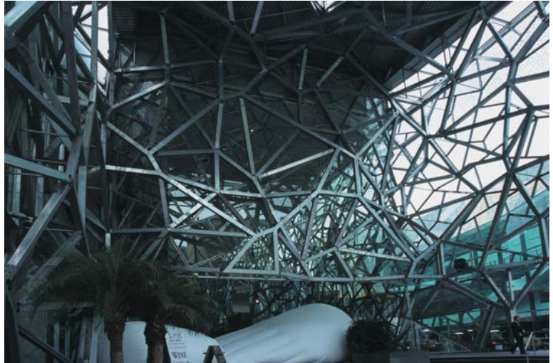
▲ 9.27 Federation Square, Melbourne, Australia, Lab Architectural Studio and Bate Smart Partners, 2002. The tangled structure of the Atrium roof.
