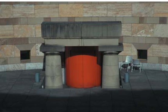
▲ 7.35 Staatsgalerie, Stuttgart, Germany, James Stirling, Wilford & Associates, 1984. A classically detailed structure frames an entrance.
