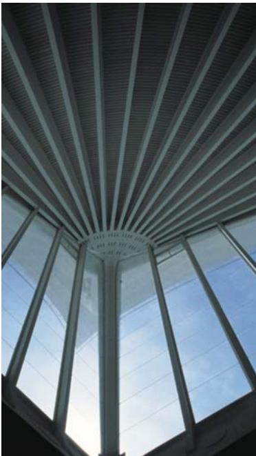
▲ 6.13 Ribs radiate over the entire terminal ceiling.
