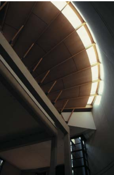
▲ 6.26 The timber roof is propped off an outer frame.
