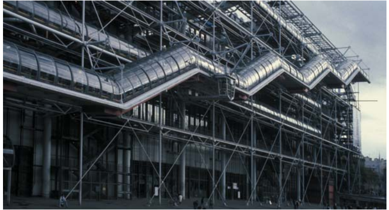
▲ 4.18 Centre Pompidou, Paris, France, Piano and Rogers, 1977. Screening effect of structure on the main façade.
