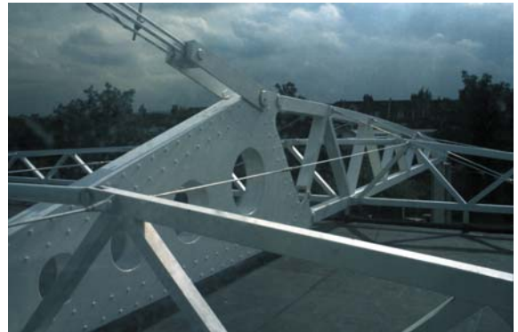
▲ 2.8 Primary truss near its connection to the core.
