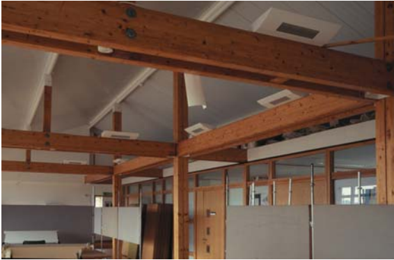
▲ 6.16 Portland Building, University of Portsmouth, England, Hampshire County Council Architects Department, 1996. The timber framework creates spatial zones within a studio.
