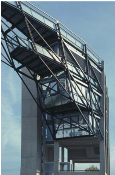
▲ 9.30 Steelwork of the braced cantilever structure.
