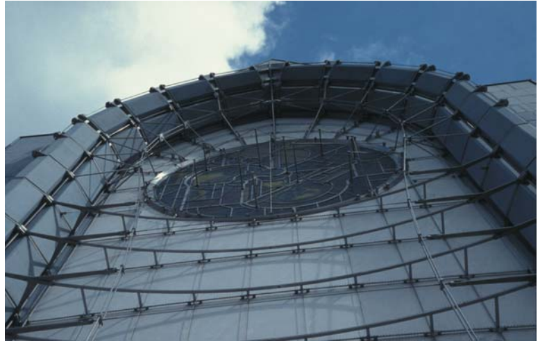
▲ 4.21 Horizontal steel structure spans between columns of a prestressed stone arch.
