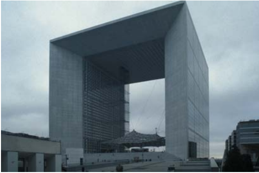
▲ 3.18 La Grande Arche, Paris, France, Johan Otto van Spreckelsen, 1989. Frames within a frame.
