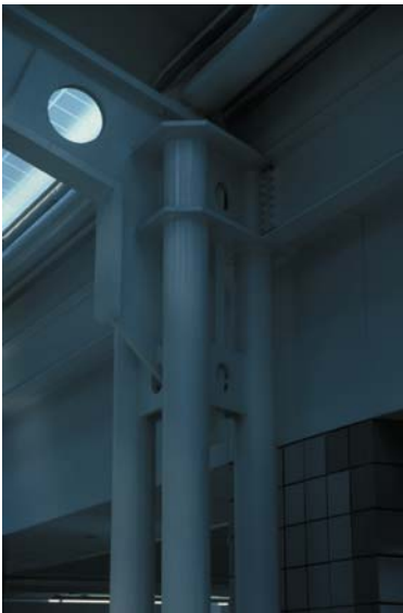
▲ 7.13 Beam-column junction.
