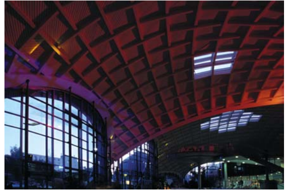
▲ 5.5 Open structure-free space under the shell roofs.
