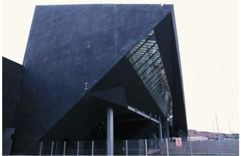
▲ 3.53 Stealth Building, Culver City, USA, Eric Owen Moss Architects, 2001. Triangular form at the northern end.
