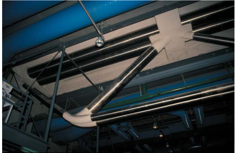
▲ 7.53 Centre Pompidou, Paris, France, Piano and Rogers, 1977. Double-chords reduce the visual mass of the truss.
