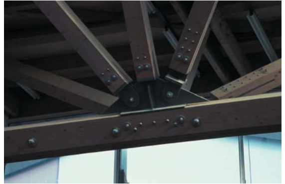
▲ 7.24 Web members connect to a truss bottom-chord.
