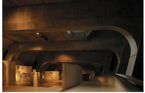
▲ 6.31 Concrete frames extend over the galleries and corridor. The sloping columns express the hill-side embedment of the building.
