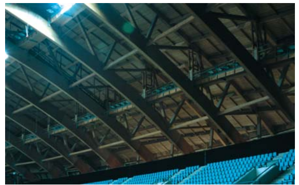
▲ 9.16 Timber trussed-arches over-sail the seating.
