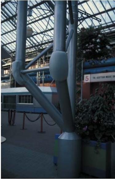
▲ 5.41 Scottish Exhibition Centre, Glasgow, Scotland, Parr Partnership, 1985. Knee pads on truss-columns.
