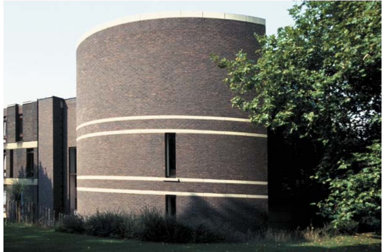
▲ 4.35 Fitzwilliam College Chapel, Cambridge, England, Richard MacCormac, 1991. A chapel side-wall with an accommodation block to the left.
