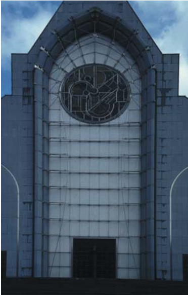
▲ 4.20 Cathédrale Notre Dame de la Treille, Lille, France, Pierre-Louis Carlier architecte, 1997. A steel filigree structure supports the nave wall.
