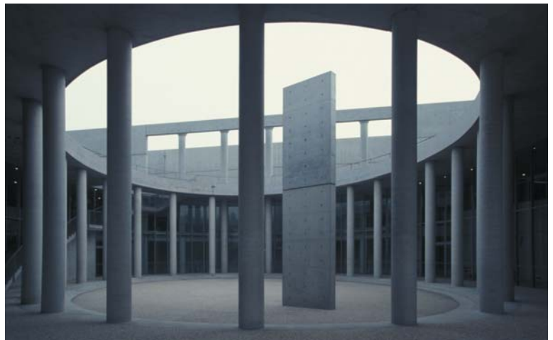
▲ 7.16 FABRICA (Benetton Communication Research Centre), Treviso, Italy, Tadao Ando & Associates, 2000. Concrete construction and materiality are clearly expressed in the structural elements defining the sunken courtyard.
