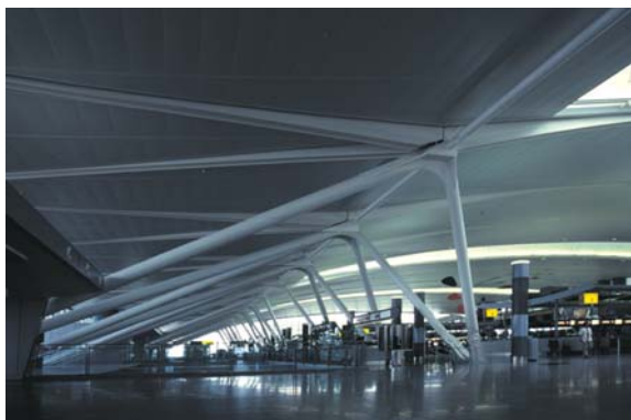
▲ 5.17 JFK Airport Terminal 4, New York, USA, Skidmore Owings & Merrill, 2001. Structure occupies the entry zone with the entrances to the left.
