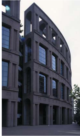
▲ 4.15 Library Square, Vancouver, Canada, Moshe Safdie and Associates Inc., 1995. A gap reveals the cross-section of the screening frame and a glimpse of the main library block behind.
