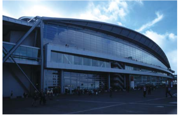
▲ 5.8 Frankfurt Messehalle 3, Frankfurt, Germany, Nicholas Grimshaw & Partners, 2001. Buttressing struts and ties for the arched roof structure penetrate the services and circulation zones located along the sides of the hall.
