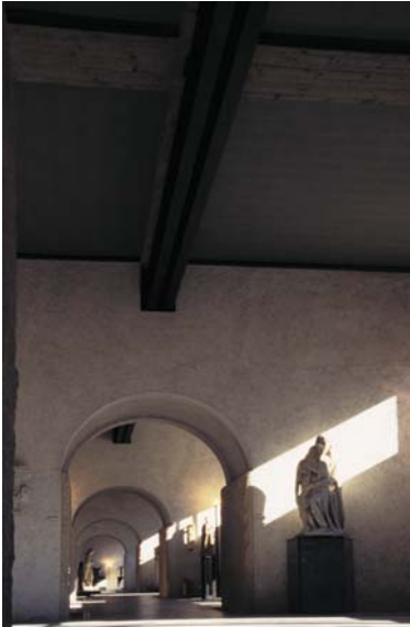
▲ 5.32 Museo di Castelvecchio, Verona, Italy, Carlo Scarpa, 1964. A central beam under the ceiling helps to articulate the linear circulation route.
