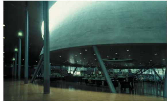
▲ 5.22 The circulation desk beneath the cone is surrounded by steel struts.
