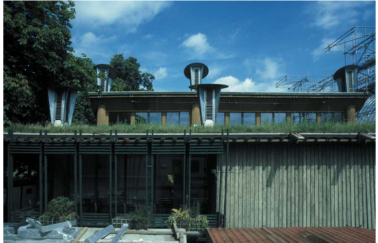
▲ 7.62 Centre for Understanding the Environment (CUE), Horniman Museum, London, England, Architype, 1997. Front façade with chimney-columns.
