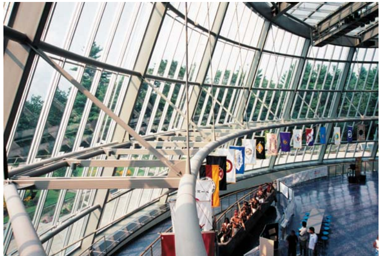
▲ 3.32 The horizontal arch supports the curved and sloping wall.
