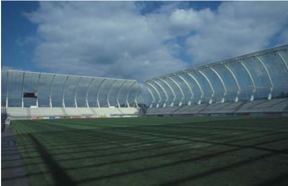
▲ 3.13 Licorne Soccer Stadium, Amiens, France, Chaix & Morel et Associés, 1999. Curved ribbed walls enclose the pitch and spectators.
