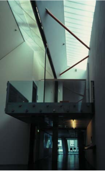
▲ 6.37 An ambiguous relationship between a cantilevering slab and a tension-tie from the roof.
