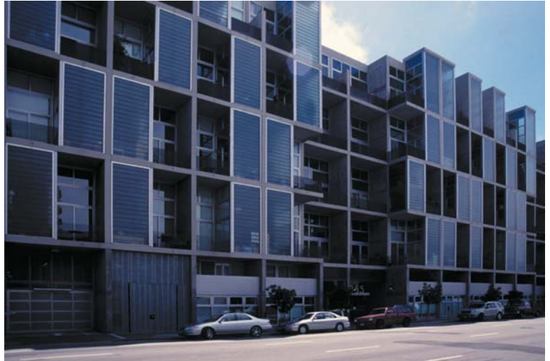
▲ 4.3 Yerba Buena Lofts, San Francisco, USA, Stanley Saitowitz Office/Natoma Architects, 2002. Walls and slabs modulate the front façade.
