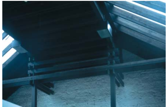
▲ 7.34 An elaborate roof-beam bracket.
