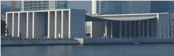
▲ 3.9 Portuguese Pavilion, Lisbon, Portugal, Alvaro Siza, 1998. The canopy drapes between two porticoes.
