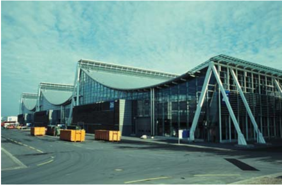
▲ 3.11 Hall 26, Trade Fair, Hanover, Germany, Herzog + Partner, 1996. Three catenaries span between masts.
