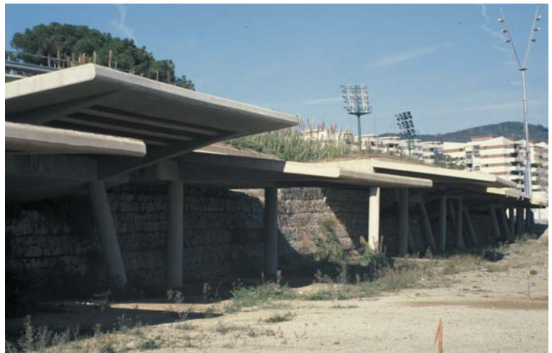
▲ 4.38 Olympic Archery Complex, Barcelona, Spain, Miralles and Pinos, 1991. Aimlessly directed columns support slabs passing over the retaining wall.
