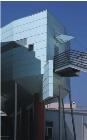
▲ 9.14 The main columns align with the keel and are flanked by stabilizing posts.
