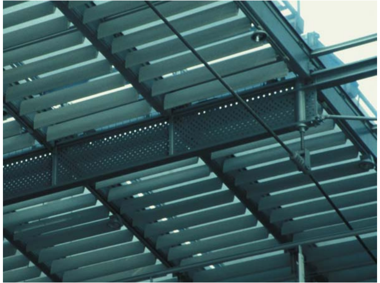
▲ 8.21 Schools of Geography and Engineering, Marne-la-Vallée, Paris, France, Chaix & Morel, 1996. A finely perforated web of a steel beam.
