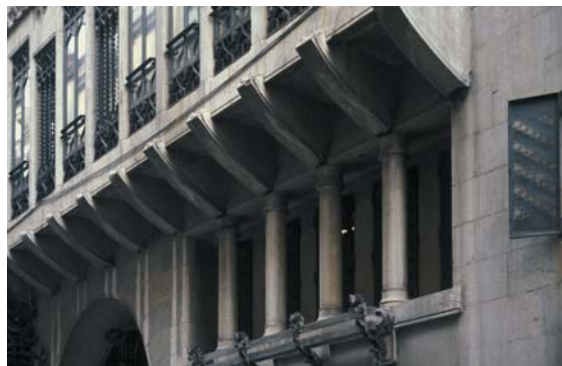
▲ 7.32 Palau Güell, Barcelona, Spain, Antonio Gaudí, 1880. Cantilevering brackets clasp the oriel floor.
