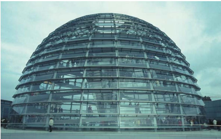
▲ 3.15 The Reichstag Cupola, Berlin, Germany, Foster and Partners, 1999. Radial ribs and circumferential tubes.
