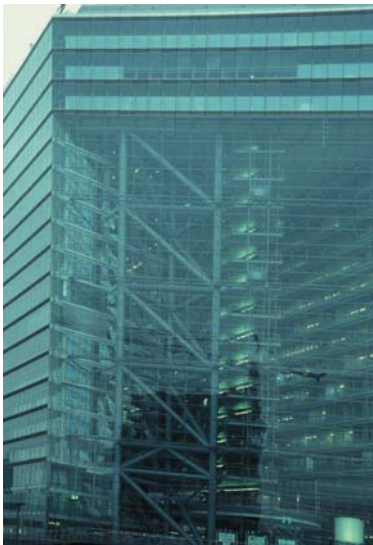
▲ 6.23 Stadttor Building, Dusseldorf, Germany, Petzinka Pink und Partner, 1998. An interior braced tower is visible through the glazing.
