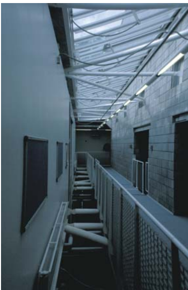
▲ 2.10 Roof and first floor diaphragm bracing.
