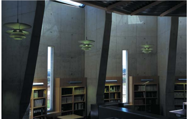
▲ 6.6 FDA Laboratory, Irvine, California, USA, Zimmer Gunsul Frasca Partnership + HDR, 2003. The perimeter wall of the library with its internal buttresses.
