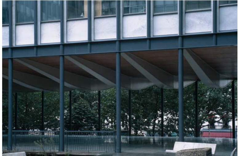
▲ 7.26 Jussieu University, Paris, France, Edouard Albert, 1965. Beam geometry expresses the bending moment diagram.
