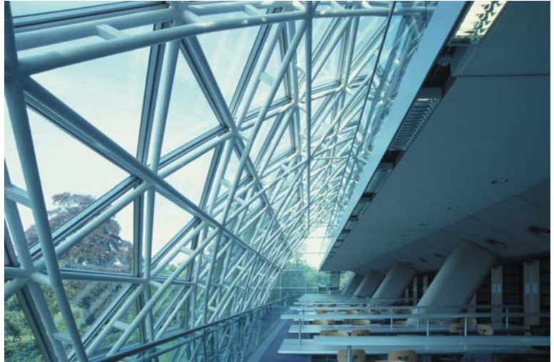
▲ 7.60 Faculty of Law Building, Cambridge, England, Sir Norman Foster and Partners, 1996. The light-weight façade structure contrasts with the concrete columns.
