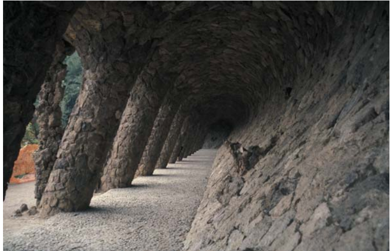
▲ 4.39 Parc Güell, Barcelona, Spain, Antonio Gaudí, 1914. The retaining structure elegantly expresses resistance to the soil pressure acting upon it.
