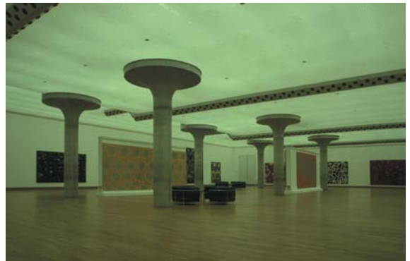
▲ 7.36 Mushroom reinforced concrete columns in a gallery.
