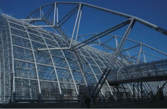
▲ 8.13 Trade Fair Glass Hall, Leipzig, Germany, Ian Ritchie Architects, 1996. Exterior trusses support the vaulted grid-shell.
