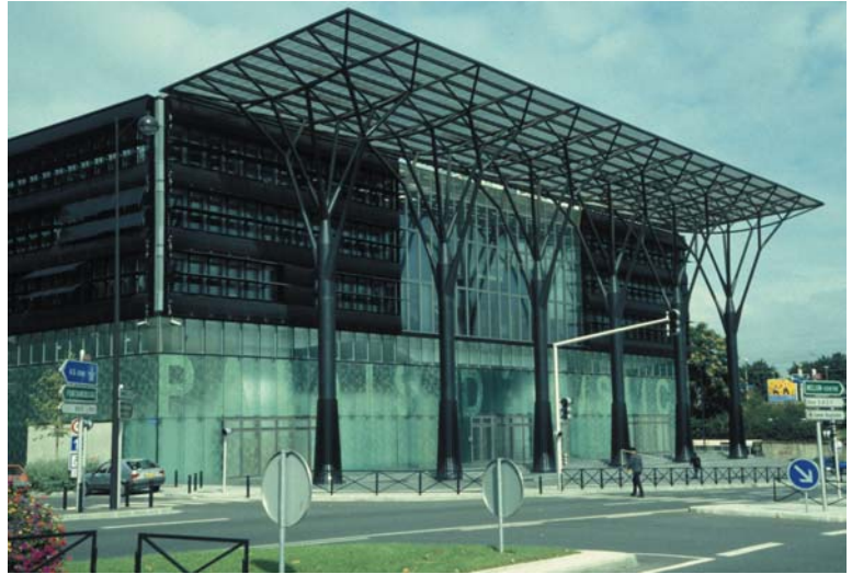
▲ 9.1 Palais de Justice, Melun, France, Jourda & Perraudin architectes, 1998. A tree-supported canopy on the main façade.
