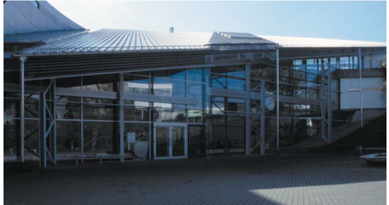
▲ 4.36 Business School, Öhringen, Germany, Gunter Behnisch & Partner, 1993. The main entrance and the haphazardly orientated buttresses.
