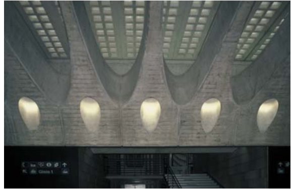
▲ 8.12 Stadelhofen Railway Station, Zürich, Switzerland, Santiago Calatrava, 1990. Integration of structure and artificial lighting.
