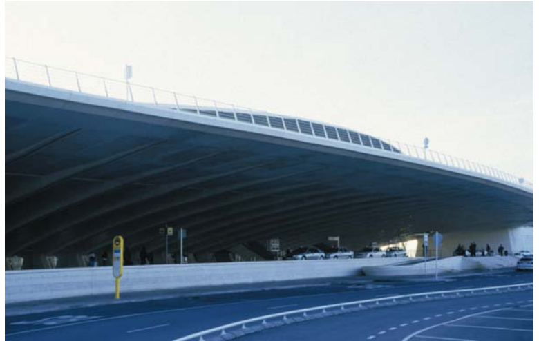
▲ 6.12 Sondica Airport Terminal, Bilbao, Spain, Santiago Calatrava, 2000. Ribs cantilever under the departure level forecourt.
