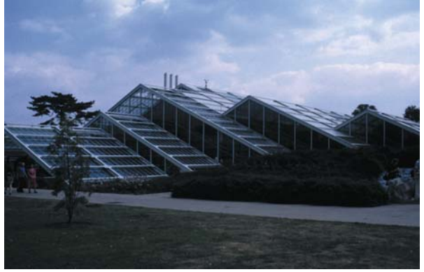
▲ 3.21 Princess of Wales Conservatory, London, England, Gordon Wilson, 1986. Pitched portal frame variations.
