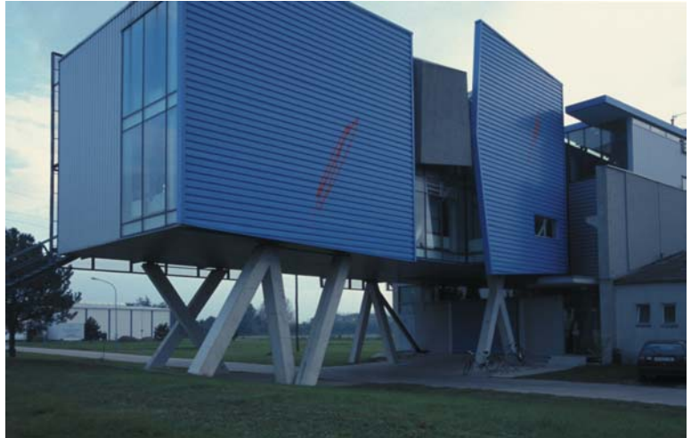
▲ 5.33 Research Centre, Seibersdorf, Austria, Coop Himmelb(1)au, 1995. The office block and its irregular columns.
