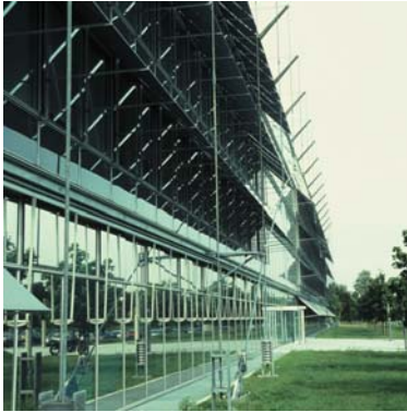
▲ 3.52 Exterior tension rods and springs.
