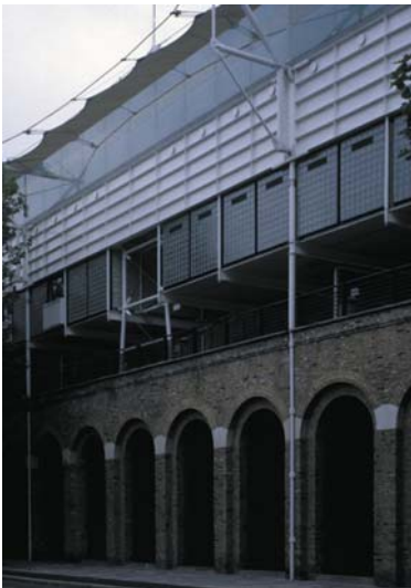
▲ 4.11 Mound Stand, Lord's Cricket Ground, London, England, Michael Hopkins & Partners, 1987. Horizontal and vertical stiffening plates texture a steel beam-wall along the rear of the stand just below the tension-membrane roof.
