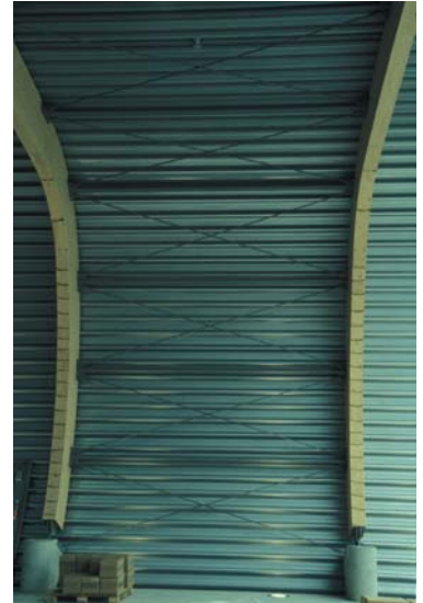
▲ 7.9 Fine diagonal bracing reads as 'stitching'.
