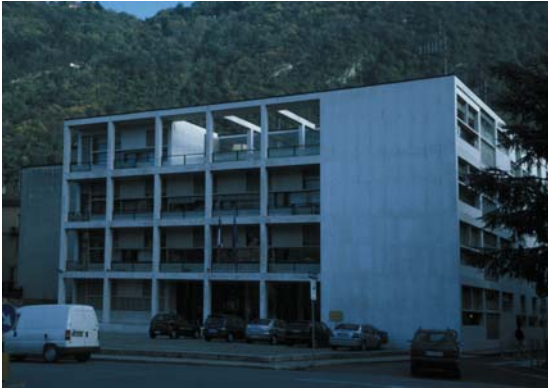
▲ 3.24 Casa del Fascio, Como, Italy, Giuseppe Terragni, 1936. Rational composition of frames and walls.
