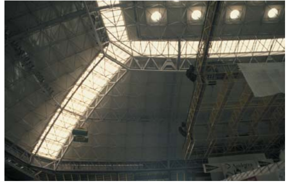
▲ 8.6 Sant Jordi Sports Hall, Barcelona, Spain, Arata Izosaki & Associates, 1990. Light enters through constructional fold-line joints, as in this corner of the roof structure.
