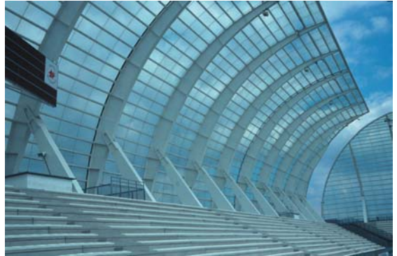
▲ 3.14 Wall ribs, props and longitudinal girders.
