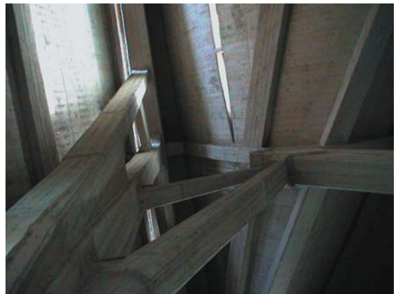
▲ 9.22 Details of the concrete structure.
