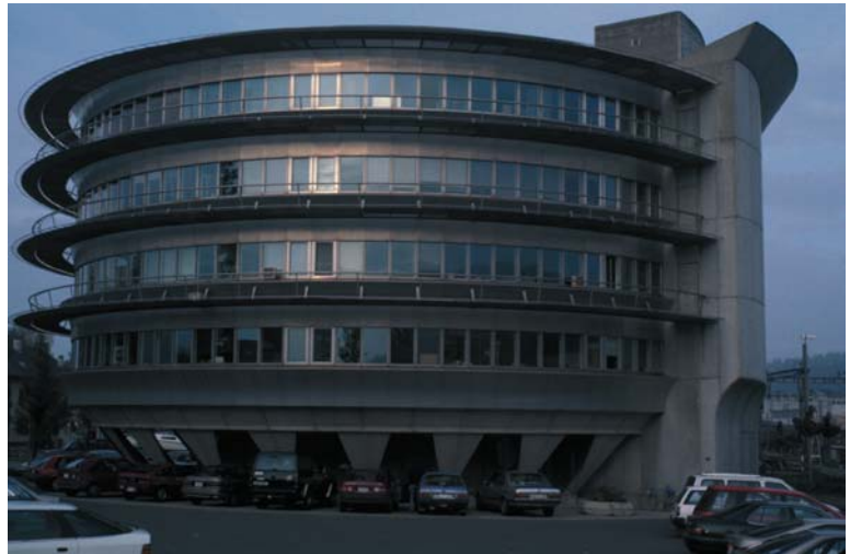
▲ 7.5 Suhr office building, Switzerland, Santiago Calatrava, 1985. The building is circular in plan, with an attached service core behind.
