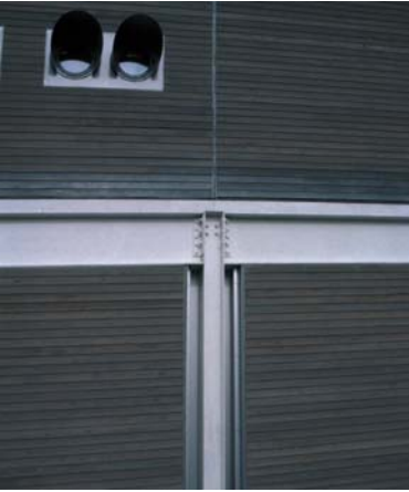
▲ 2.5 Exterior column recessed within an external wall.
