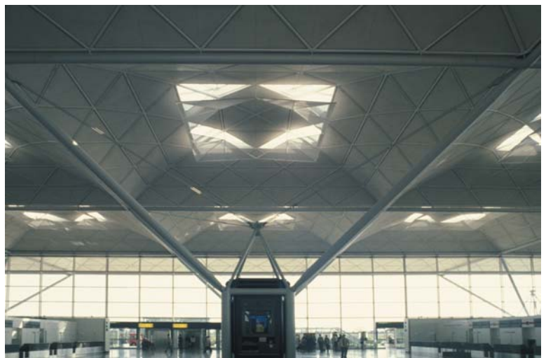
▲ 9.8 Stansted Airport terminal, Essex, England, Foster Associates, 1991. A typical interior structural tree.
