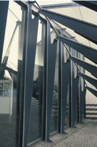
▲ 9.11 Foot-like base-plates to the window mullions behind the canopy.
