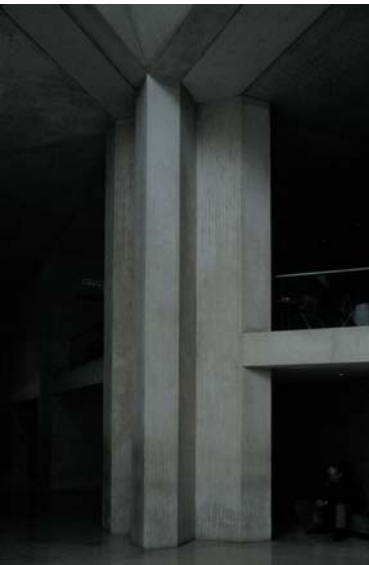
▲ 7.4 Triangular recesses in the central column relate to the pyramid above.
