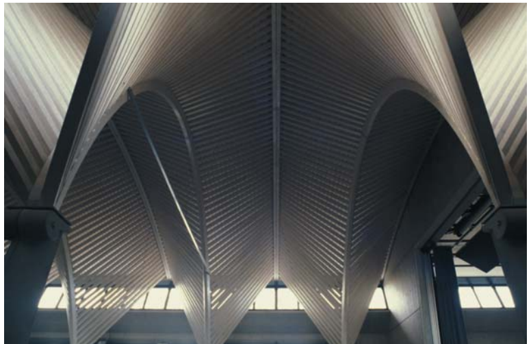
▲ 6.19 Looking across the hall.
