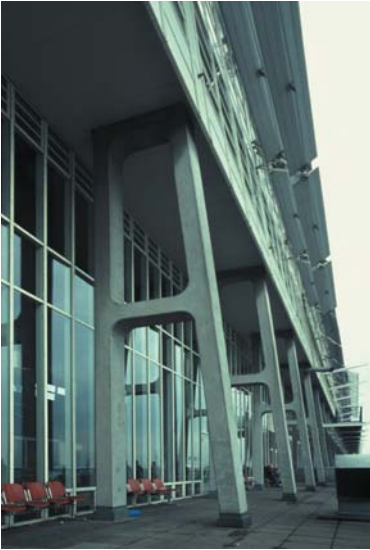
▲ 7.17 Ferry Terminal and office building, Hamburg, Germany, Alsop and Störmer, 1993. Partially exposed precast concrete A-frames.
