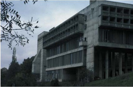
▲ 5.35 Convent of La Tourette, Eveux, France, Le Courbusier, 1959. The western façade and three levels of irregularly-spaced mullions.
