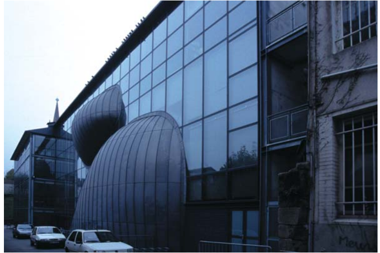
▲ 6.40 Law Faculty Extension, Limoges, France, Massimiliano Fuksas, 1997. Walls of the interior lecture theatres protrude from the exterior wall.
