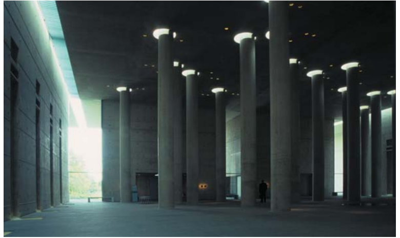
▲ 2.15 Light-slot between the side wall and the roof slab.
