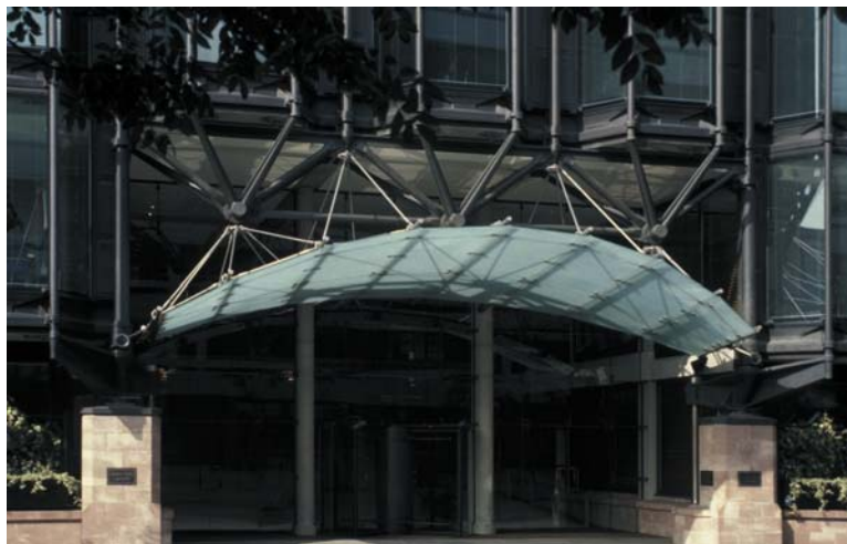
▲ 7.39 Bracken House, London, England, Michael Hopkins and Partners, 1991. Main entrance canopy.
