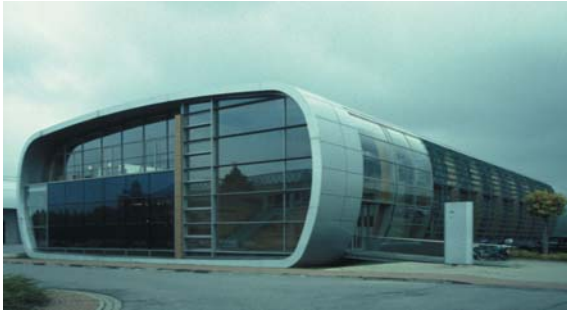
▲ 3.30 Tobias Grau headquarters, Rellingen, Germany, BRT Architekten, 1998. Glue-laminated ribs enclose the ground floor interior concrete structure.
