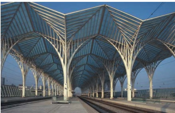
▲ 9.4 A view along the canopy structure.
