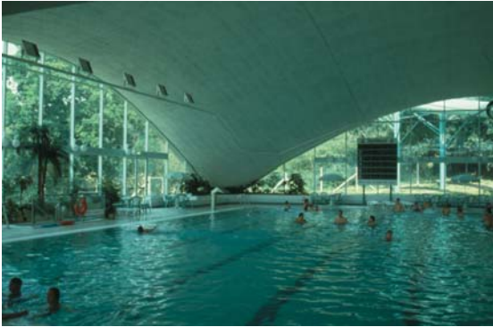
▲ 3.2 Interior of a concrete shell structure. (Courtesy J. Chilton)
