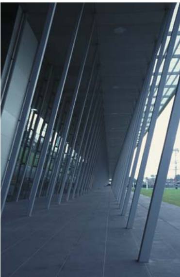
▲ 4.14 A view along the verandah.
