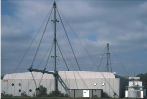
▲ 5.2 Oxford Ice Rink, England, Nicholas Grimshaw & Partners, 1985. Exterior masts and projecting horizontal spine beam.
