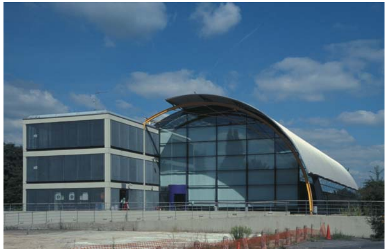
▲ 7.58 Learning Resource Centre, Thames Valley University, Slough, England, Richard Rogers Partnership, 1996. The two exterior forms.
