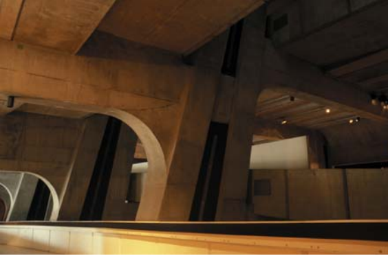
▲ 6.30 Museum of Gallo-Roman Civilization, Lyons France, Bernard Zehruss, 1975. A central row of continuous and sloping columns.
