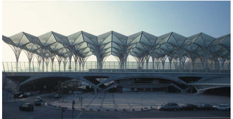
▲ 9.3 Oriente Station, Lisbon, Portugal, Santiago Calatrava, 1996. A light-weight platform canopy atop a heavy base.
