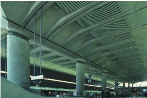
▲ 5.30 Canary Wharf Underground Station, London, England, Foster and Partners, 1999. The ticket hall with its central columns and spine beam.
