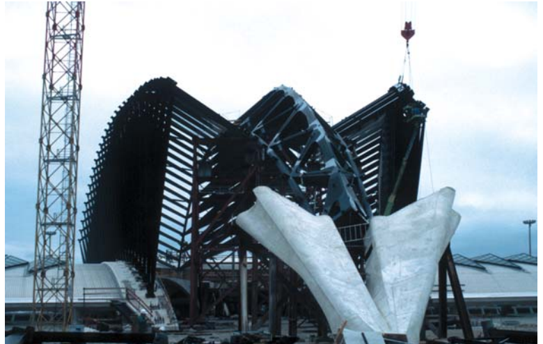
▲ 9.12 Terminal building, Railway Station at Satolas Airport, Lyons, France, Santiago Calatrava, 1994. The central arched-spine and its supporting buttresses (during construction).
