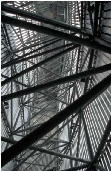
▲ 9.26 Imperial War Museum-North, Manchester, England, Studio Daniel Libeskind, 2002. Structural members dominate the Air Shard volume.
