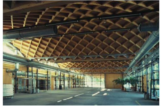
▲ 6.9 Building Industry School, Hamm, Germany, Heger Heger Schlieff, 1996. Lamella timber vaults span the workshop.
