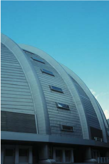
▲ 4.6 Ludwig Erhard House, Berlin, Germany, Nicholas Grimshaw & Partners, 1998. Arched ribs modulate the rear surfaces of the building.
