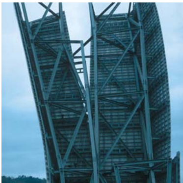
▲ 7.20 The tower structure.
