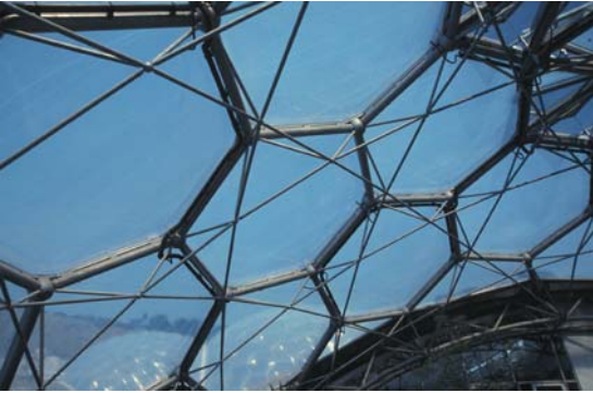
▲ 3.6 Biome interior structure consisting of outer primary hexagons and an inner layer of braced rods.
