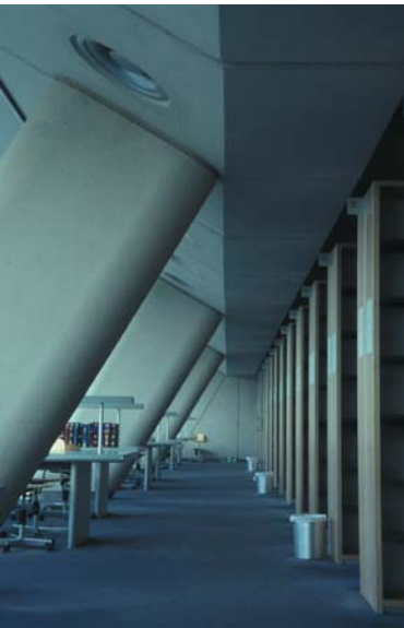
▲ 7.61 Raking concrete columns with a 'softening' sand-blasted finish.
