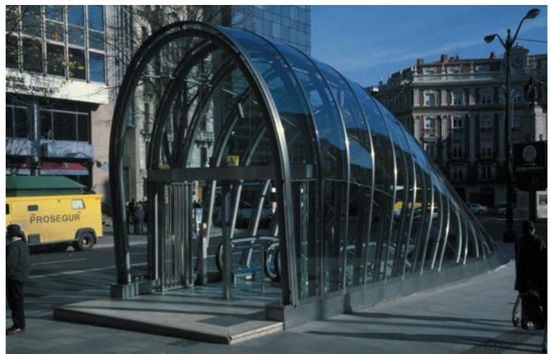
▲ 5.29 Bilbao Metro, Bilbao, Spain, Foster and Partners, 1996. Rounded frames express movement to and from an underground station.
