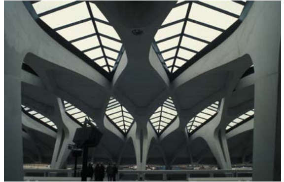
▲ 8.10 A view across the concourse. Glazed areas are integrated with the pattern of ribs.
