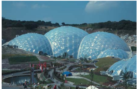
▲ 3.5 Eden Project, Cornwall, England, Nicholas Grimshaw & Partners, 2001. A cluster of interlinked biomes.
