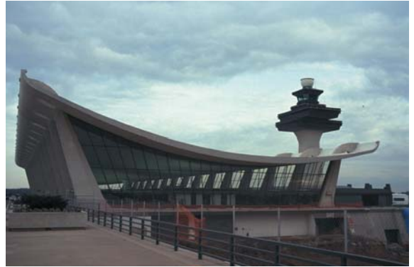
▲ 3.10 Dulles International Airport, Washington, DC, USA, Saarinen (Eero) and Associates, 1962. Inclined piers support the catenary slab.
