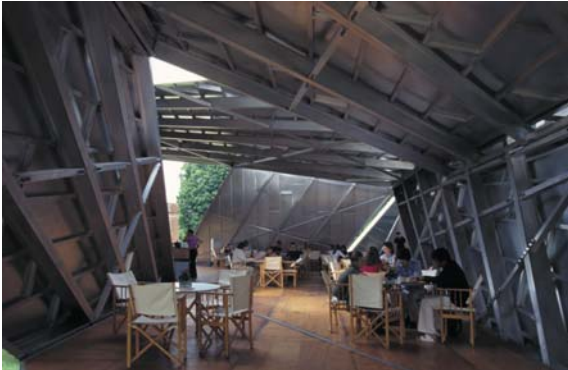
▲ 3.37 Interior ribbed surfaces.
