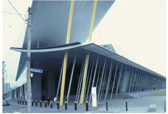
▲ 4.13 Exhibition Centre, Melbourne, Australia, Denton Corker Marshall, 1996. Verandah posts visually soften the façade.
