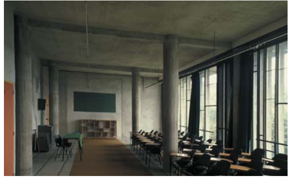
▲ 5.36 Two columns on the right are set-in from the exterior wall and intrude upon a teaching space.
