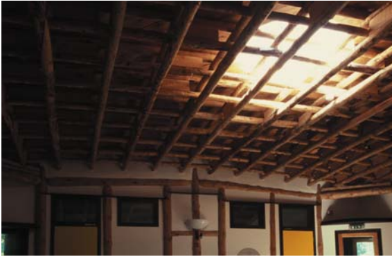
▲ 6.8 Westminster Lodge, Hooke Park, Dorset, England, Edward Cullinan Architects, 1996. A grillage of roundwood beams spans the main space.
