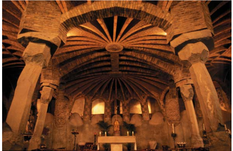
▲ 6.7 Güell Colony Crypt, Barcelona, Spain, Antonio Gaudí, 1917. Columns support an inner arcade ring and the textured ceiling above.
