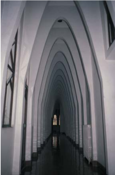
▲ 5.27 Colegio Teresiano, Barcelona, Spain, Antonio Gaudí, 1889. The first floor arched corridor.
