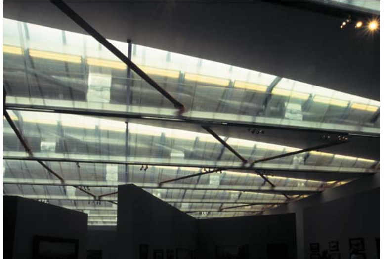
▲ 6.36 Unusually configured roof-plane bracing.
