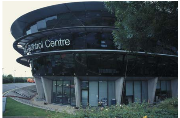
▲ 4.5 RAC Control Centre, Bristol, England, Nicholas Grimshaw & Partners, 1995. Structural piers modulate the base perimeter.
