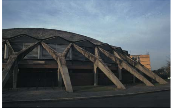
▲ 3.3 Palazzetto dello Sport, Rome, Italy, Pier Luigi Nervi with A Vitellozzi, 1957. Inclined struts support the shell roof.
