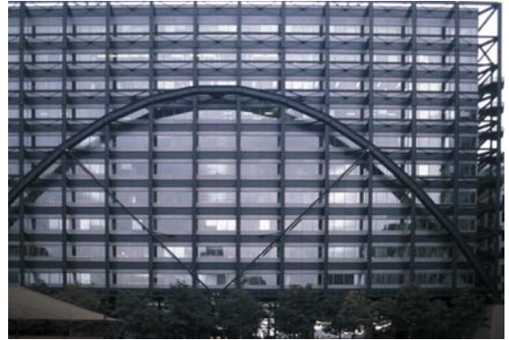
▲ 3.40 Exchange House, London, England, Skidmore, Owings & Merrill, 1993. Arches enable the building to span the site.
