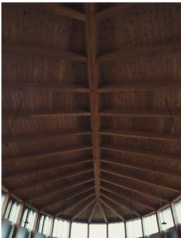
▲ 6.5 Ribbed roof structure.
