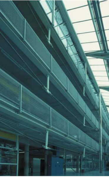
▲ 8.17 School at Waidhausenstraße, Vienna, Austria, Helmut Richter, 1995. Composite steel walkway beams.
