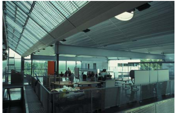
▲ 7.45 Unrefined steel beams pass over a work-space atop the lecture block inserted into the atrium.
