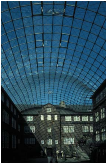
▲ 7.68 Hamburg Museum Courtyard Canopy, Hamburg, Germany, Von Gerkan, Marg and Partner, 1989. General view of the canopy.
