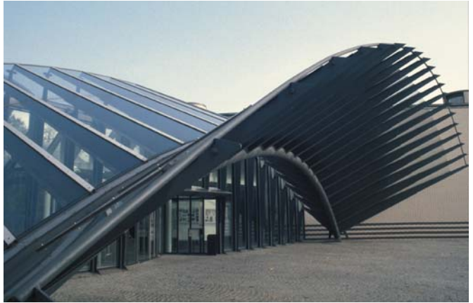
▲ 9.10 Wohlen High School entry canopy, Switzerland, Santiago Calatrava, 1988. Ribs cantilever from the main arch.
