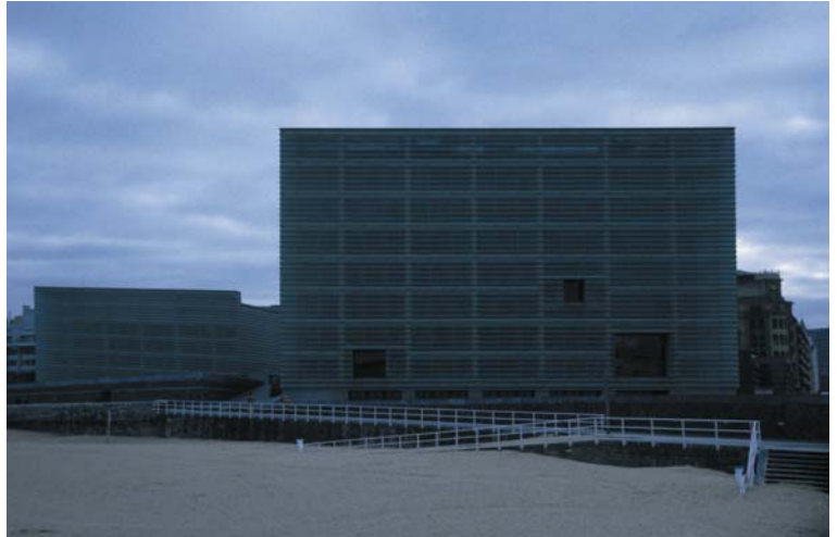
▲ 4.2 Kursaal Auditorium and Conference Centre, San Sebastian, Spain, Rafael Moneo, 1999. Structure behind translucent glazed panels modulates exterior walls.
