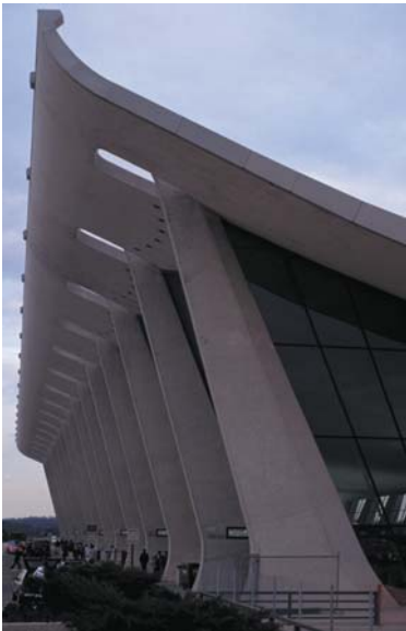
▲ 4.9 Dulles International Airport, Washington, DC, USA, Saarinen (Eero) and Associates, 1962. Piers create deep bays along the façade.
