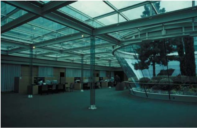
▲ 8.24 Town Administrative Centre, Saint-Germain-en-Laye, Paris, France, Brunet and Saunier, 1995. Glass columns support roof beams.
