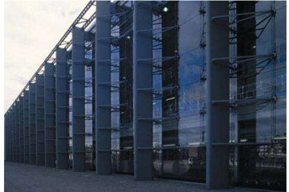
▲ 5.3 Financial Times printing works, London, England, Nicholas Grimshaw & Partners, 1988. Exterior columns along the main façade.
