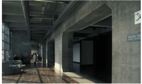
▲ 3.19 An interior vierendeel truss to the right.
