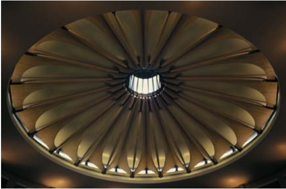
▲ 6.1 Entrance foyer roof, Wohlen High School, Switzerland, Santiago Calatrava, 1988. Attractive structural roof framing pattern.
