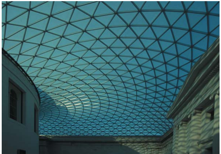
▲ 3.55 The Great Court, British Museum, London, England, Foster and Partners, 2000. Triangulated lattice roof with the circular Reading Room on the left.
