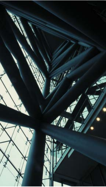
▲ 6.24 A view up through a tower.
