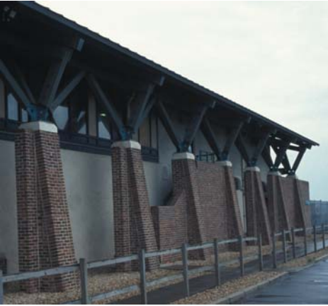
▲ 9.9 Outdoor Activities Centre, Portsmouth, England, Hampshire County Architects, 1995. Where the building is approached from the car park in the background, the partial or full disappearance of the wall panels suggests a process like erosion.
