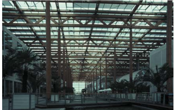
▲ 3.27 Interior timber structure.
