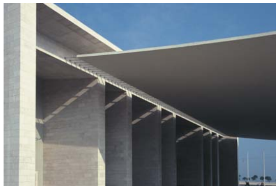
▲ 8.8 Portuguese Pavilion, Lisbon, Portugal, Alvaro Siza, 1998. Light passes through the slit in the concrete slab and between the stainless-steel tendons.
