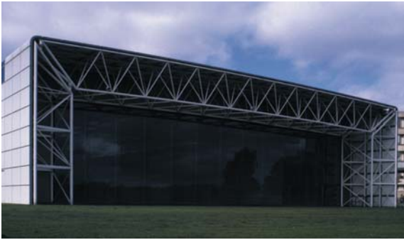
▲ 5.7 Sainsbury Centre for Visual Arts, Norwich, England, Foster Associates, 1977. The vertical wall structure that is visible on the end elevations houses support functions.
