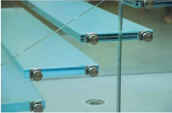
▲ 8.27 Stair treads connect to the glass wall.
