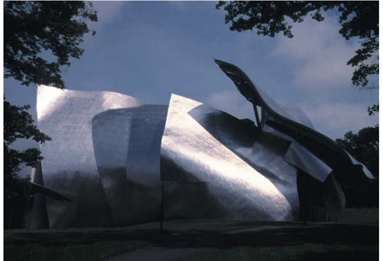
▲ 7.21 Fisher Center, Bard College, Annadale-on-Hudson, New York, USA, Frank O. Gehry & Associates, 2002. Side elevation with the main entry canopy to the right.
