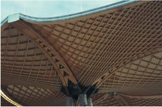
▲ 4.12 Canopy structure, World Exhibition Centre, Hanover, Germany, Herzog + Partner, 1999. Attractive textured soffit surfaces.
