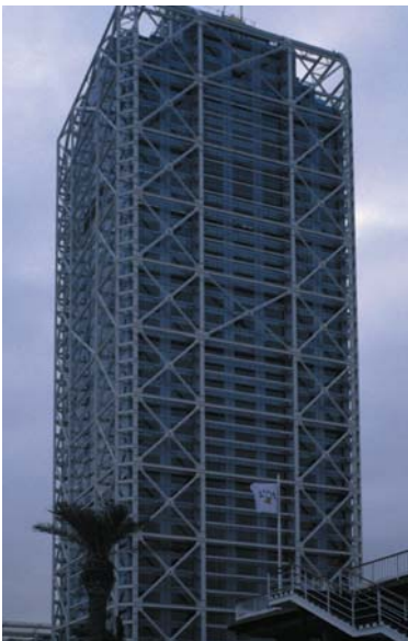
▲ 4.22 Hotel de las Artes, Barcelona, Spain, Skidmore Owings & Merrill, 1992. Structural bracing appears frail in relation to the building elements behind.
