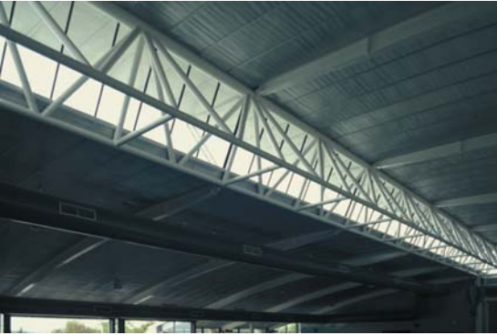
▲ 8.5 Kew Swimming and Recreation Centre, Melbourne, Australia, Daryl Jackson Architects, 1990. Light penetrates the truss that defines the step in the roof.
