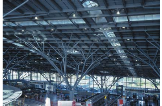
▲ 3.43 Stuttgart Airport Terminal, Germany, von Gerkan • Marg + Partner, 1991. Structural 'trees'.
