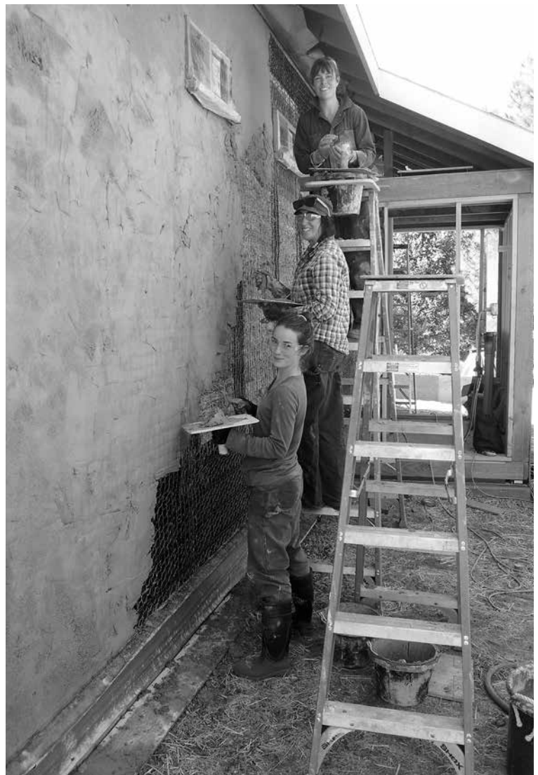
6-22. Plaster crew working a diagonal.
