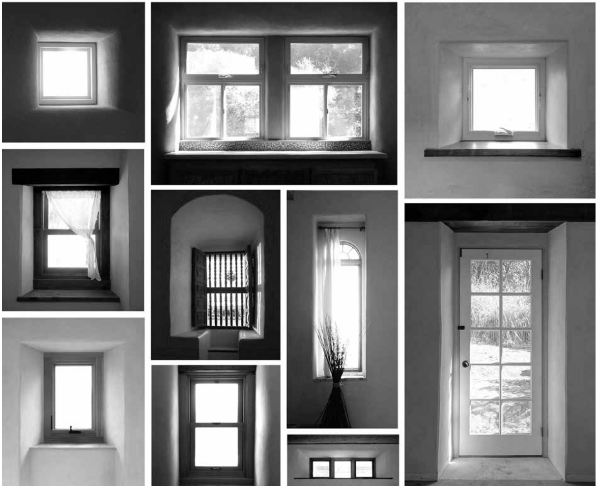
6-2. Plastered returns around doors and windows.
