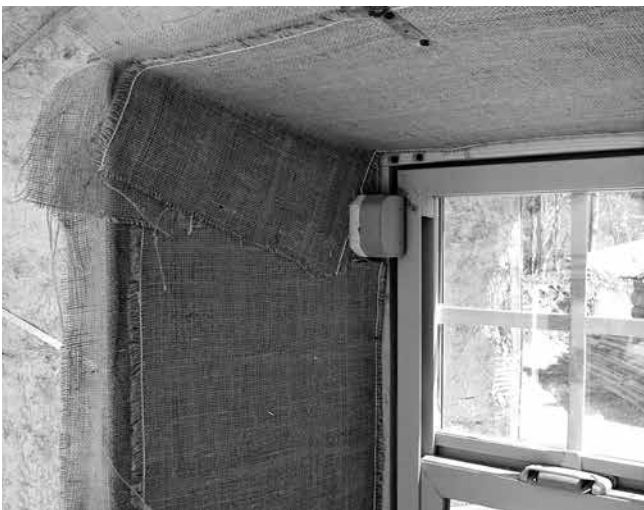
6-19. Installing bio-lath dry and wet.
