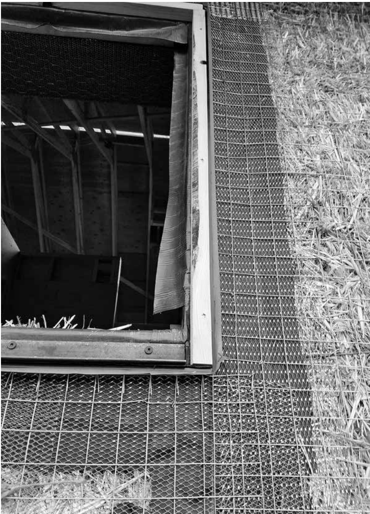
6-16. Expanded metal lath reinforcing window corner.
