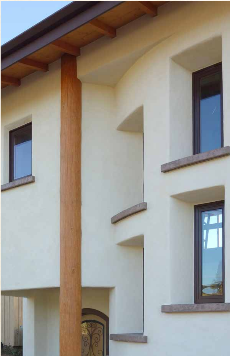
Exterior window and door openings in the wall require well designed and executed details to prevent water intrusion and keep bales dry.
