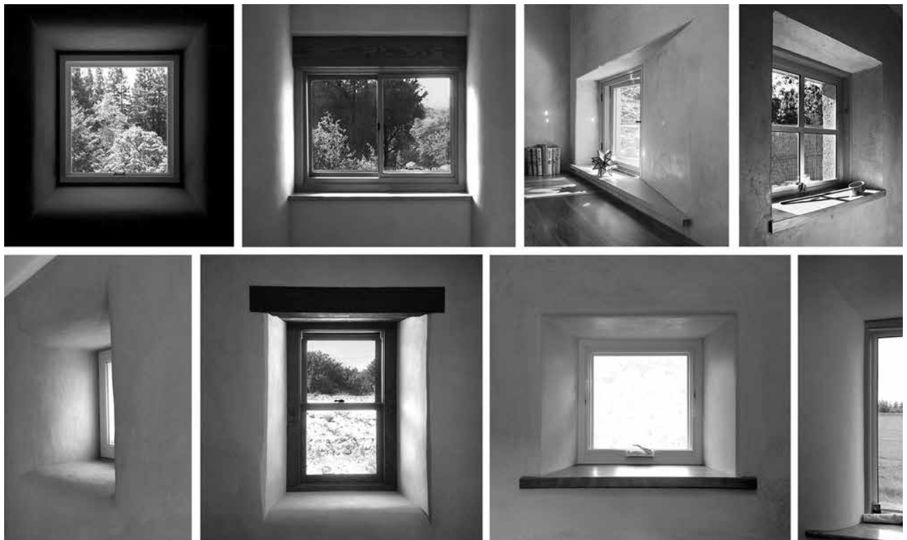
2-13. Shape of window reveal and effects on light.
