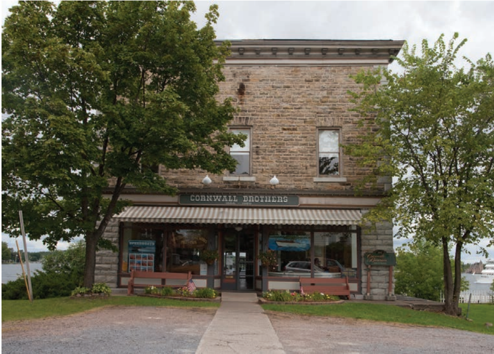
13.3. The Market Street façade of the Cornwall Brothers Store became popular when tourists flocked to nearby hotels in the late 1800s.
