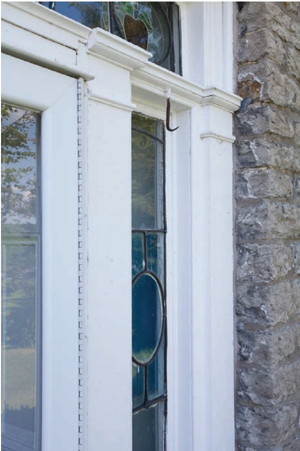
5.2. At the entrance to the Salisbury House, a forged hook hangs above a side light.
