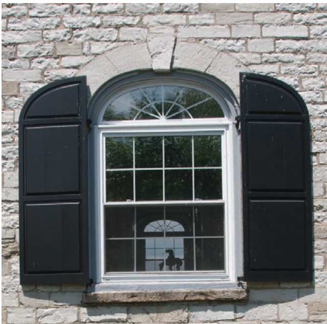
10.3. Stone House: detail of the window with an elliptical arch and fan light.
