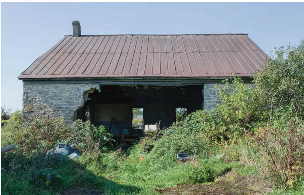
18.1. School House No. 3, Evans Road, Town of Hounsfield. View from the side, where collapsed stone and windows allow entrance for farm vehicles.
