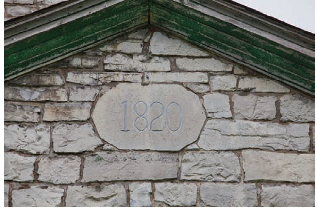
17.18. Date stone in the side gable of the Samuel Cronkhite House, 1820.
