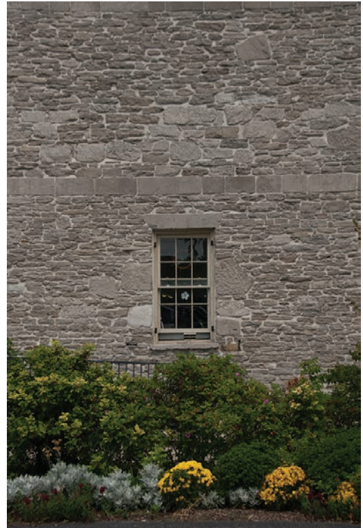
7.4. Union Hotel: the southwest wall of rubble with an ashlar belt course and a splayed lintel over the window. Many of these stones are weather-smoothed and are probably from a nearby shore.
