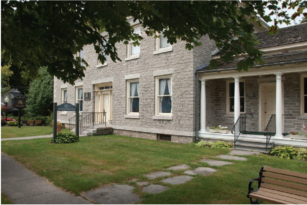
7.19. The conchoidal stone on this side wall of the Sackets Harbor Bank is similar to that used on Christ Episcopal Church, a couple of blocks away. The rear ell holds the offices of the Sackets Harbor Historical Society, which was instrumental in saving the building.
