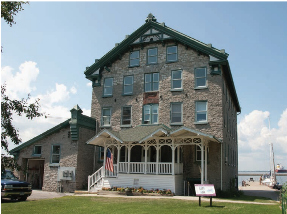
10.8. Duvillard Mill, US Bureau of Fisheries, 1856. Designed by John Antoine Duvillard, built by Ignatius Wiley. The mill was run by steam power from the small building on the south wall, which until recently had a large chimney.
