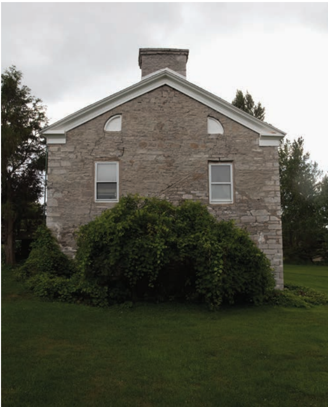
9.11. The gable ends of the Ryder House feature small attic windows that are now closed, and broad stone chimneys.
