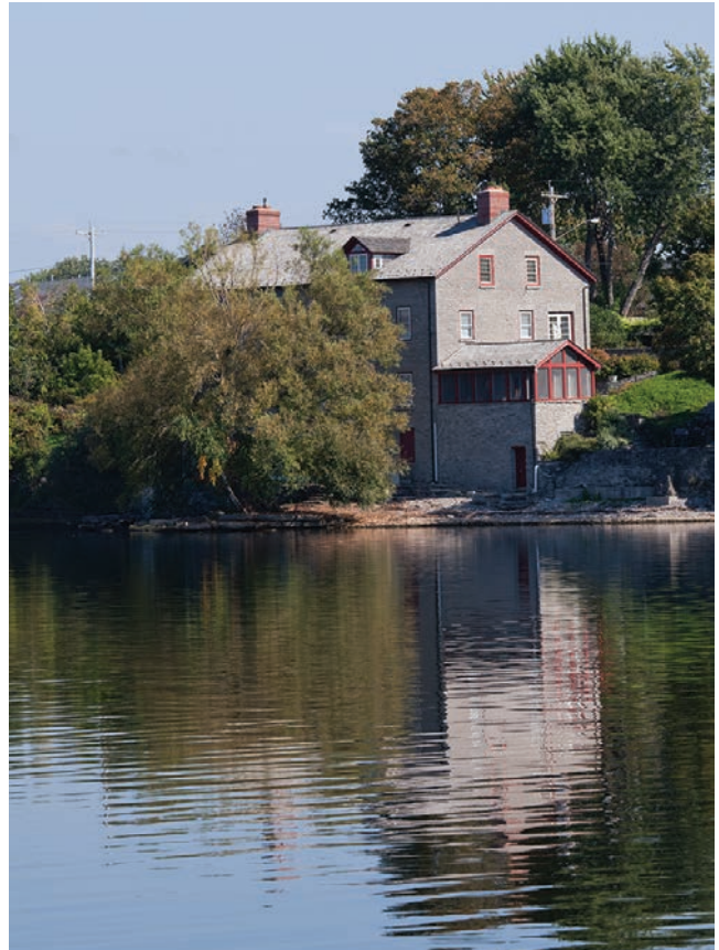
7.15. The Old Mill, 1808–1818, has walls at the base that measure five feet thick. It was built by an industrious early settler, Elisha Camp, who promoted Sackets Harbor as a commercial center.
