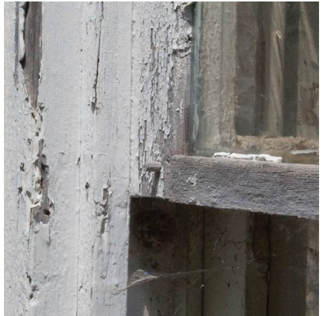
17.16. Detail of a window with a wooden peg in the Harger Mansion.
