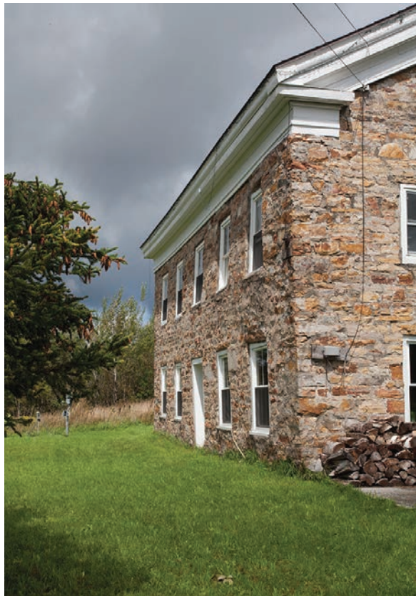
14.4. The even front façade of the Ostrander House has a wide cornice and return. Its walls seem to be emerging from the ground.
