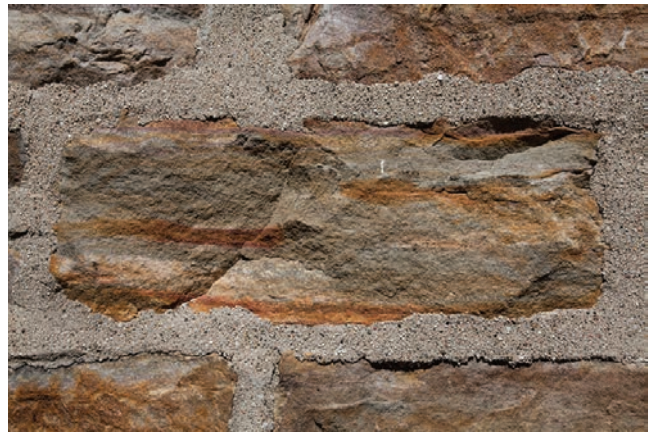
15.6. Detail of the sandstone in the Ira Hinsdale House.
