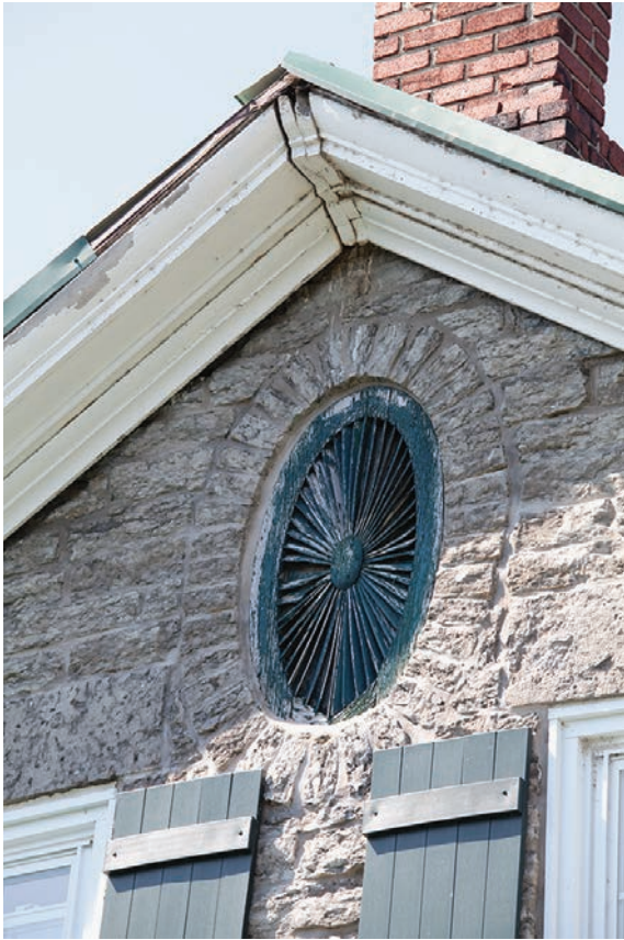
5.3. Each gable end of the Salisbury House features an elliptical fan surrounded by stone voussoirs.
