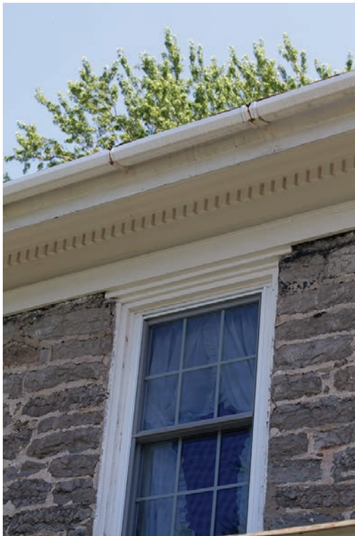
6.9. The cornice of the Dobson House has delicate dentil molding.
