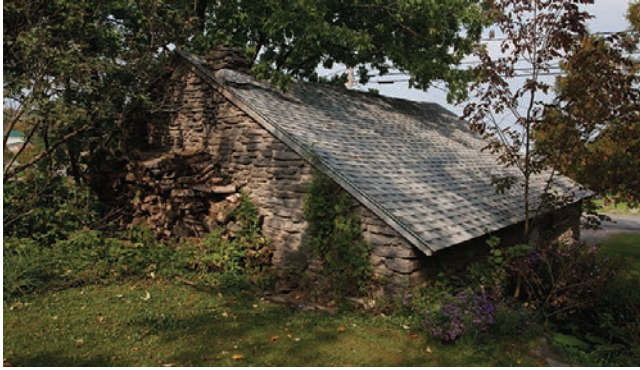
1.15. Stone barn near the Asa Gates House.
