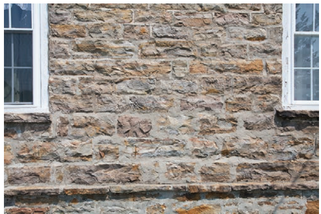
14.8. Detail of the careful stone work of the Harry Hunt House with its water table.
