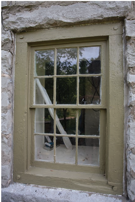
17.13. The original pegged window on the rear of the Harger House.
