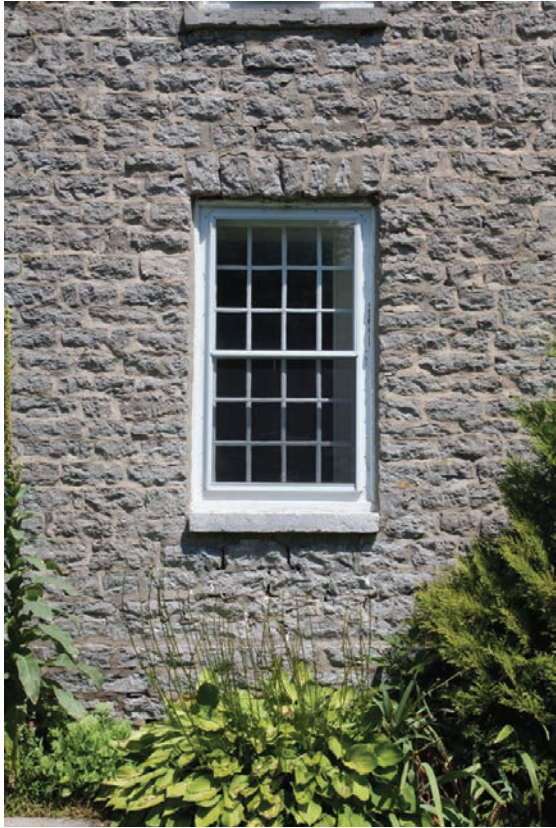
3.8. John Thompson House: a side wall of rubble stone with an 8/8 window over the smooth stone sill.
