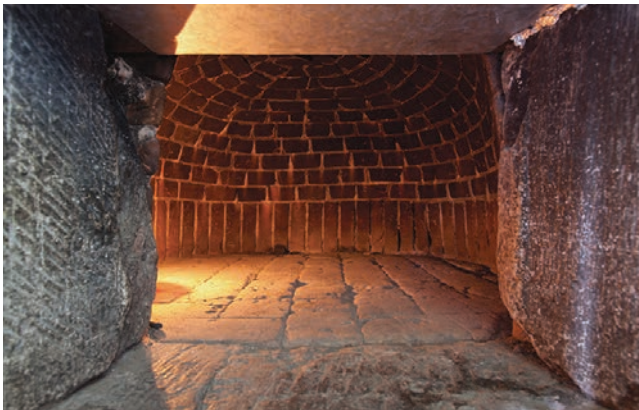
1.7. Interior of the brick beehive oven in the Noadiah Hubbard House.
