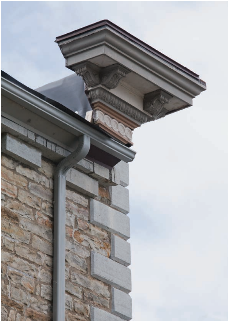
13.6. The Cornwall Brothers Store: detail of the cornice and limestone quoins, reputedly from Kingston, Ontario.
