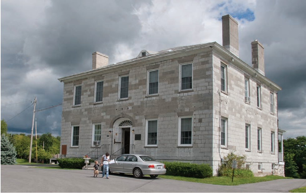
8.2. General Jacob Brown Mansion, 1811–15. Built of large blocks of limestone quarried nearby, the grand square mansion was noted for the cords of wood needed to keep its many fireplaces going. Once the proud home of the founder of Brownville, it has been the site of military meetings and political gatherings. Today it remains a proud focal point for the community.
