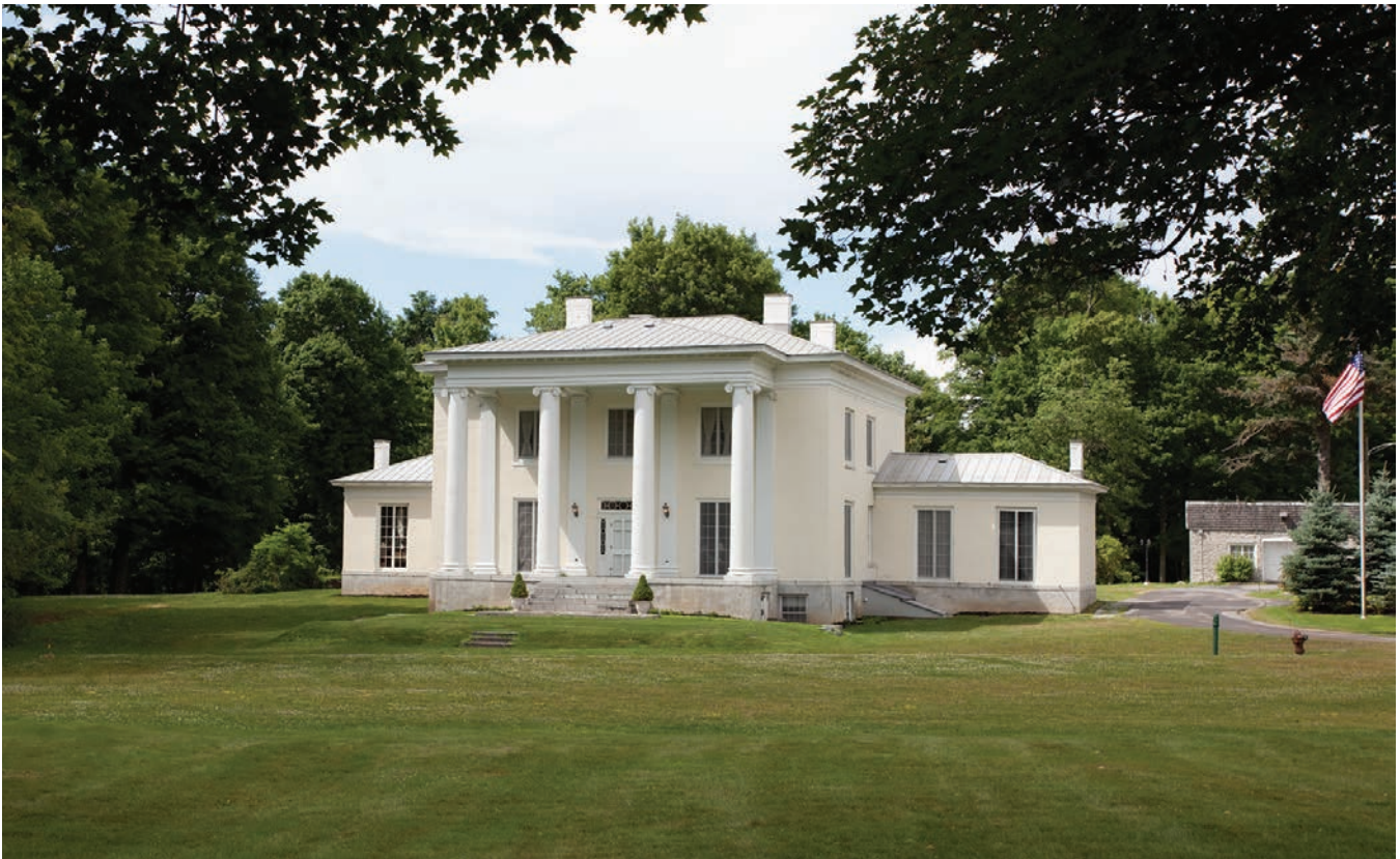
16.2. The south elevation of the LeRay Mansion was originally reached by a long drive with a bridge that crossed a stream.
