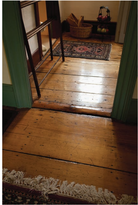
3.12. The Ballard, Denny House has floorboards with some planks nineteen inches in width.
