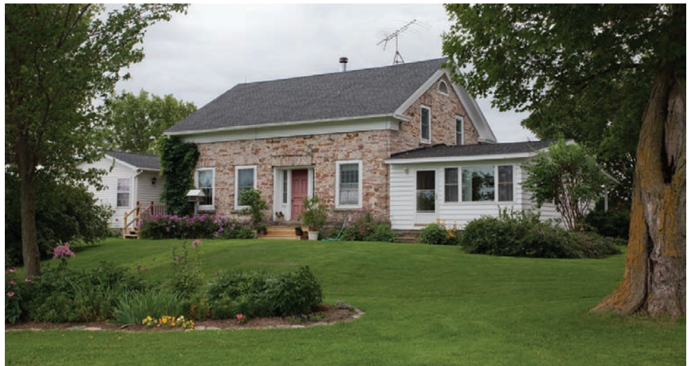
13.8. The Asa Newman House, 1826–27. The front façade has four bays with an off-center doorway. All openings are topped with voussoirs.
