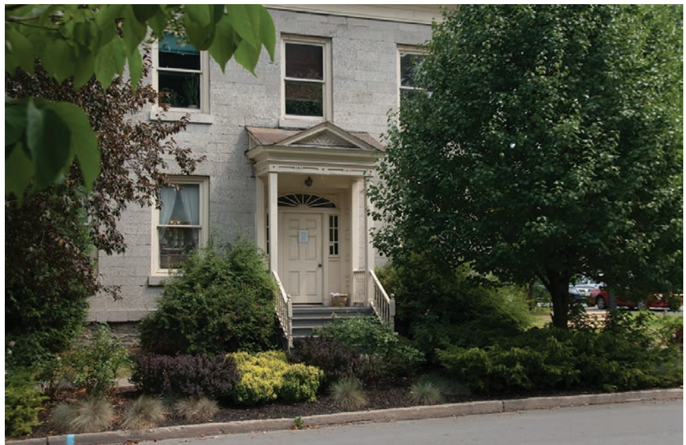
7.18. Sackets Harbor Bank, 1834. The beautifully cut ashlar limestone makes for an impressive front façade on West Main Street.
