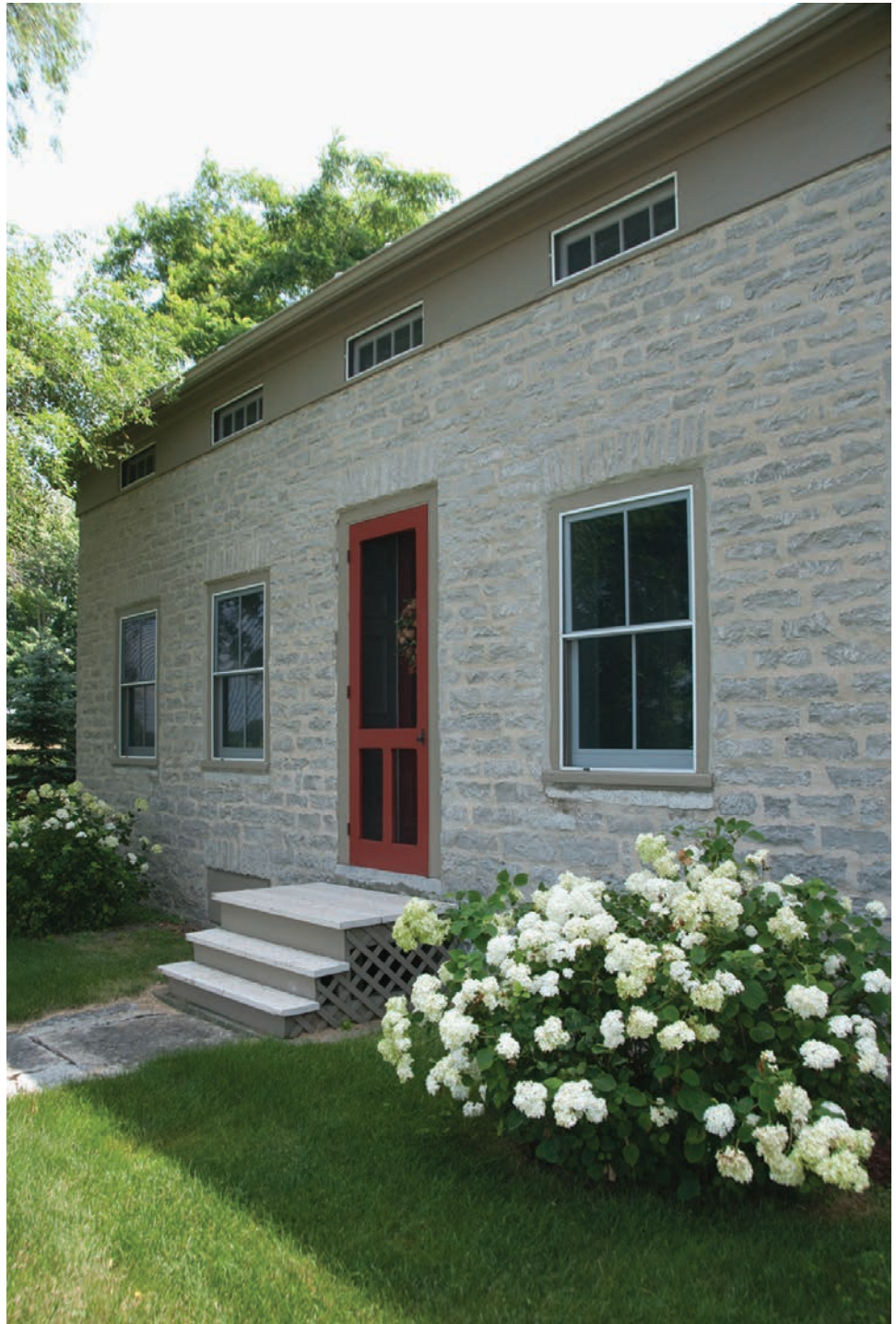
10.21. The George Cough Jr. House, c. 1835, is noted for its eyebrow windows, which provide a view of Wilson Bay from the second floor of the house.
