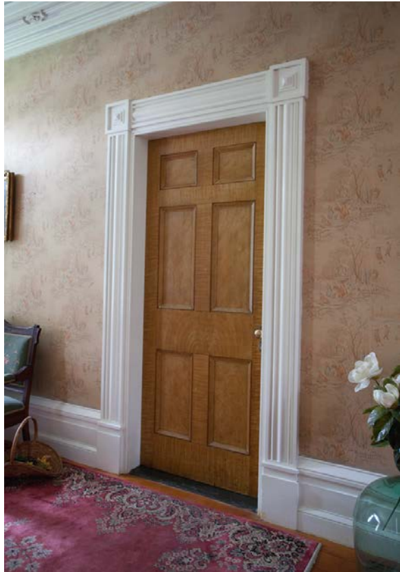
2.8. Felt Mansion: interior painted faux-wood door.
