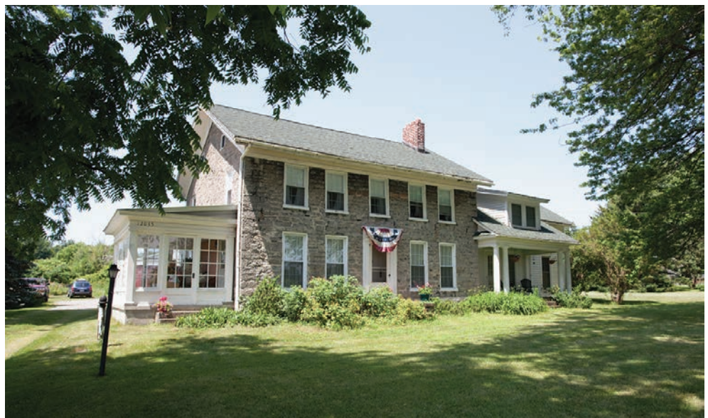
6.8. The Dobson House was built around 1820 by a Welsh-born stonemason, on the old road leading to Henderson Harbor.
