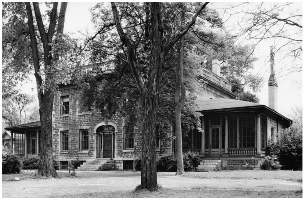
3.5. Sterling Mansion, by David F. Lane for the Watertown Daily Times . In this early photograph, Sterling’s imposing stone building shows off its stonework and wooden balustrade.
