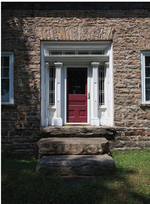
14.7. The entrance to the Harry Hunt House is broad and flanked by transom and sidelights.
