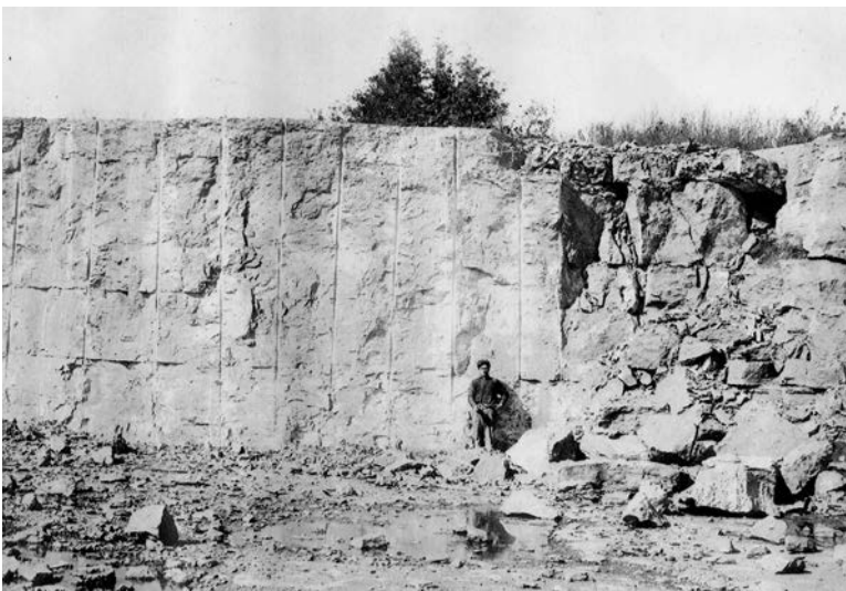
19.9. Saw Mill Bay limestone quarry near Chaumont (no date), showing the depth already cut. There is another eight to ten inches of stone still to be cut before reaching the water level. The Heritage of Chaumont 1874–1974 . Courtesy of Lyme Heritage Center, Three Mile Bay, NY.
