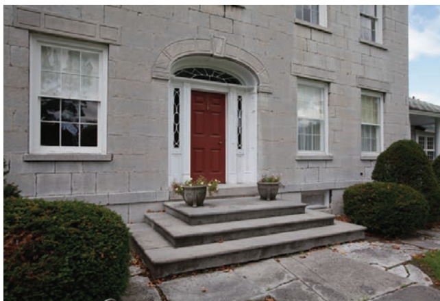
2.4. Felt Mansion entrance with carved marble lintels and sills. The steps are large blocks of limestone, gently curved at the edges.
