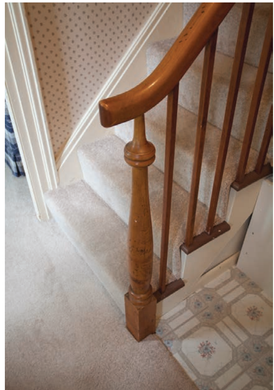
13.10. The Asa Newman House has its original interior stairway, with its comfortable railing and flaring newel.
