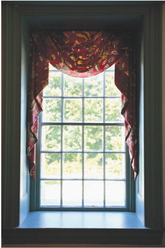
3.13. Ballard, Denny House. This original 12/12 pane window sits within its deep paneled well.
