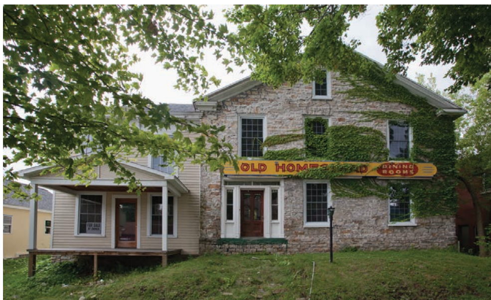
13.1. The Azariah Walton House, 1835, was built when the port of Alexandria Bay was young. Its gable front with 9/9 windows faces onto busy James Street.
