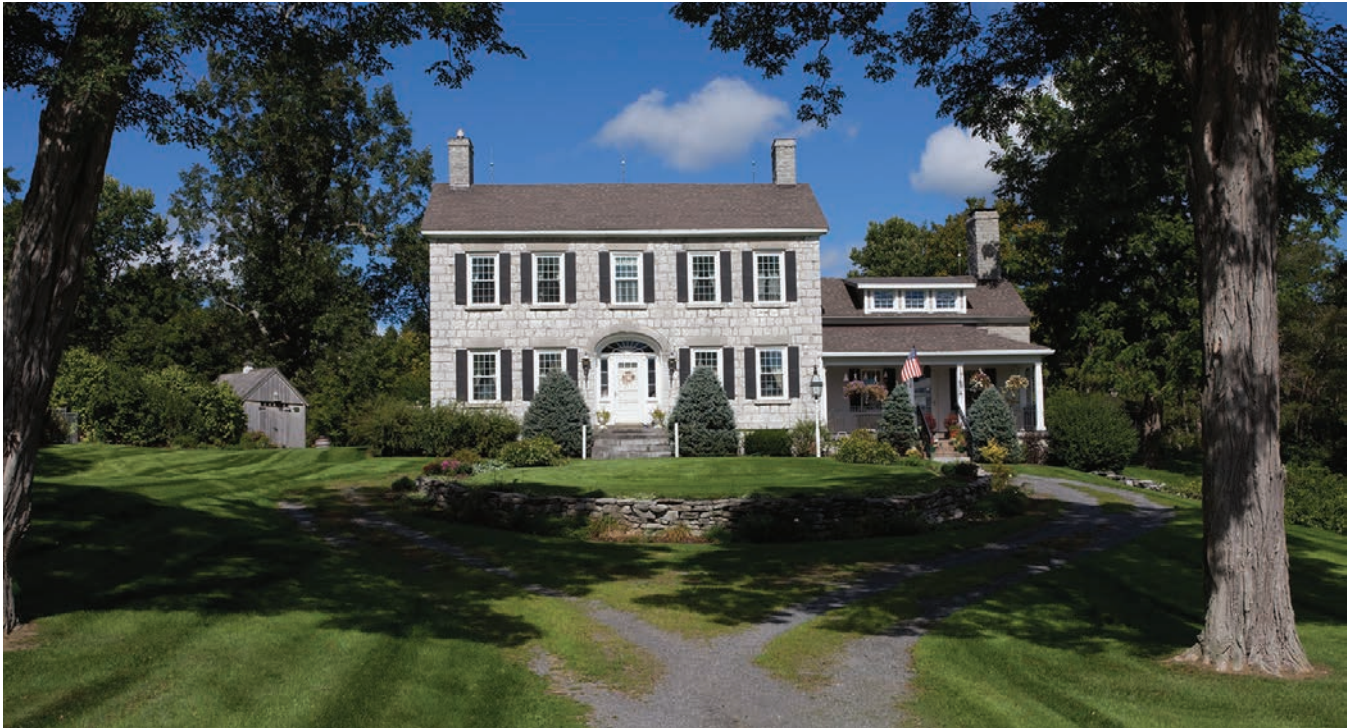
8.4. Henry Brown Mansion, 1830. This mansion has a wonderful symmetry in its five-bay façade. The stone work is especially fine and uses large blocks of local limestone in contrasting shades of gray.
