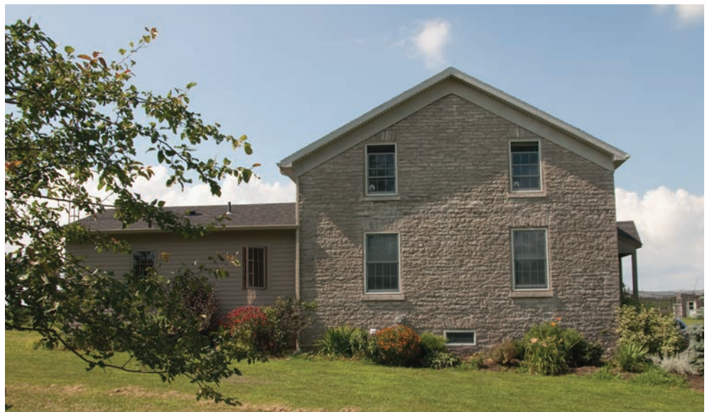
10.10. Wiley House, c. 1847, built by stonemason Ignatius Wiley with stone cut from the bed of the Kent Creek, which flowed nearby.
