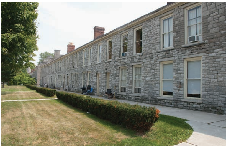
7.8. Stone Row, officers' quarters, 1816–19. Except for the two end houses on the sally port, this row was originally one story high, with an attic that was a continuous open space. The stone is well cut and varies in type over the length of the row. This is probably due to fire, abandonment, and rebuilding in the late twentieth century.
