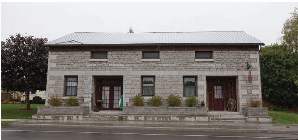
9.17. Old Stone Shop, Three Mile Bay, 1838. Closely resembling the stone work in the Charles Wilcox House, the shop has a running entablature of smooth faced stone across the front of the building and quoins at the corners and around the wide door openings. It is noted as a building well designed for two blacksmiths.
