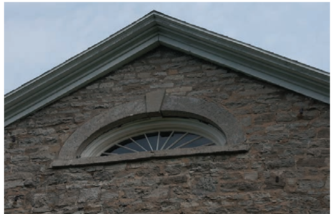
7.22. Each gable end of the Tisdale Mansion has a fan window surrounded by an elliptical stone arch with keystone.
