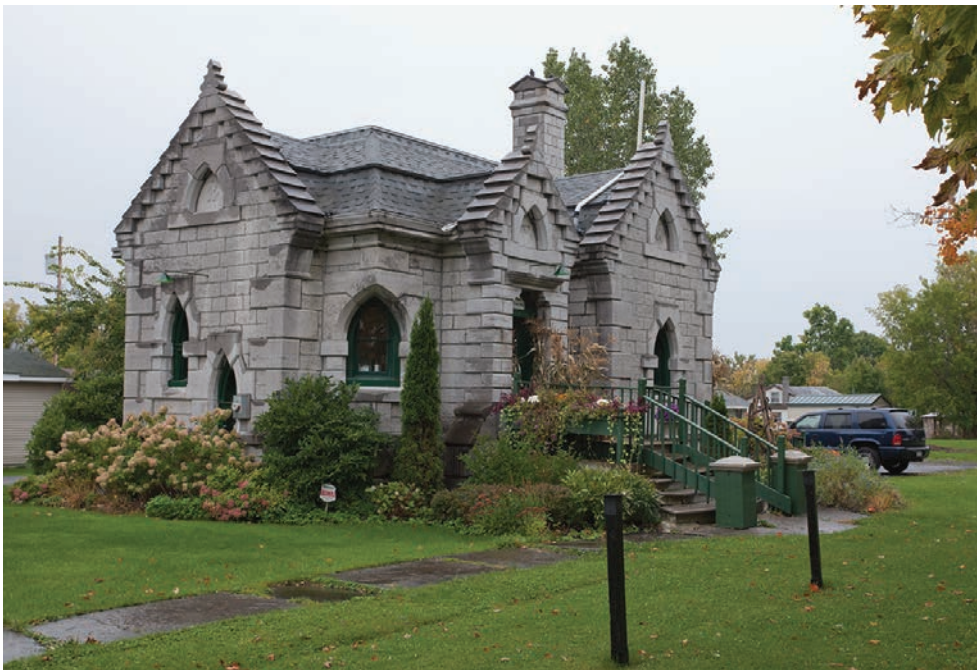
9.5. The Copley, Adams, Duford Stone Office, 1872, is a remarkable structure that displays a range of limestone techniques and finishes. It was the sales office first for the Copley lumber and lime business and later for a local quarrying company.
