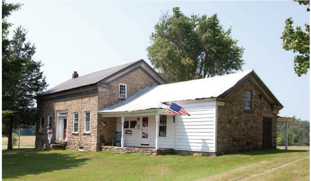
14.6. The Harry Hunt House, 1830s. This house is one of several vernacular farm houses in the area. The stone work in both the house and side ell is very evenly laid.
