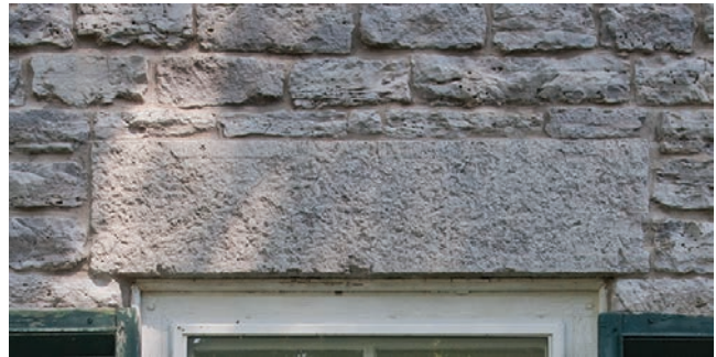
I.11. Lintel on a window of the Charles Wilson House, Three Mile Bay, Lyme Township.
