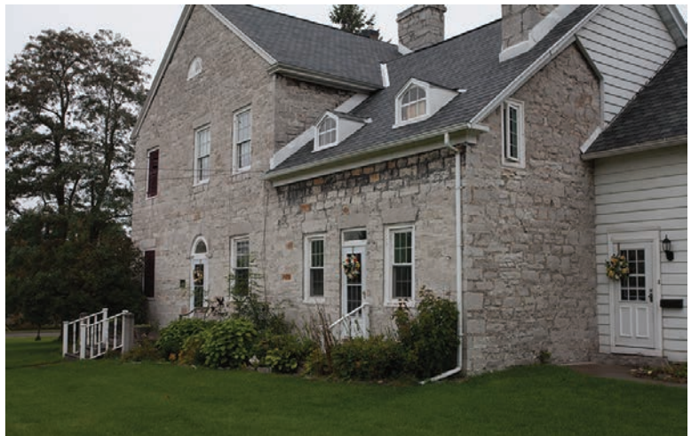
9.4. Evans, Gaige, Dillenback House. This side view shows the the rear ell, which was actually an earlier separate small house containing a kitchen with a stone fireplace.
