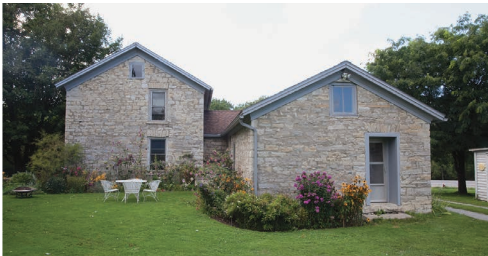
10.26. The David Dodge House from the rear shows the gable ends of the two-story house and that of the rear ell.
