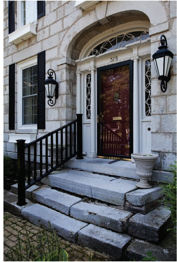
3.3. Hungerford Mansion. The elegant Federal style entrance has attached Ionic columns and delicate tracery in the fanlight and sidelights.
