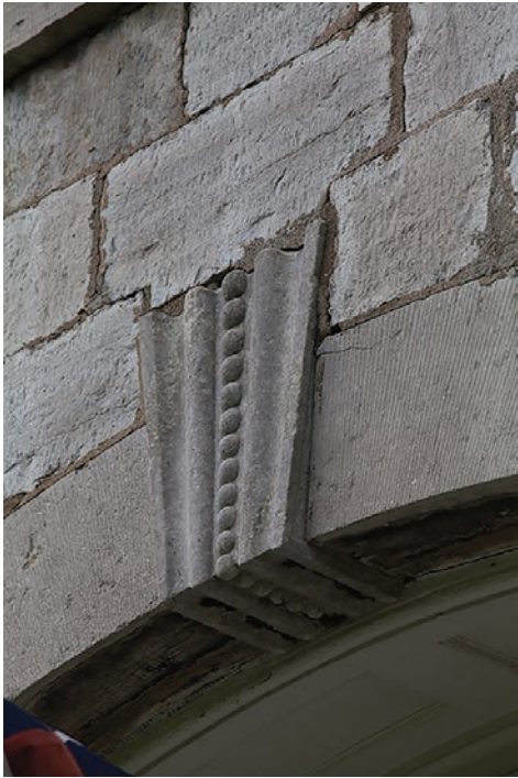
1.4. Hiram Hubbard House. Detail of beading on the keystone over the doorway.
