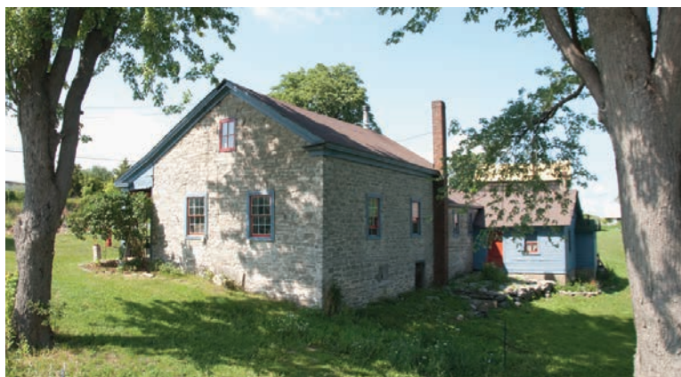
10.15. The gable end and rear view of the Reuber Dye House shows its placement in the landscape.
