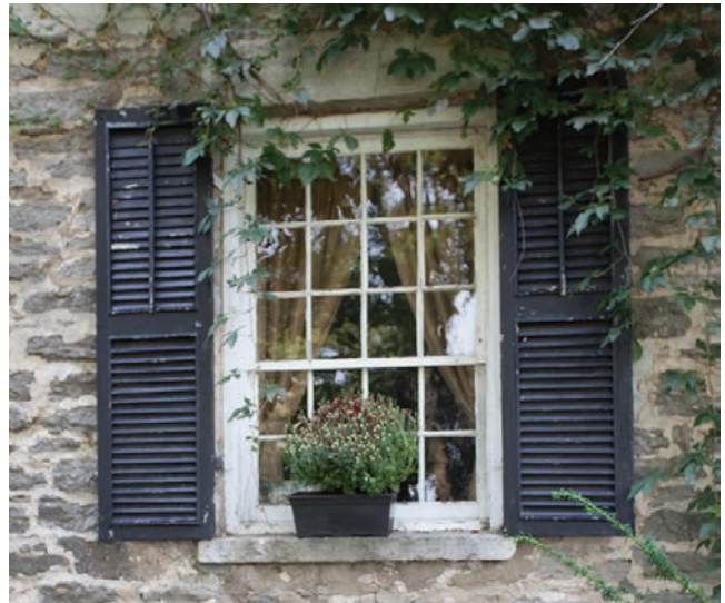
1.14. Original 12/8 window in the kitchen of the Asa Gates House.
