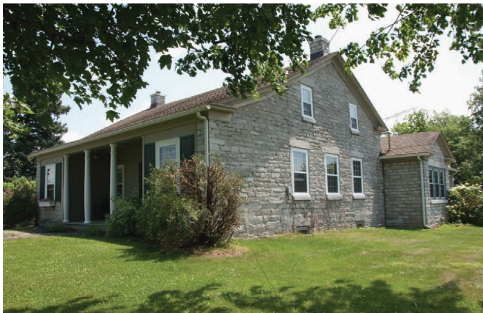
10.22. The Eber Kelsey House, 1832, was built by an early settler and land agent. Its one-and-a-half stories are of rough cut stone with smooth lintels and sills.
