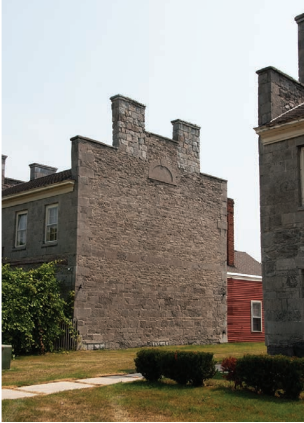
7.9. Stone Row: sally port with date inscription “Commenced Aug. 1, 1816. Completed Oct., 1819.” Iron brackets remain that would have supported two sets of large wooden gates at each end of the port.
