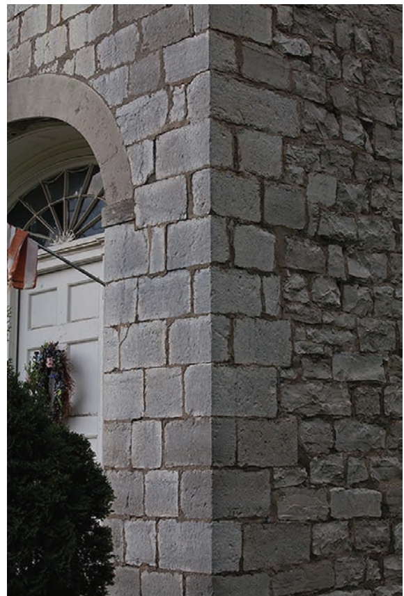
1.3. Hiram Hubbard House. Corner of Hiram Hubbard house showing the dressed stone of the front and the coursed stone of the side.
