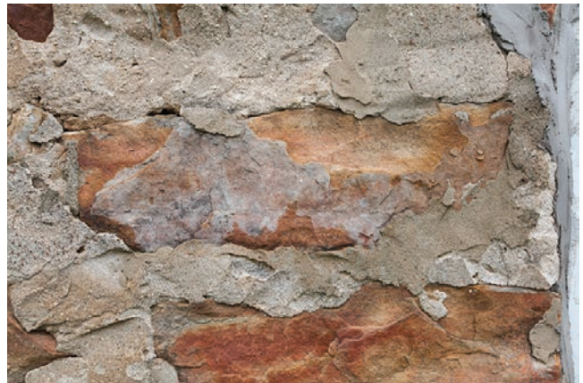
14.5. Detail of the sandstone in the Ostrander House.
