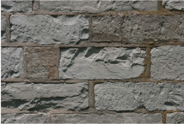
10.4. Stone House: detail of regularly coursed limestone of even height.
