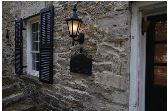
1.10. Front of the Asa Gates House showing rubble stone construction.
