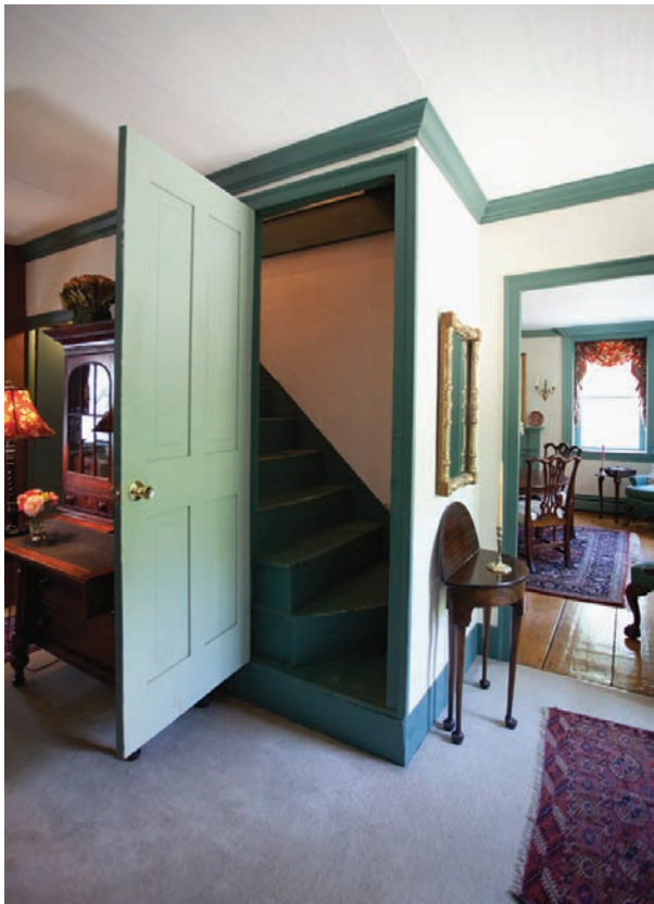
3.11. The Ballard, Denny House's enclosed interior stairway and panel door.
