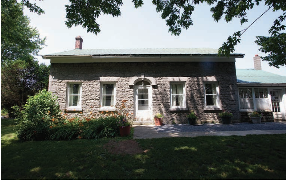
6.13. The Oliver Bates House, c. 1820, is known for its association with Mormon missionaries. Like other one-and-a-half-story houses in the area, it has a narrow entrance topped with a hemispherical arch and keystone.
