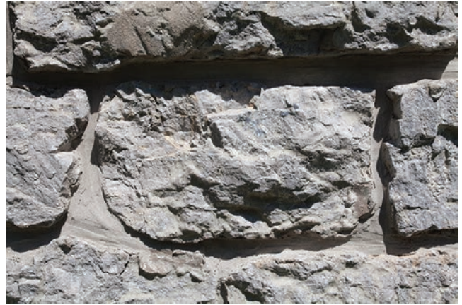
3.16. Rough coursed stonework on the south side wall of the Losee House.
