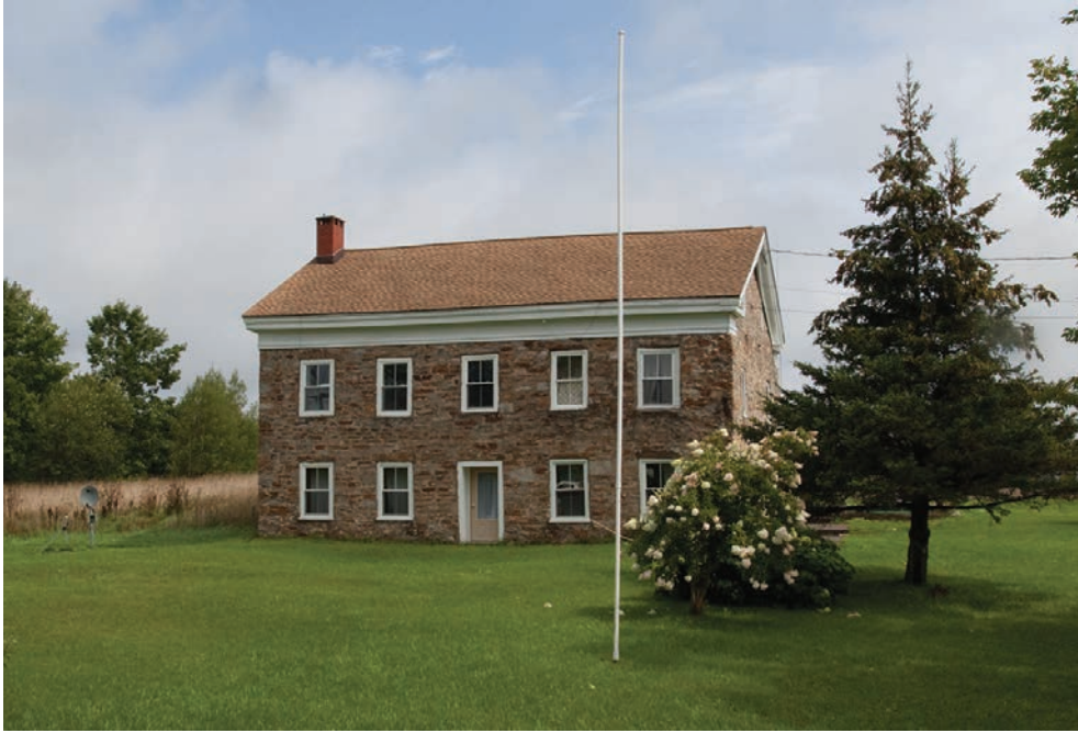
14.3. The Ostrander House, 1830s. Its original owner is unknown, but the house is a landmark in the Theresa area.
