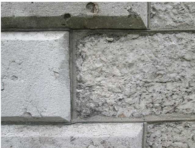
19.4. The Black River Group, Chaumont Formation: the Copley, Adams, Duford Stone Office, Chaumont. The stone on the left is beveled and worked more finely than the stone on the right.
