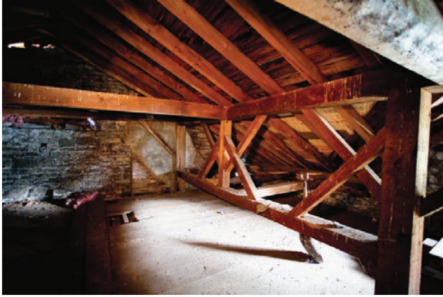
2.11. Queen post roof structure of the Felt Mansion
