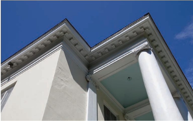
16.3. The cornice of the LeRay Mansion with its decorative modillion blocks.
