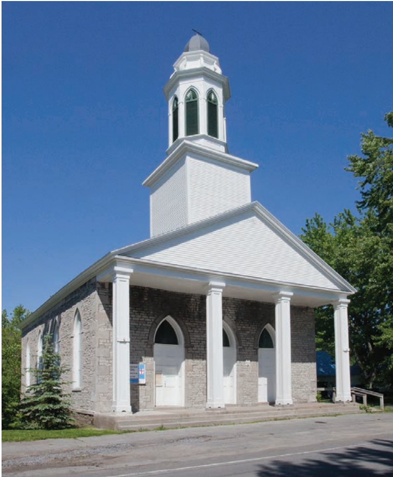
7.17. Christ Episcopal Church, built between 1823 and 1832, is one of Jefferson County's earliest churches and represents the determination of its congregation. The stone building is enhanced by a wooden-columned portico and belfry. Its pointed Gothic revival windows have smooth quoins set against a rubble stone wall.
