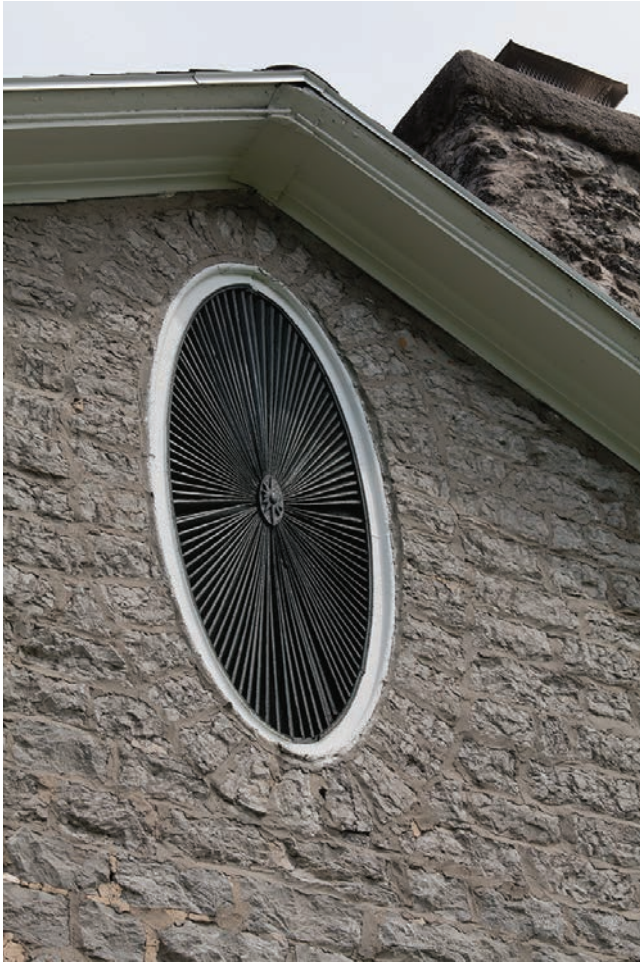
6.4. Each gable end of the Burnham House has a louvered oculus set within voussoirs.
