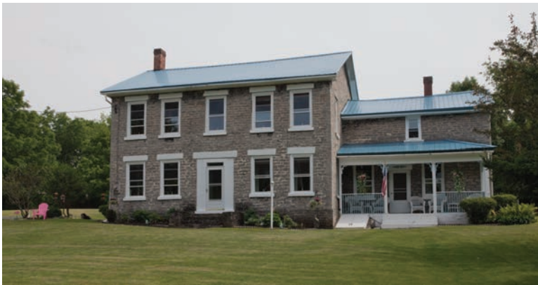
6.2. Painted lintels on the Weeks House accentuate the symmetry of the façade. A porch on the side ell provides a sheltered outdoor area in this early stone house.
