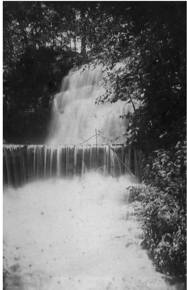
4.3. Talcott Falls in the late nineteenth century, showing the surge of water that provided power. The dam for the sawmill extends across the base of the falls. Edward Greene family scrapbook.
