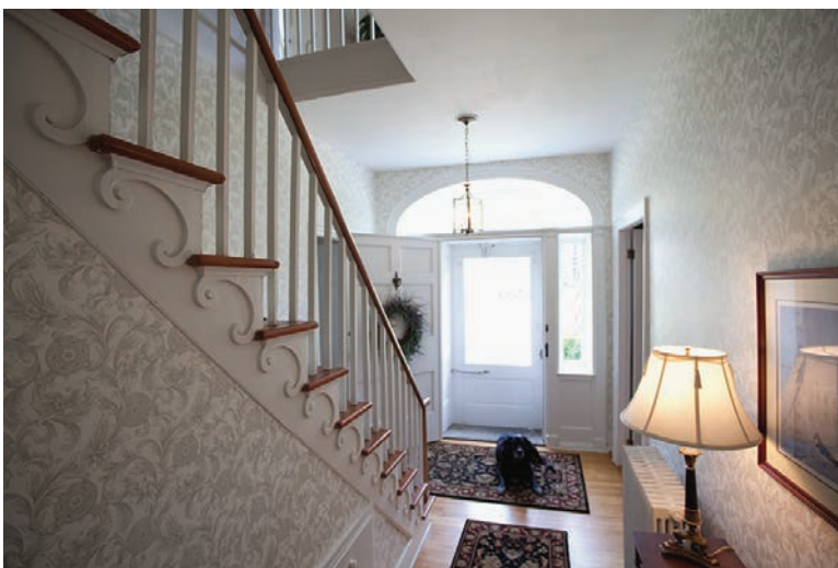
6.5. The Burnham House center stairway may have been built by a ship’s carpenter who applied carved detailing to the stair ends and a series of drawers to maximize the space underneath.
