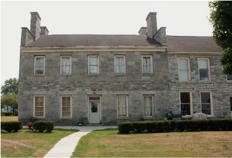
7.11. Stone Row, end house with stepped gables adjacent to the sally port. Here, the stonework of the front is ashlar. It is laid uniformly on the first floor, with a rubble section and more ashlar above what was a portico. Note the differences in stonework from the adjacent officer's house, which is possibly of quarried cut stone from Chaumont.
