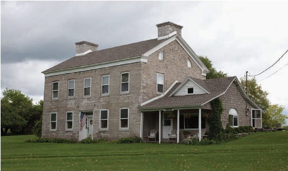
9.10. Ryder House, 1820. Built by an early settler, the house's five-bay façade and deeply recessed front entry look over Chaumont Bay. It sits on bedrock, without a cellar.
