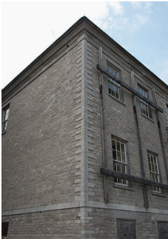
7.13. The stonework in the hospital is exemplary, with corner quoins perfectly aligned up the two stories of the building. Above is a stone cornice, and below, a well-defined watertable.
