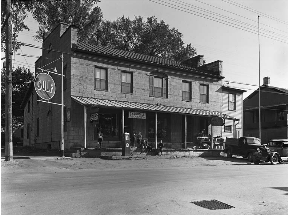
16.7. The Hoover Tavern, 1821, is an example of the fine stone work of mason Josiah Fuller. It boasts smooth ashlar blocks of Black River limestone, and stepped gables. This photograph of its use as a gas station was taken by David F. Lane for the Watertown Daily Times in 1944.
