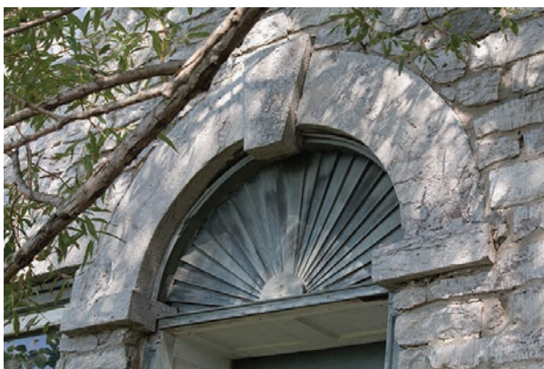
4.9. A semicircular arch with keystone tops the front entrance of the Austin Robbins House.
