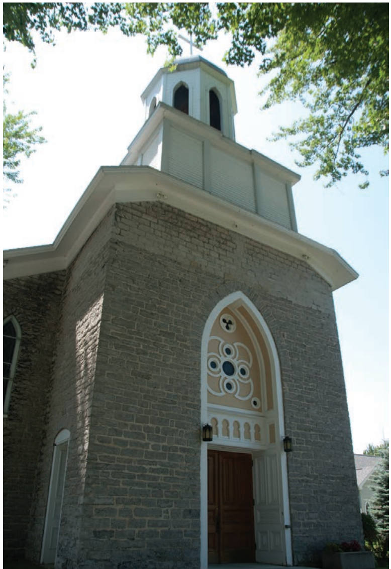
10.5. St. Vincent of Paul Church, 1851, was built by stonemason Ignatius Wiley, a German immigrant who is noted for construction of several buildings in Cape Vincent.
