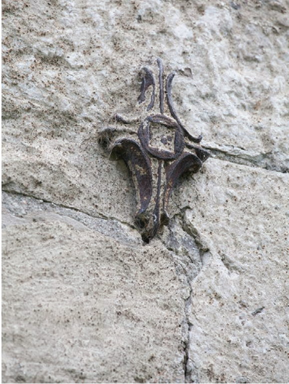
9.13. An iron detail surrounds a rod reinforcing the Ryder House.
