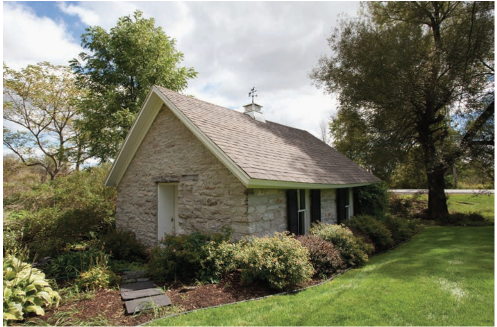
8.6. The Henry Brown Mansion's springhouse with its double stone wall bestrides Philomel Creek. It was used for keeping milk cool, separating cream, and making butter.
