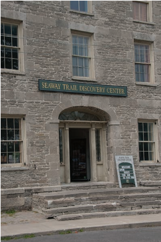
7.3. Union Hotel: coursed stonework with ashlar quoins at the corners and around the windows, and a belt course above the first floor windows.
