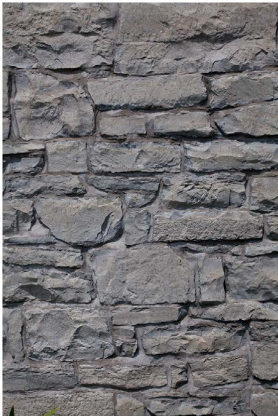
17.5. Detail of Pamela limestone of the Black River Group, side of the Parrish House.
