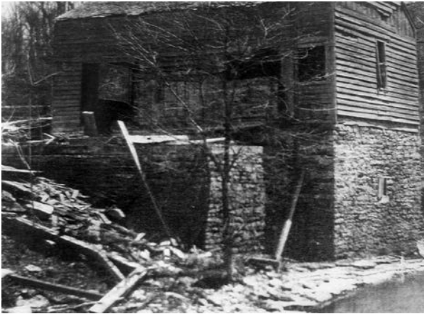
4.4. Remains of the mill at Talcott Falls with its stone foundation and wooden upper portion. Edward Greene family scrapbook.
