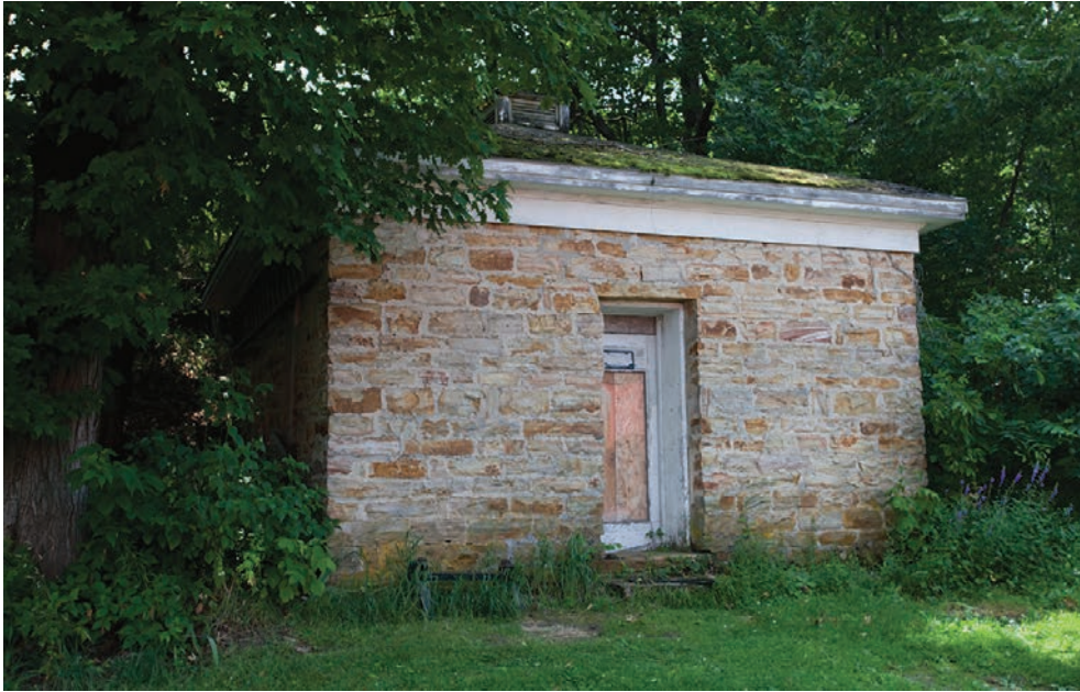
14.9. The Theresa Jail's history is unclear, but it is a small, solid structure of local sandstone.
