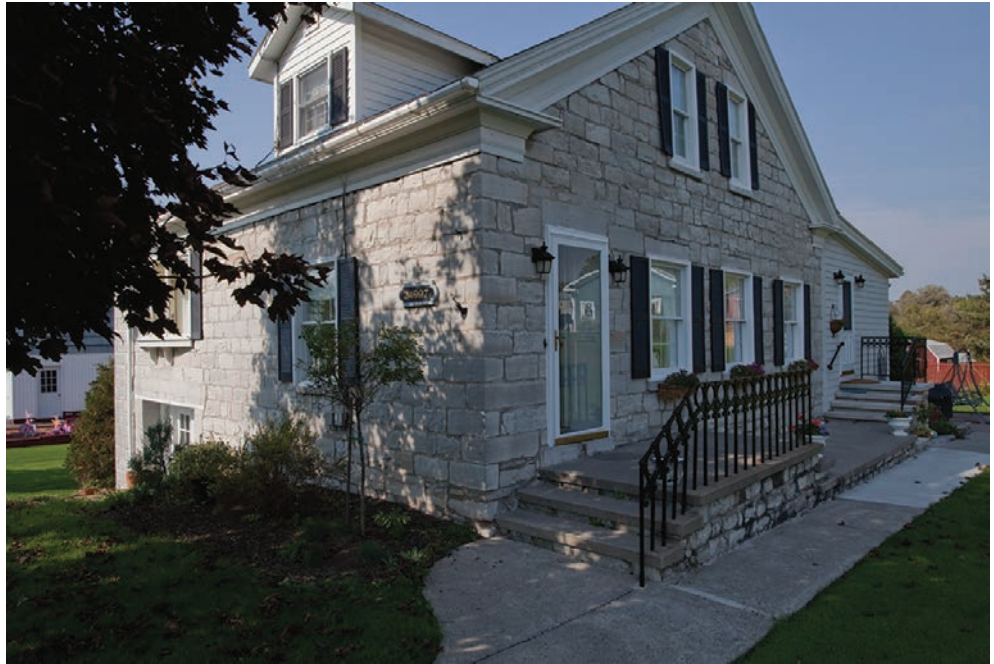
17.10. The Absalom House residence, 1830s or 1840s, is a small cottage in the cluster of stone buildings at Pamela Four Corners.
