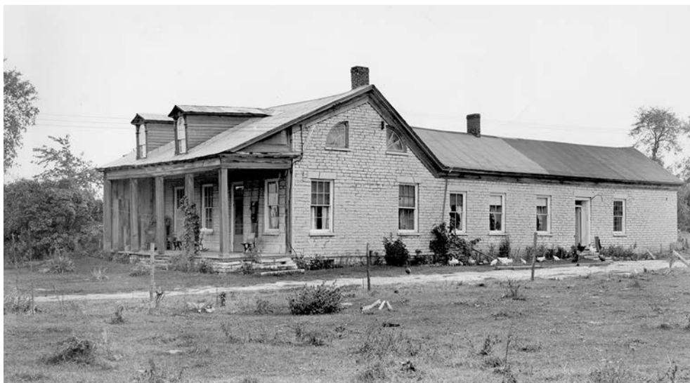
18.4. The North wing and ell of the La Farge Mansion housed the kitchen with a large bake oven, servants' quarters, and woodshed. David F. Lane for the Watertown Daily Times , December 4, 1941.
