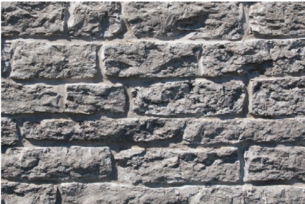
5.4. The Salisbury House was built of Coburg limestone of the Trenton group brought by oxcart from nearby Sandy Creek. The similar-sized stones are very evenly laid.
