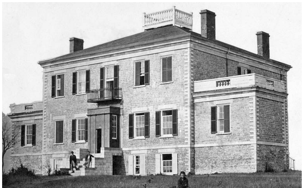
7.12. Hospital, west entrance, 1838. It is possible that the stone to build the hospital was brought by barge from Chaumont. The lighter-colored smooth cut stones of the quoins, lintels, and water table contrast well with the evenly coursed rougher stones. Photograph from the 1860s.
