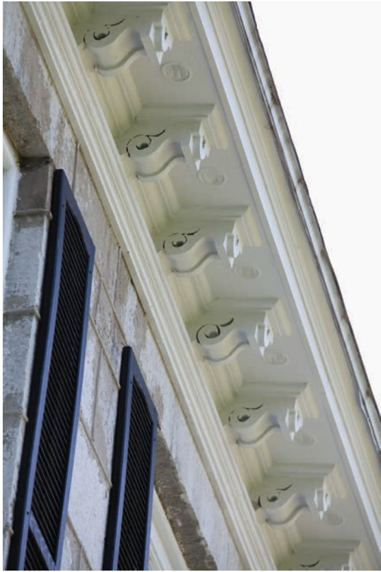
3.4. Hungerford Mansion. The cornice features intricate scroll modillions.
