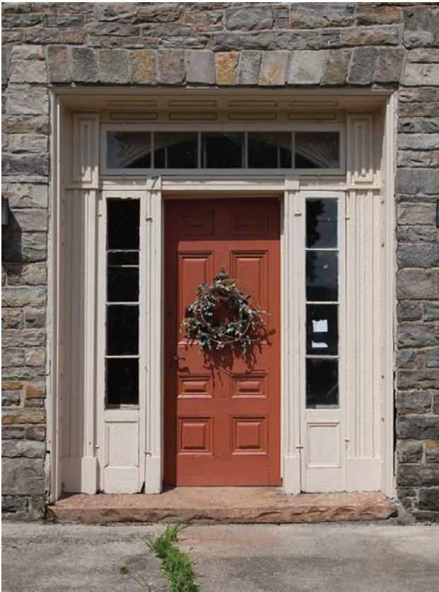
15.2. The Copeland House entry is broad with transom light and side lights. The voussoirs are short, stout blocks of stone.
