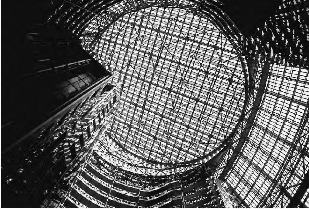
Figure 12.5c General view of atrium drum with wall-climber lifts and stairs
