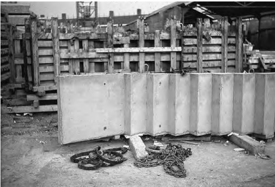
Figure 8.3a Pre-cast stairs: Site factory at Wates Housing Development
