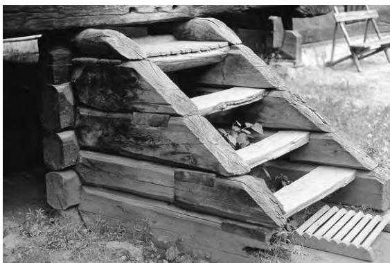
Figure 6.1a Ladder steps made from planks, circa twelfth century, Norway
