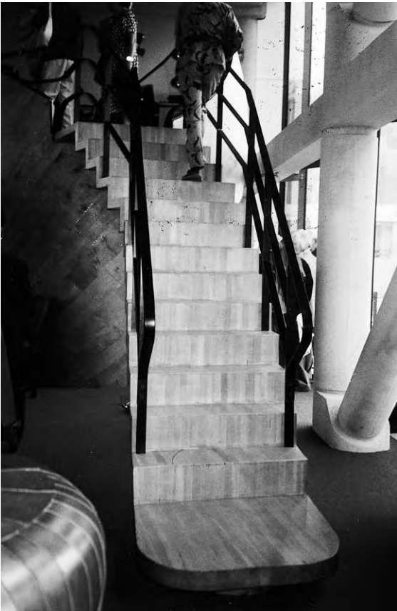
Figure 13.5b General view of stair
