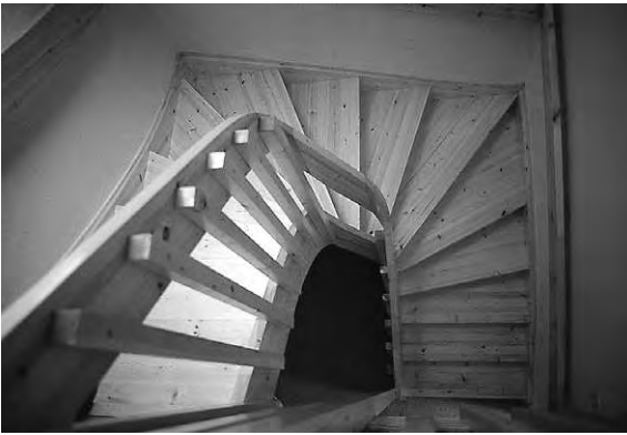
Figure 4.4 Standard Danish Stair installed in the 'Marchesi' system built house (1981)
