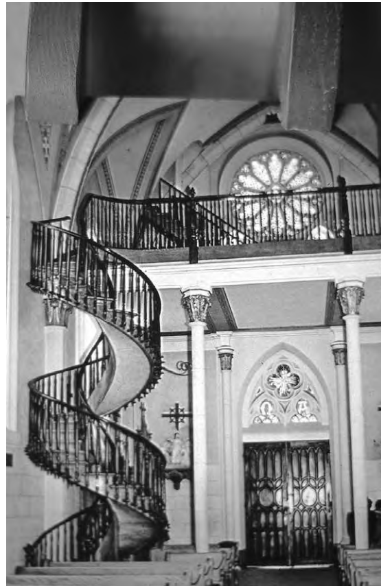
Figure 6.1d Spiral stairs, called the Miraculous Stairs, built without nails, 1878, Our Lady of Light Chapel, Santa Fe, New Mexico
