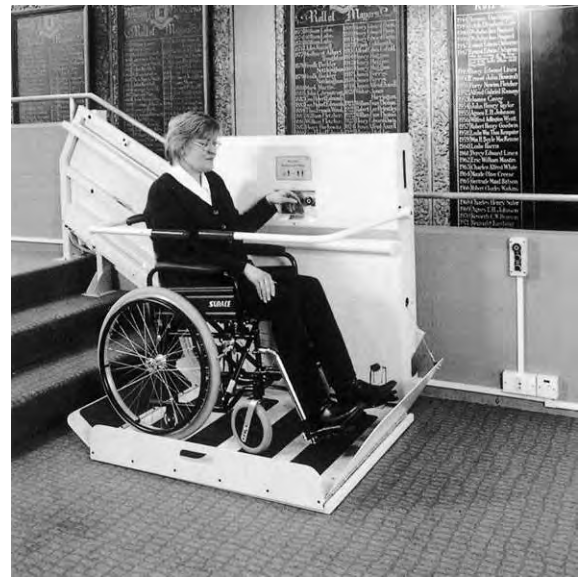
Figure 11.9c Stair lift for wheelchair
