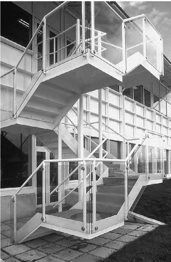
Figure 7.2c Typical tubular framing to support landings of dog-leg stairs, offices at Stockley Park, 1989, Architects: Arup Associates
