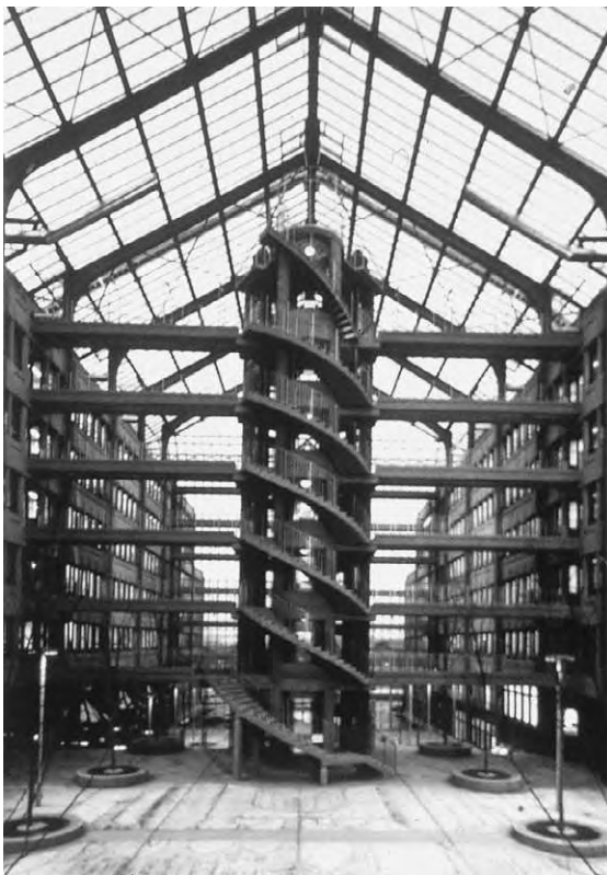
Figure 2.22b Zublin-Haus: Free-standing screen of lifts and stairs in central space
