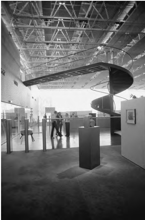
Figure 7.5b Spiral stairs, Sainsbury Arts Centre, Anglia University, 1977, Architect: Foster and Partners
