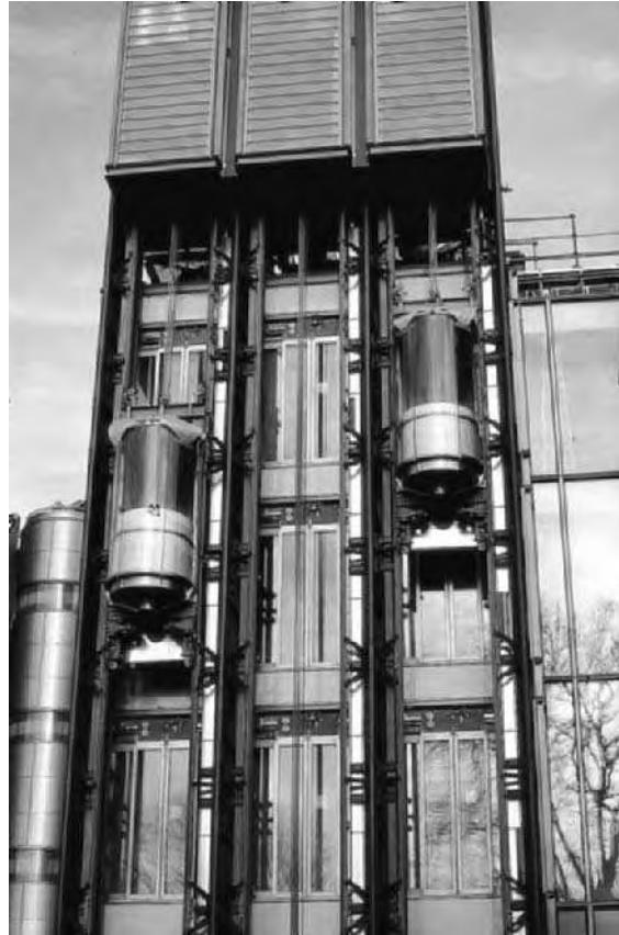
Figure 11.5b External wall-climber lifts, Channel 4, 1994 (Richard Rogers Partnership)
