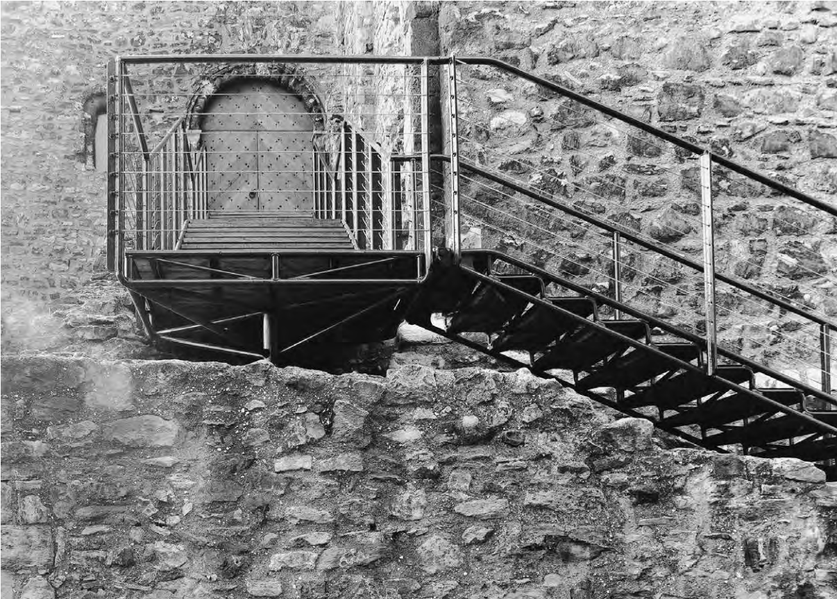
Figure 7.1c Addition of external steel stairs to Rochester Castle for visitor access, 1990, John Winter (courtesy of John Donat)
