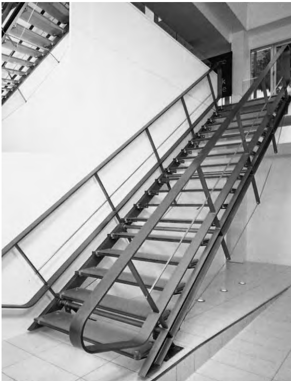
Figure 13.9a View looking up (Spiral Staircase Systems)
