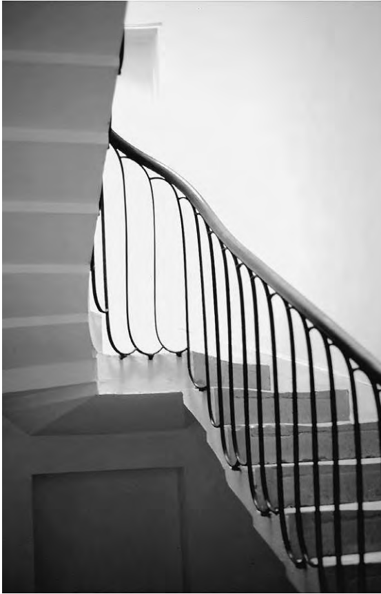
Figure 7.9a Unusual construction: Wrought iron loops, John Soane Museum, London, 1790
