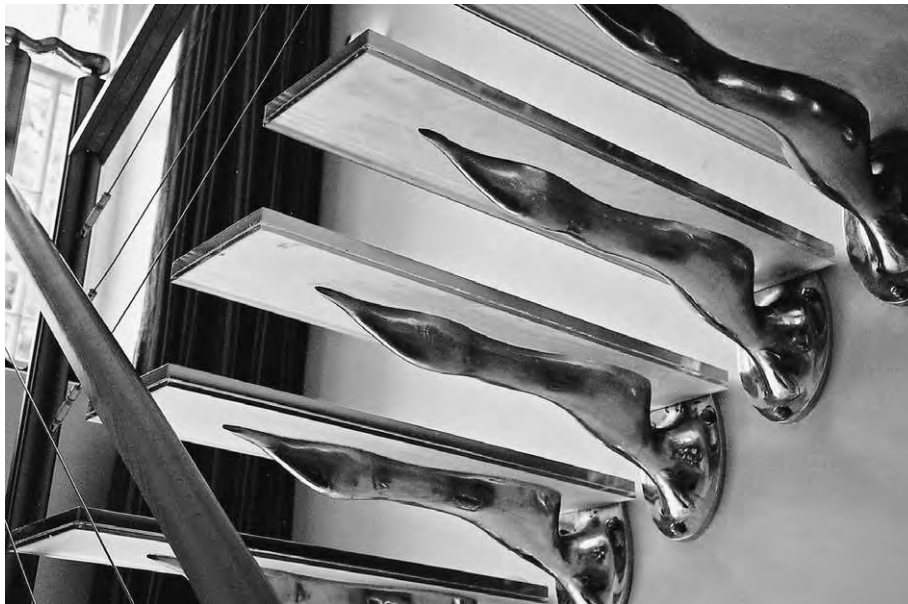
Figure 13.6b Detail of cantilever brackets
