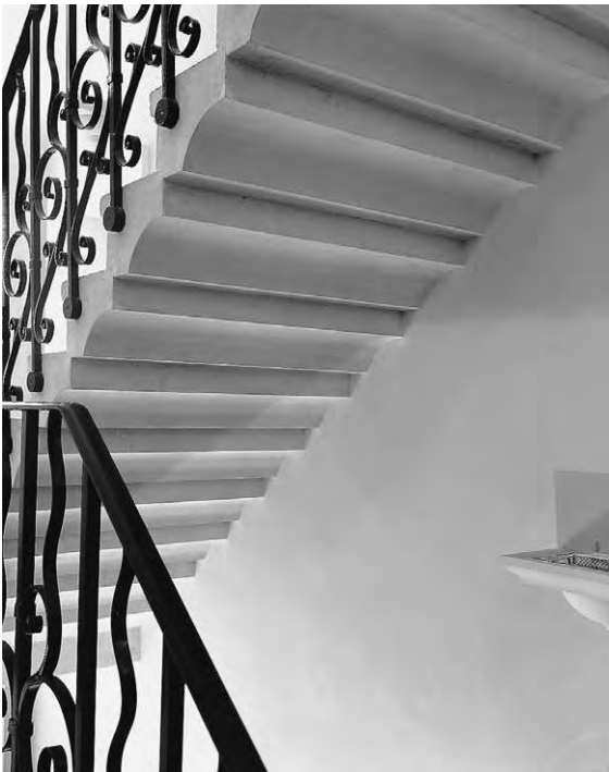
Figure 9.2j General view, Da Costa House, Highgate, 1990, Architect: Russell Taylor, Engineer: Sam Price of Price and Myers
