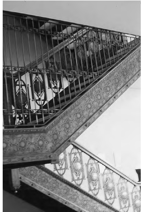
Figure 7.1b Copper coated wrought-iron stairs, Stock Exchange Building, Chicago, 1893-4, Architects: Adler and Sullivan
