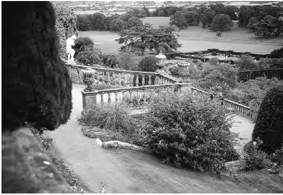
Figure 5.7d Italiante detail: Differing heights of balustrade to give greater distance, Powys Castle (date unknown)
