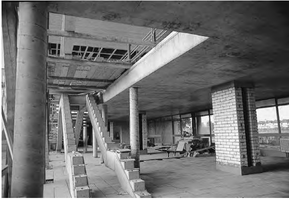
Figure 8.3b Pre-cast beam stair prepared for tread fixing
