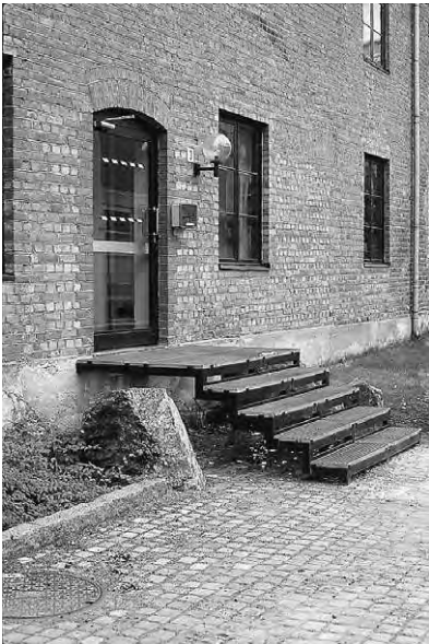
Figure 5.12c Stair platform in steel
