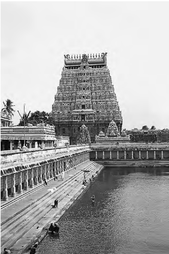
Figure 5.2a Water steps and tank, Temple at Chidambaram, India (Courtesy of Timothy Blanc)
