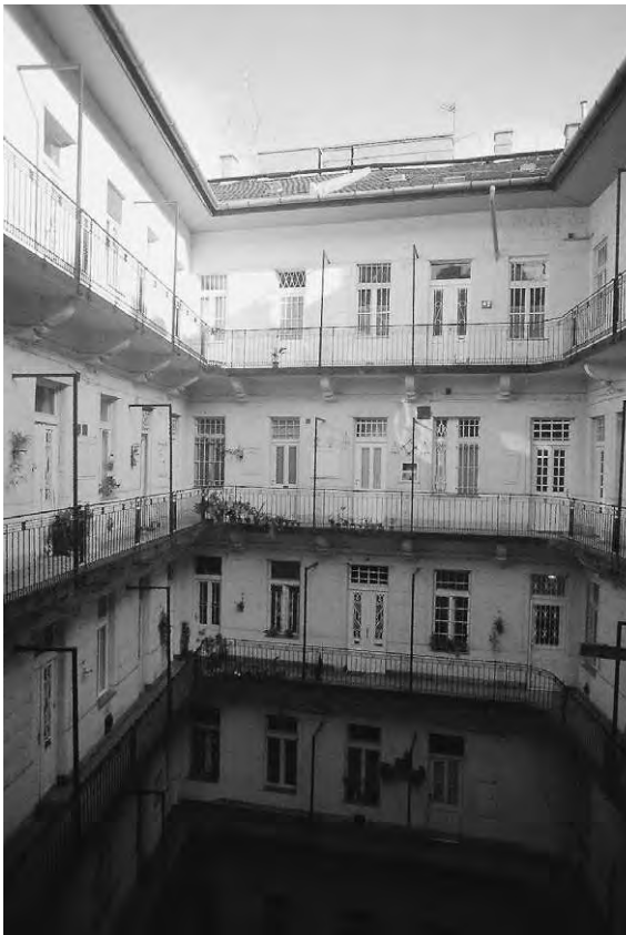
Figure 4.23 Nineteenth-century flats in Budapest on the Famillistere pattern, with balcony access and corner stairs
