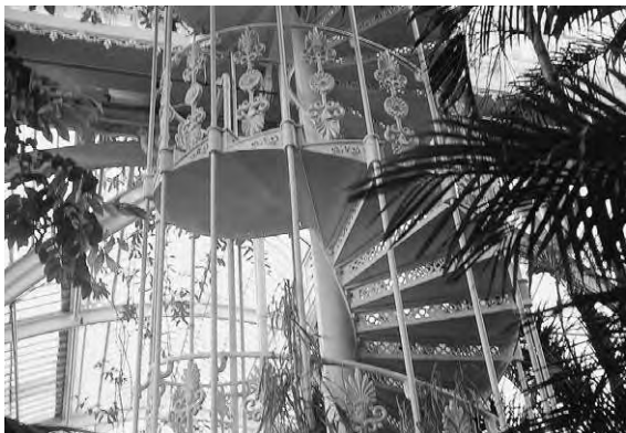
Figure 7.1a Cast-iron sectional spiral stairs, Palm House, Kew Gardens, London, 1844-8, Designers: Turner and Burton
