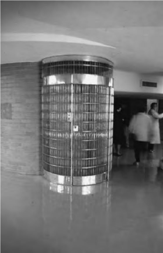
Figure 11.5a The 'bird cages' designed for screens and cars at the Johnson Building, Racine, 1936, Architect: Frank Lloyd Wright
