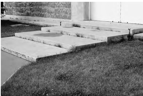
Figure 5.12a Constructional restraints upon design: Independent slab steps
