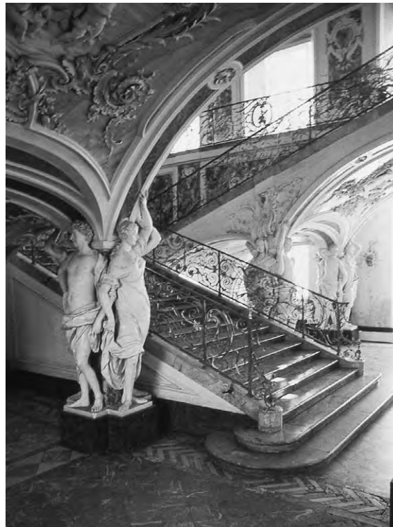
Figure 2.12d Rococo stairs, Schloss Brühl, 1748 (Neumann)
