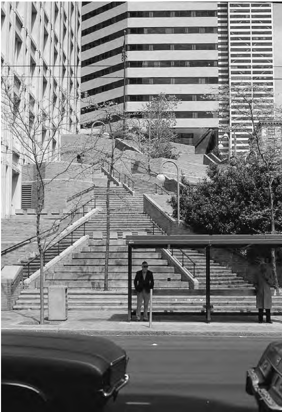
Figure 5.11b Splayed form at entry to Federal offices, Seattle, USA, 1974, Landscape Architect: Richard Haag
