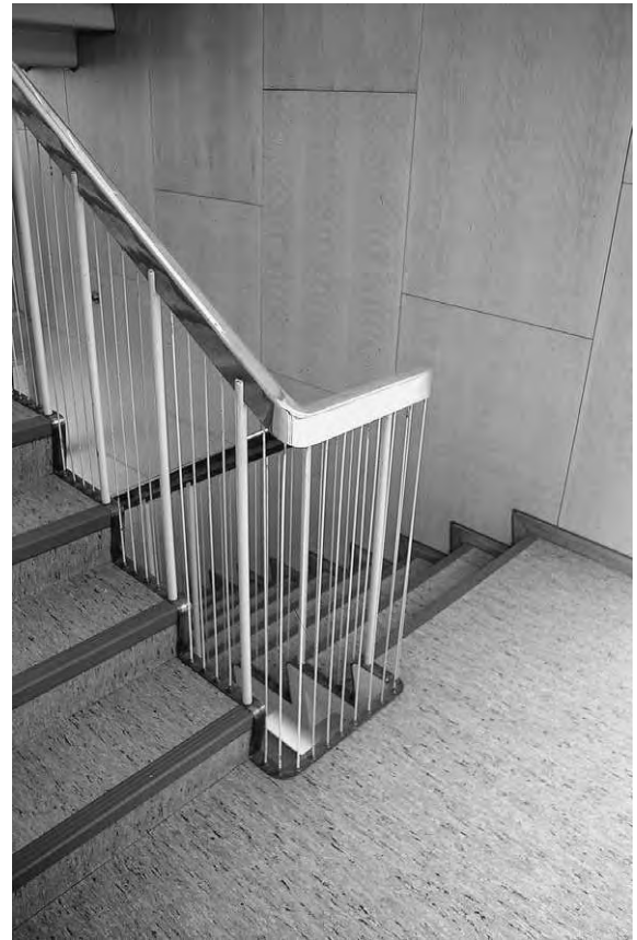
Figure 7.9b Unusual construction: Brass frame, with handrail, enamelled standards, wires as infill and capping to string, Aarhus City Hall, 1943, Architect: Arne Jacobsen
