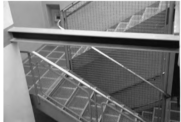
Figure 7.5d 'Nevada' glass used in treads to Maison Clarté, Geneva, 1932, Architect: Le Corbusier
