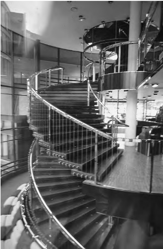
Figure 7.9c Unusual construction: Trussed balustrade with steel handrail, verticals and folded steel treads, Havas Conseil, Paris, 1960s
