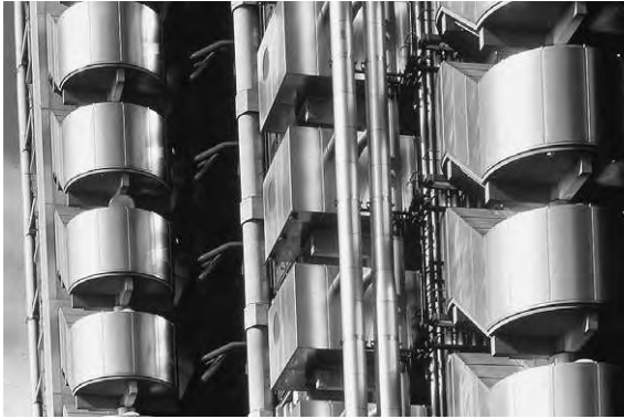
Figure 11.7a Lloyd's Building, London, 1986, Architects: Richard Rogers Partnership. External view of staircase towers
