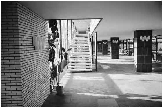
Figure 8.3c Completed work with treads and balusters in place
