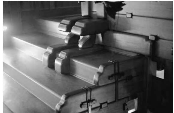
Figure 6.1b The ultimate in timber elaboration. The main stairs at the Gamble House, Pasadena (balustrade modelled on the ‘lifting cloud’ motif of Japan), 1908, Architects: Henry and Charles Greene
