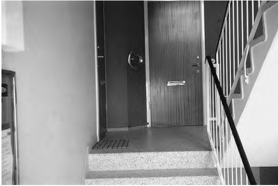
Figure 8.4b Finished tread with terrazzo surface of different colours including non-slip insets
