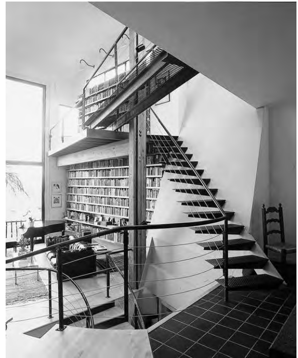
Figure 12.7 View of steel cantilevered stair from living room to library gallery (courtesy of Arcaid)
