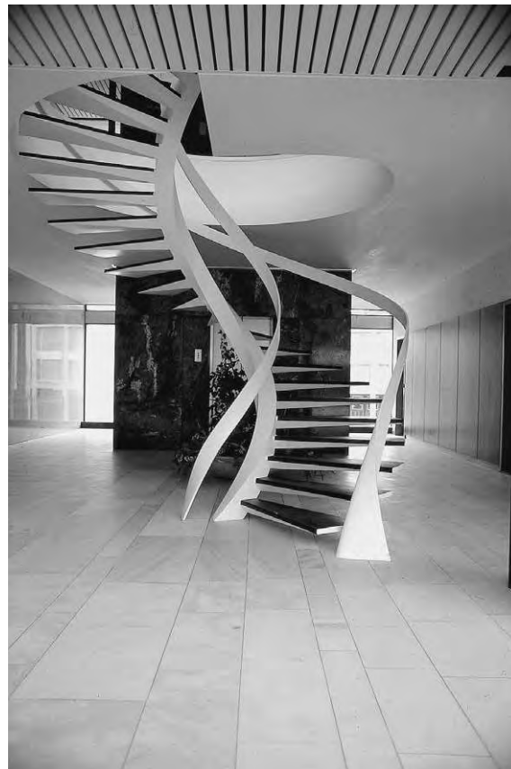
Figure 7.5a Special stairs: Welded plate to form hollow profiles for newel and for cantilever treads: accommodation stairs at City Hall, Arnhem, General view
