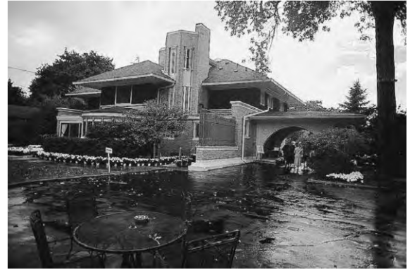
Figure 4.20 Vertical or thermometer window featured in the rear elevation of the Winslow House, Chicago, 1893, Architect: Frank Lloyd Wright
