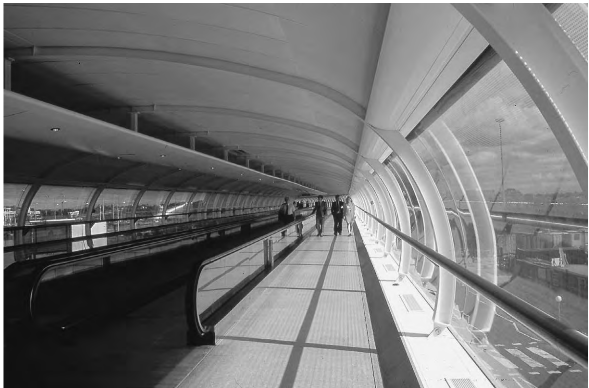
Figure 11.8b Manchester Airport's new 240 m travelator (courtesy of Paul Miller)
