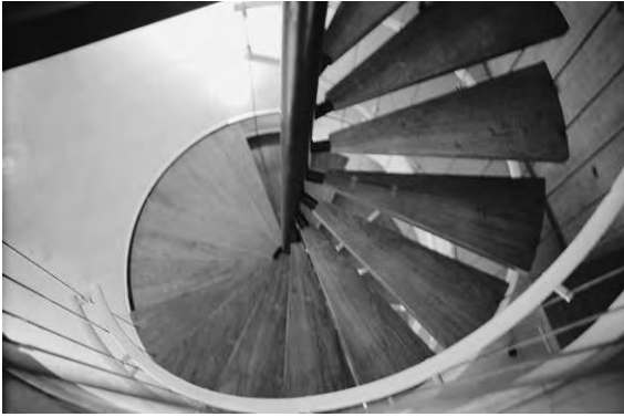
Figure 7.6d Suspended stairs: Cable suspension, former Hille Showroom, London, 1963, Architect: Peter Moro
