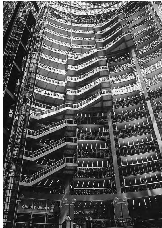
Figure 12.5b Detail view of stairs
