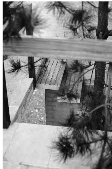
Figure 5.12b Cantilever slab stairs
