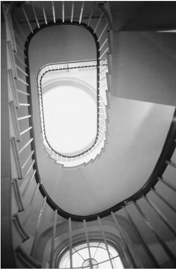
Figure 6.1c Elegant wooden flight reinforced by a wrought iron fitch within the strings (late eighteenth century), Stamford Assembly Rooms
