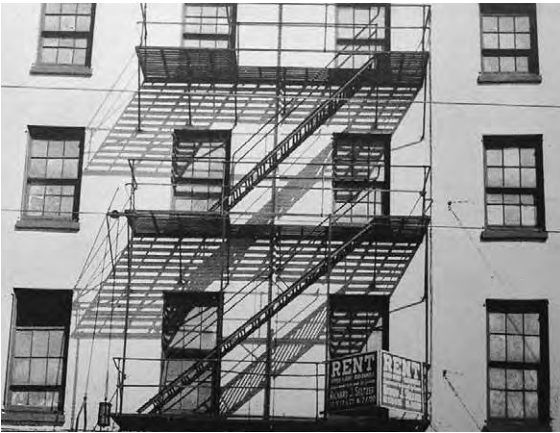
Figure 7.2b Vernacular escape stairs in USA
