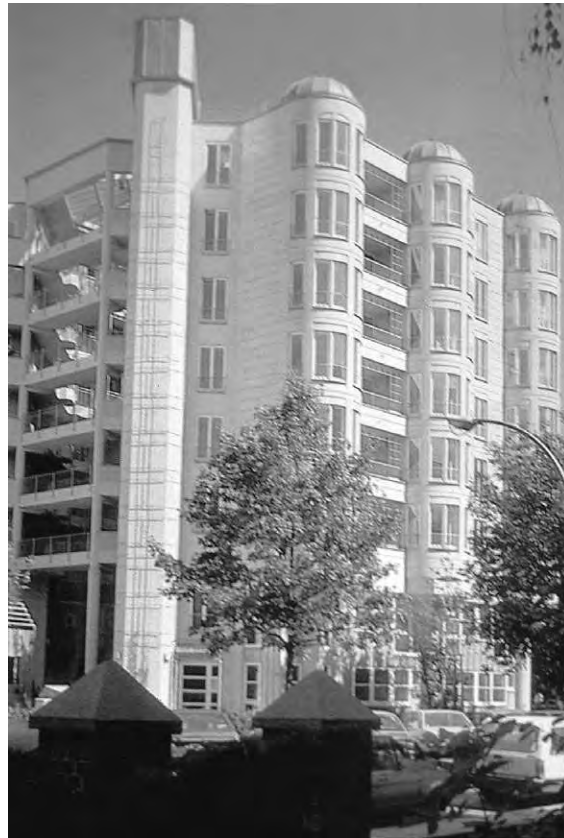
Figure 4.27 a Staircase fenestration in flats: Identification elements: Fasenenplatz , Berlin, 1984, Architect: Gotfried Bohm
