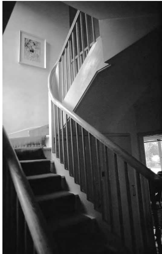
Figure 6.5d Curved framing: Curved newel to support strings and handrail, Wood House, Shipbourne, 1938, Architects: Gropius and Fry
