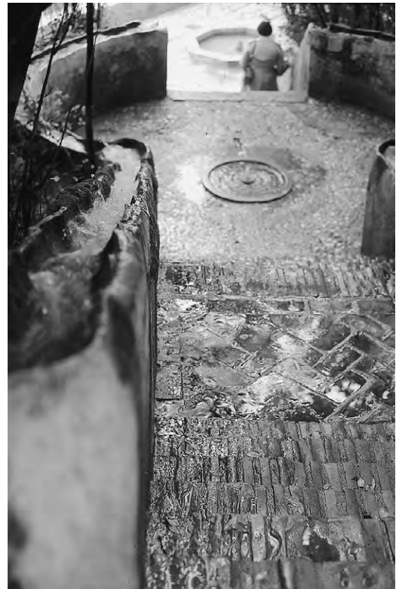
Figure 5.3 b Pebble ramps, enlivened by fountains bordered by walls having waterfall copings
