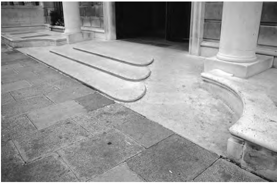
Figure 5.9c Combined pattern. New entry steps at RIBA HQ, London, 1980s, Architect: J. Carey
