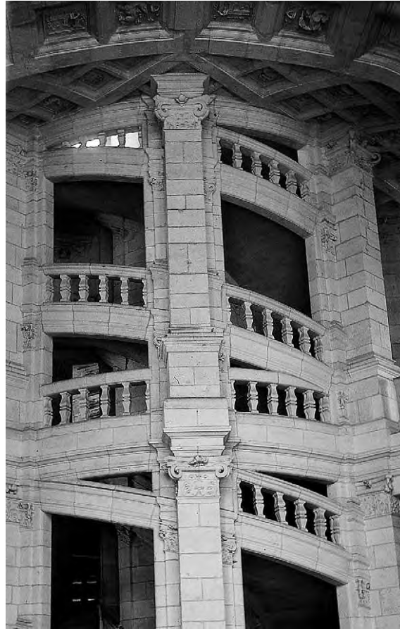
Figure 2.21a Double cylindrical stairs at Chambord, 1519–47
