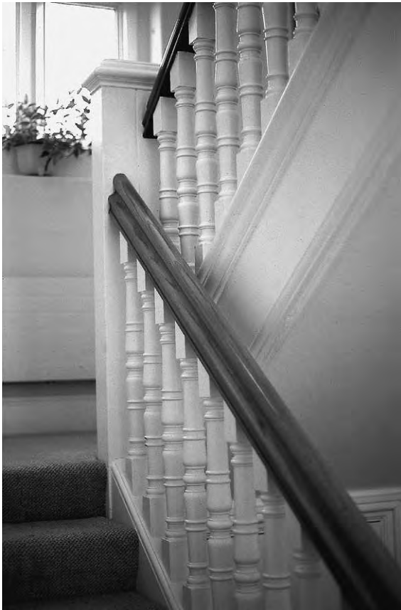
Figure 6.5e Curved framing: Traditional newel post
