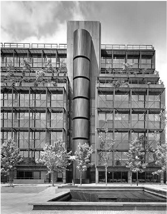
Figure 3.7c No. 1 Finsbury Avenue, City of London, 1985, Architects: Arup Associates: Façade with stair nodes expressed as towers
