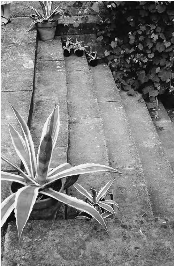
Figure 5.7e Italiante detail: Curved line of tread to improve visual effect. Renishaw, 1990s, designer: Sir George Sitwell
