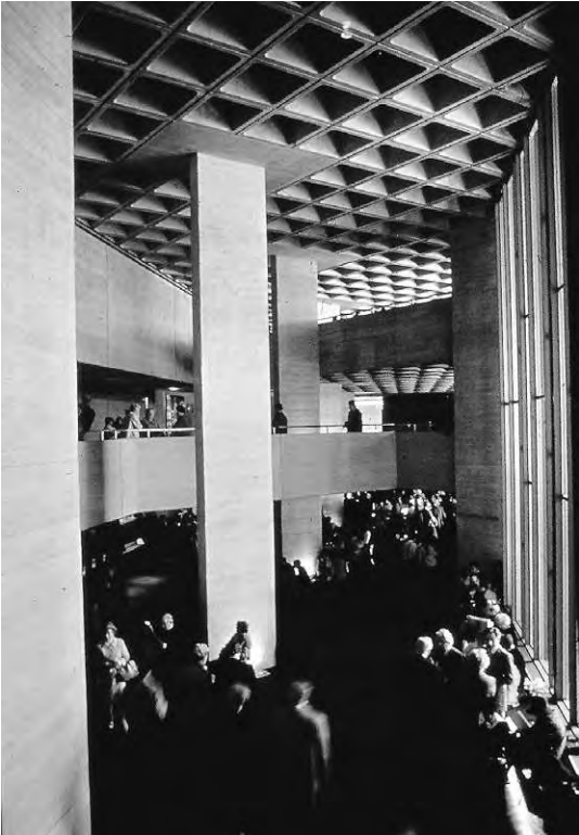
Figure 8.2f Cast in-situ concrete work to stair shafts, Royal National Theatre, 1967-76, Architects: Denys Lasdun, Redhouse and Sofley
