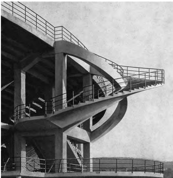
Figure 8.1d Confident use of reinforced concrete structure in stairs, Florence Stadium, 1932, Engineer: Pier Luigi Nervi
