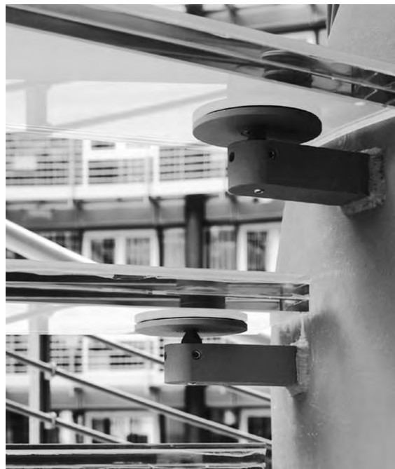
Figure 12.6c Detail of tread support
