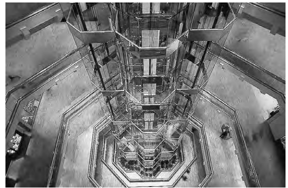
Figure 3.18b Another view of Water Tower Place
