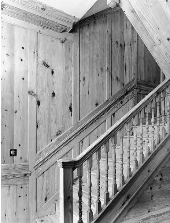
Figure 6.4b Historic examples: Replacement stair, Morton House, Highgate, London, 1990 (Julian Harrap)
