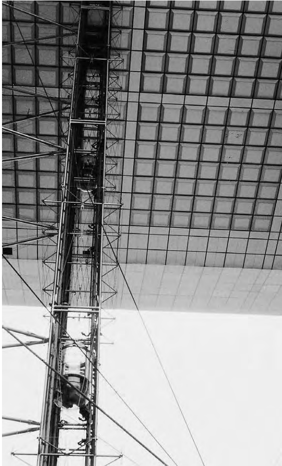
Figure 11.5g Detail view of lift construction, Le Grand Arche
