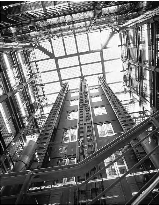
Figure 3.8c Bracken House: Steel plate towers to support wall-climber lifts (courtesy Alan Delaney, Wordsearch)
