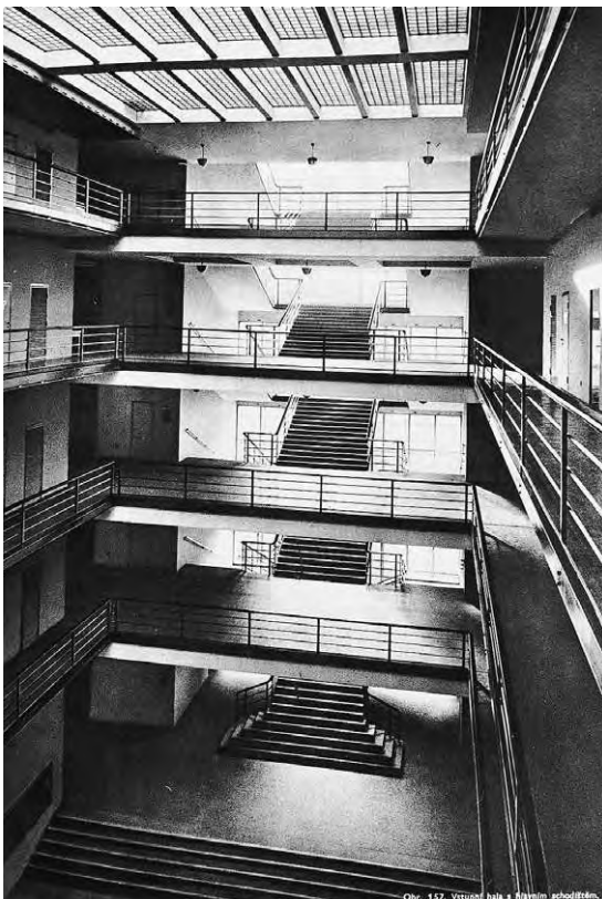
Figure 3.15 Pre-eminence of stairs, Electricity Board offices and showrooms, Prague, 1935, Architects: Adolf Bens and Josef Kriz
