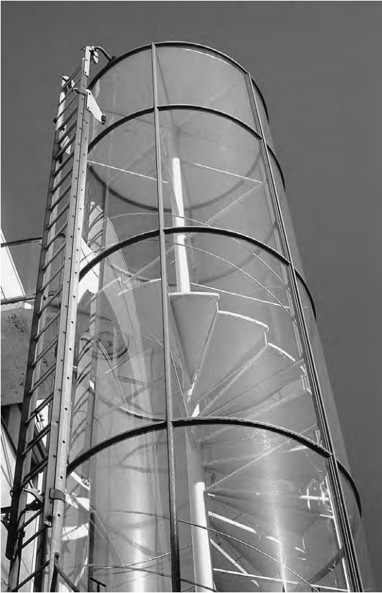
Figure 7.2f Minimal escape stairs with glass enclosure, 'Novo' factory, Copenhagen, 1961, Architect: Arne Jacobsen (Danish regulations permit spiral escapes)
