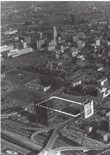
FIGURE 2 The Bunker Hill area in downtown Los Angeles 1967. Most building structures have been razed in order to make space for new superblocks. In this phase, late nineteen-sixties to early nineteen-seventies, most plots were temporarily converted into parking lots. The white line indicates the plot of the Westin Bonaventure Hotel. Photograph reproduced from Anastasia Loukaitou-Sideris and Tridib Banerjee (1998, 22).
