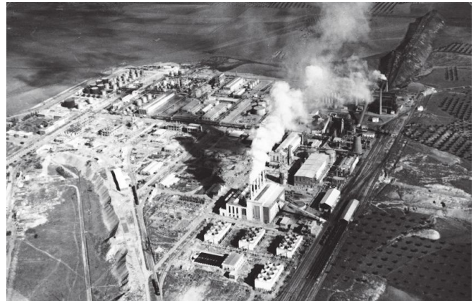
FIGURE 2 A distillery that made use of the oil shale stock (ENCASO) and a thermal plant that consumed coal were set up in 1952. In the eighties ENCASO was transformed in the present petrochemical plant.
