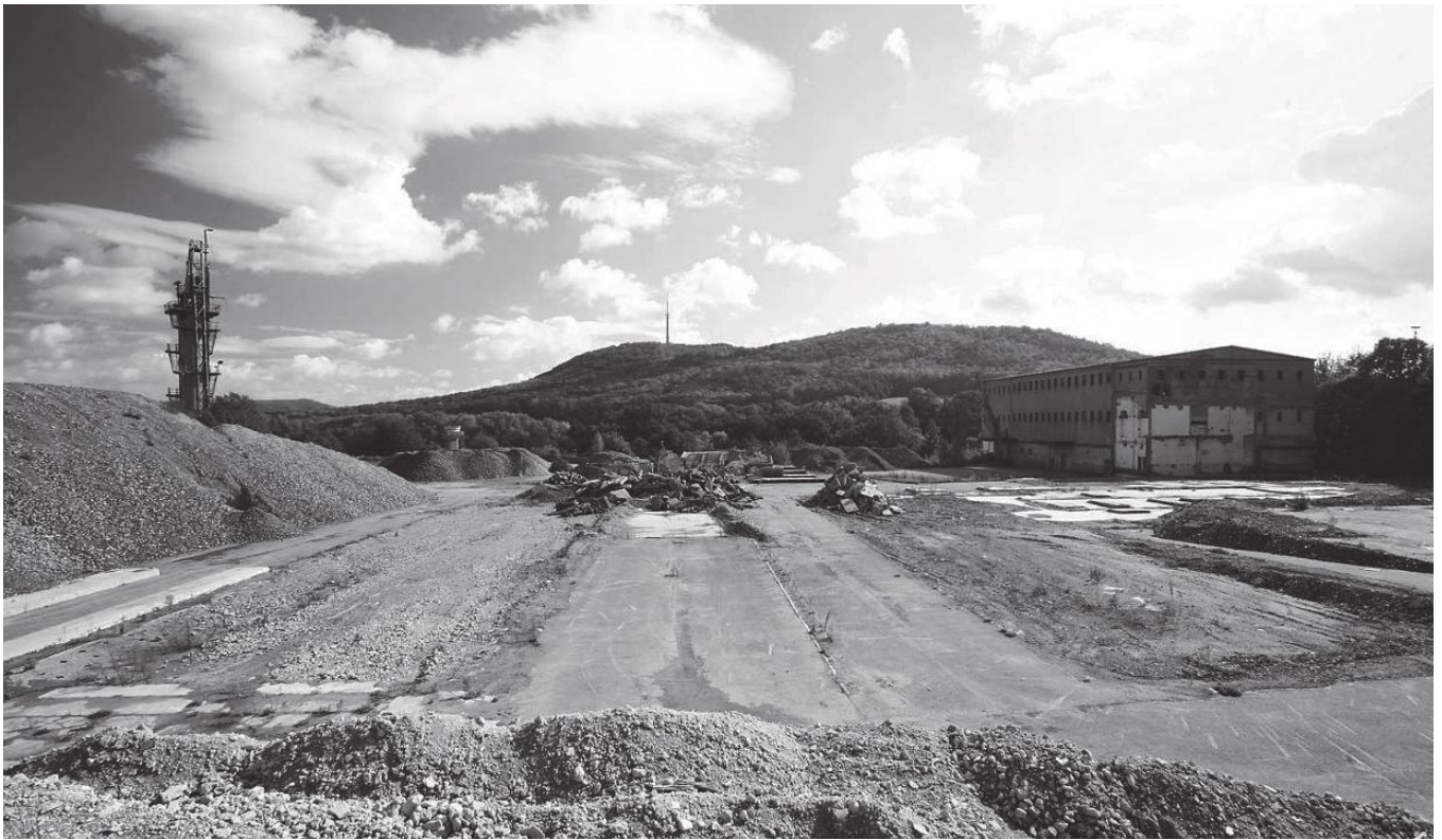
FIGURE 1 Built on sugar: sugar plateau and old storehouse
