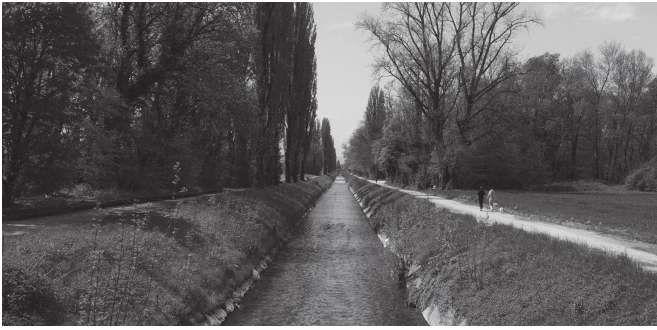
FIGURE 6 View along the concrete reinforced canal of River Aire, 2013 (author).
