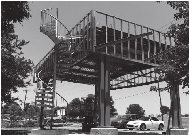
FIGURE 4 Structural steel and pavilion fascia erection (Credits: Warren Cory Gallo)
