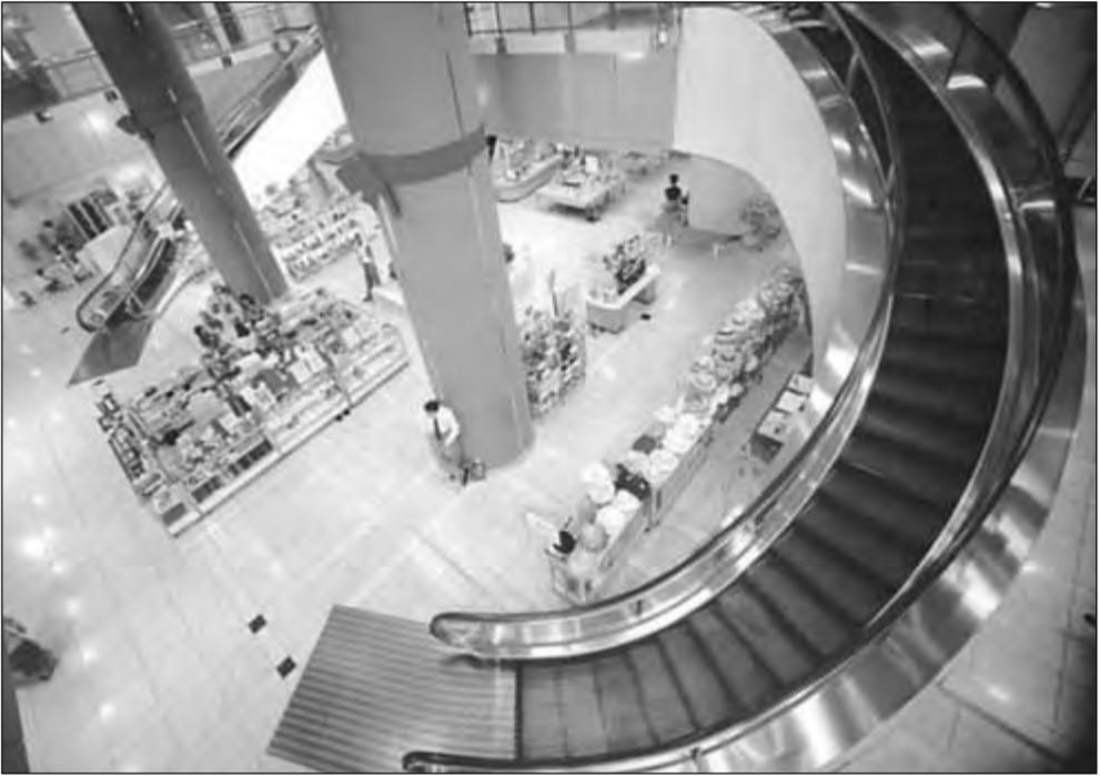
**FIGURE 11.14** A spiral escalator effectively used in the Yamako Department Store in Kofu, Japan. (Courtesy Mitsubishi Electric Corporation)
