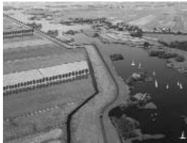
The combination of housing and water retention is worked up in detail for an area near Kamerik, near Amsterdam.
