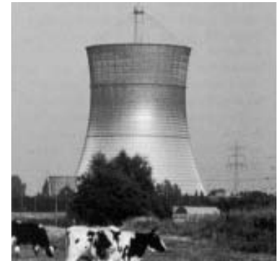
project: cooling tower of nuclear plant at Schmehausen engineers: Günter Mayr and Jörg Schlaich location: Germany year: 1974
