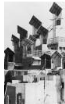
Ancient wind scoops in Hyderabad, Pakistan, channeling cool afternoon air into each room of the multi-storey housing.
